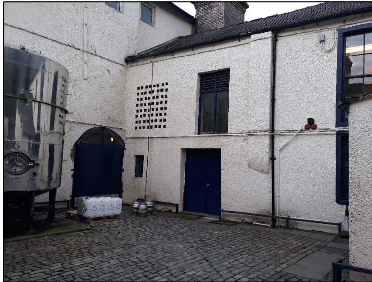
Plate 12: Doorway 7, facing south-west
