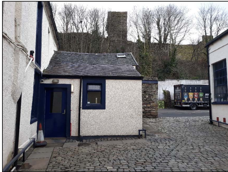
Plate 11: Doorway 6, facing north-east
