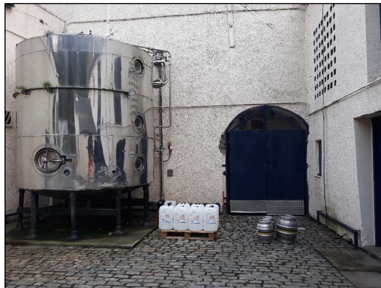
Plate 13: Doorway 8, facing south-west
