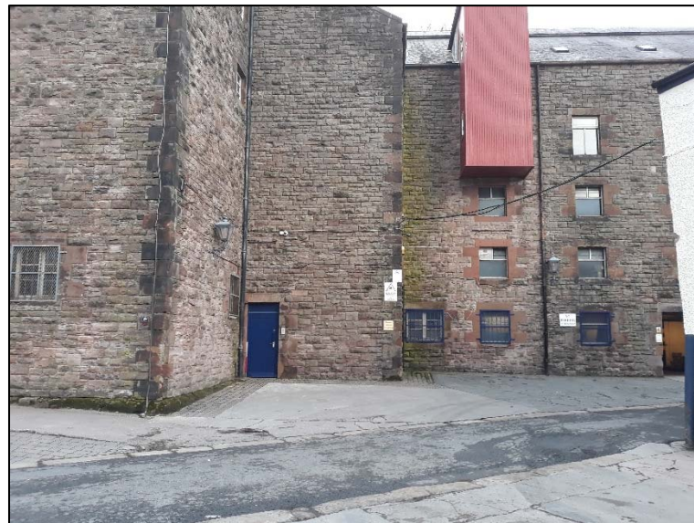
Plate 6: Doorway 2, facing north-east
