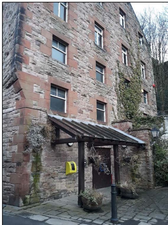
Plate 10: Doorway 5, facing north
