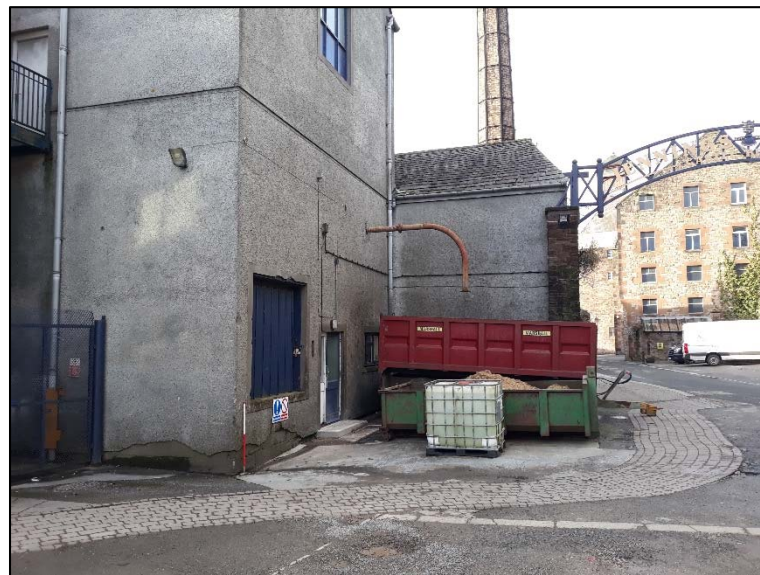
Plate 18: Doorway 13, facing west
