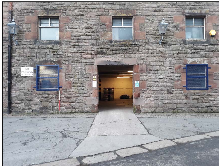
Plate 7: Doorway 3, facing north-east
