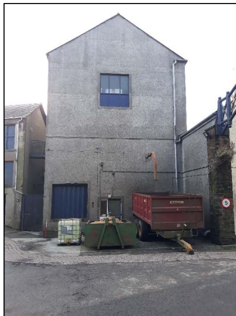
Plate 17: Doorway 13, facing south-west
