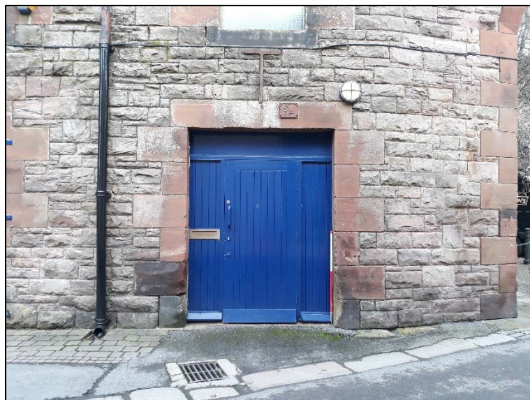
Plate 9: Doorway 4, facing north-east
