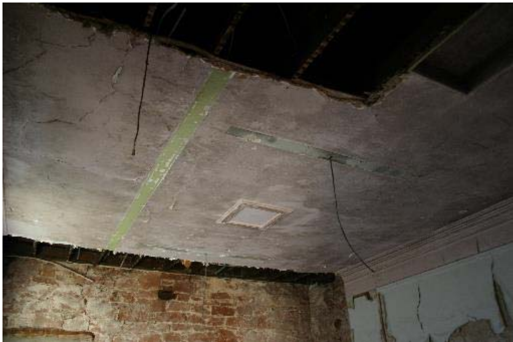
Plate 69: No 23, FF4 partially removed ceiling
