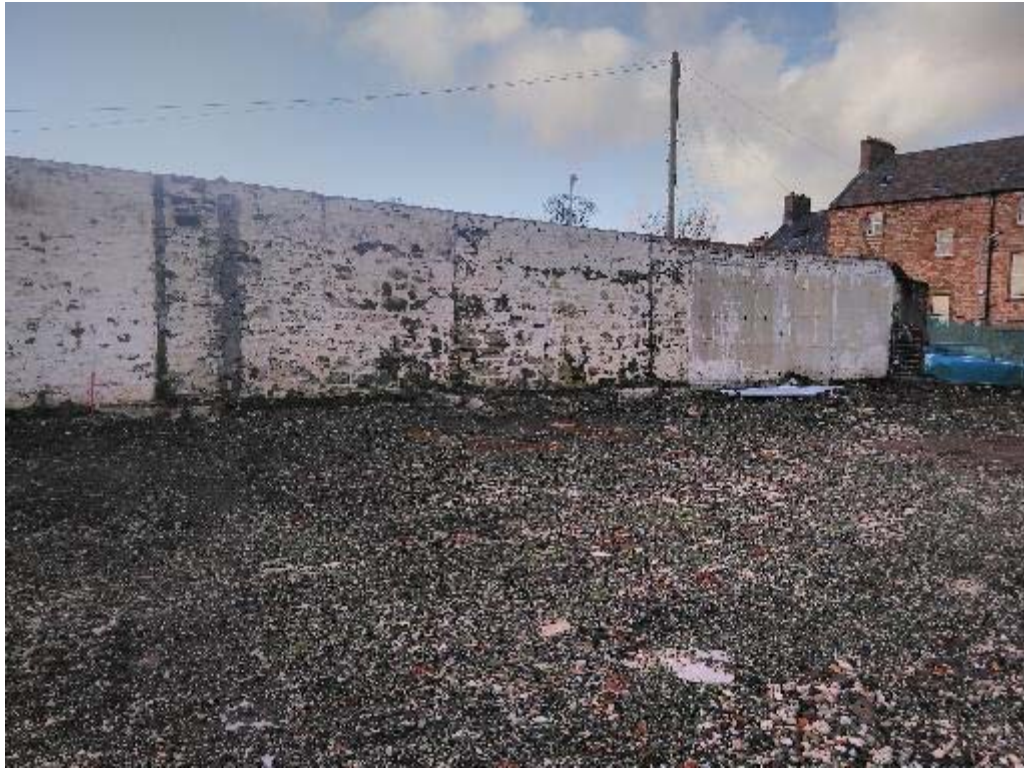
Plate 94: Northern section of western boundary wall
