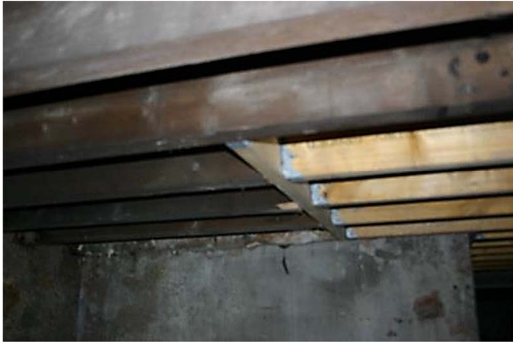
Plate 34: replacement of timbers due to rot
