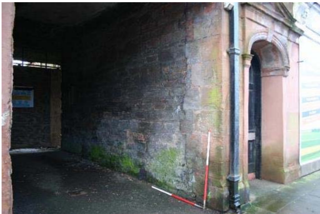
Plate 5: Driveway, east facing elevation
