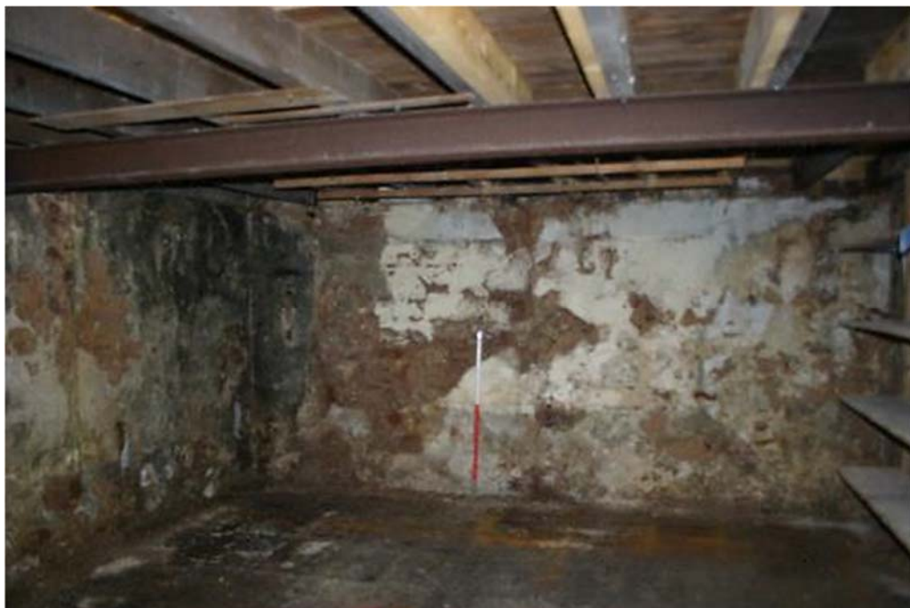
Plate 37: Northern cellar room of No 23
