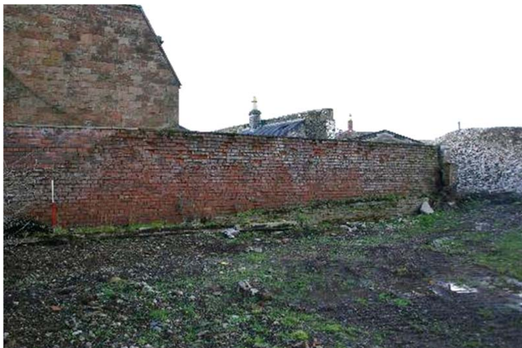
Plate 83: Red brick boundary wall of the small yard
