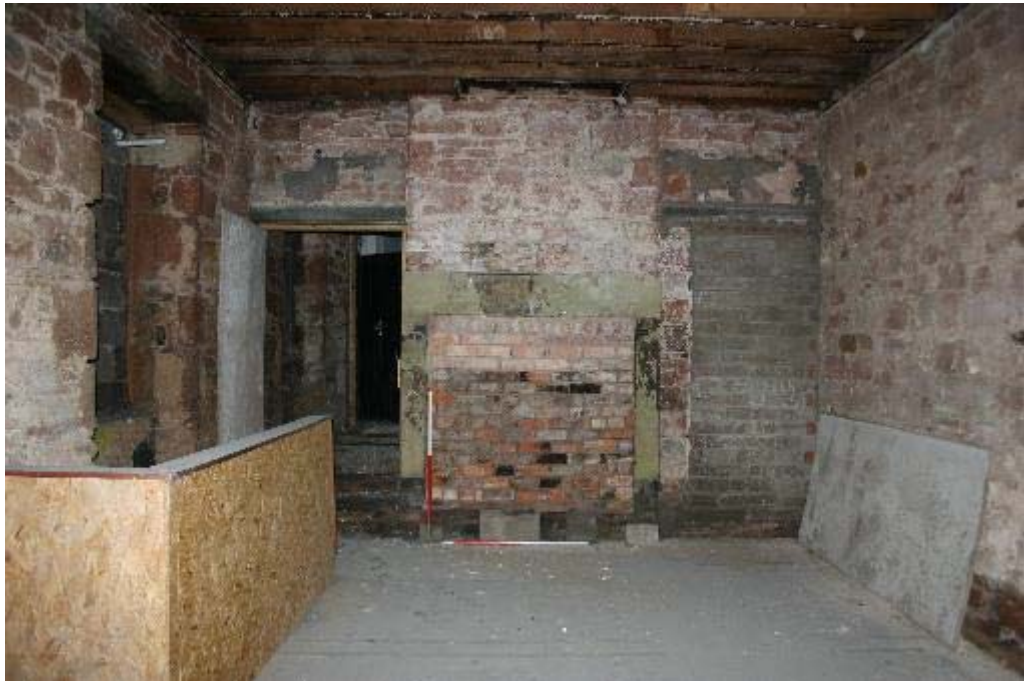
Plate 56: No 23, GF5 blocked off fireplace and doorway to GF6
