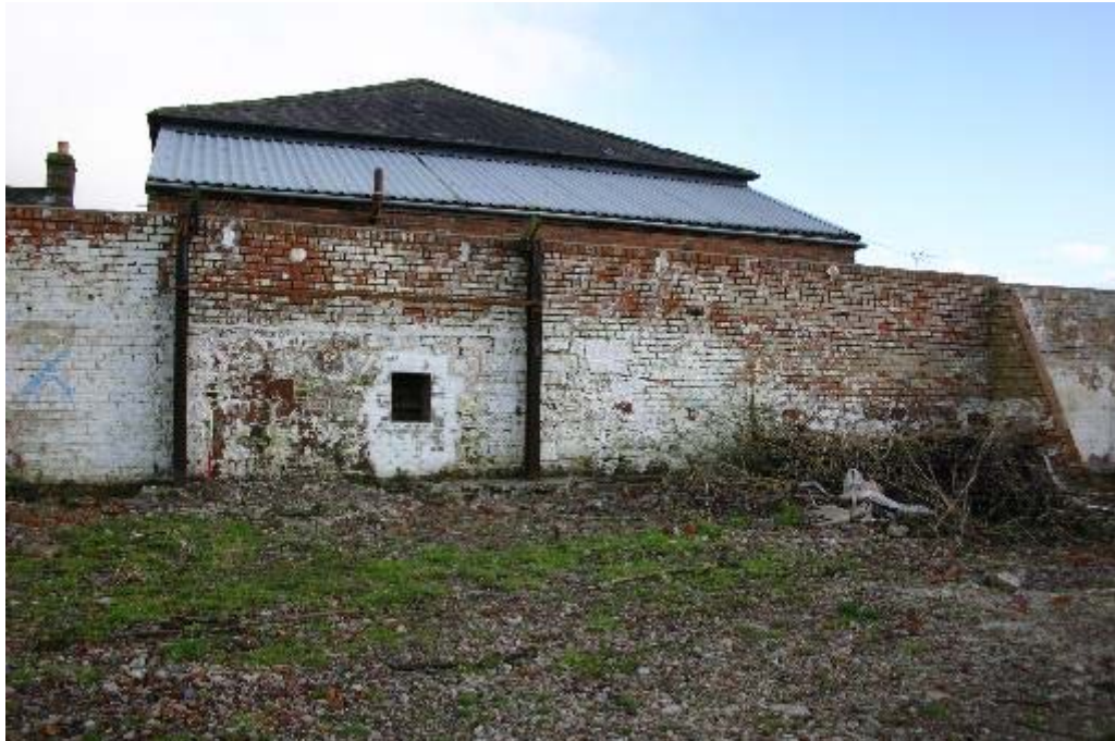
Plate 86: Northern section of eastern boundary wall
