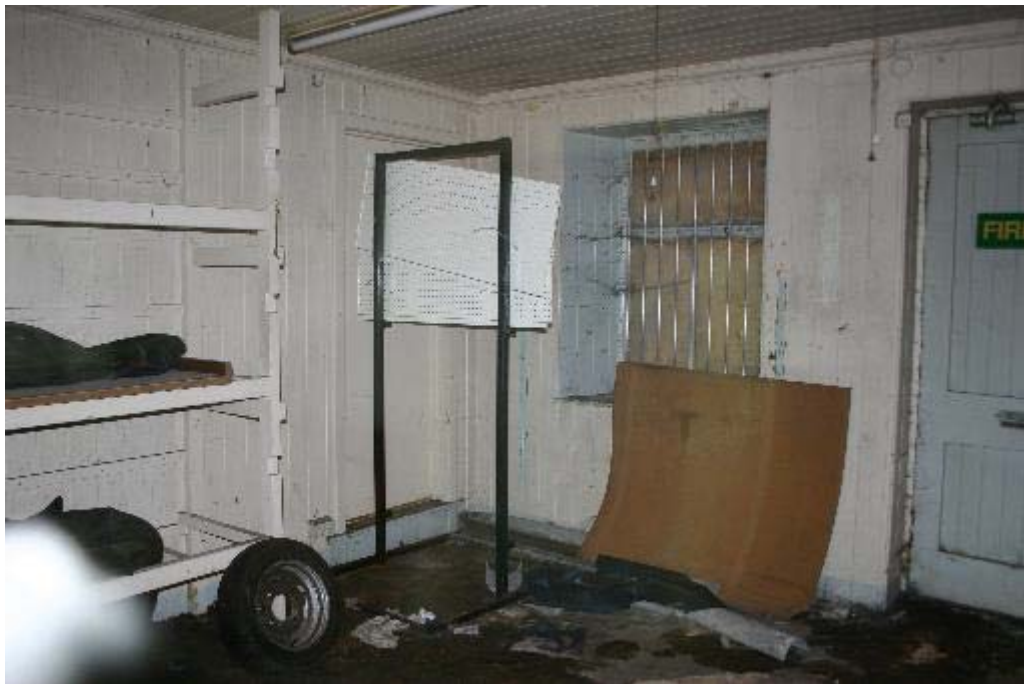
Plate 51: No 25, GF4 general view
