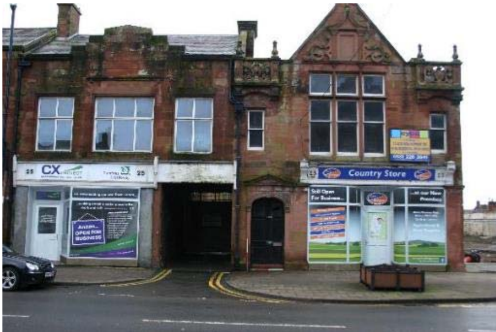
Plate 1: North facing elevation of No 23 and 25
