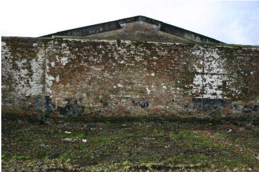
Plate 92: Western boundary wall
