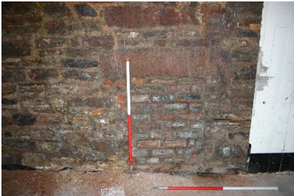
Plate 50: No 25, GF3 blocked off opening at the east elevation
