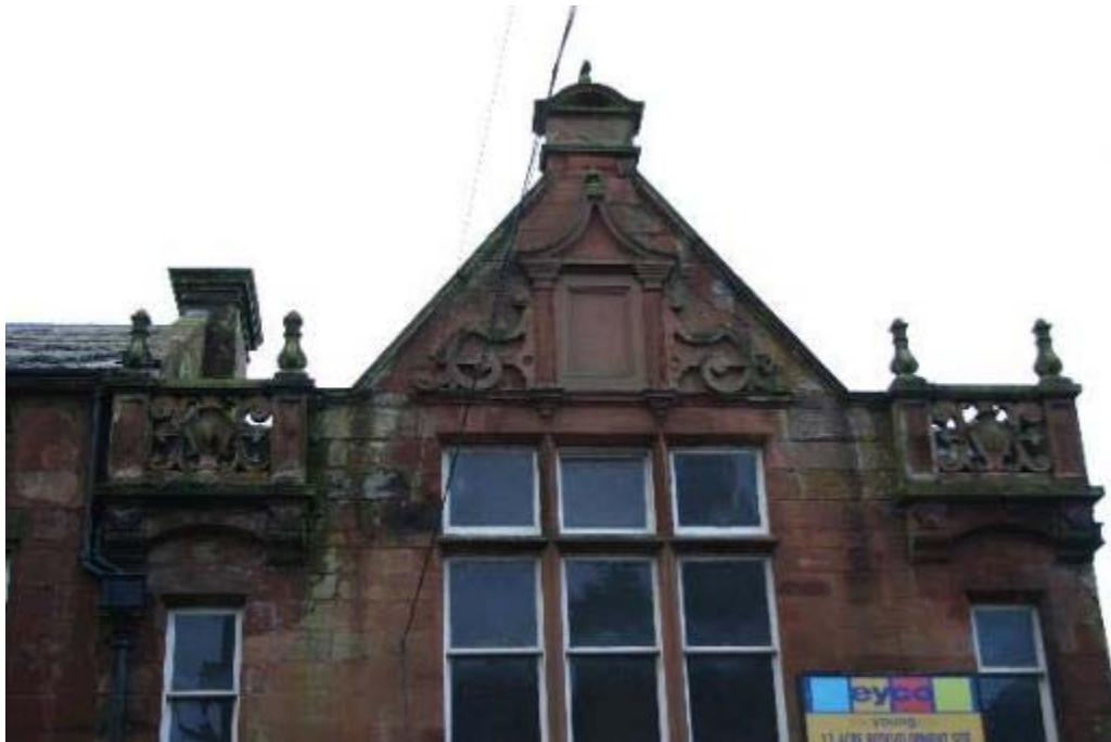
Plate 2: Detail at north facing elevation of No 23
