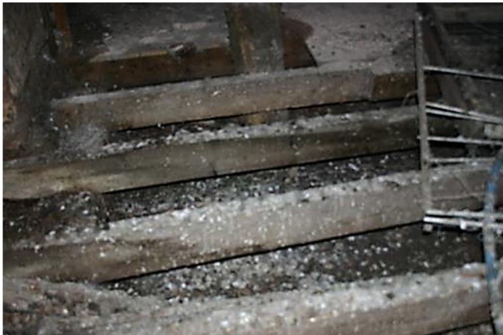
Plate 58: No 23, GF6 current state of the flooring
