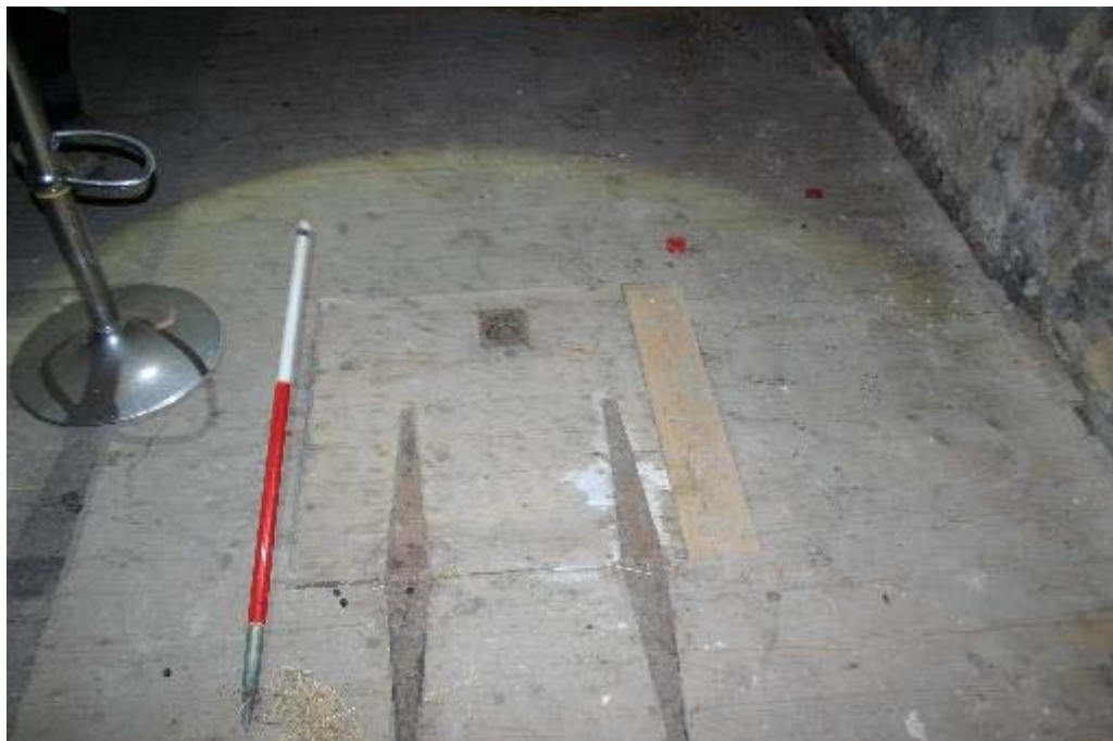
Plate 42: No 25, GF2 hatch towards the cellar
