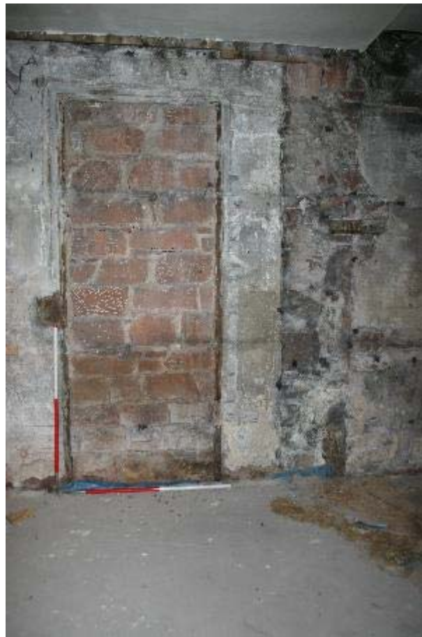
Plate 45: No 25, GF2 blocked doorway
