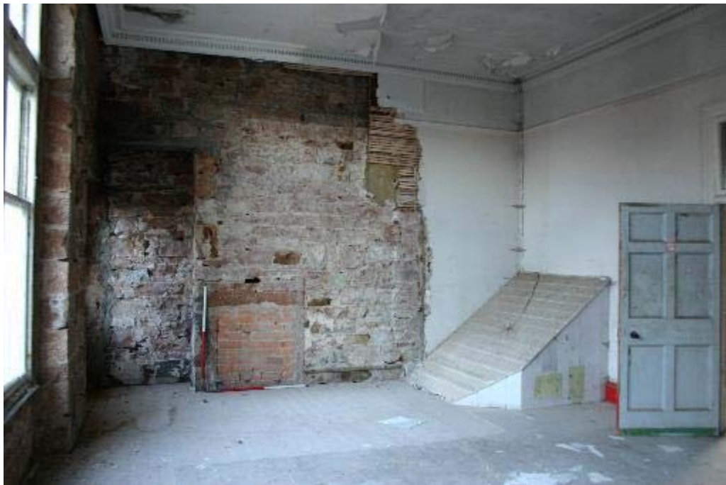
Plate 59: No 23, FF1 blocked off fireplace and inserted staircase space
