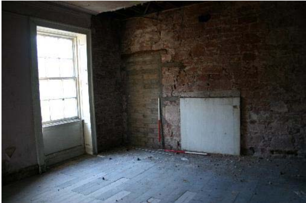
Plate 66: No 23, FF4 sash window with hidden shutters
