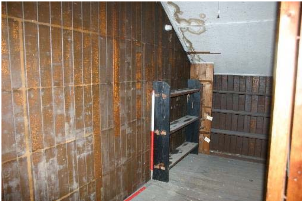
Plate 79: No 25, attic room, partitioned off section of room
