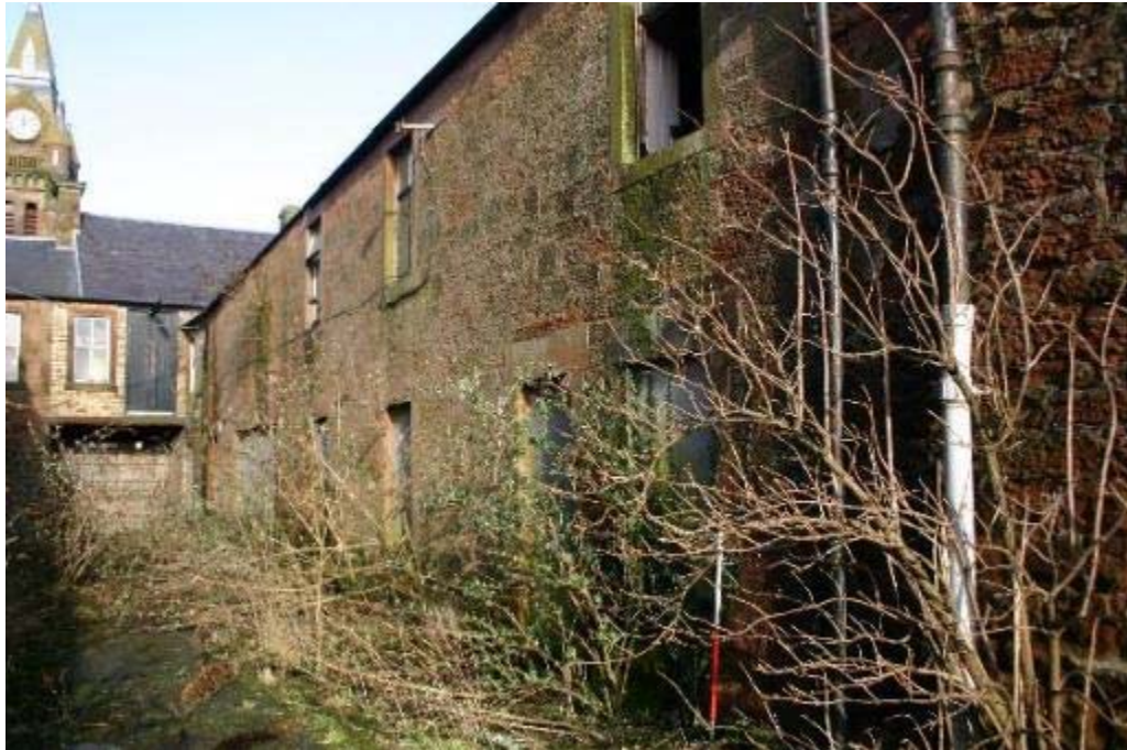
Plate 12: West facing elevation, 1920's section to the north of No 25
