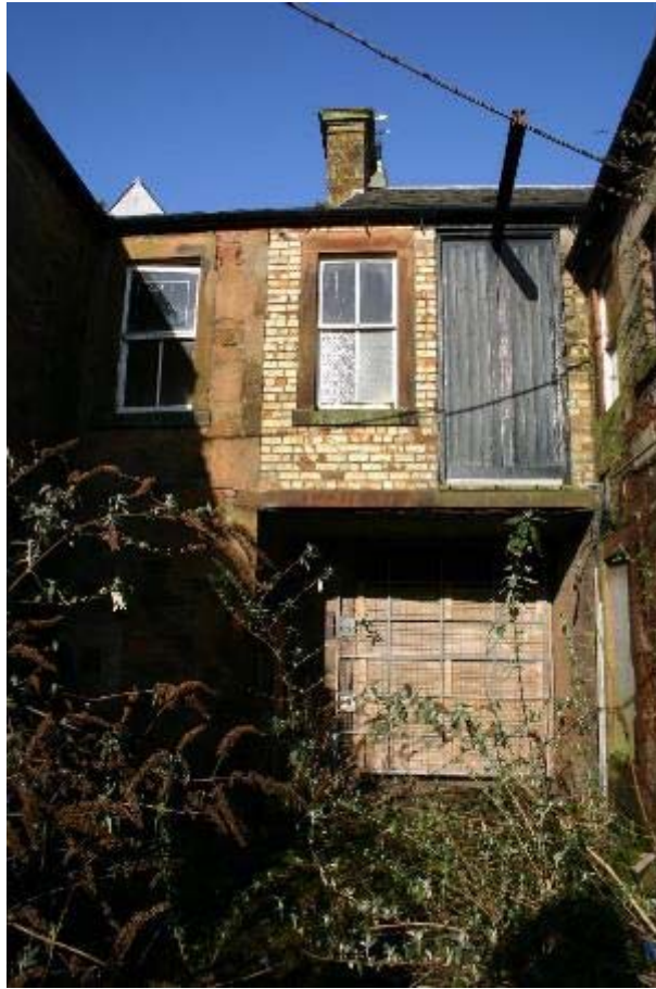
Plate 29: Bridged over driveway
