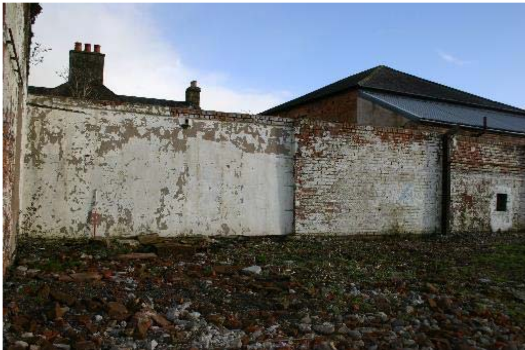
Plate 85: Northern section of eastern boundary wall
