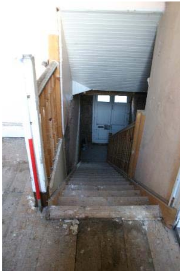
Plate 63: No 23, FF2 staircase towards GF1
