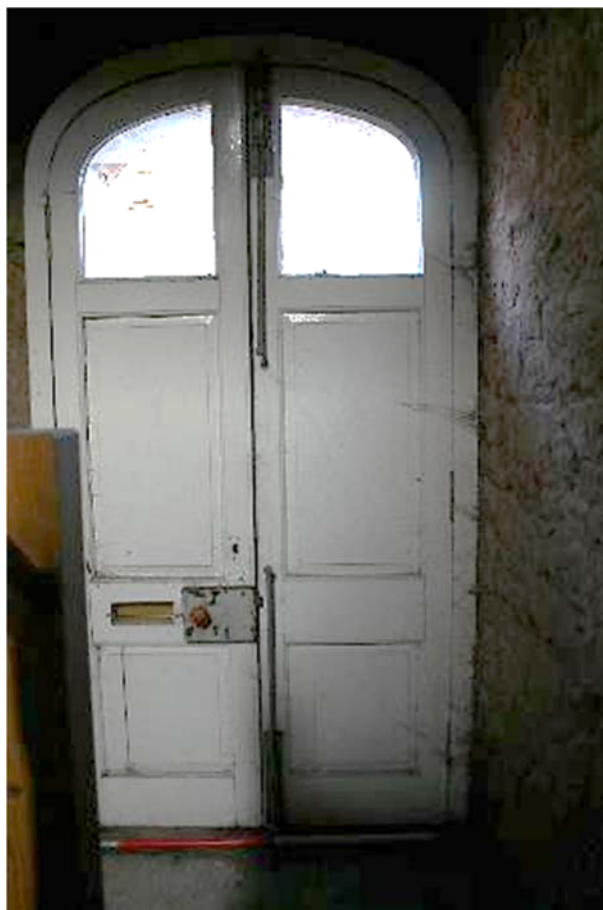
Plate 38: No 23, doorway in GF1
