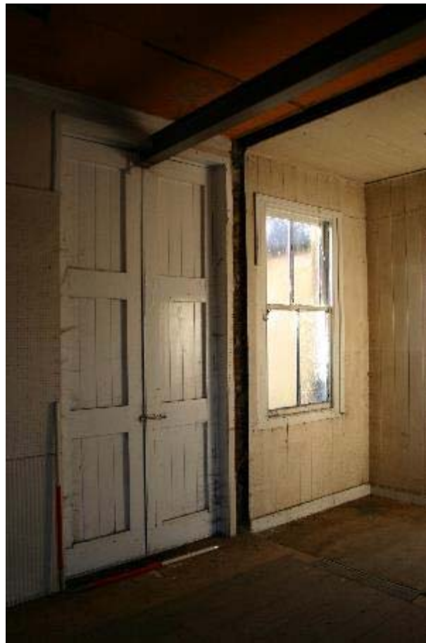
Plate 74: No 25, FF5 loading bay door at overbridging section
