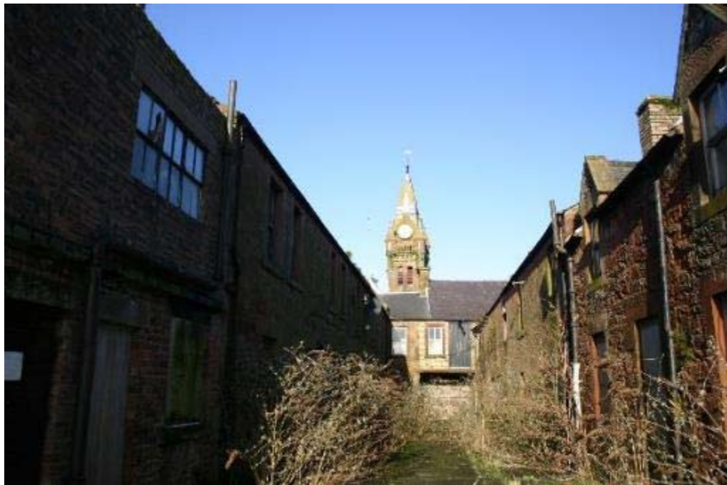
Plate 24: General view of east elevation of No 23
