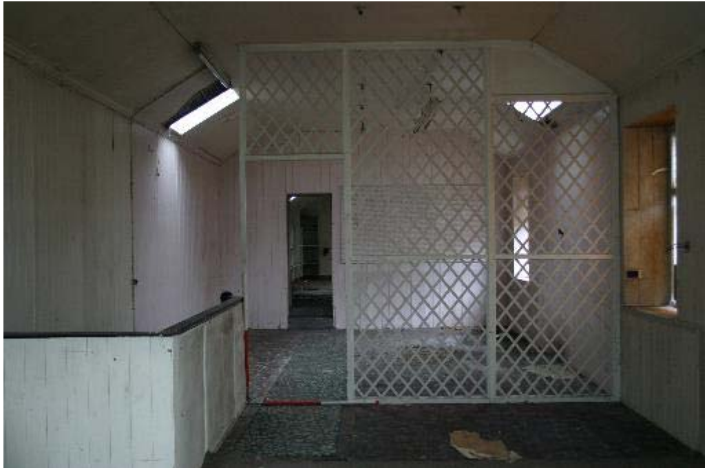
Plate 76: No 25, FF6 wooden partition at south end of room
