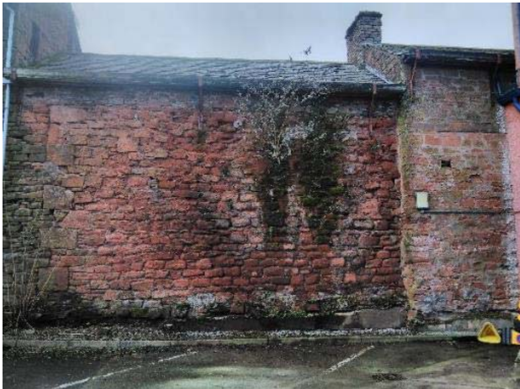
Plate 32: East facing elevation of No 25 from police car park
