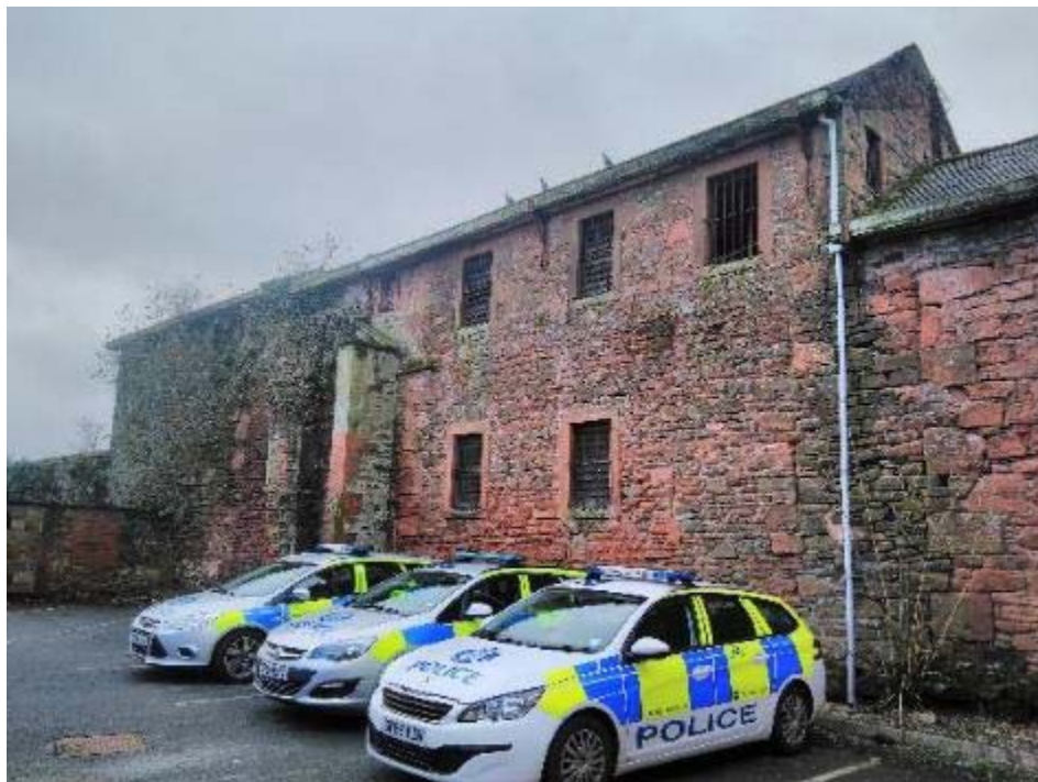
Plate 30: East facing elevation of No 25 from police car park
