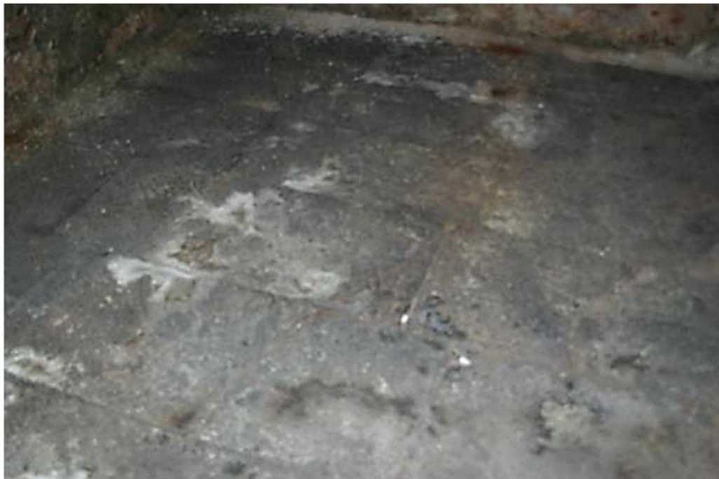
Plate 35: Cellar flag stones in southern cellar of No 23
