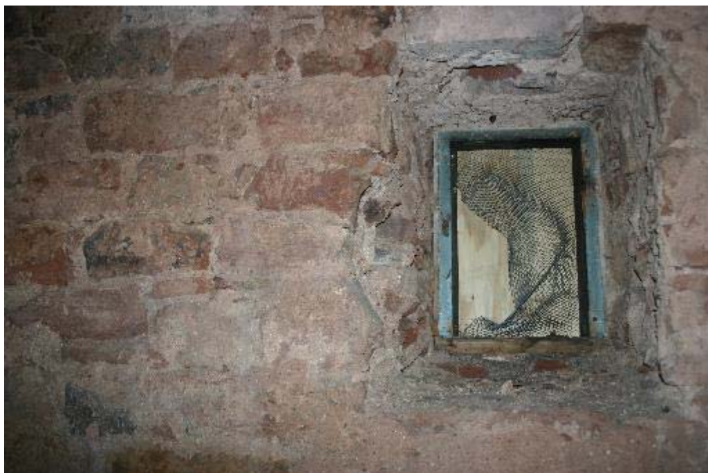
Plate 40: No 23, GF1 boarded up small window at east elevation
