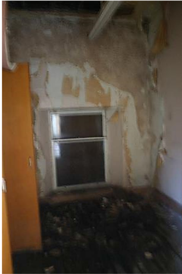
Plate 64: No 23, view into not accessible FF3 with blocked off staircase window
