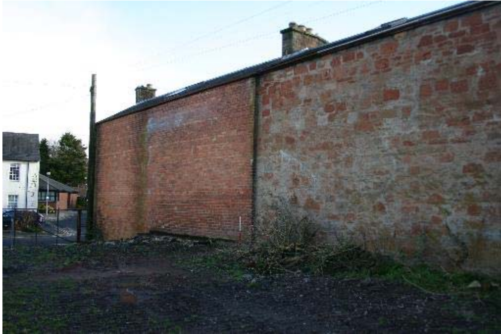
Plate 81: Southern boundary wall at smaller yard to the south-east
