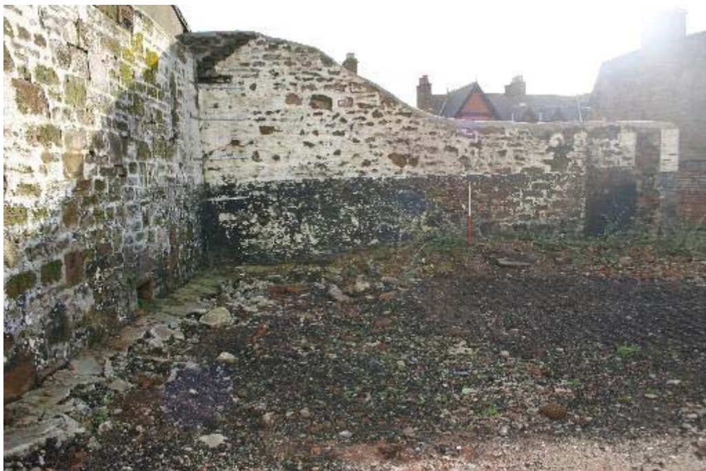
Plate 89: Eastern section of southern boundary wall
