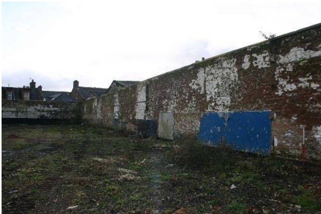
Plate 93: General view of western boundary wall
