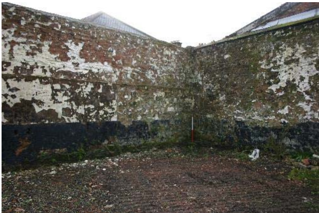
Plate 91: Corner of southern and western boundary wall
