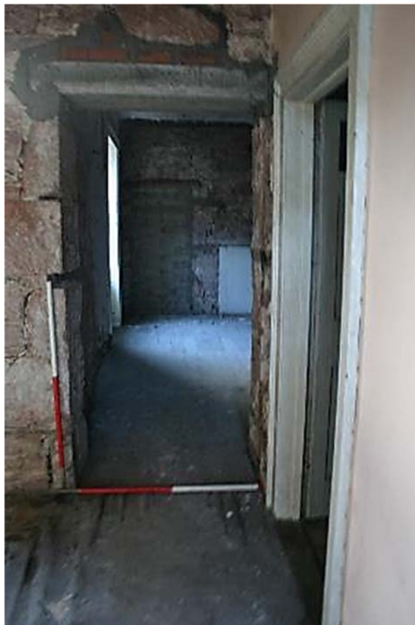
Plate 62: No 23, FF2, concrete lintel of doorway to FF4
