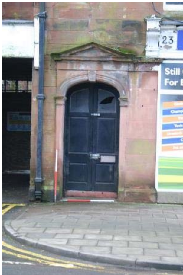
Plate 3: Detail at north facing elevation of No 23
