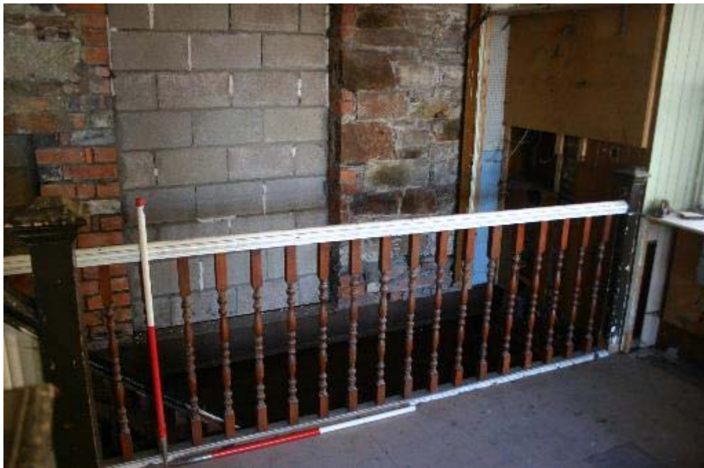
Plate 73: No 25, FF5 staircase to GF2 at south side
