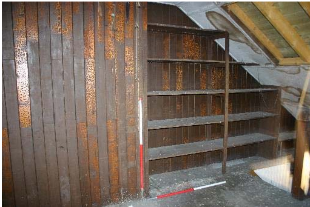
Plate 80: No 25, attic room, built in shelving at east elevation
