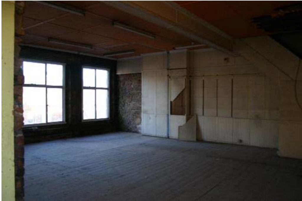
Plate 70: No 25, FF5 general view to the north-east
