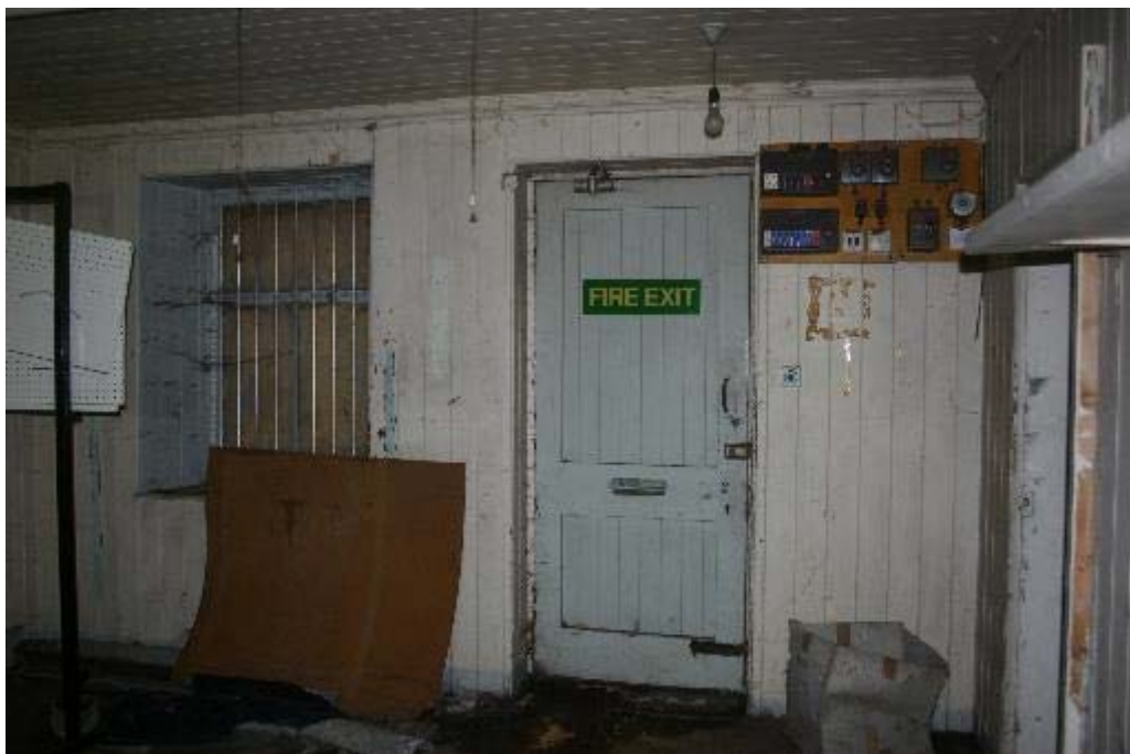
Plate 52: No 25, GF4 doorway and window at west elevation
