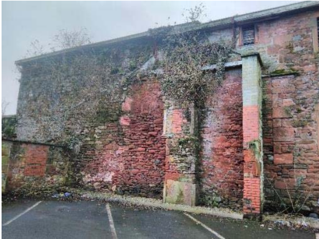
Plate 31: East facing elevation of No 25 from police car park
