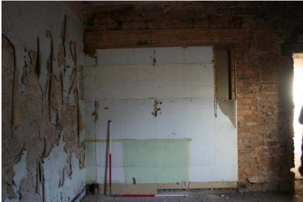
Plate 68: No 23, FF4 blocked off doorway towards FF3
