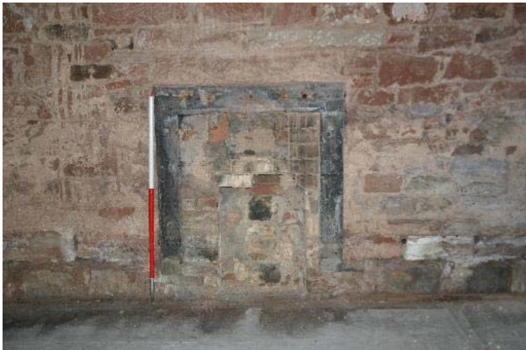
Plate 54: No 23, GF5 blocked off fireplace at the west elevation
