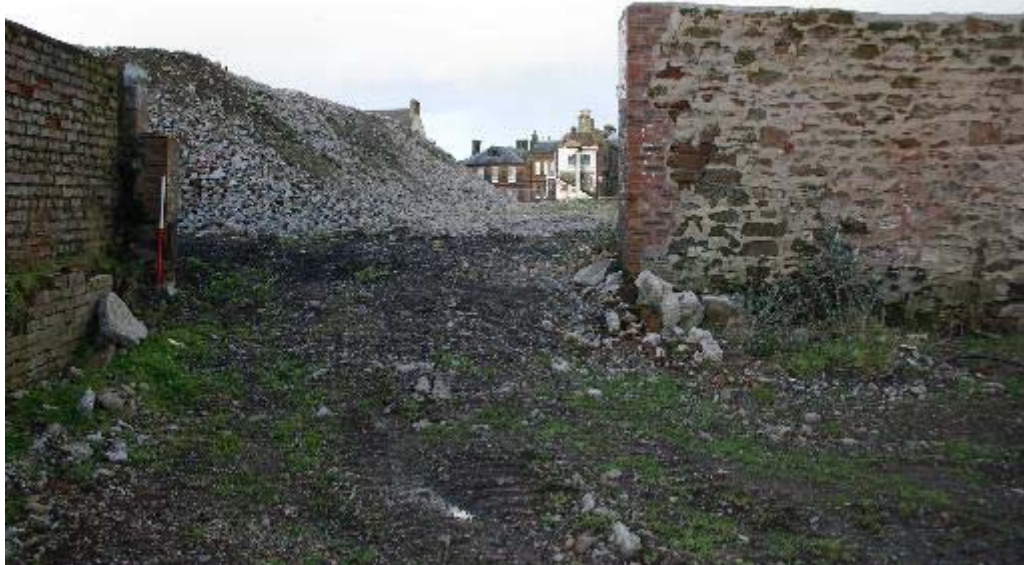
Plate 84: boundary walls with access to main site at small yard
