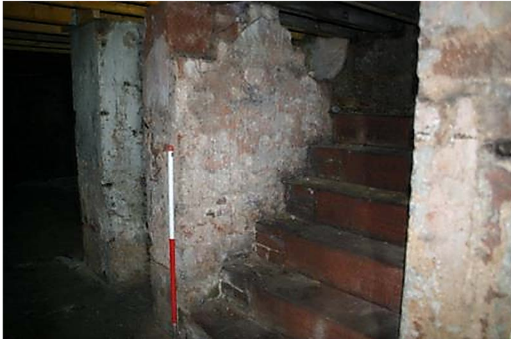
Plate 36: Old staircase towards GF5 in No 23
