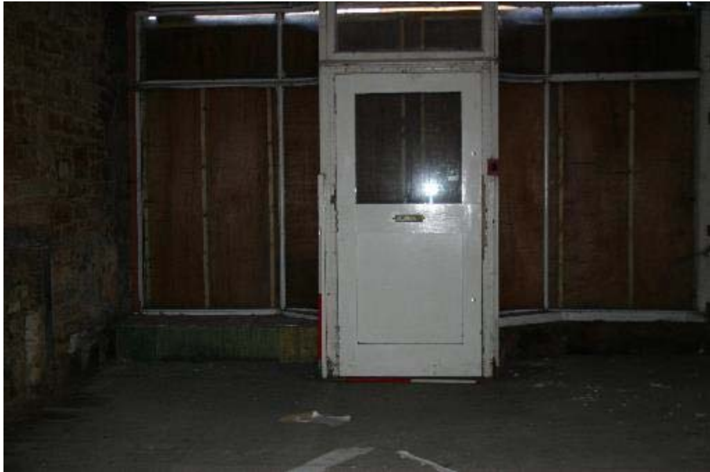
Plate 53: No 23, GF5 window shop front to the north
