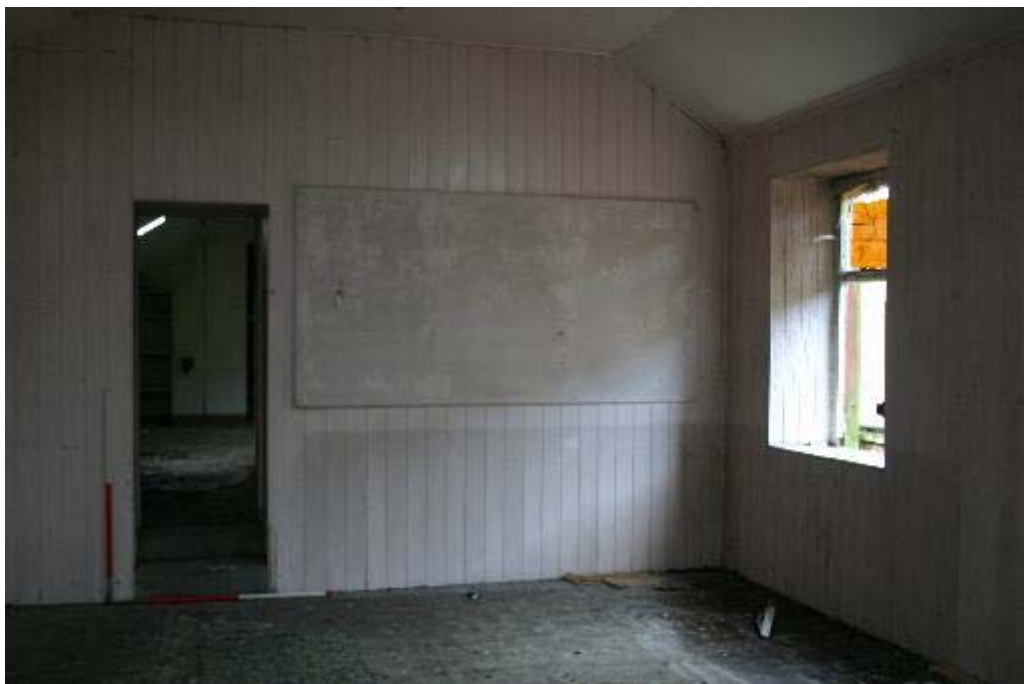
Plate 77: No 25, FF6 doorway with two steps towards FF7
