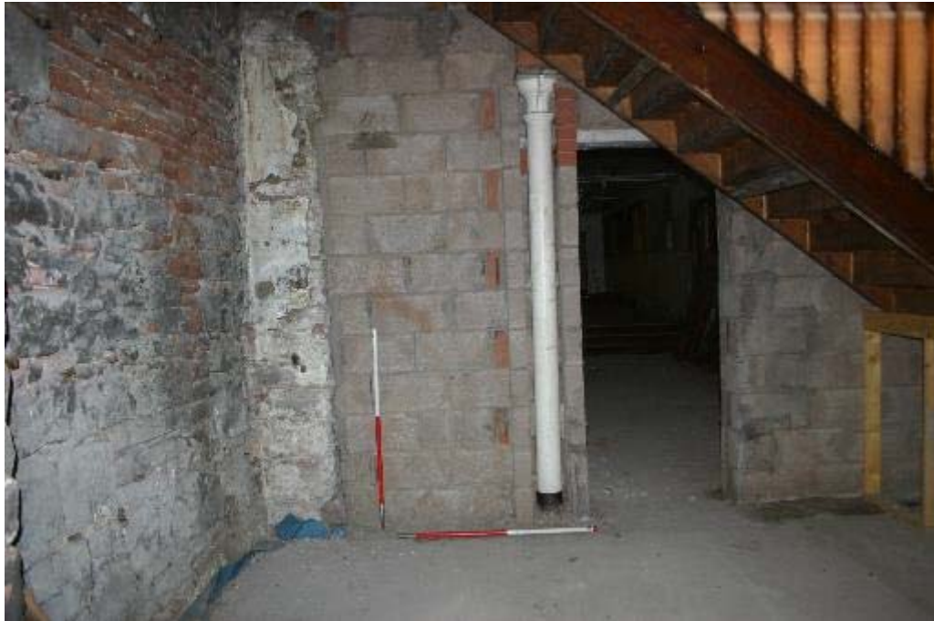
Plate 47: No 25, GF2 modern inserted concrete brick wall and cast iron column
