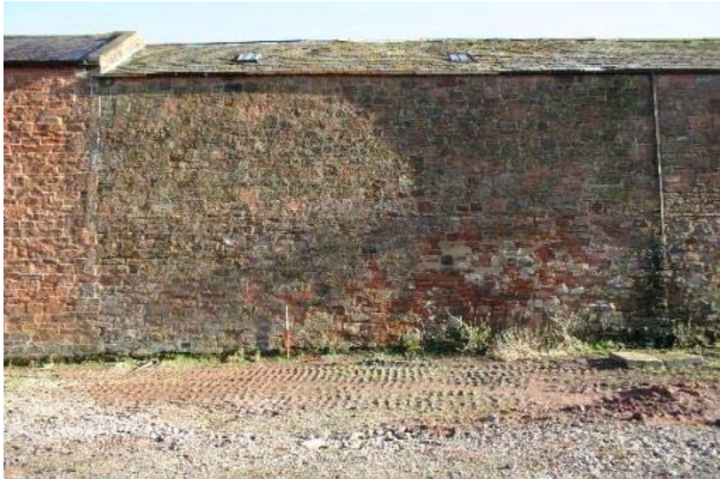
Plate 8: West facing elevation, northern central section of No 23
