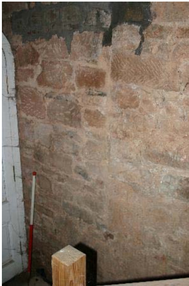
Plate 39: No 23, GF1 blocked off opening
