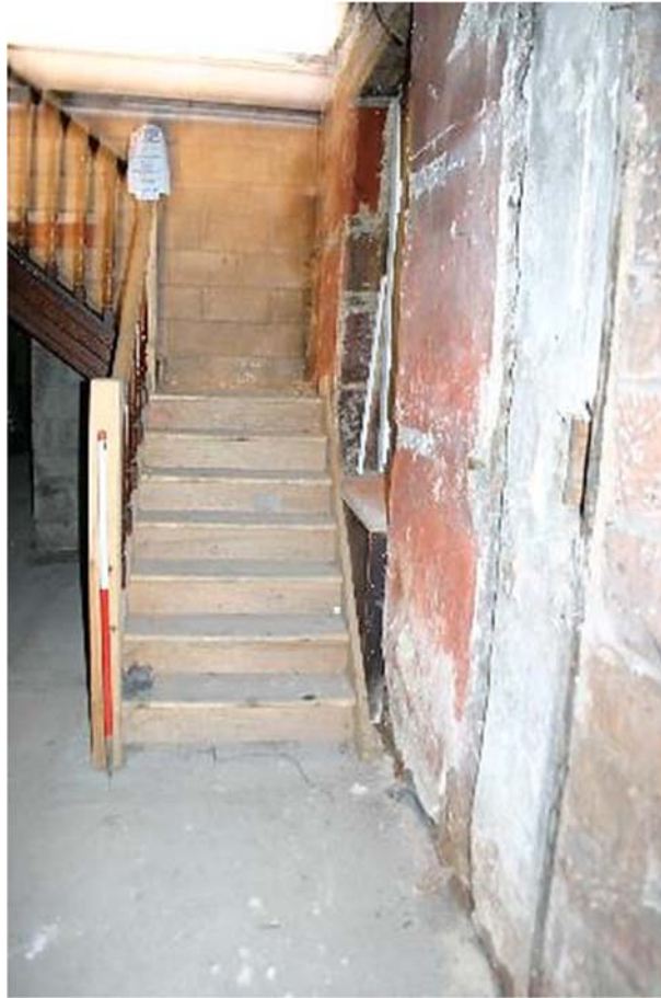
Plate 41: No 23, GF2, staircase to FF5
