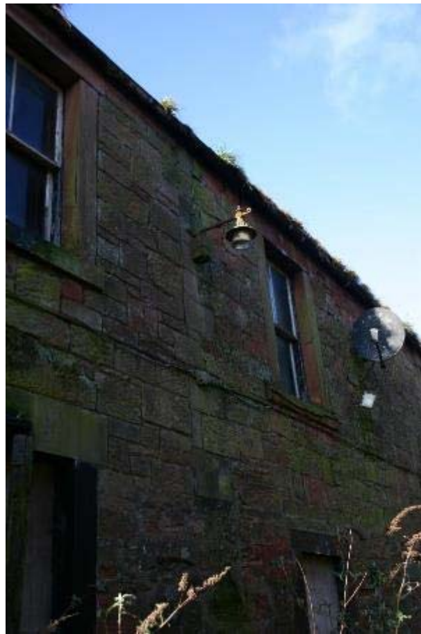
Plate 27: East elevation, visible break in fabric and modernised historic lamp at No 23
