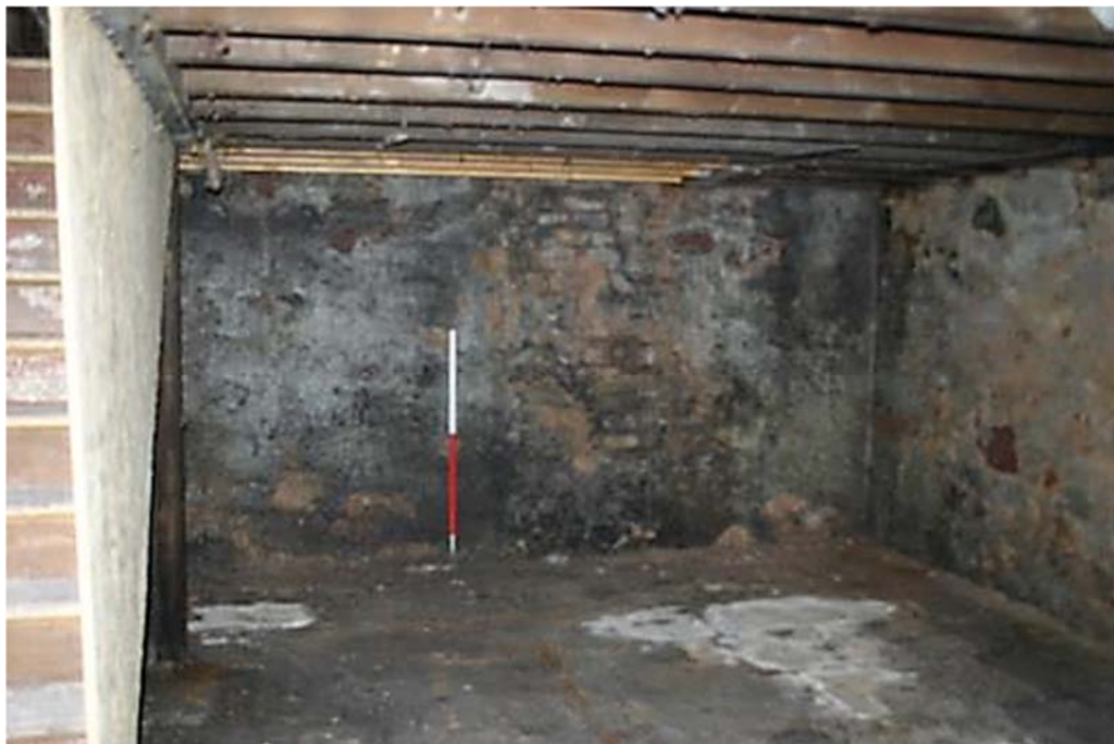
Plate 33: Southern cellar room of No 23
