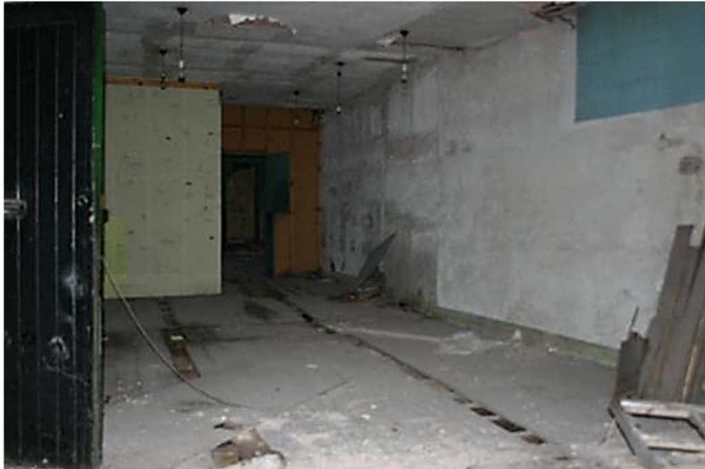
Plate 57: No 23, GF6 general view
