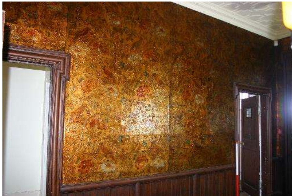
Plate 2: General view of east elevation
