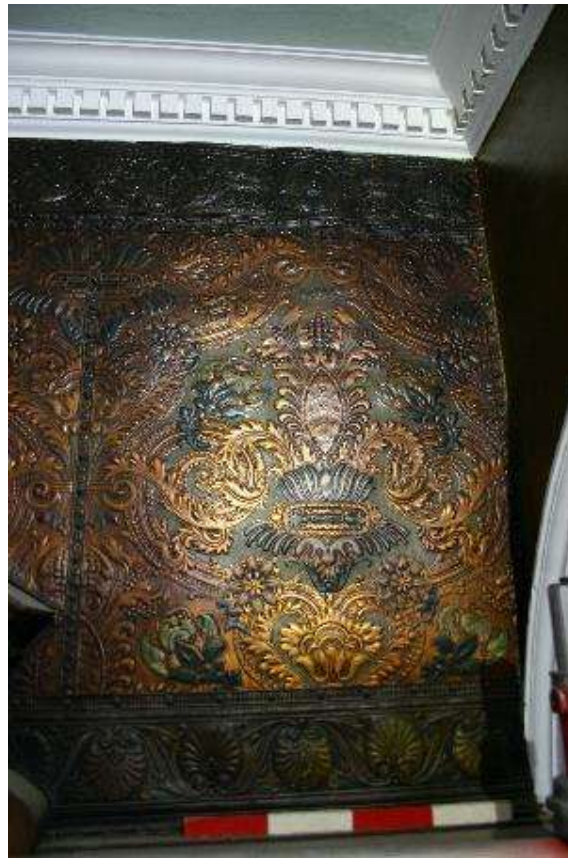
Plate 1: South-west corner section of wallpaper with well-preserved colours
