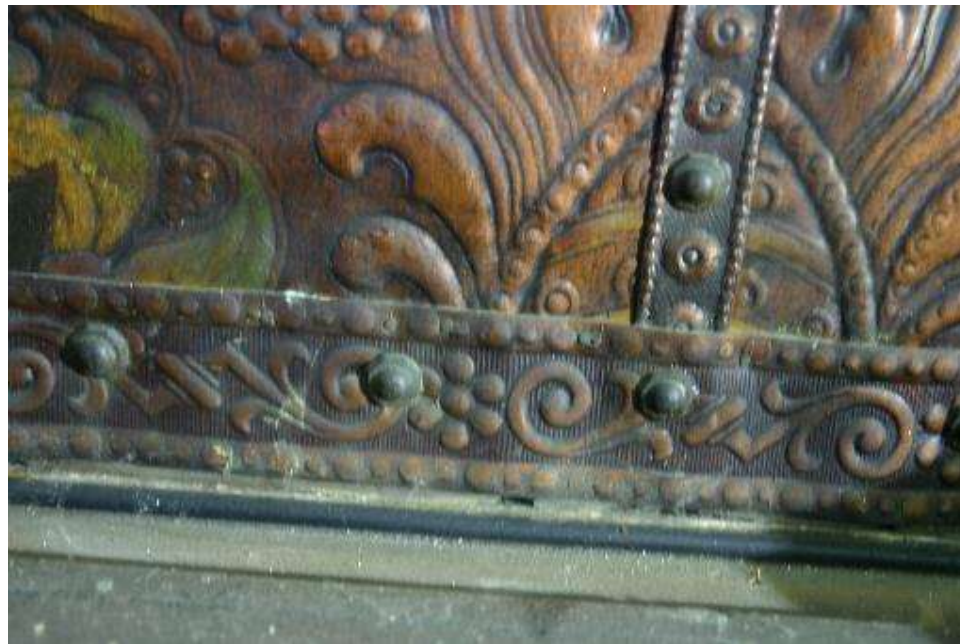
Plate 14: Detail of strips and metal studs holding the wallpaper together
