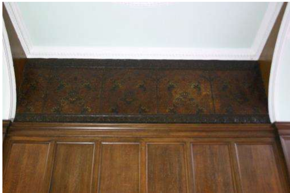
Plate 6: Central-south section of wallpaper above staircase with areas of well-preserved colour
