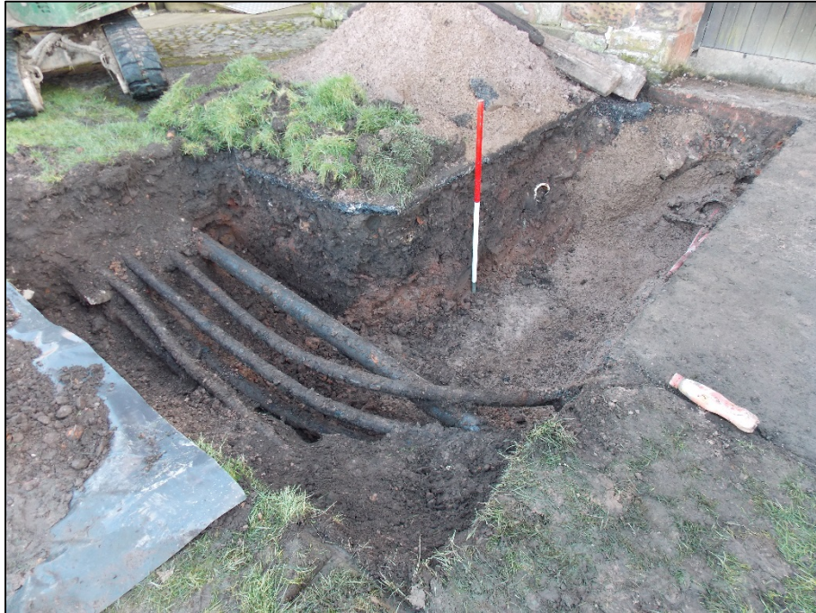
Plate 2: L-shaped trench showing exposed high voltage electric cables, facing south-east
