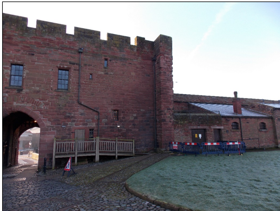
Plate 1: Location of groundworks. Safety barriers are to the front of the electric substation access doors, facing south-west
