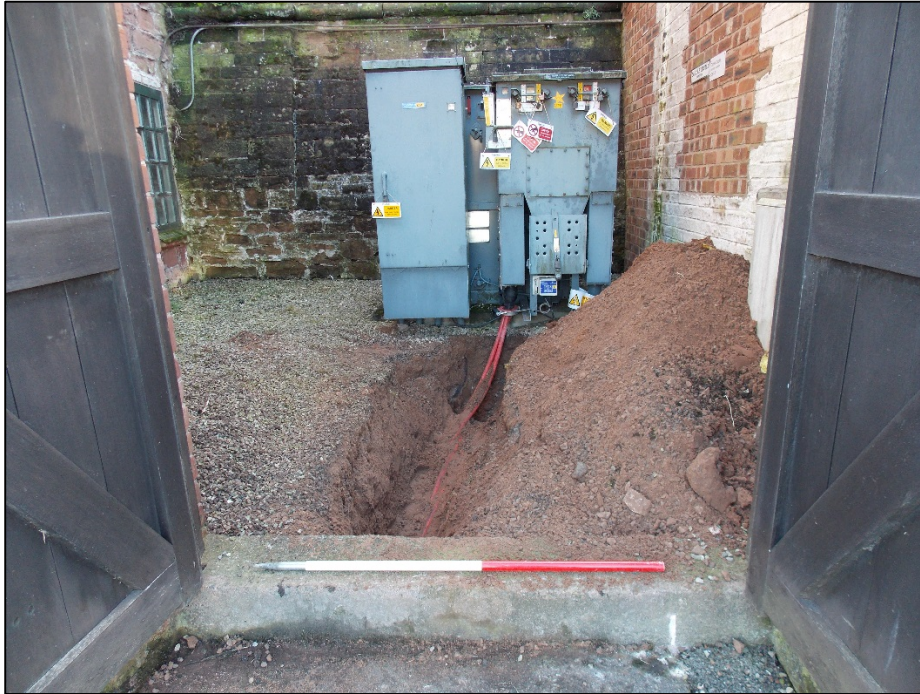
Plate 3: trench showing exposed high voltage electric cables and substation, facing south
