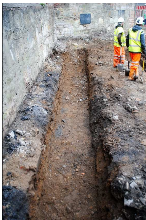
Plate 3; View east of Foundation Trench 1
