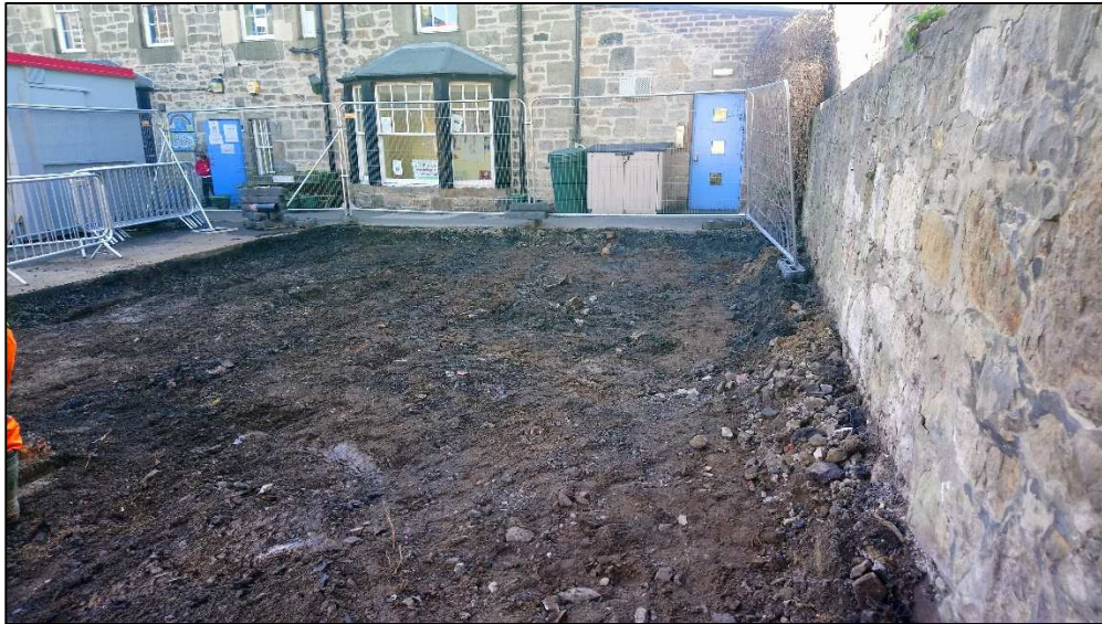
Plate 1; Area of foundation trenches before stripping facing west.
