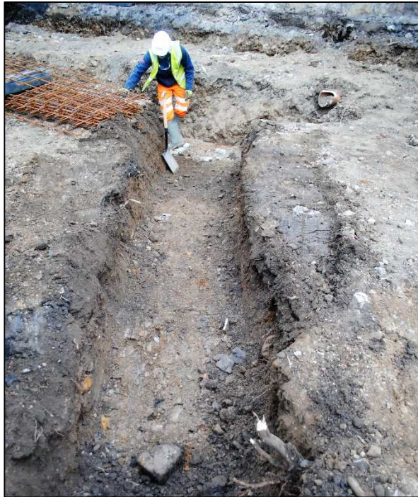
Plate 5; View north of Foundation Trench 3
