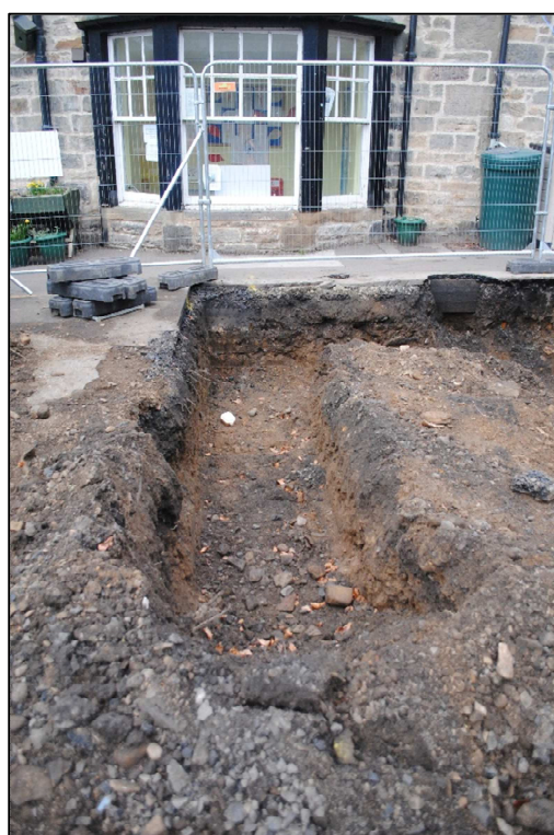
Plate 4; View west of Foundation Trench 2
