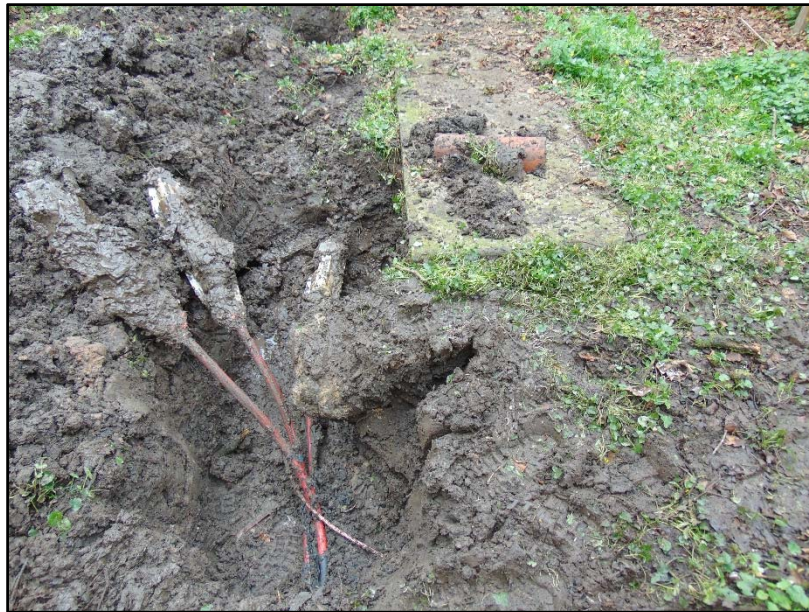
Plate 3; Trench 2 looking south, showing made topsoil deposit.
