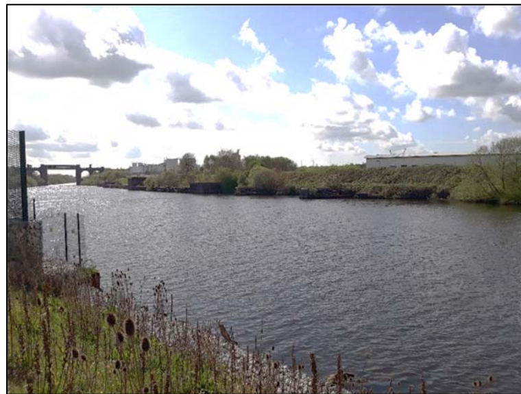
Plate 15: Showing jetties, possible surviving landing stage (Asset 38) and hydraulic lift (Asset 36) towards south-western part of south-eastern boundary of proposed development site, facing south-west
