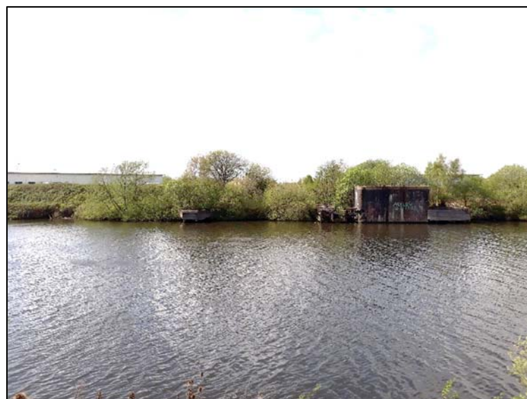
Plate 16: Showing jetties, and remnants of early 20 th century hydraulic lift (Asset 40), towards north-eastern part of south-eastern boundary of proposed development site, facing north-west
