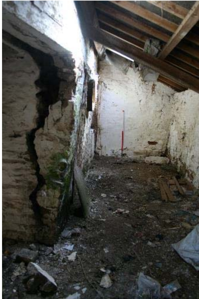
Plate 49: General view of the central lean-to with tilting chimney
