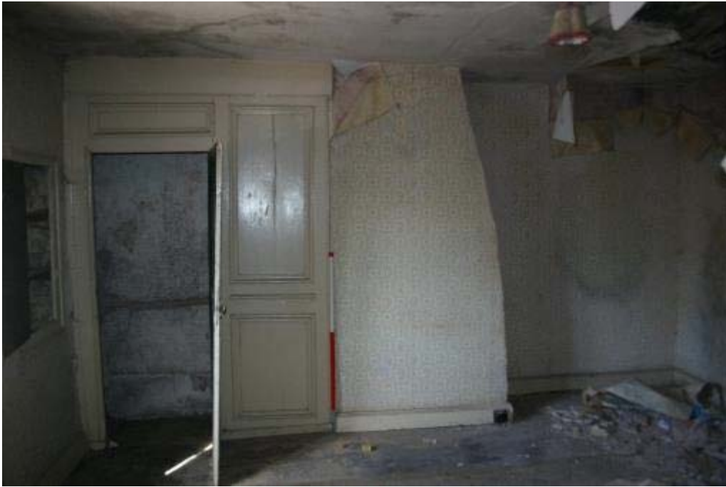
Plate 36: FF-4 chimney breast and built in cupboard
