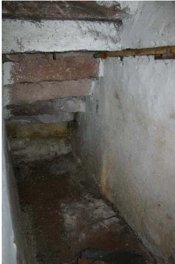
Plate 19: GF-4 under the stairs cupboard
