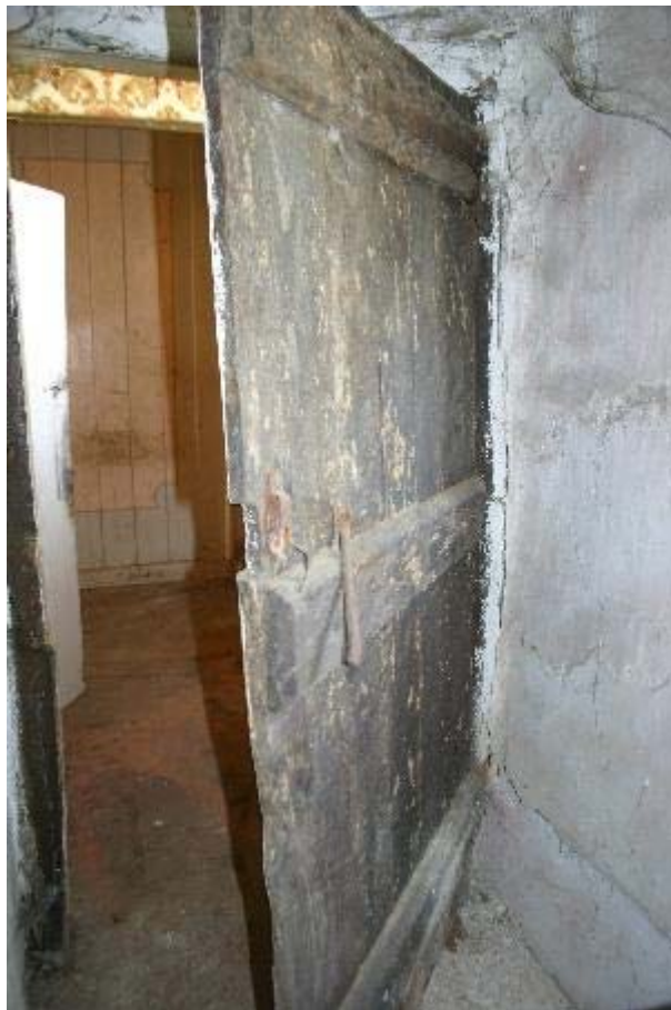
Plate 25: GF-6 timber doorway with round headed strap hinges
