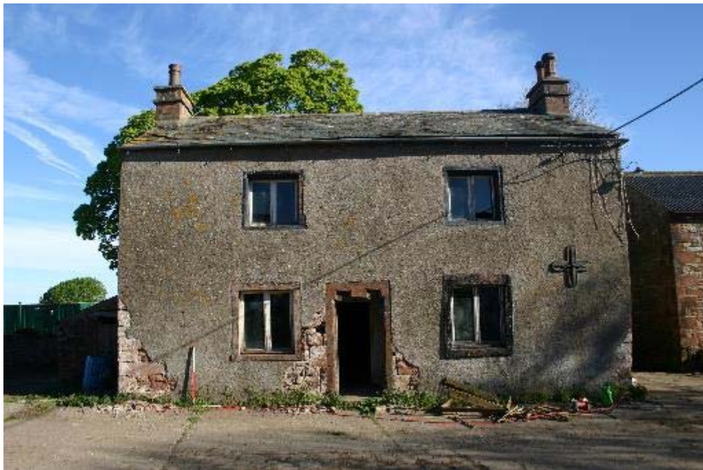
Plate 1: South facing elevation
