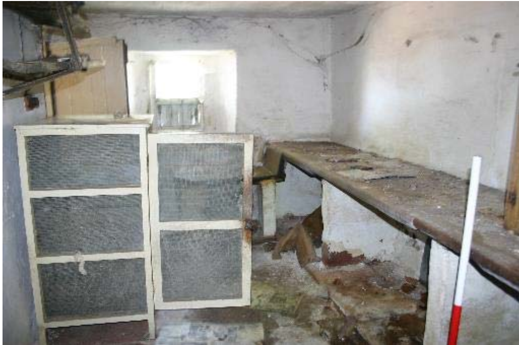
Plate 23: GF-6 storage room with workbenches
