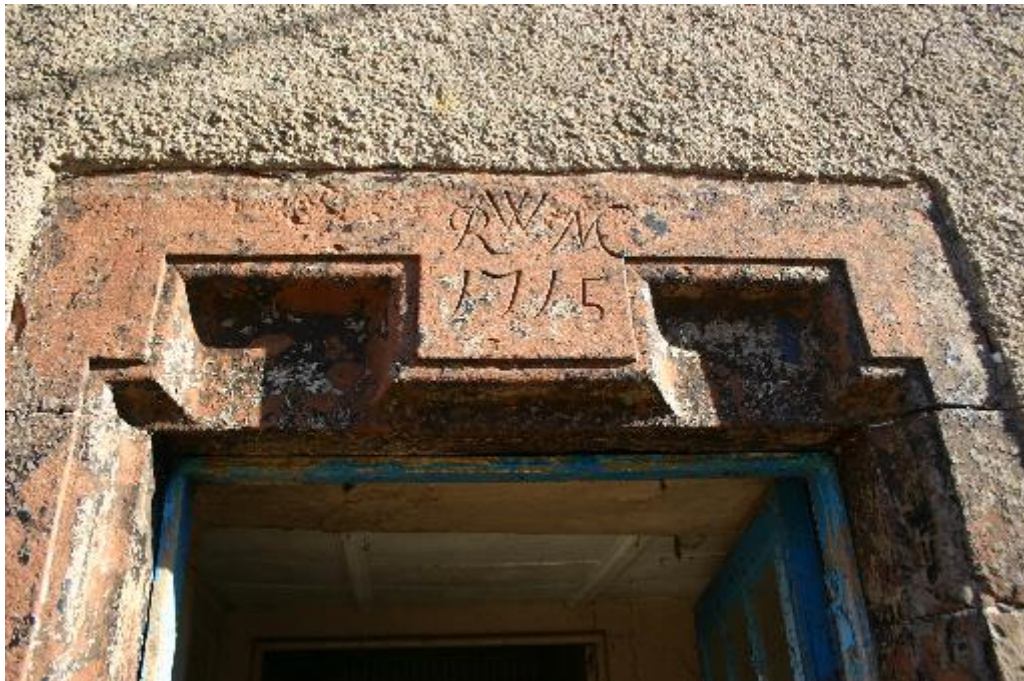
Plate 2: Detail: datestone in lintel
