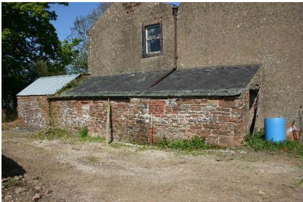
Plate 44: Two sandstone lean-tos with modern red brick extension
