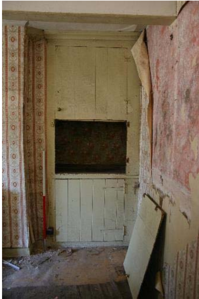
Plate 10: GF-2, built in cupboard with butterfly and strap hinges
