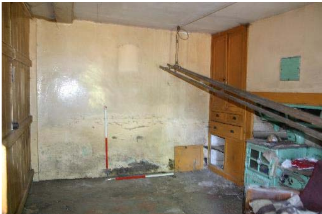
Plate 20: GF-5 general view of old kitchen
