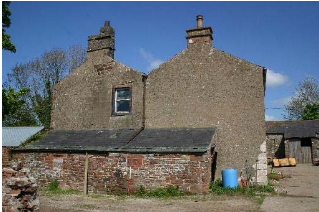
Plate 3: West facing elevation with lean-to
