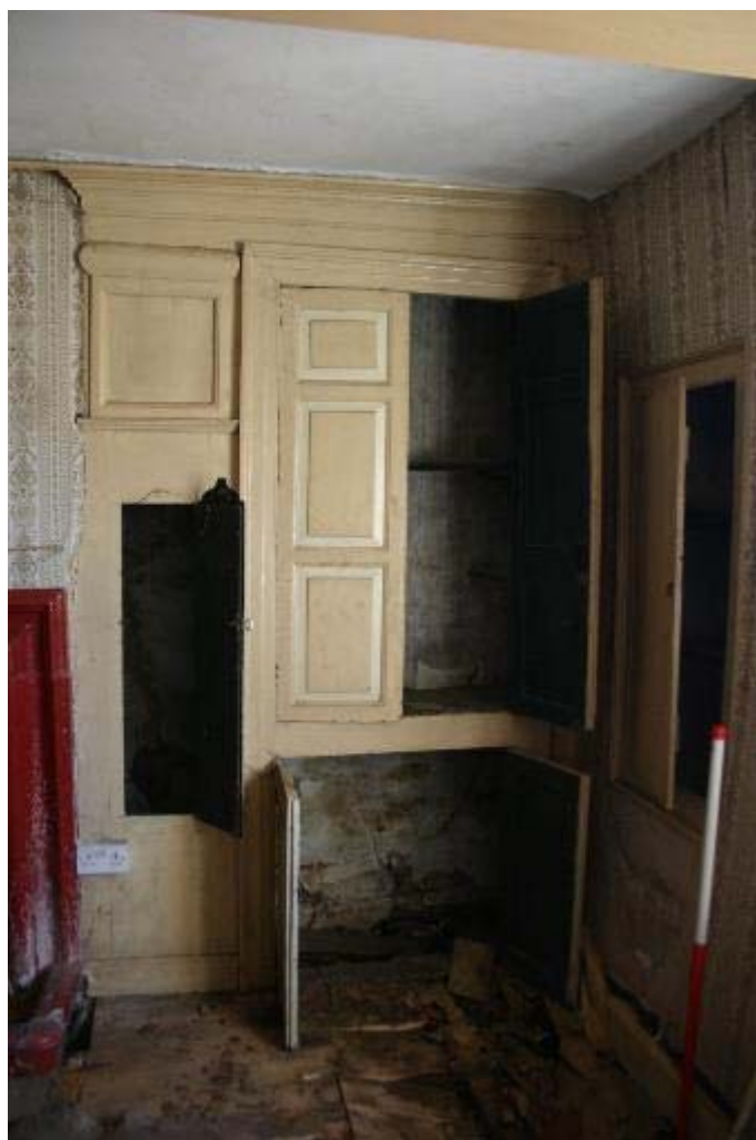
Plate 13: GF-3, built in Victorian cupboard
