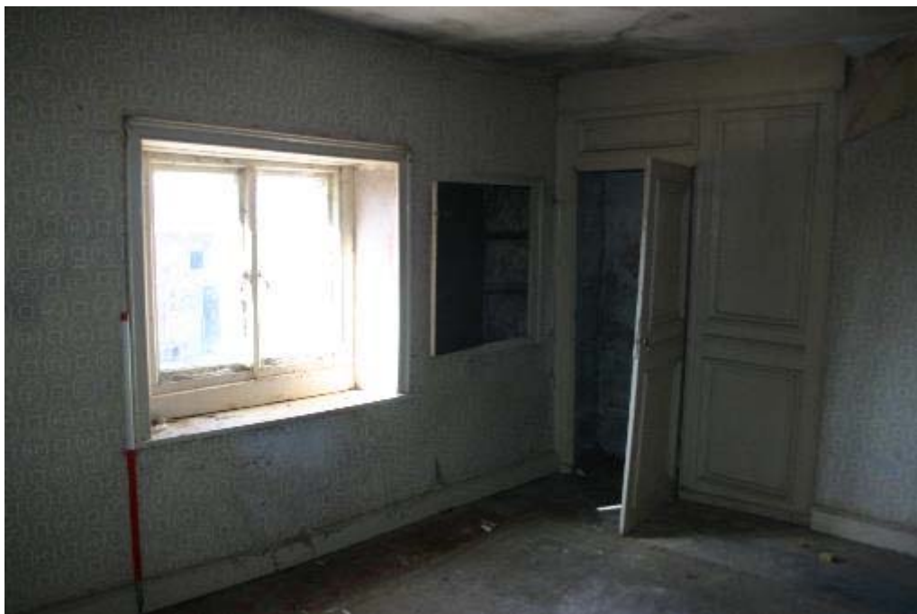
Plate 35: FF-4 general view, built in cupboards
