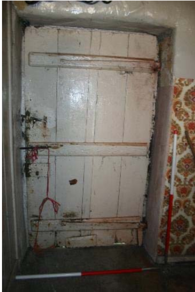
Plate 18: GF-4 doorway to back yard with round headed strap hinges
