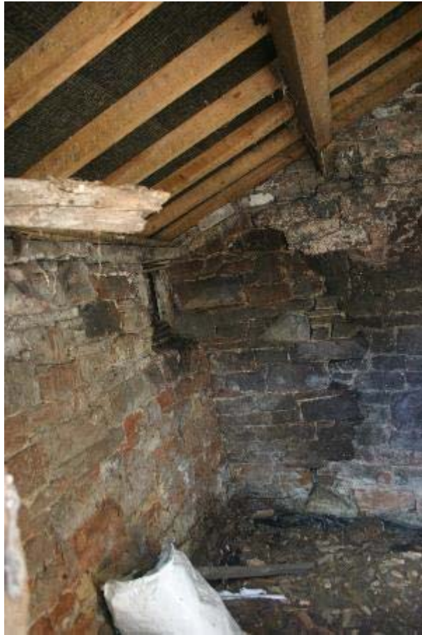
Plate 47: Southern lean-to with bricked up window at corner
