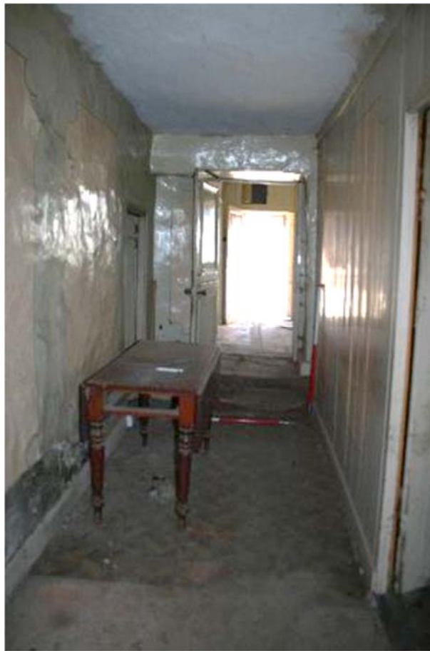
Plate 15: GF-4 hallway room
