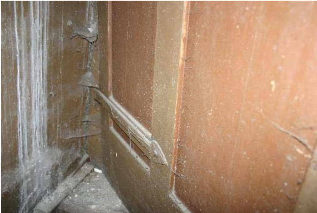
Plate 42: FF-6 door with strap hinges with spearhead shaped ends
