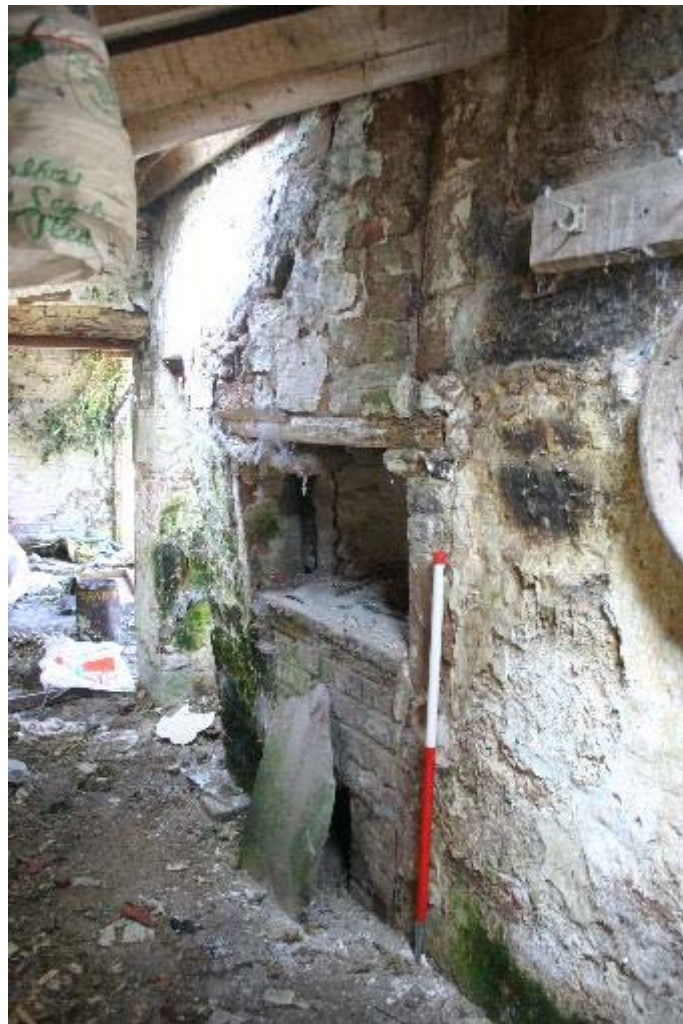
Plate 51: Oven in central lean-to
