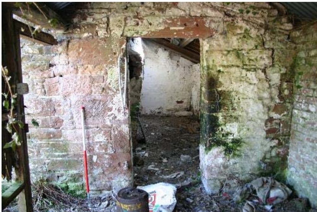
Plate 48: Doorway to the central lean-to from the red brick extension
