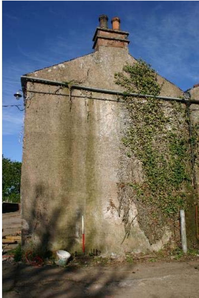
Plate 5: Southern section of east facing elevation
