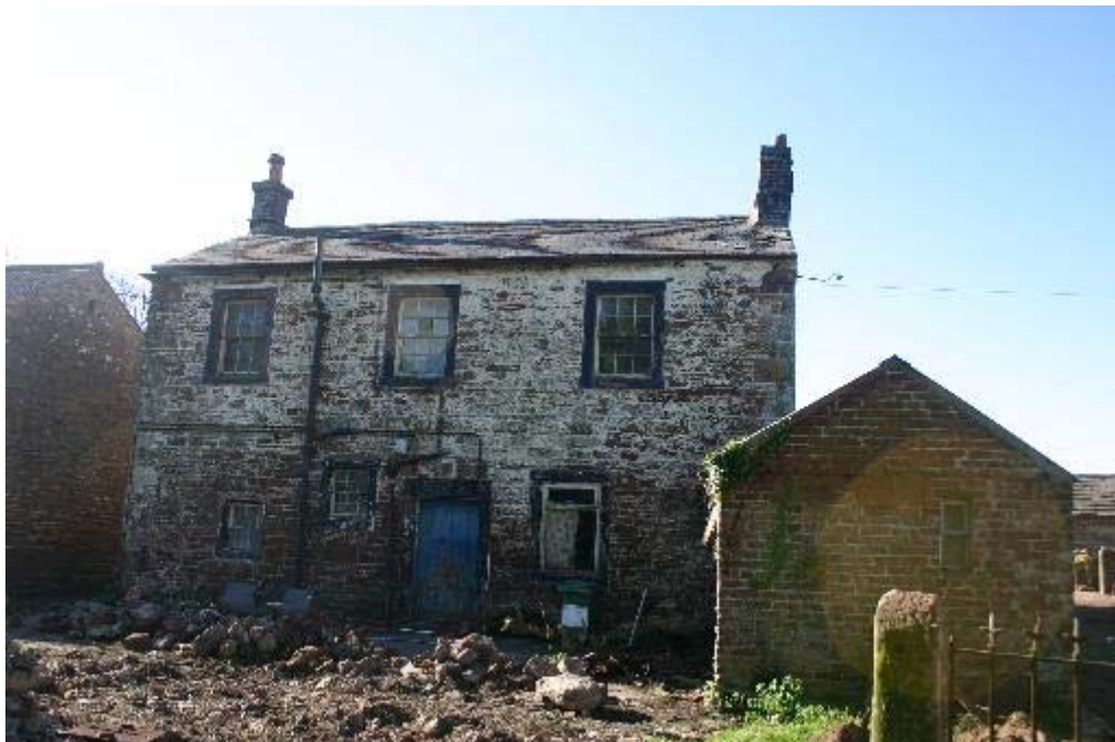
Plate 4: North facing elevation with modern brick extension of lean-to
