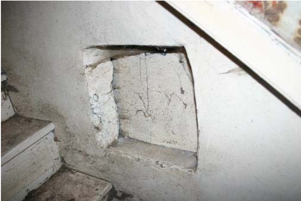
Plate 28: Small niche halfway up the staircase for lighting
