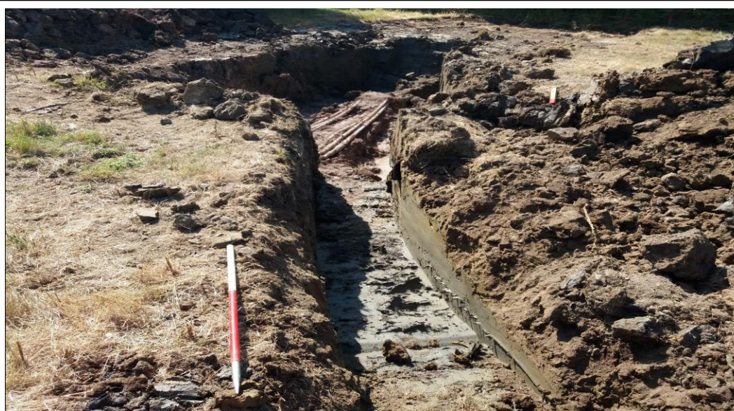
Picture Taken: 11/07/2018 Plate No. 9 Title: Cable trench and drill point hole within Area A, facing SE with one 1m scale.
