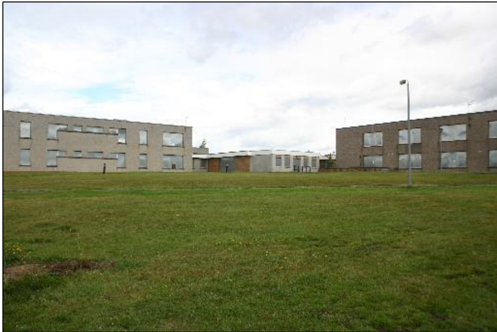
Plate 7: Boarded up modern hospital structures
