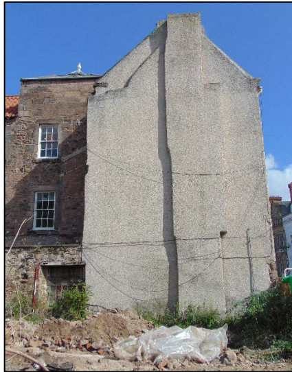
Plate 11: Rendering obscuring detail of south-eastern extent of eastern part of wall
