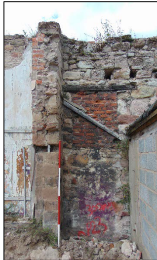
Plate 7: South-western blocked window in central part of wall, facing north-west
