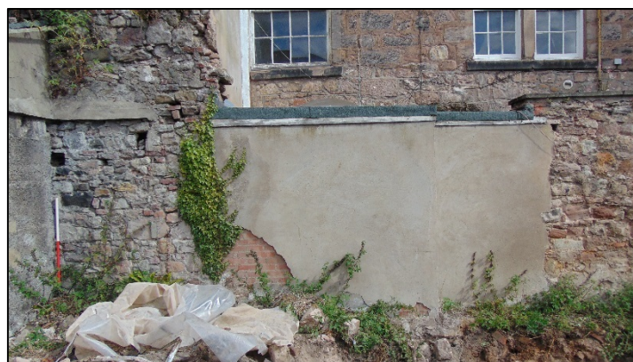
Plate 10: Rendering obscuring detail of north-western part of central area of eastern part of wall
