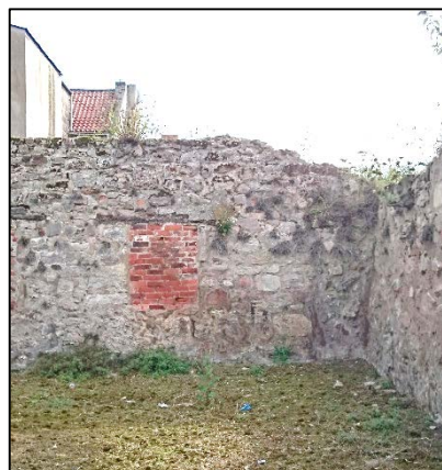
Plate 8: South-western blocked window with second former window (at left extent of image), in north-west facing elevation of central part of wall
