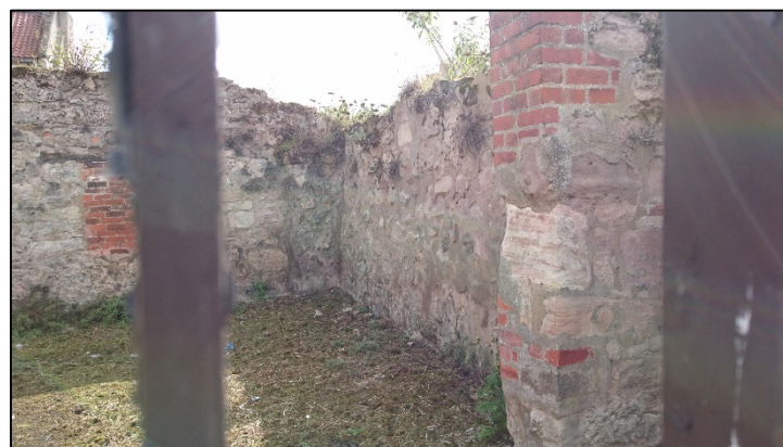
Plate 5: Restricted view of north-east facing elevation of western part of wall
