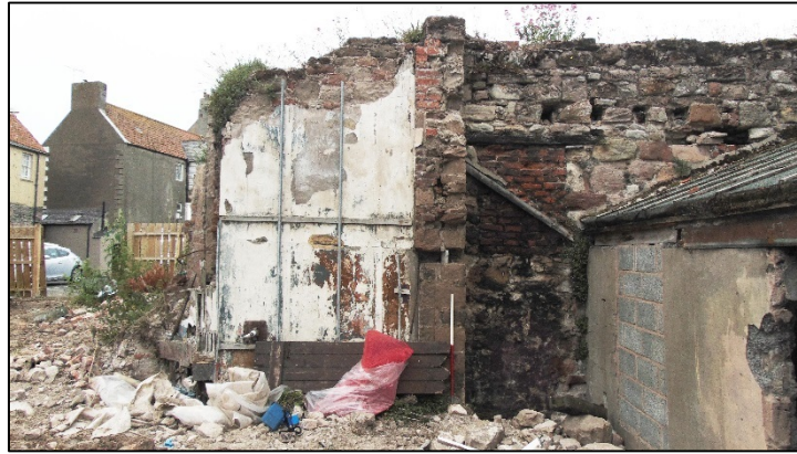
Plate 6: Central part of boundary wall, south-east facing elevation, facing north-west
