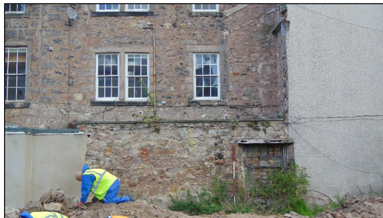
Plate 14: Former opening in south-west elevation of eastern part of wall, facing north-east
