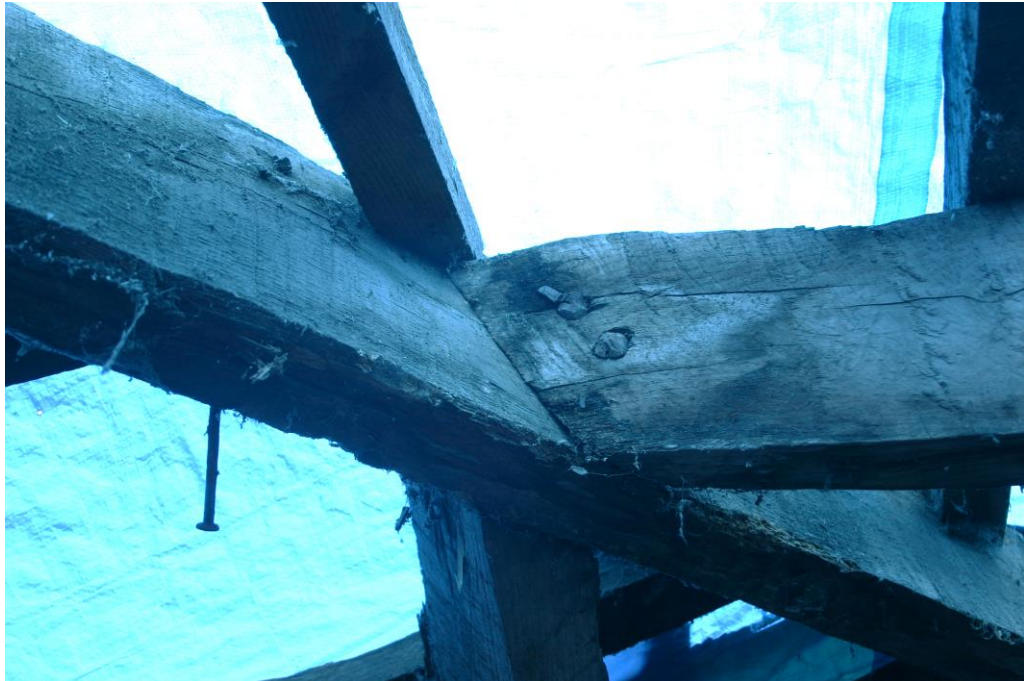
Plate 7: 19th century metal nails at purlin (f) to hip-rafter (d)
