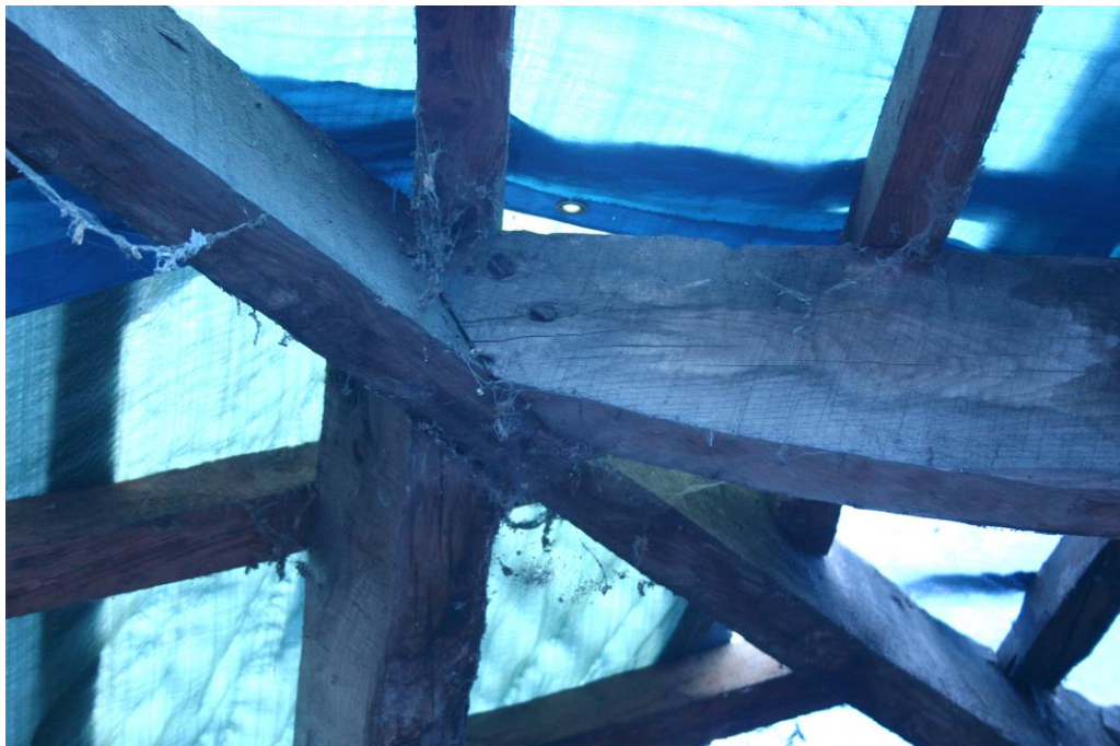
Plate 8: 19th century metal nails at purlin (h) to hip-rafter (d)
