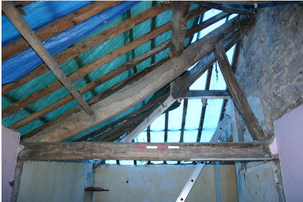
Plate 1: General view of the truss, with tie-beam (a), strut (b), and principal (c)
