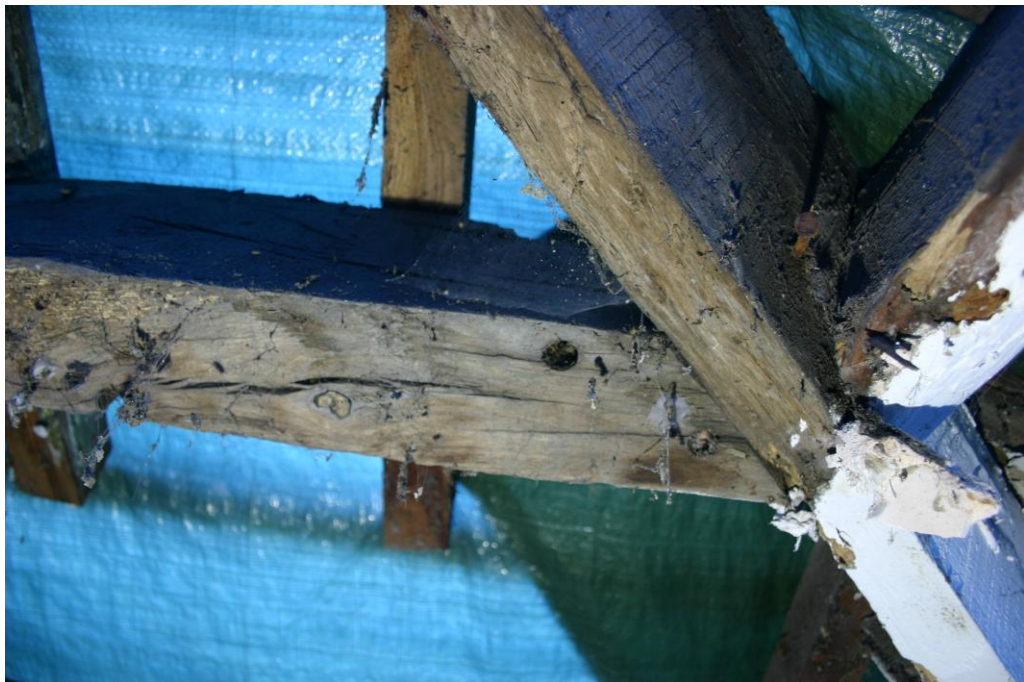
Plate 6: Dowel hole in purlin (f)
