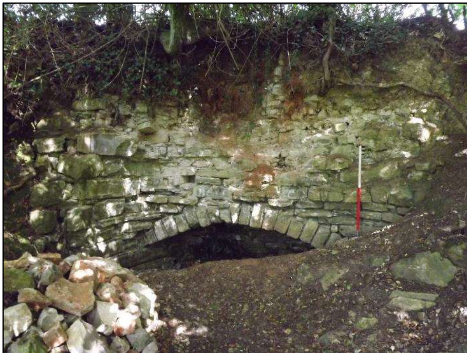
Plate 24; Limekiln draw-hole {10} (HER Ref. MDV70581), looking NNE, 1x1m scale.
