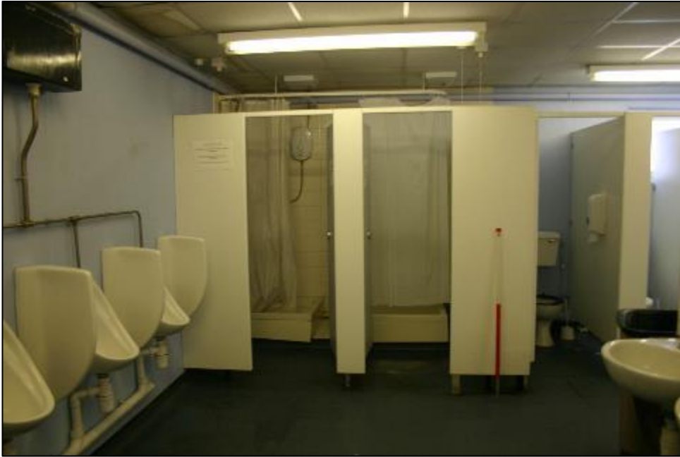
Plate 15: GF11 Men's toilet and shower room, looking north, 1980's toilet fittings
