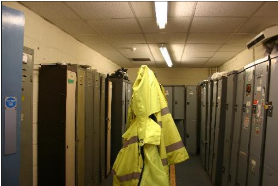
Plate 27: GF18 changing room, looking east
