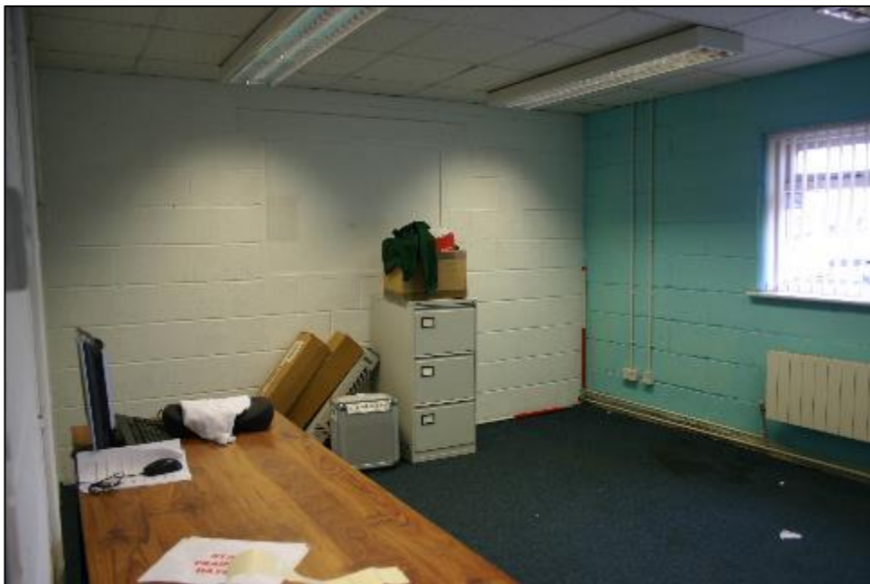
Plate 24: GF16 small office, looking north-west
