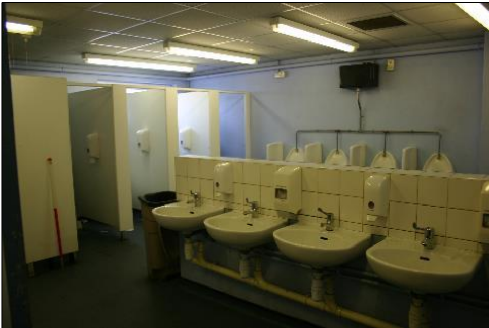
Plate 16: GF11 Men's toilet and shower room, looking north-east
