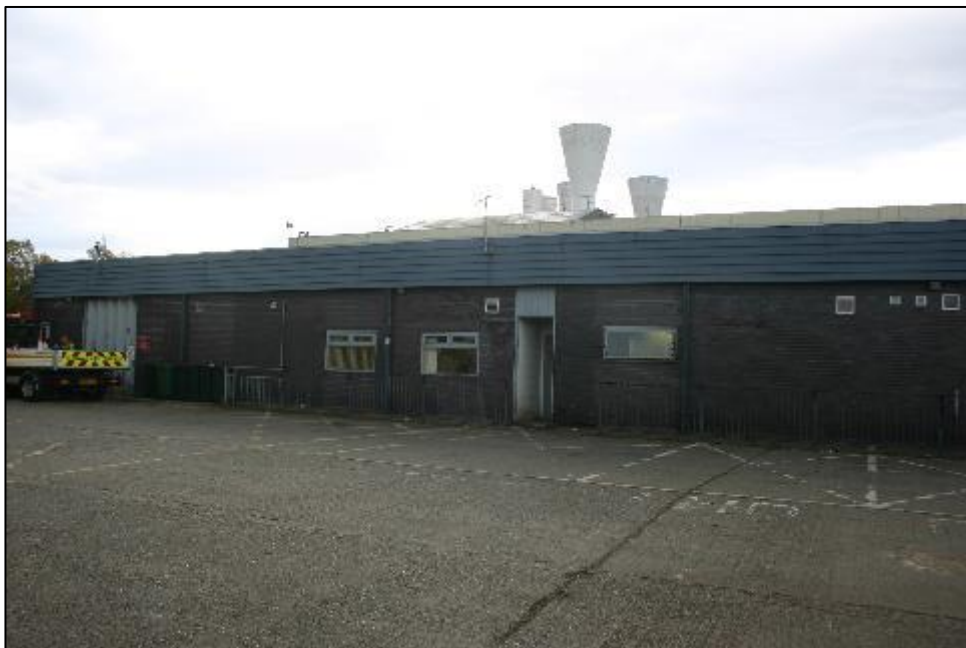
Plate 4: Eastern end of the north facing elevation, visible repairworks
