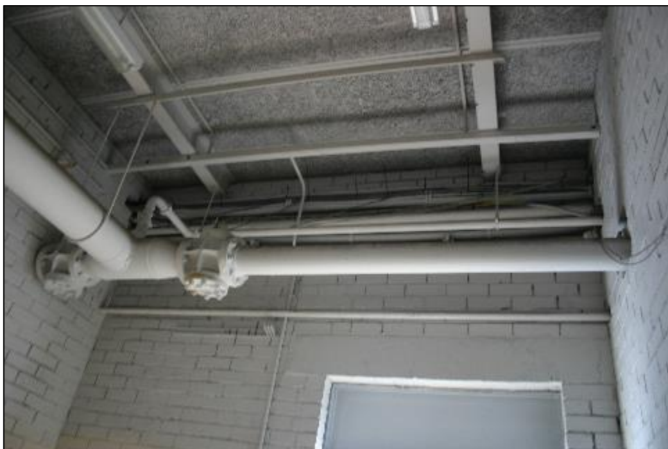
Plate 34: GF24 storage room, large pipework at upper level, looking south
