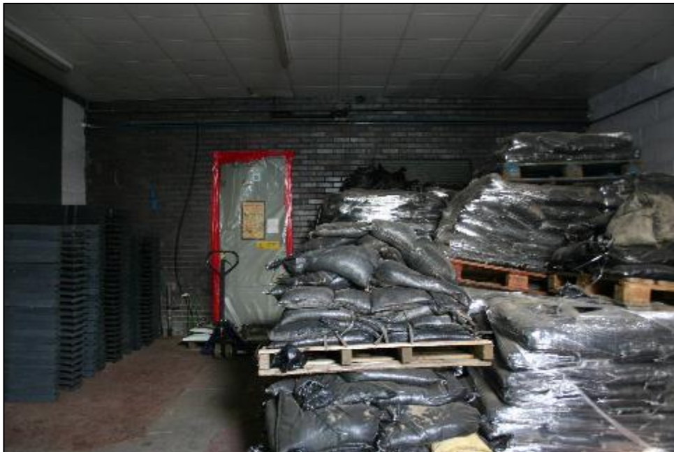
Plate 38: GF27 loading bay, looking south to former exterior elevation and sealed off doorway
