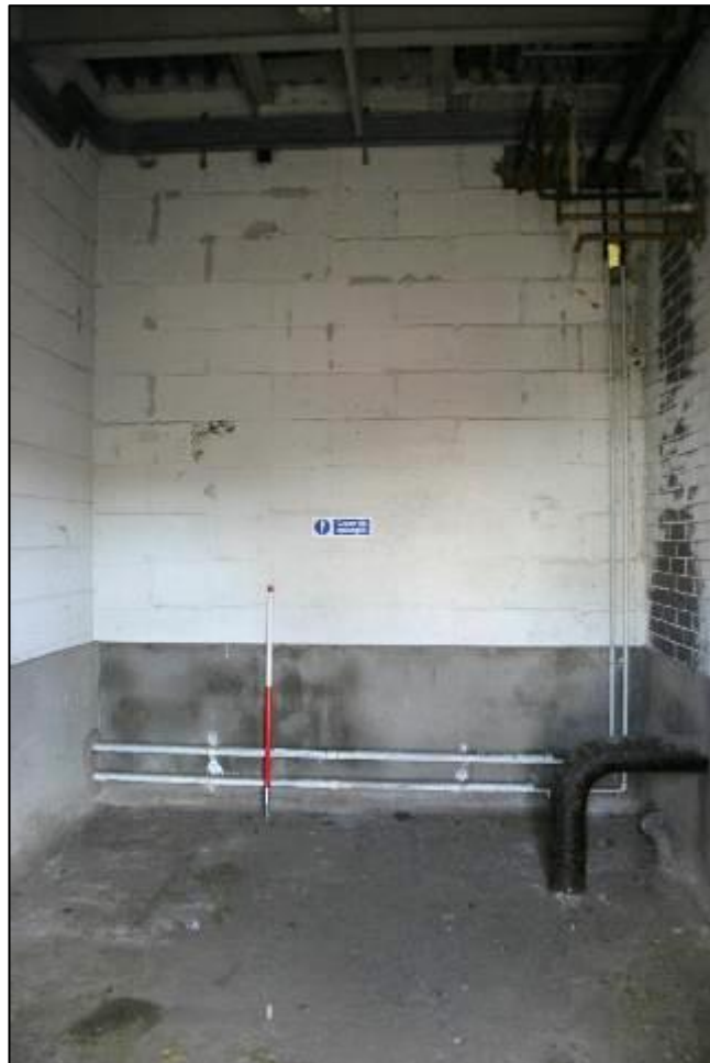
Plate 30: GF21 storage room, large pipe at south elevation
