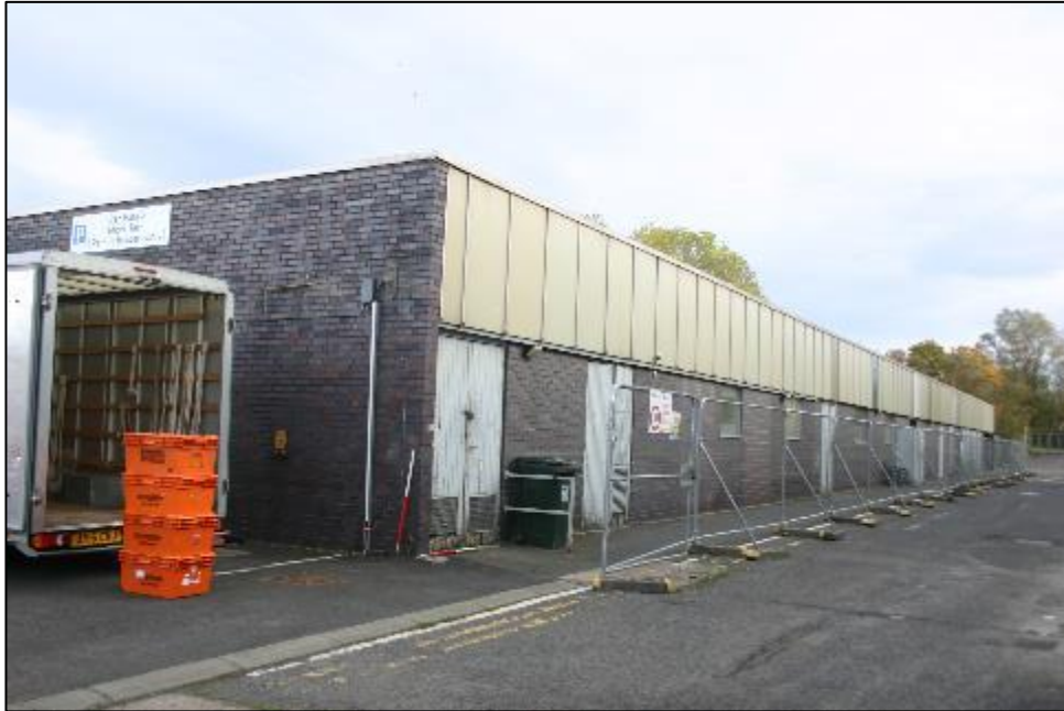
Plate 1: South facing elevation, bricked up doorways visible at the western section
