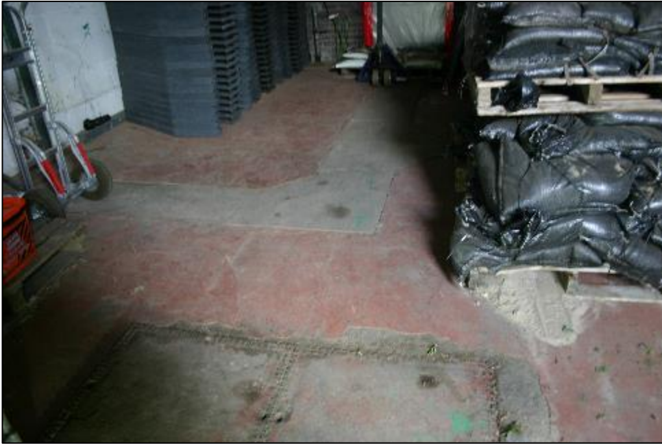
Plate 39: GF27 loading bay, tracks in concrete flooring, looking south
