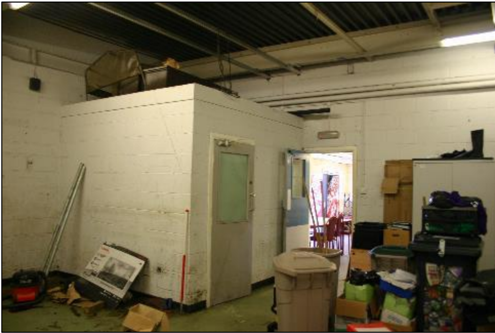
Plate 29: GF19 looking towards GF20 built into north-east corner
