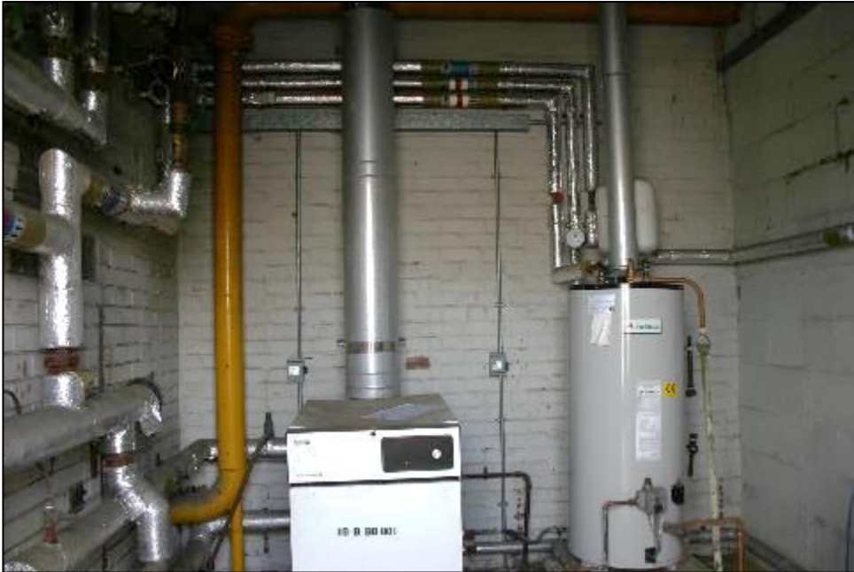
Plate 31: GF22 boiler room, general view looking east
