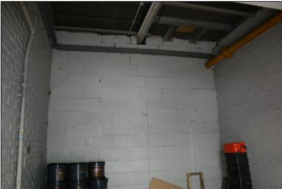
Plate 36: GF25 storage room, looking north
