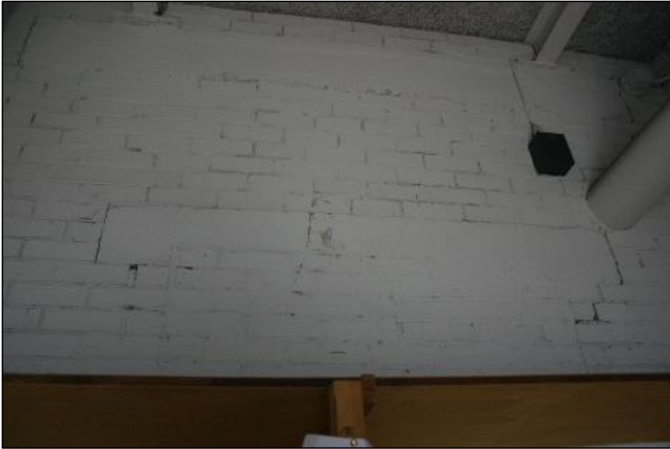
Plate 35: GF24 concrete lintel of blocked door below concrete support of roof steel beams
