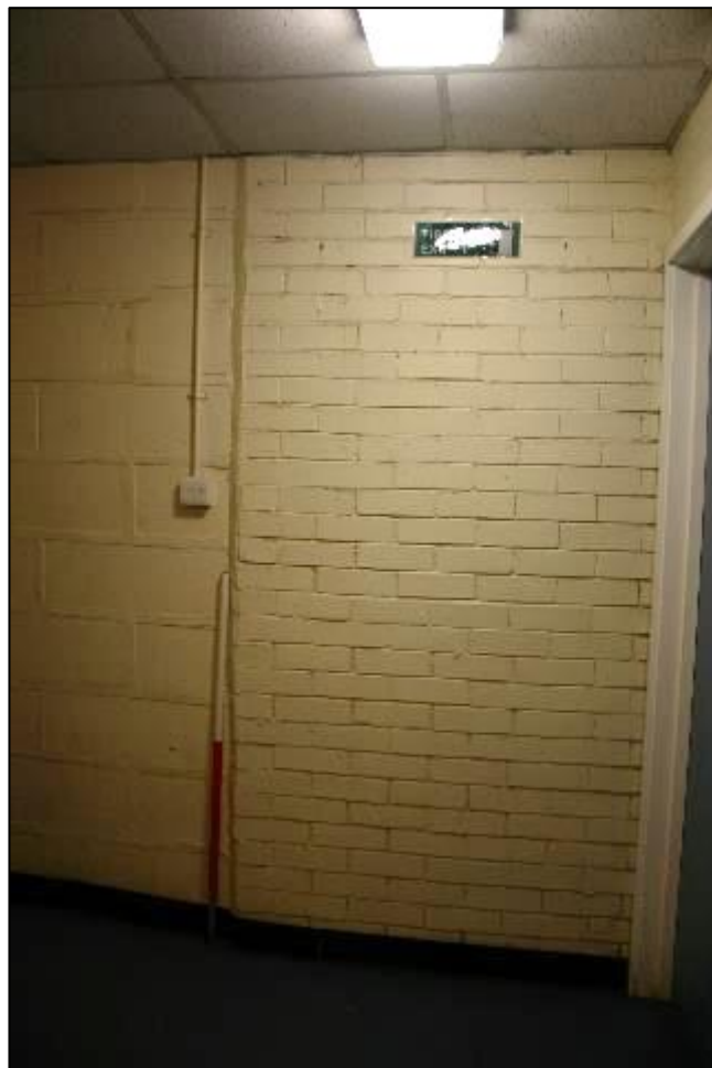
Plate 10: GF3, change between original brick and added concrete breeze blocks
