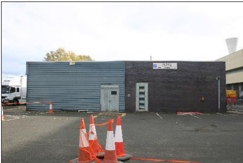
Plate 2: West facing elevation
