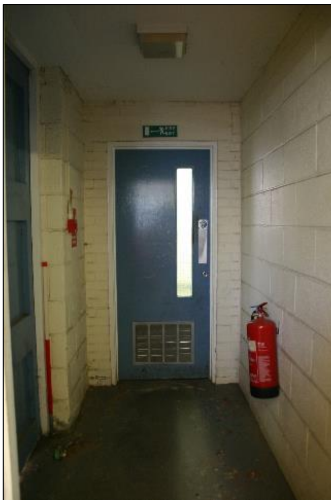
Plate 21: GF14, hallway, looking west
