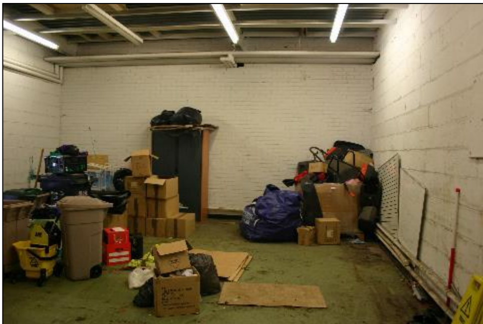
Plate 28: GF19 storage area, looking south to former external wall
