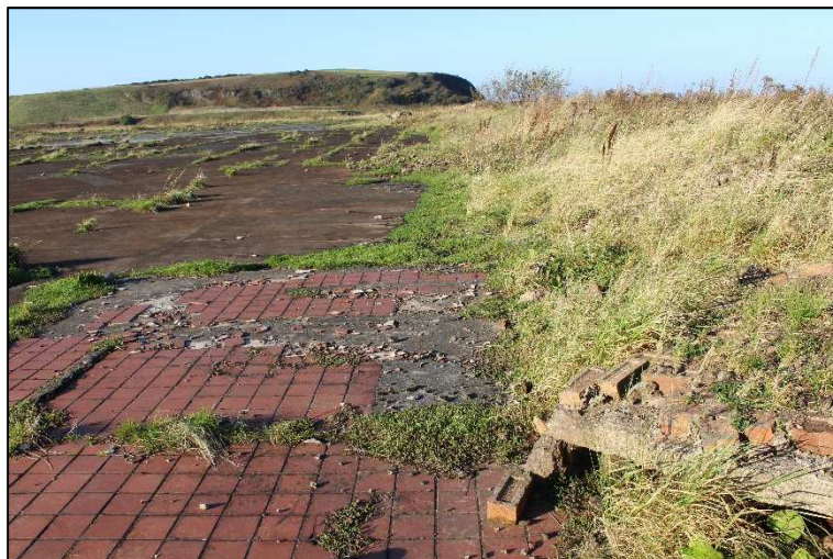
Plate 22: Example of surviving former floor surface at Marchon Works (Asset 25)
