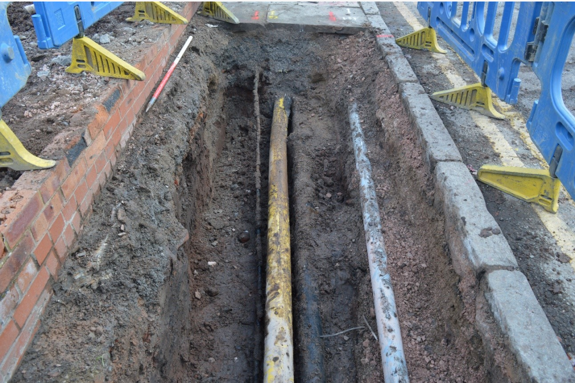
Picture Taken: Plate No. 40 Title: Excavation for gas diversion in western extent of Hunter Street, looking east with 1m scale
