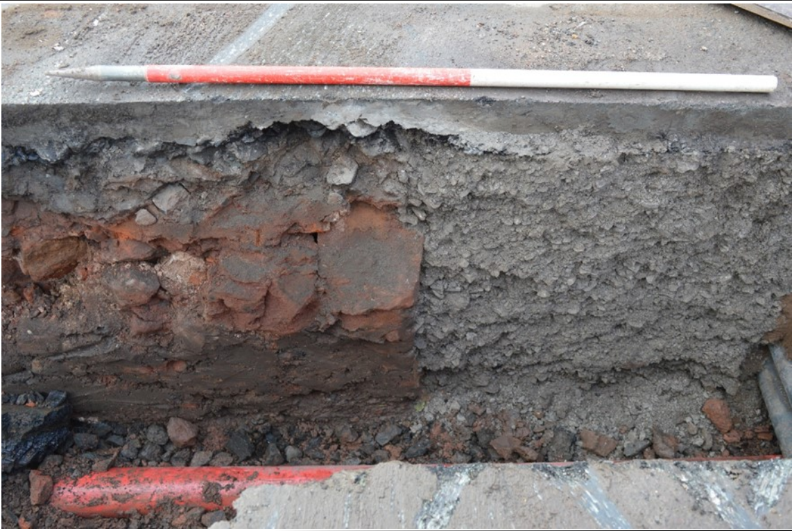
Picture Taken: Plate No. 37 Title: East-facing section of electric service trench through Hunter Street, with 1m scale
