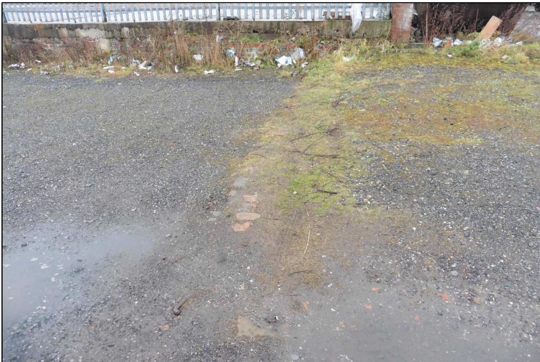
Plate 4: Remains of brick wall, northern car park
