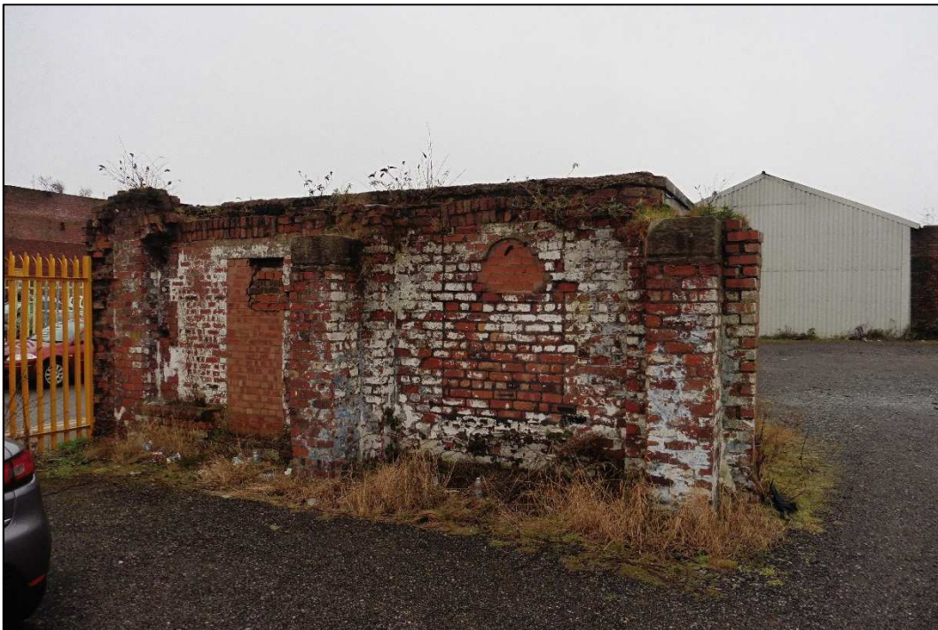
Plate 6: Upstanding brick structure in northern car park (western elevation)
