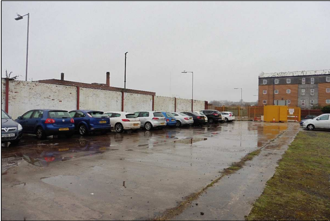
Plate 5: Brick wall bounding north-eastern boundary of the northern car park
