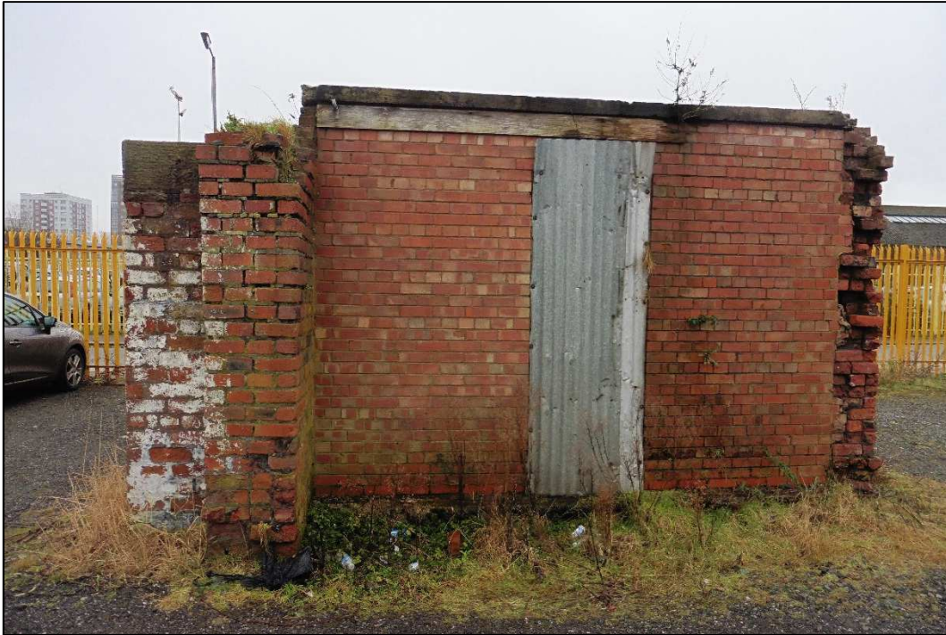
Plate 7: Upstanding brick structure in northern car park (northern elevation)
