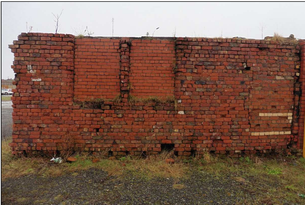
Plate 8: Upstanding brick structure in northern car park (western elevation)
