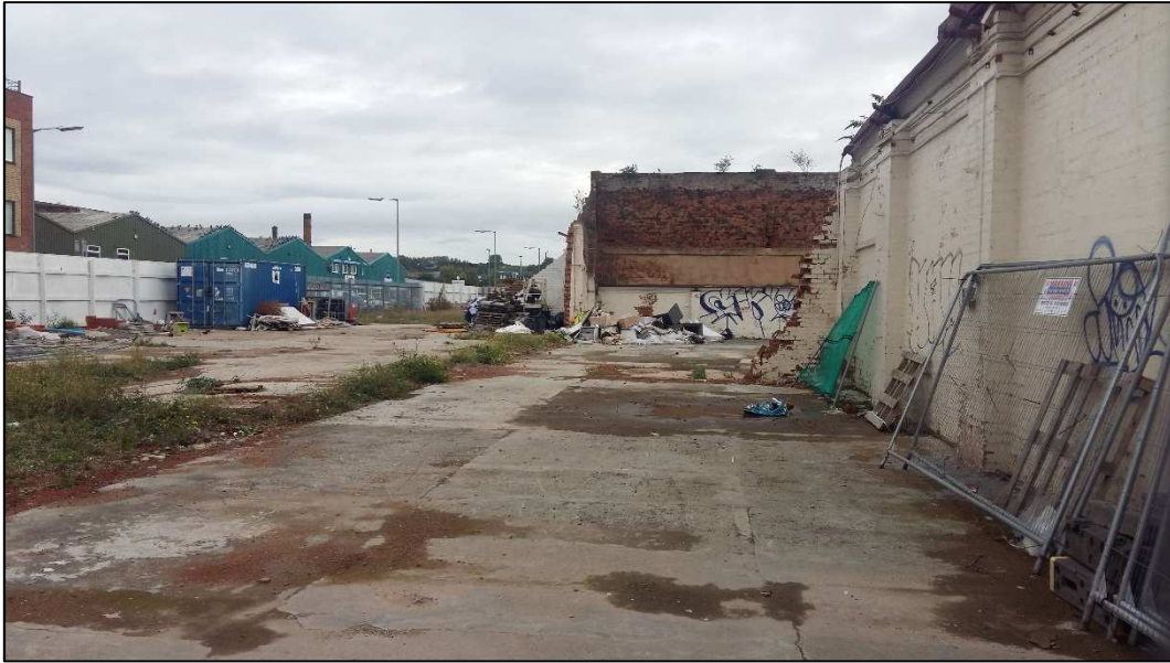
Plate 9: Cleared land in north-west of the Site
