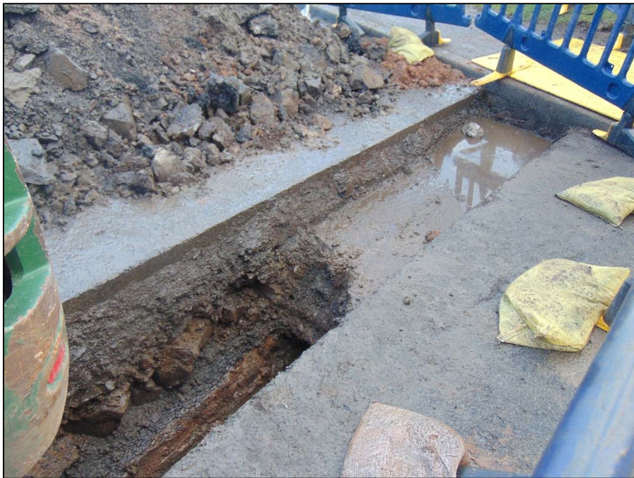
Plate 2; Trench showing modern cut [106] and concrete block (103), Facing North East
