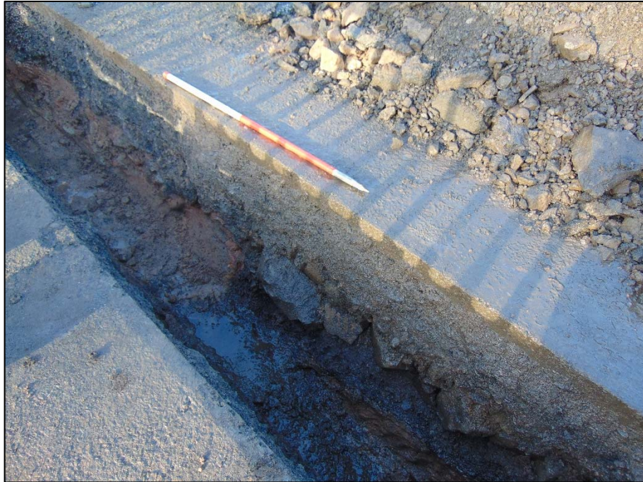
Plate 1; Trench showing modern cut [106], Facing North West, 1m Scale.
