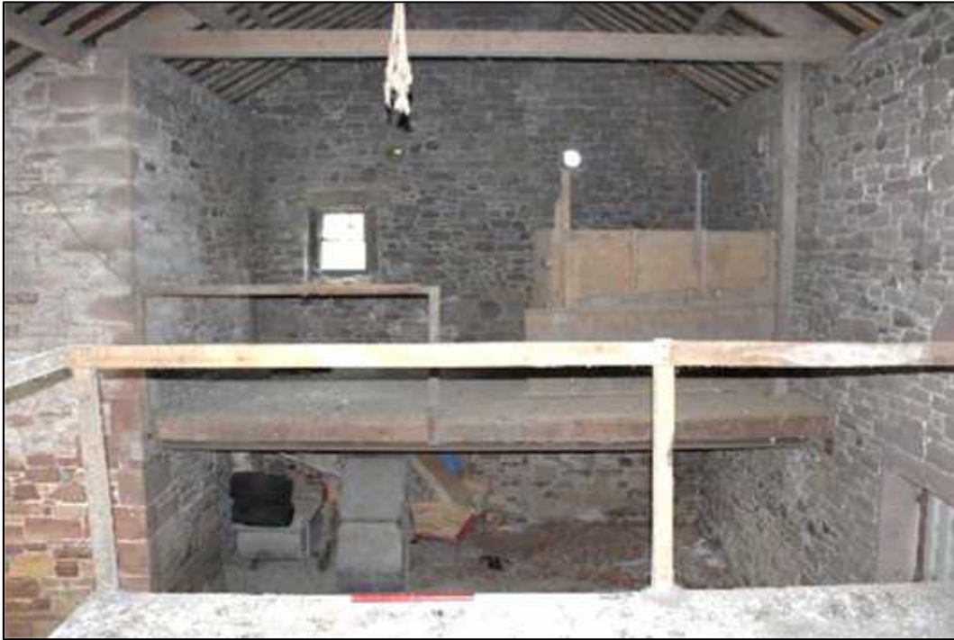
Plate 21: Interior of Building B, northern extent, showing inserted floor above north bay (Feature 117)
