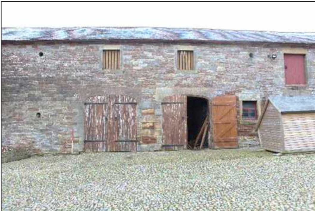
Plate 28: West elevation of Building B, central section
