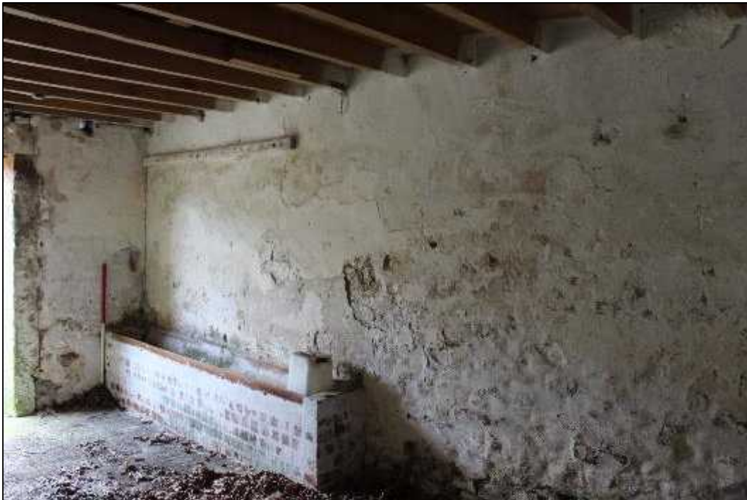
Plate 81: Building F, penultimate southern area, south elevation
