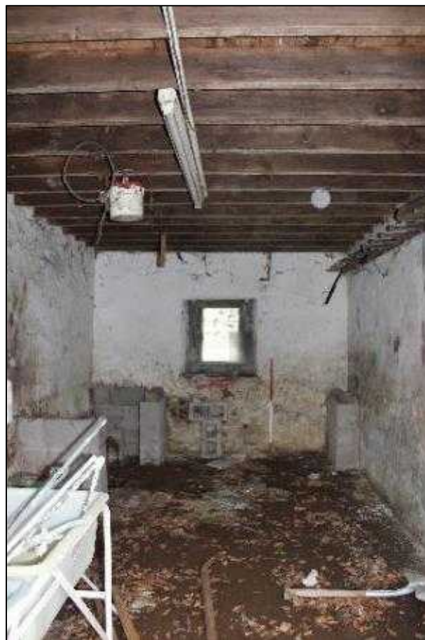
Plate 32: Building B: central section, interior of southern cart entranceway, east elevation
