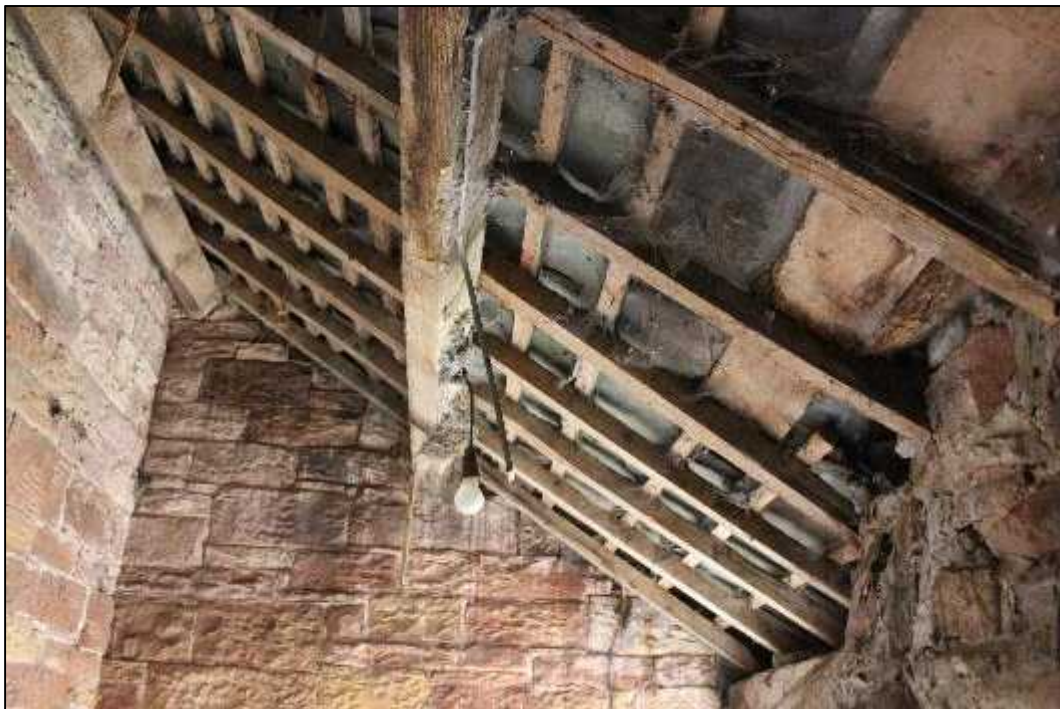
Plate 46: Link Building A/B, interior, roof structure
