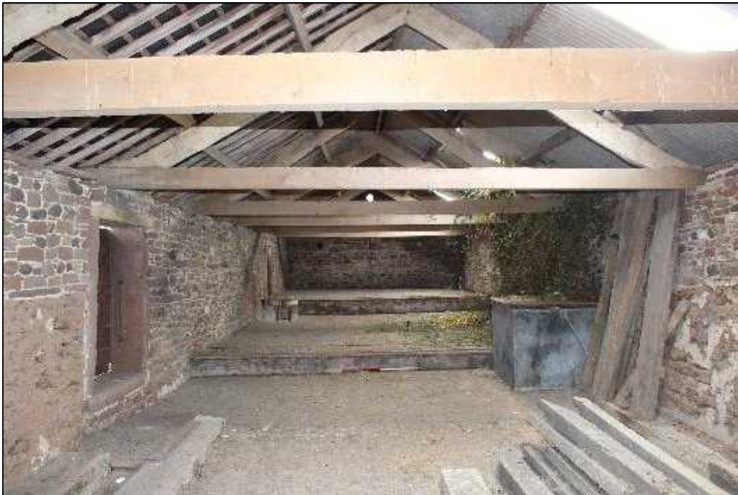
Plate 83: Building F, loft space, south elevation and stepped levels
