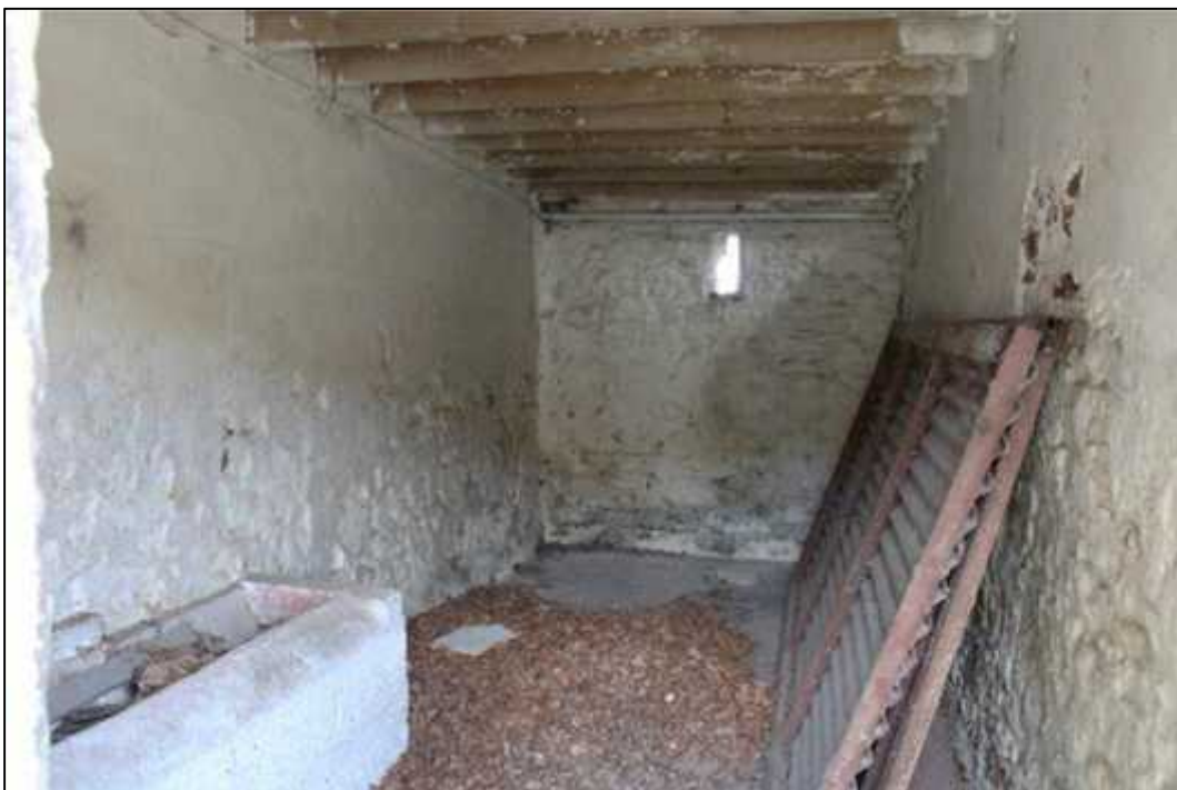
Plate 82: Building F, southern extent, south and west elevations
