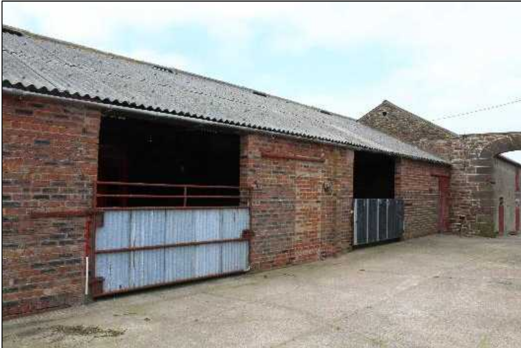
Plate 97: Building G, exterior, east elevation, oblique
