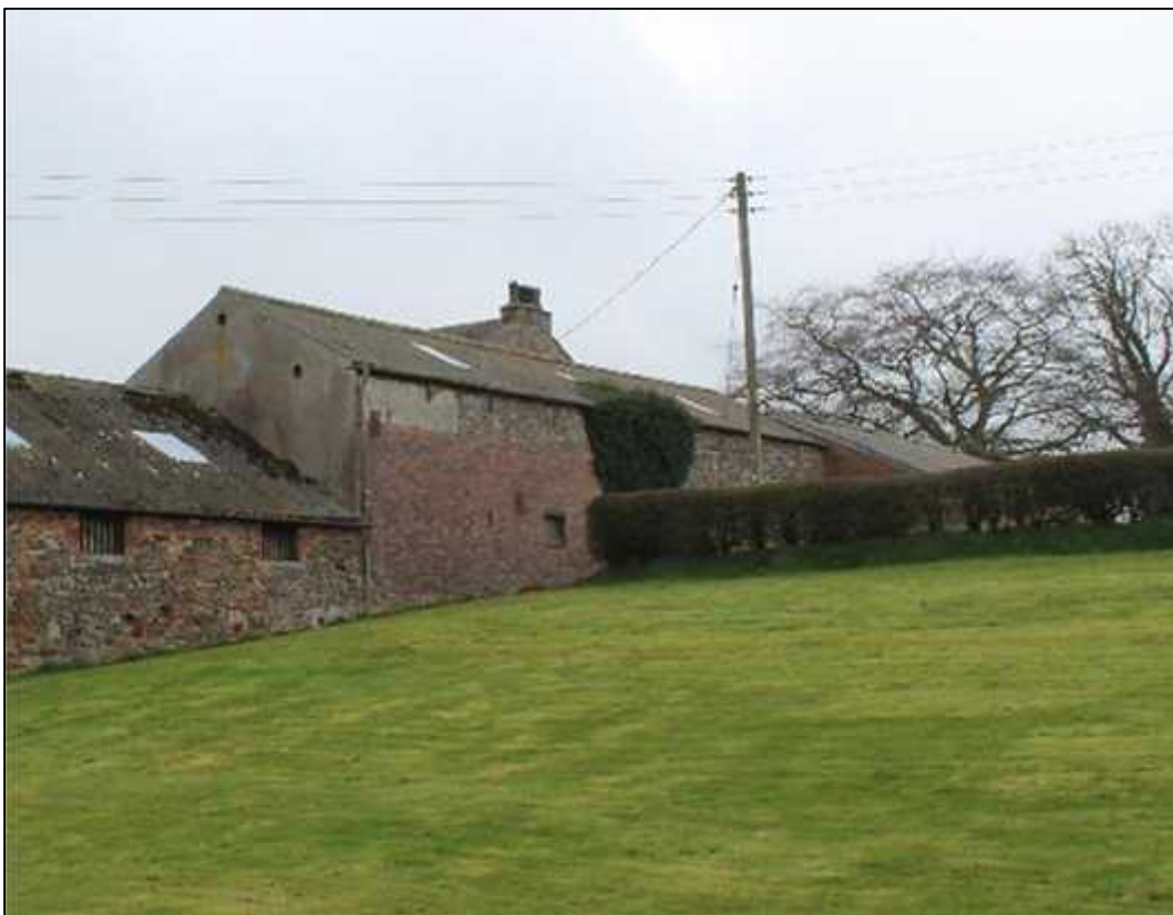
Plate 64: Building F, west elevation
