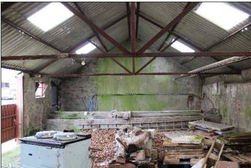
Plate 60: Building E, interior, south elevation
