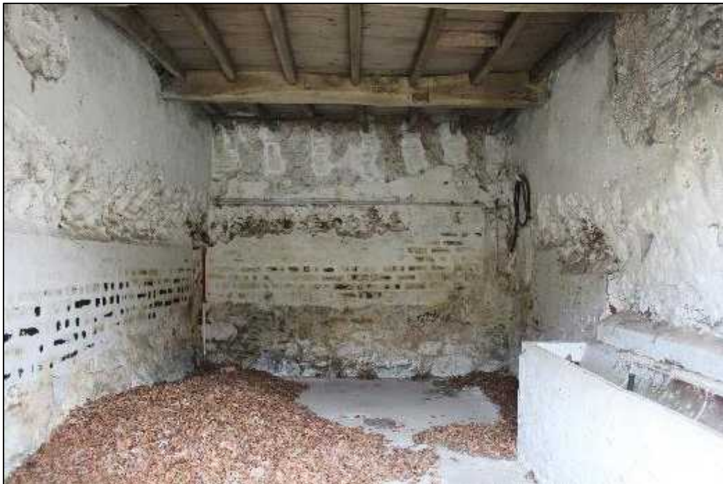
Plate 66: Building F, interior, northern extent, west elevation
