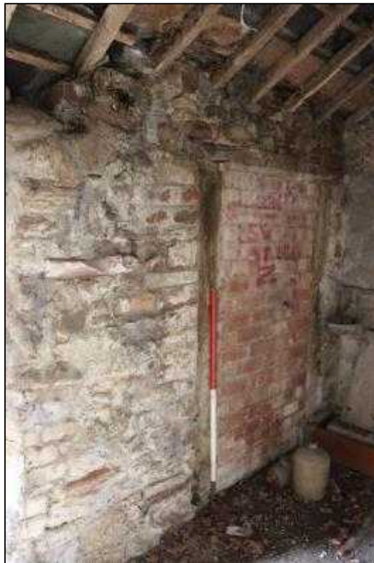
Plate 44: Link Building A/B, interior, west elevation (Feature 102)
