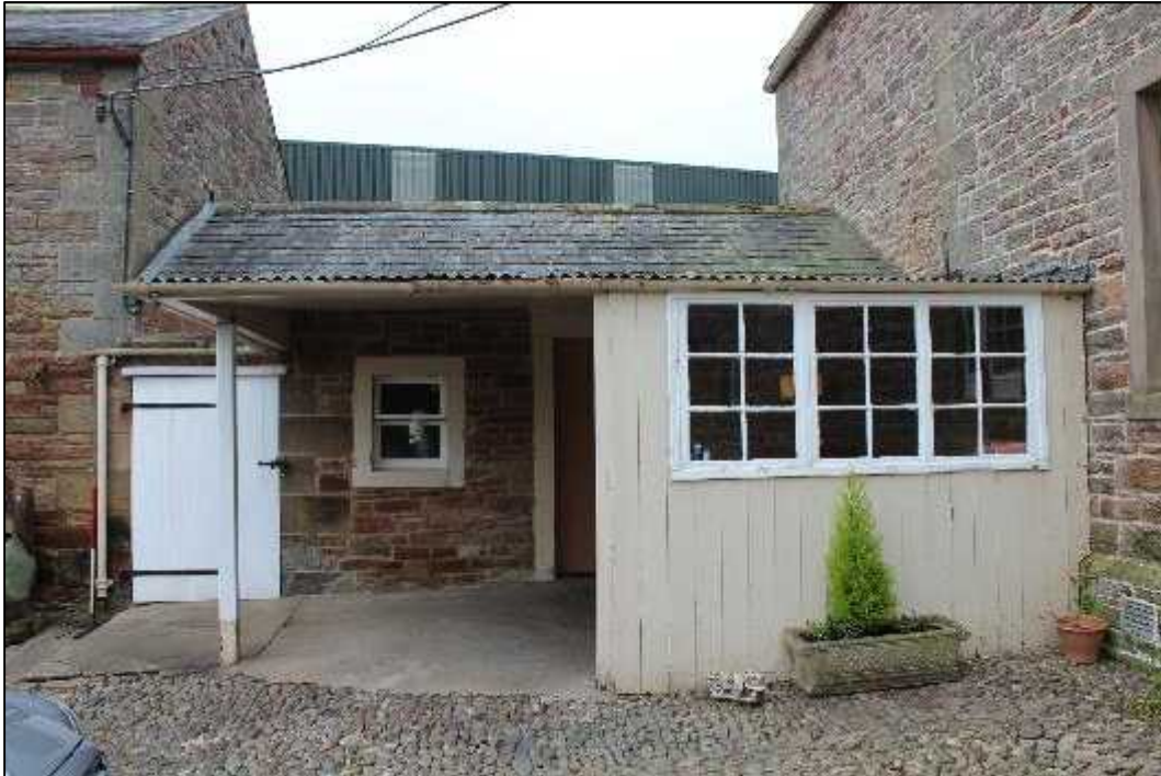
Plate 47: Building C, west elevation
