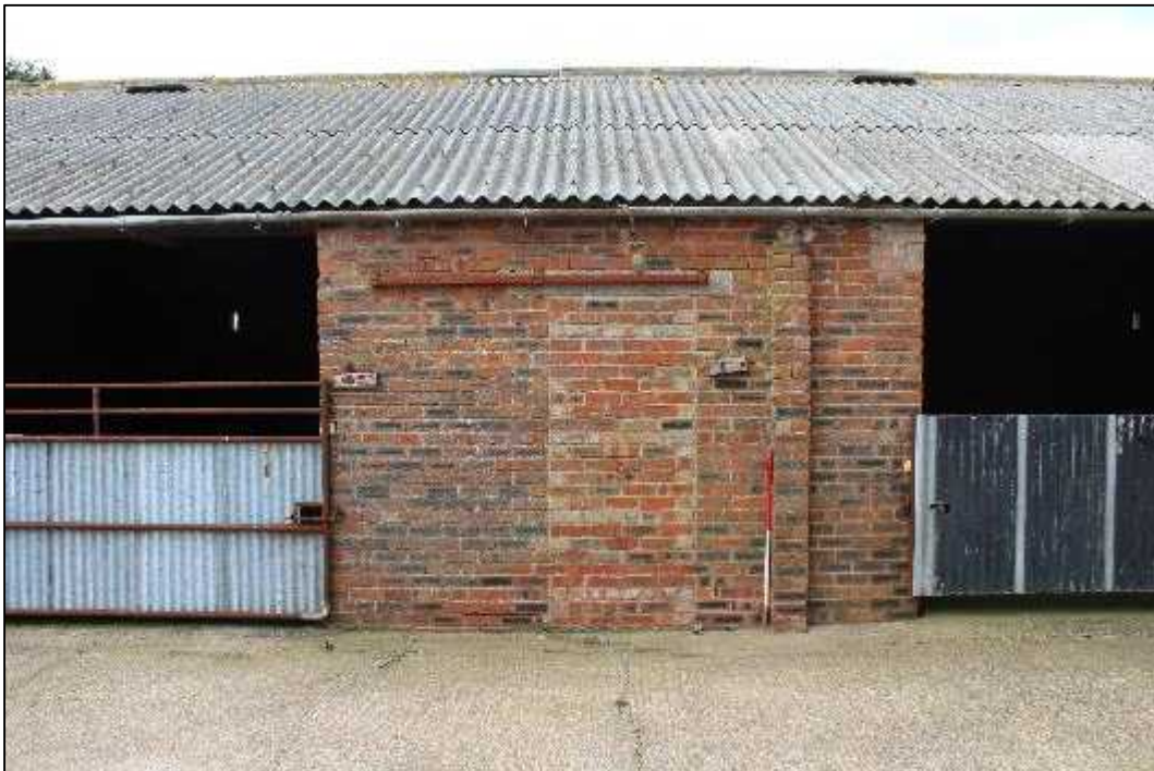
Plate 98: Building G, exterior, east elevation, former doorway (Feature 112)
