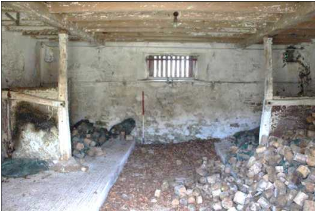
Plate 75: Building F, southern byre, west elevation with window, stalls and boskins
