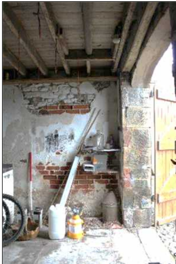
Plate 30: Building B: central section, interior of northern cart entranceway, south elevation
