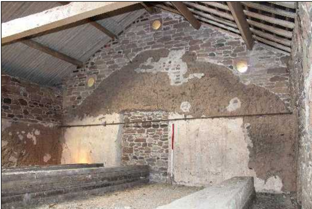
Plate 86: Building F, loft space, north elevation (Feature 111)
