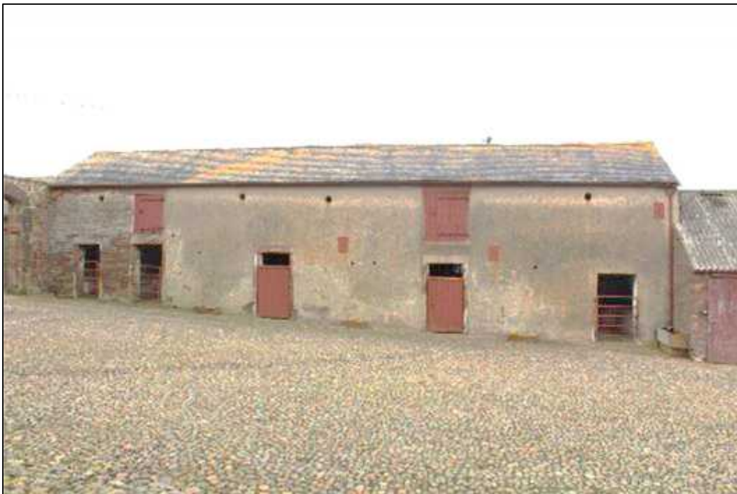
Plate 62: Building F, east elevation
