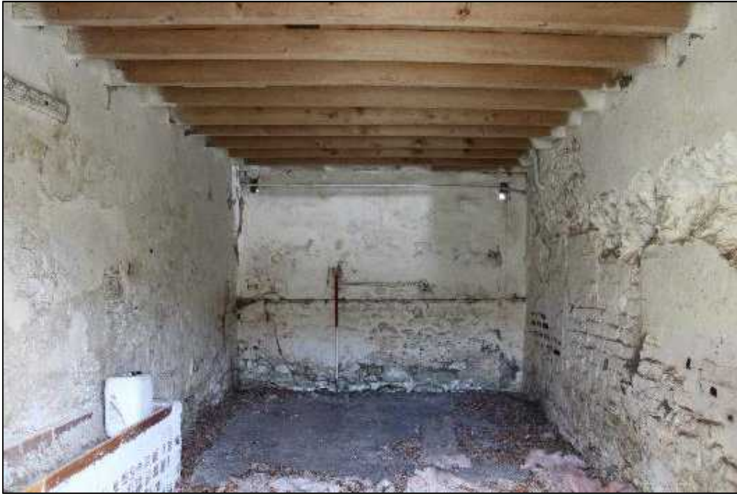
Plate 79: Building F, penultimate southern area, west elevation
