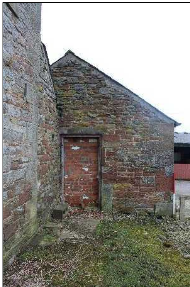
Plate 6: West elevation of Building A (showing Feature 101)
