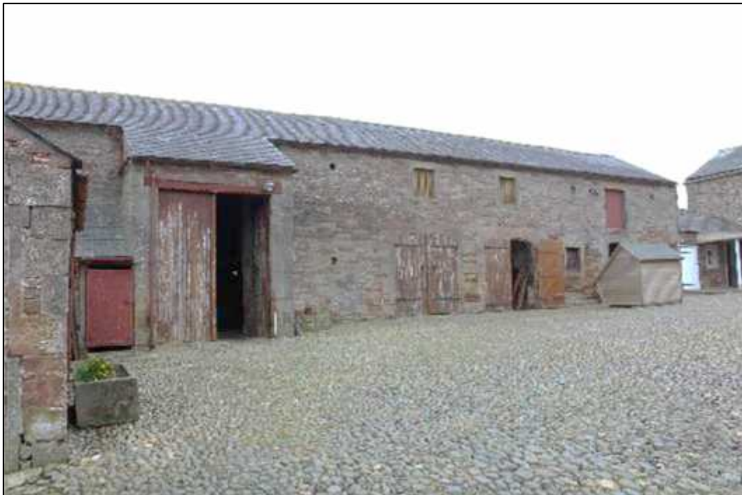
Plate 16: West elevation of Building B, oblique, south-eastwards
