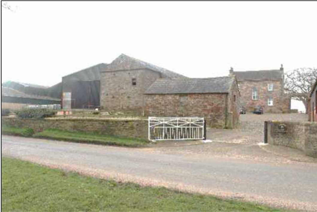
Plate 1: General view of Buildings A, B and farmhouse with modern agricultural sheds to the east
