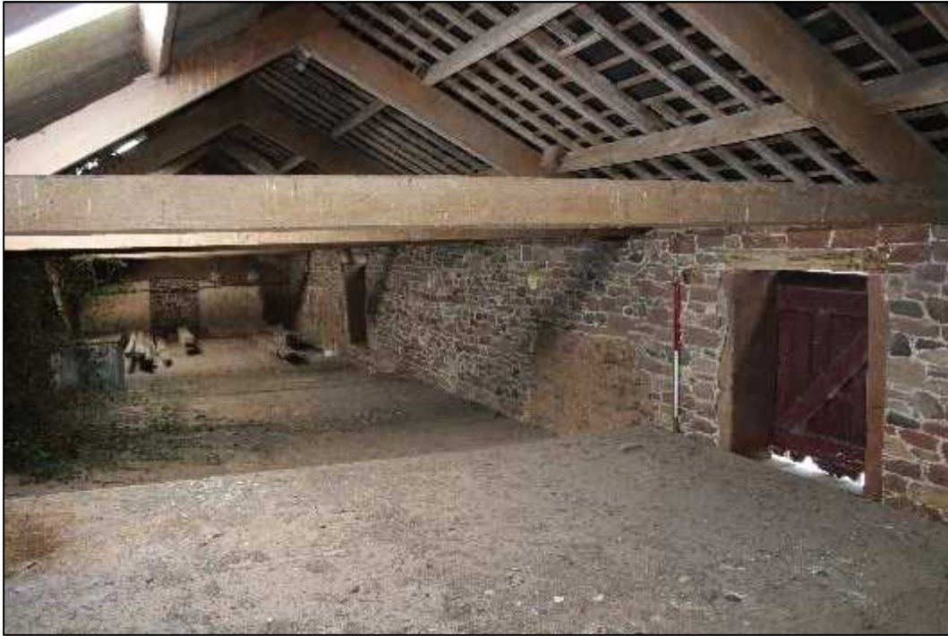
Plate 85: Building F, loft space, east and south elevations
