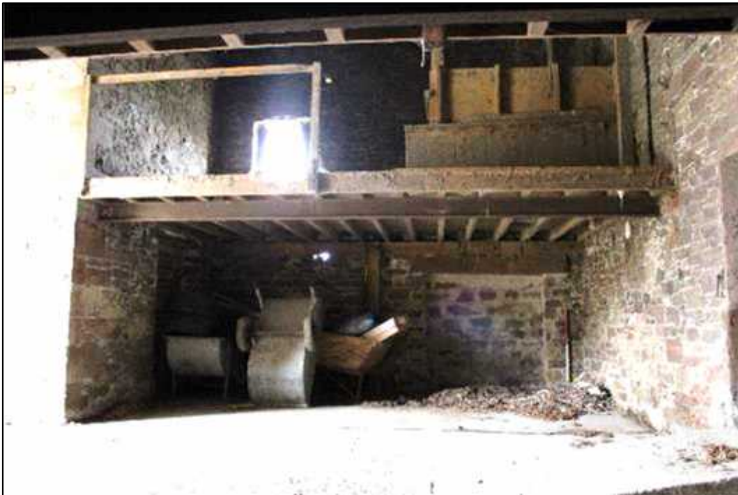
Plate 25: Interior of Building B, northern extent, showing lintel above recessed area (Feature 116)
