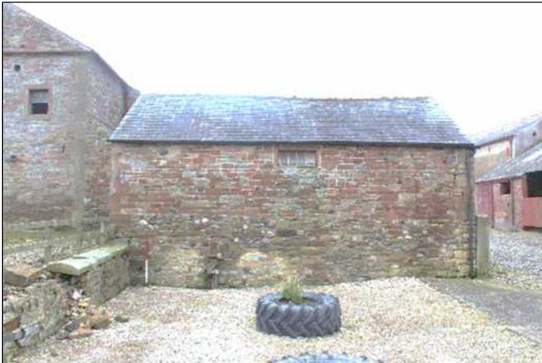
Plate 5: North elevation of Building A (showing Feature 118)
