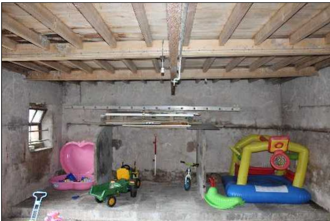
Plate 40: Building B: southern section, interior, showing north elevation
