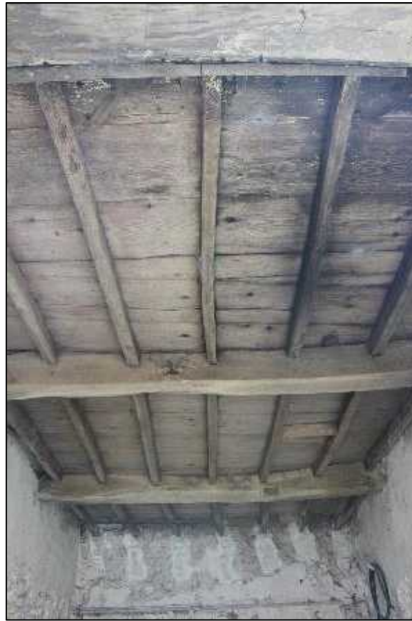
Plate 67: Building F, interior, northern extent, ceiling, facing west (Feature 108)
