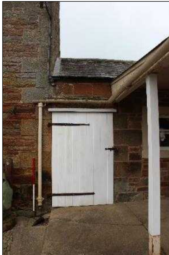
Plate 48: Building C, west elevation, northern doorway
