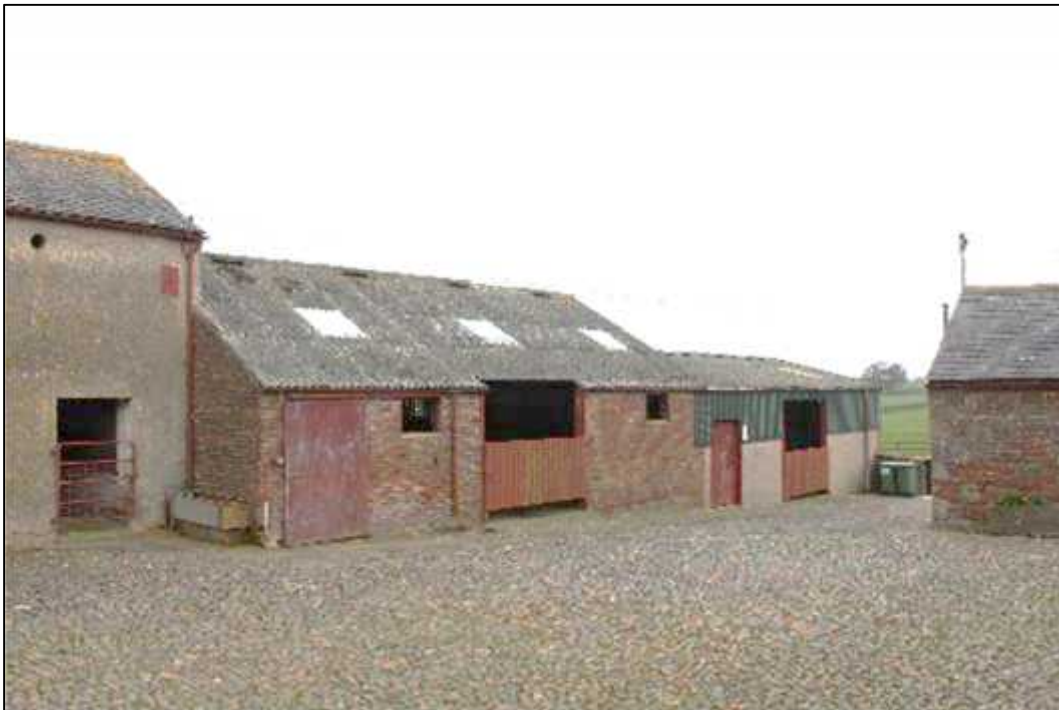
Plate 58: Building E, east and south elevations
