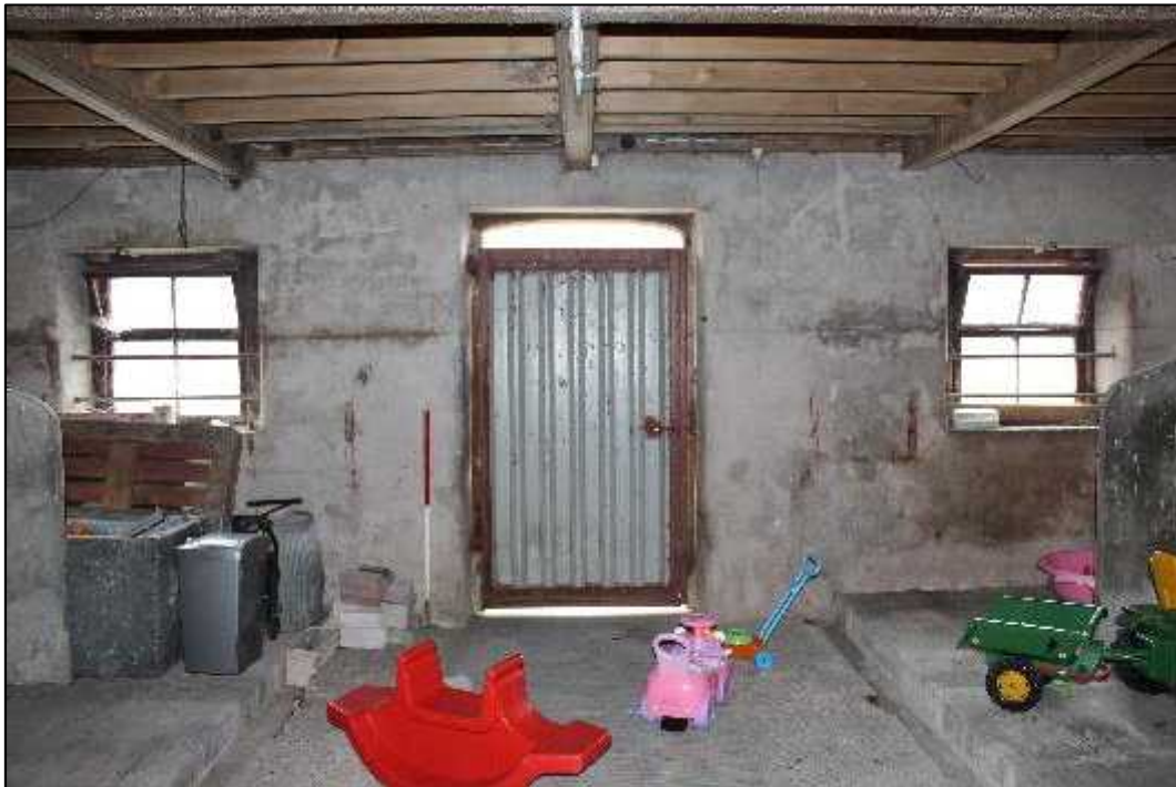
Plate 39: Building B: southern section, interior, showing west elevation
