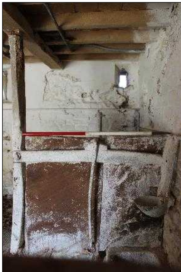
Plate 72: Building F, northern byre, detail of boskin (Feature 109)
