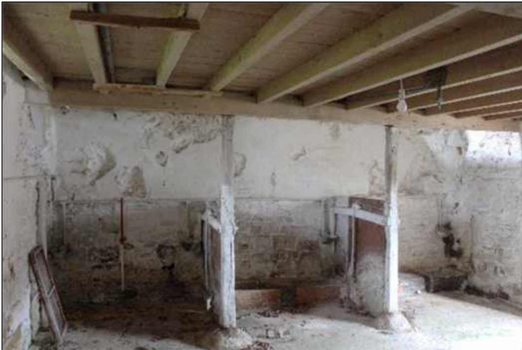
Plate 73: Building F, northern byre, detail of stalls and boskins (Feature 109)
