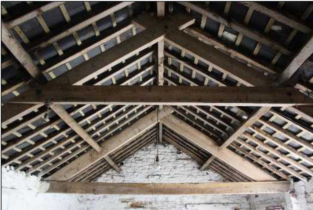
Plate 9: Interior of Building A showing roof structure
