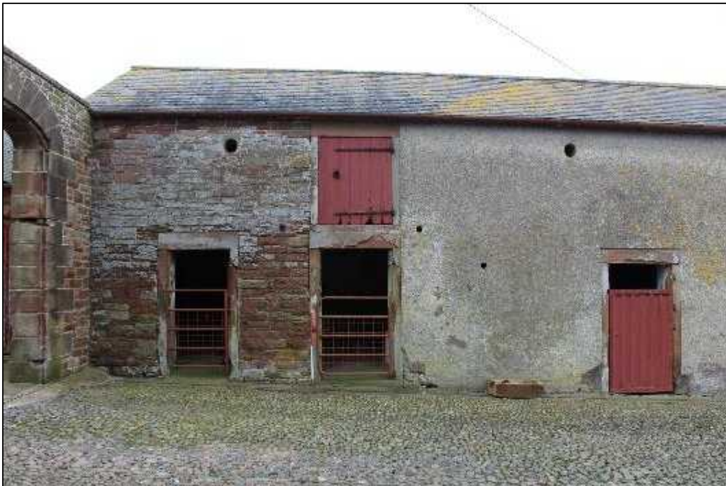
Plate 78: Building F, exterior, east elevation, southern extent
