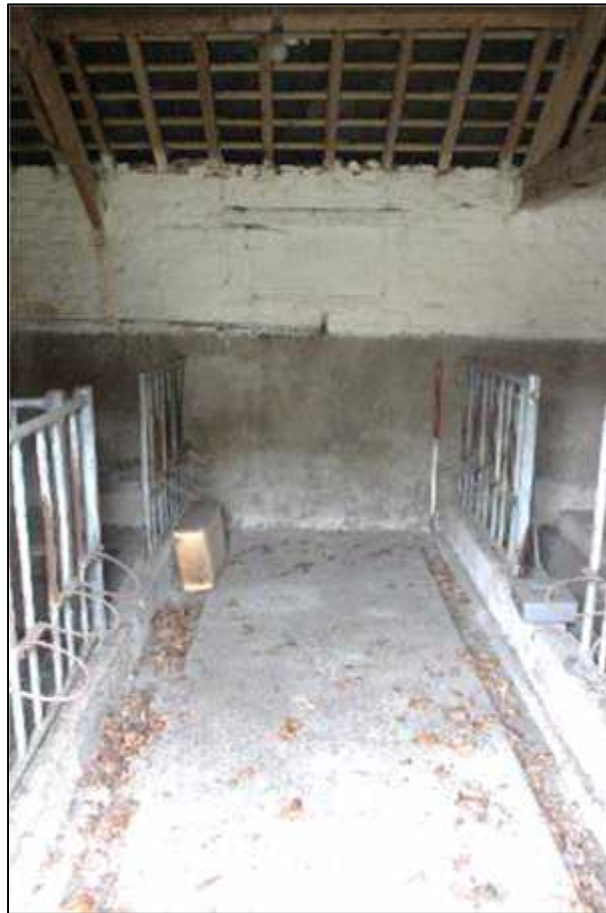
Plate 11: Interior of Building A showing north elevation
