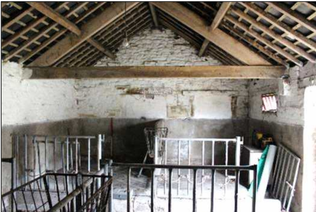
Plate 10: Interior of Building A showing east elevation (and Features 102 and 103)
