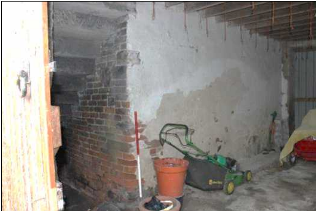
Plate 29: Building B: central section, interior of northern cart entranceway, north elevation
