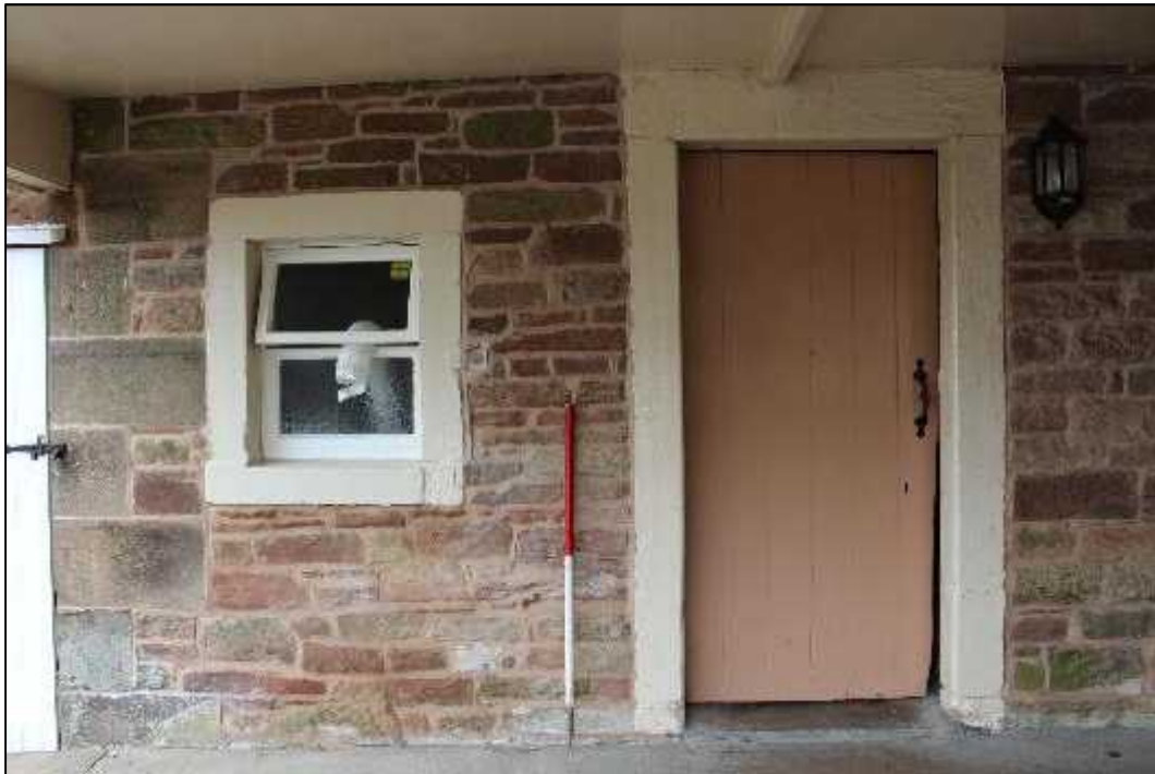
Plate 51: Building C, west elevation, southern doorway
