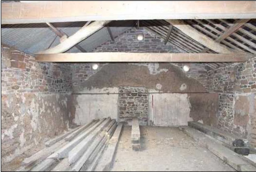
Plate 87: Building F, loft space, north elevation (Feature 111)
