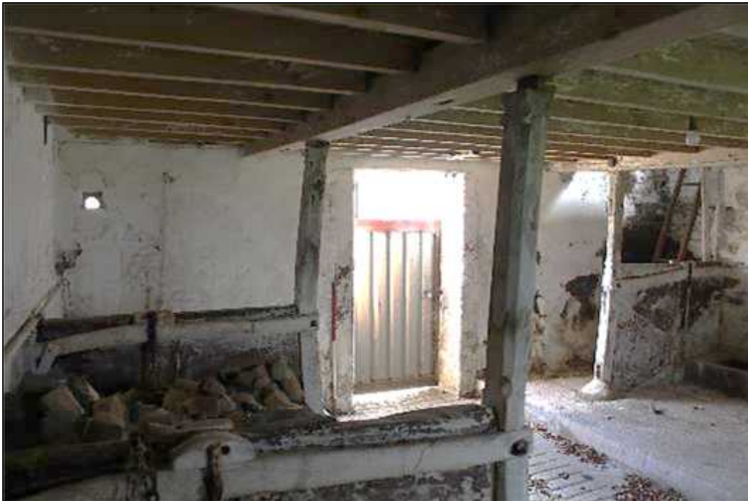
Plate 77: Building F, southern byre, east elevation with door, stalls and boskins (Feature 109)
