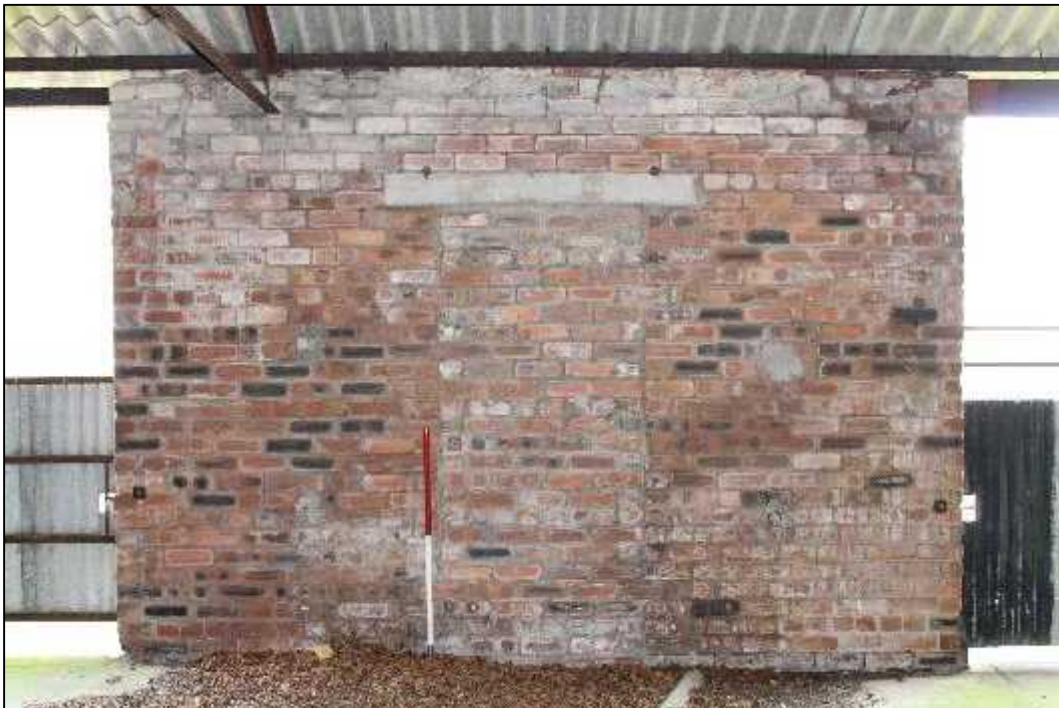
Plate 100: Building G, interior, former doorway, east elevation (Feature 112)
