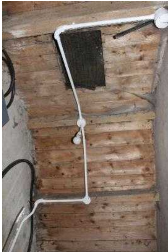
Plate 50: Building C, interior of northern area showing roof structure
