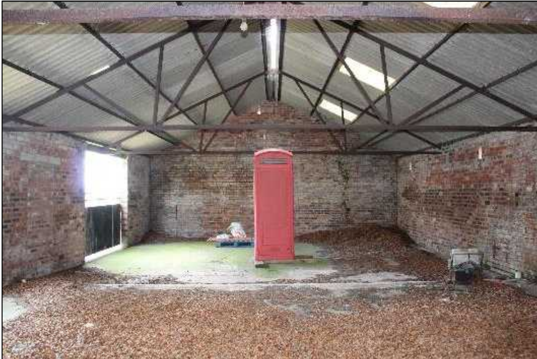
Plate 99: Building G, interior, south elevation
