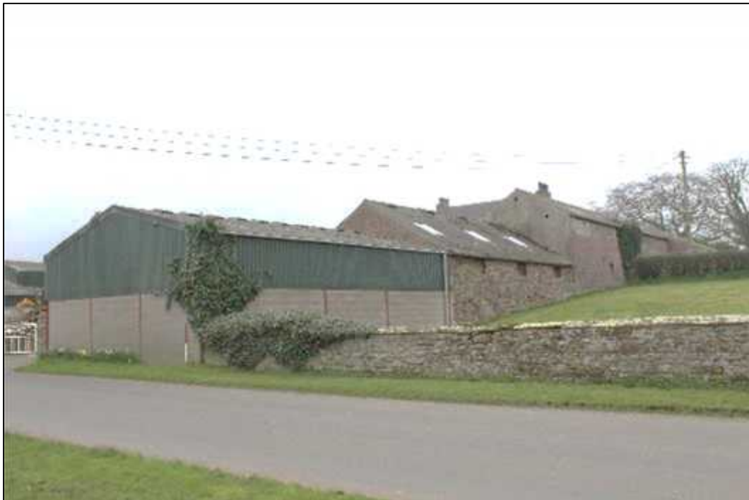
Plate 54: Building D, north and west elevations
