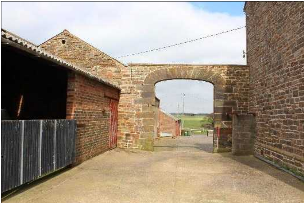
Plate 63: Archway and south elevation of Building F
