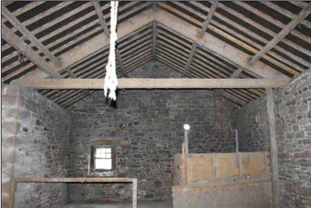
Plate 27: Interior of Building B, northern extent, showing roof structure
