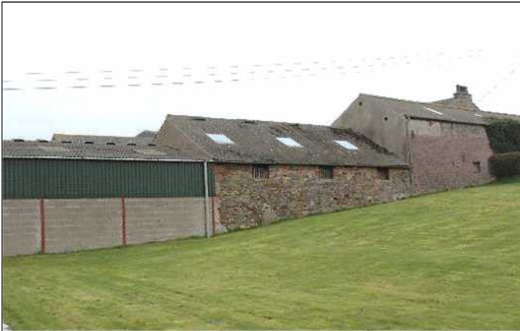
Plate 59: Building E, west elevation (showing Feature 105)
