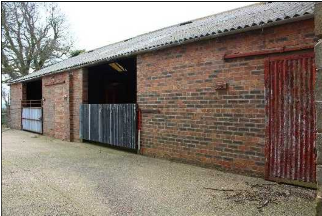
Plate 96: Building G, exterior, east elevation, oblique
