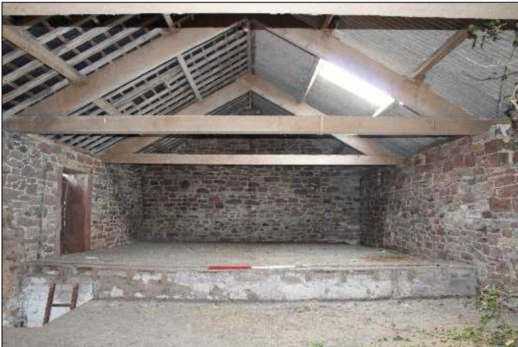
Plate 84: Building F, loft space, south elevation
