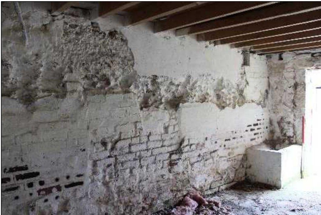
Plate 80: Building F, penultimate southern area, north elevation
