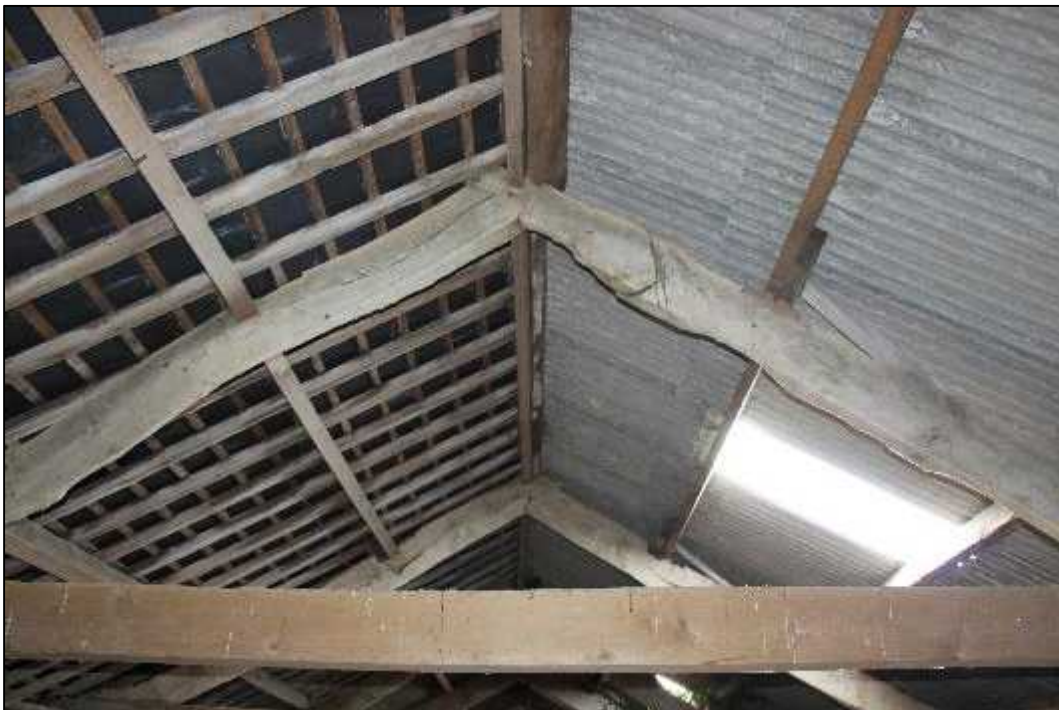
Plate 92: Building F, loft space, roof structure
