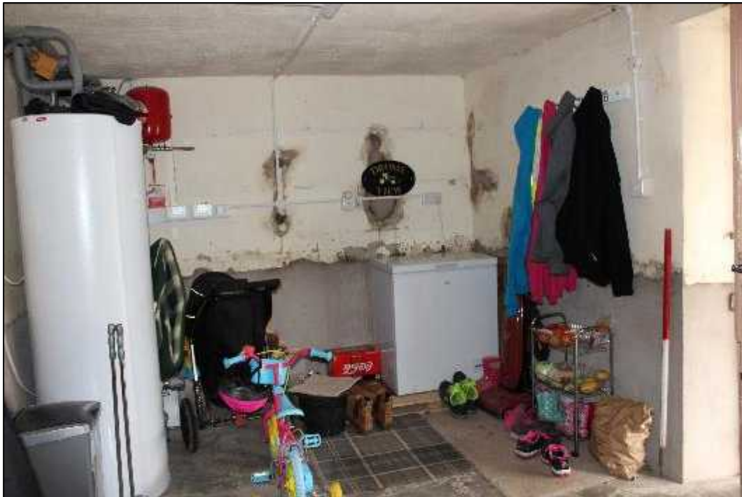
Plate 53: Building C, interior, southern area, south elevation
