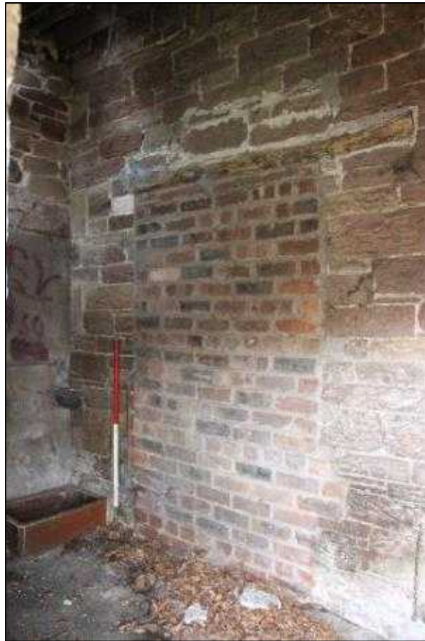
Plate 45: Link Building A/B, interior, east elevation (Feature 103)
