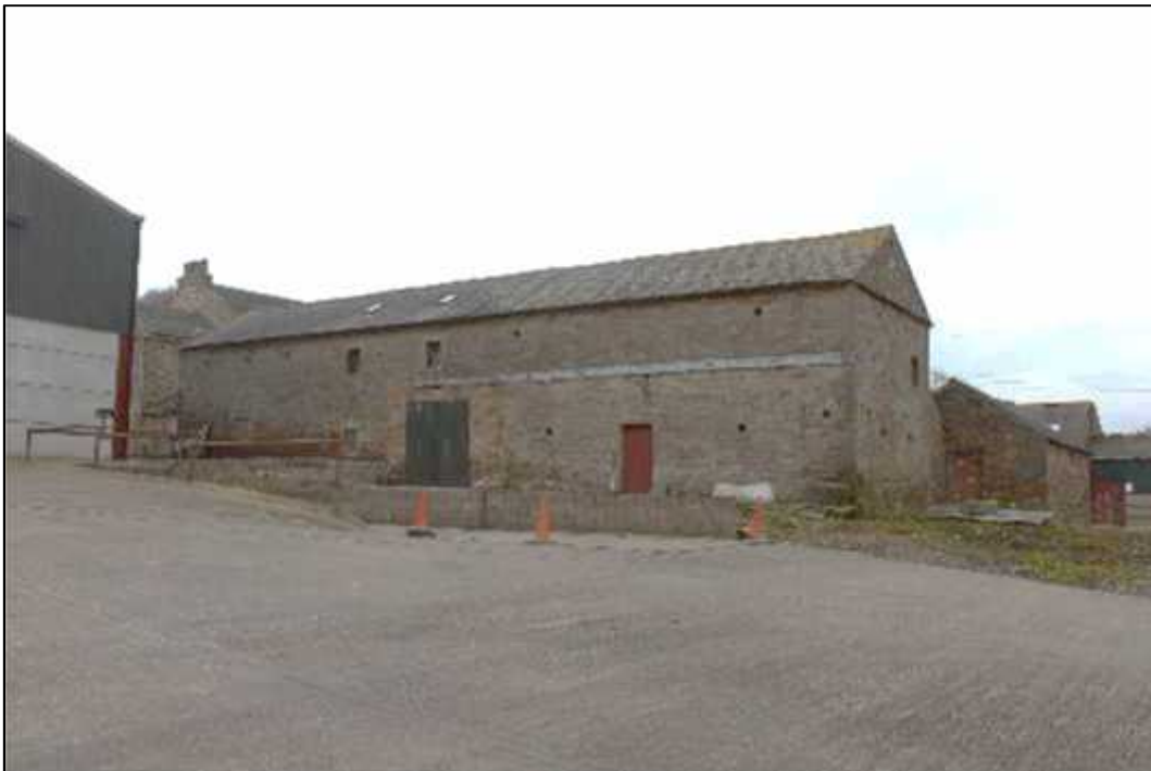
Plate 14: East elevation of Building B, oblique
