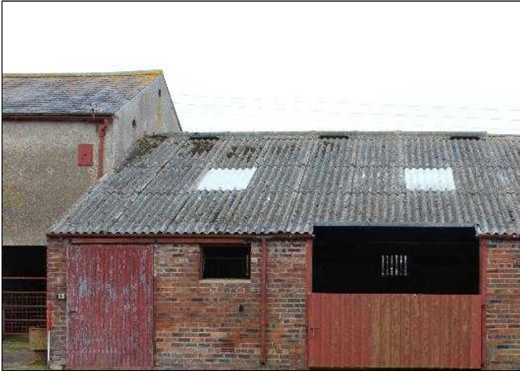
Plate 61: Building F, north elevation adjacent to Building E
