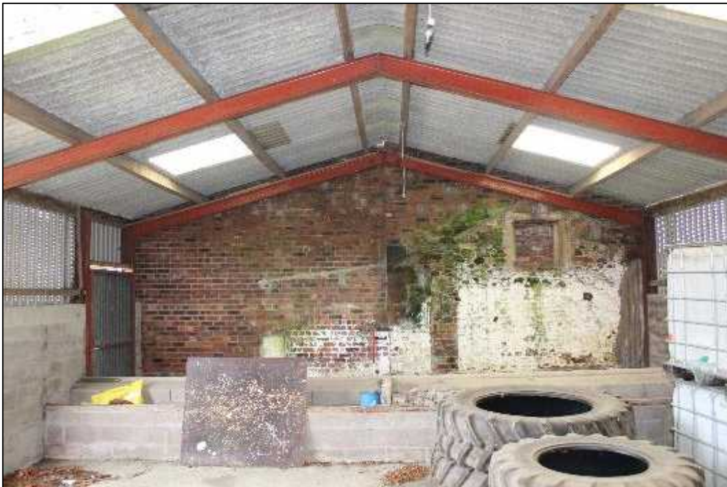
Plate 56: Building D, interior, south elevation (Feature 107)
