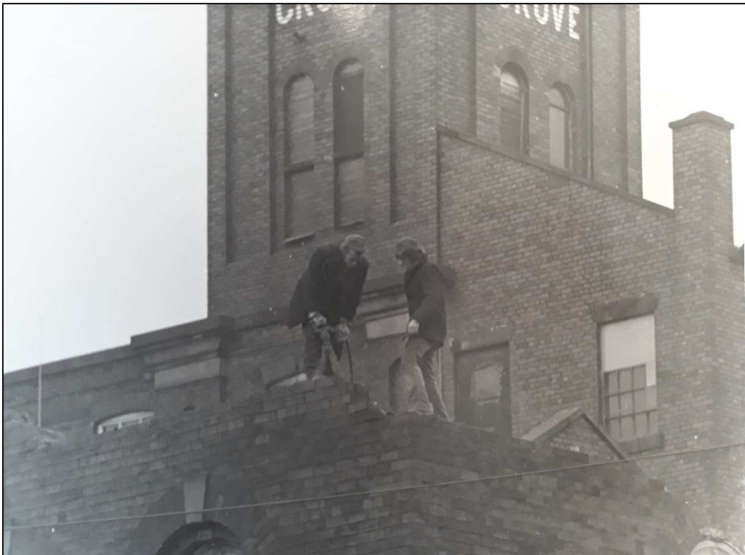
Plate 4: Grove Mill, demolition, 1975 (RLSC RB 443 191 DIG)
