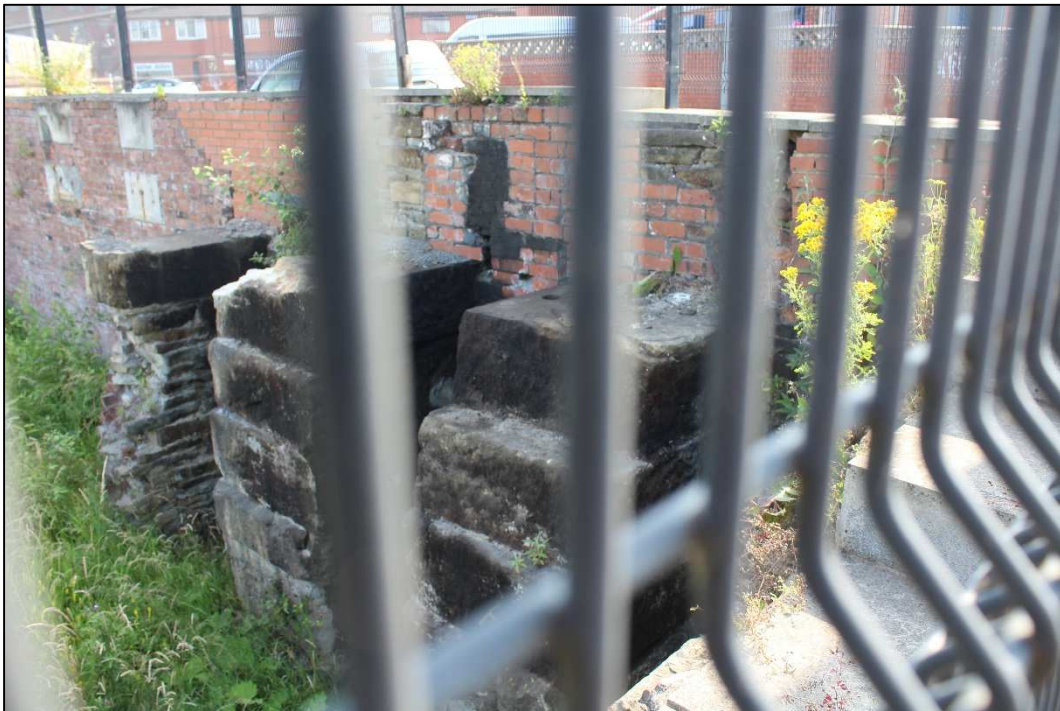
Plate 23: Structural remains within north-western corner of site, facing west-south-west
