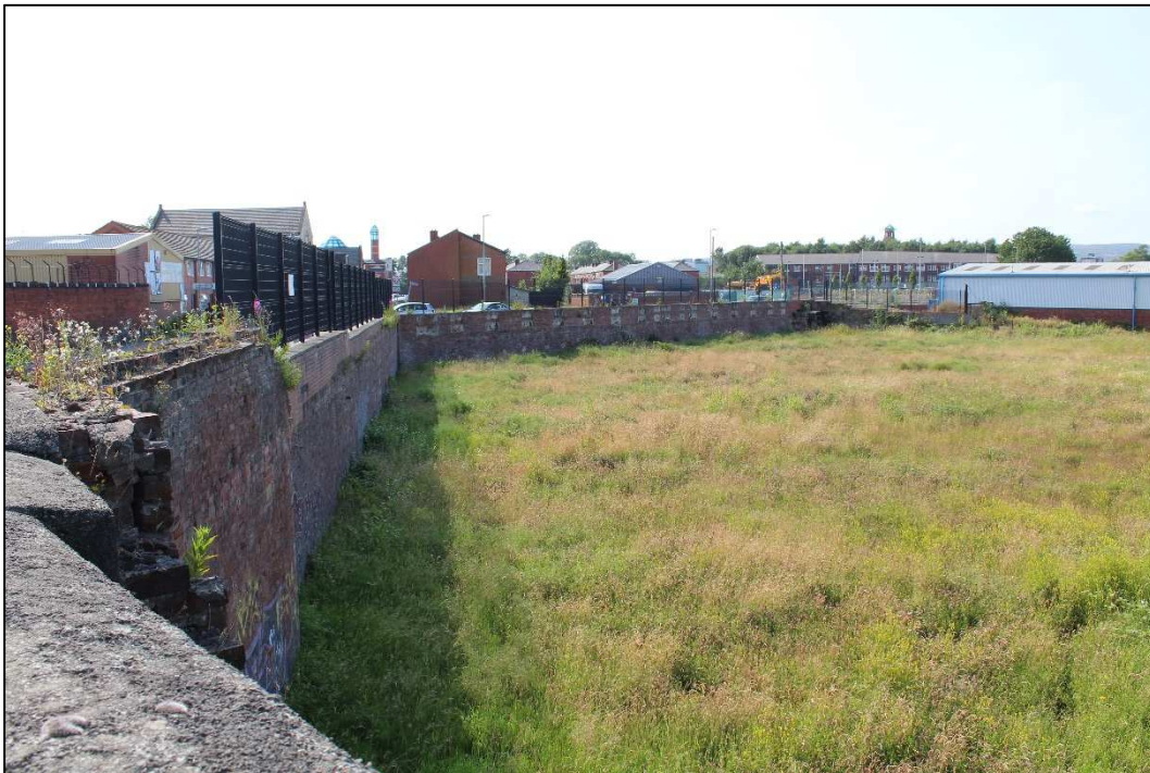
Plate 25: South-western and western boundary walls of site, facing west
