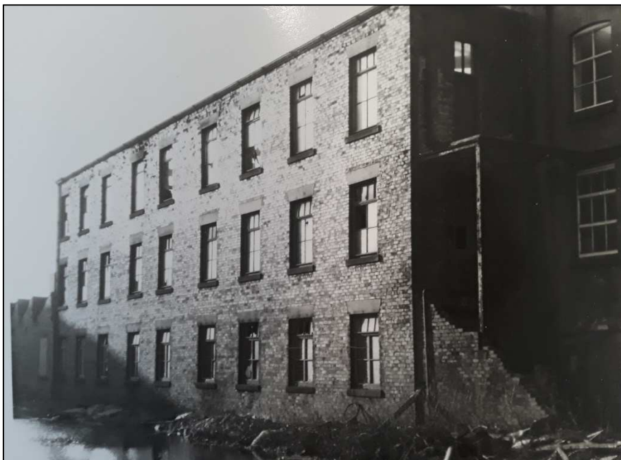
Plate 10: Grove Mill, before demolition Mill exterior, 1975 (RBB 443 190 DIG)
