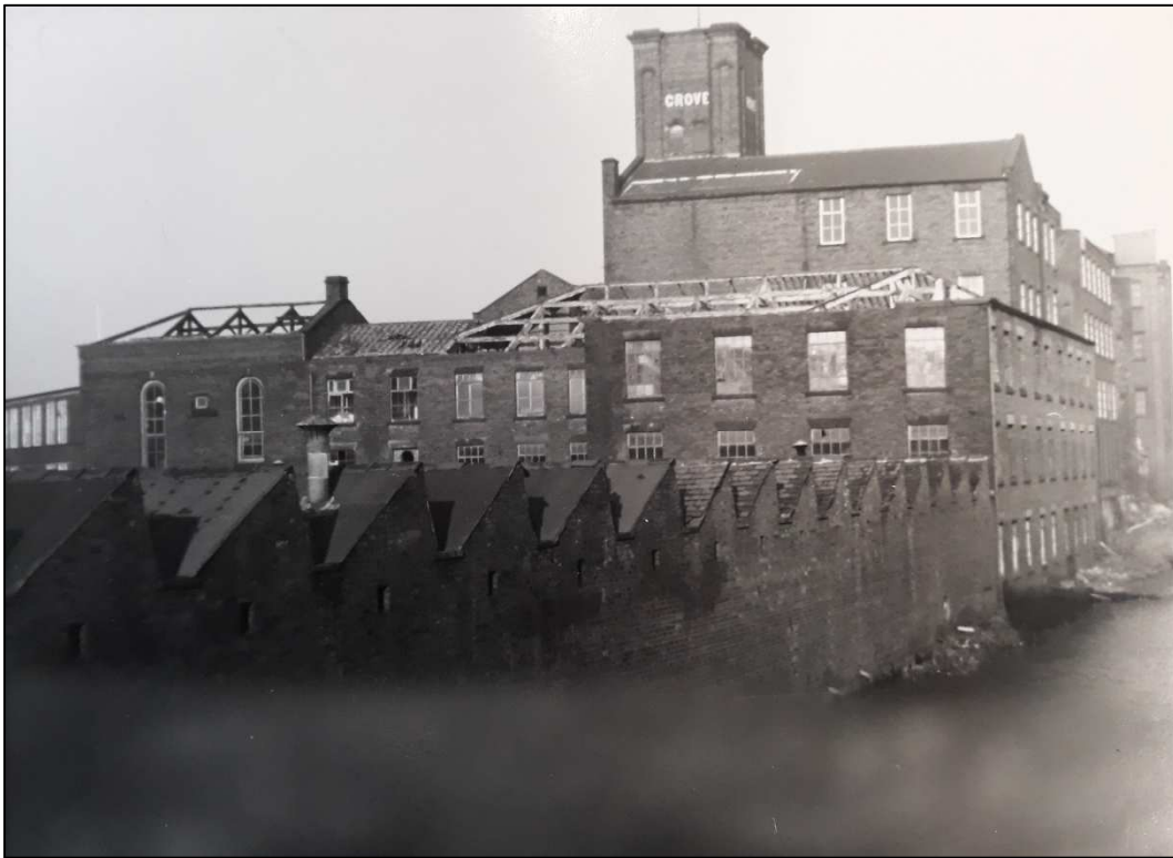
Plate 3: Grove Mill from canal, 1975 (RLSC RB 443 193 DIG)
