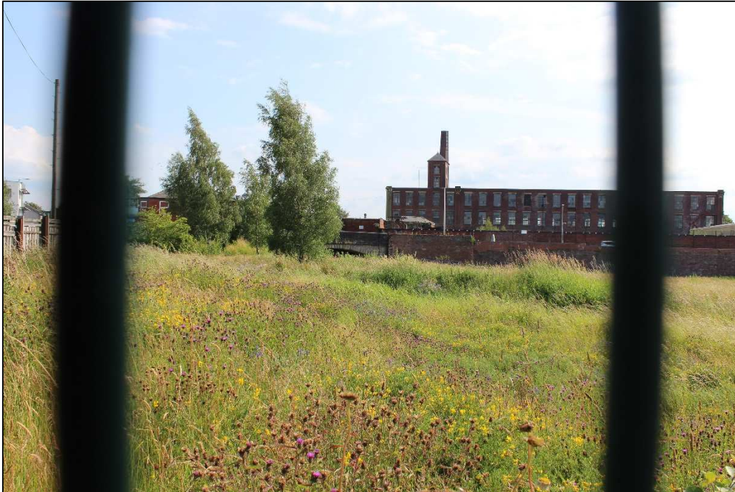
Plate 21: General view of site from the north, facing south-west
