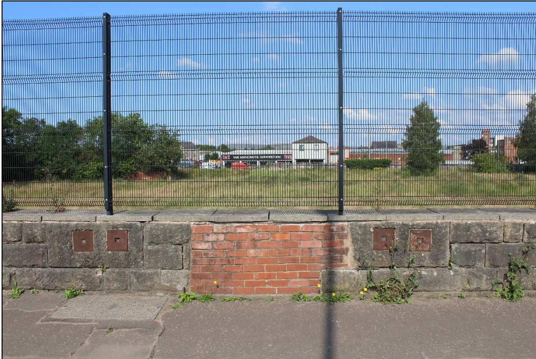
Plate 27: Detail of part of western boundary wall of site, facing east-north-east
