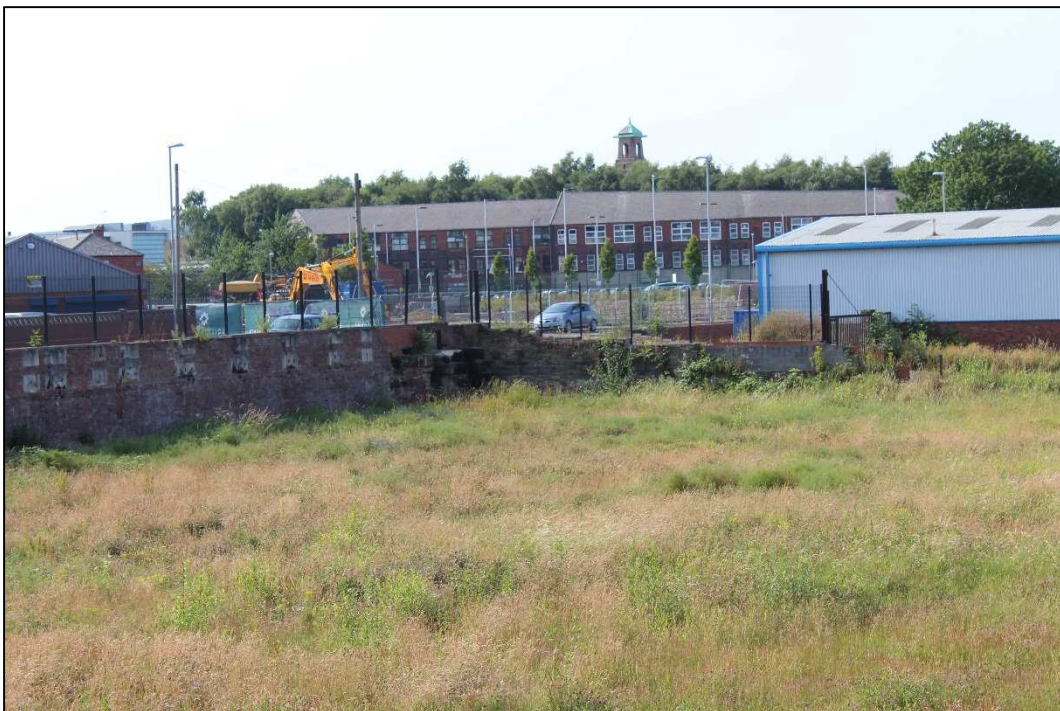
Plate 24: Structural remains within north-western corner of site, facing north-west
