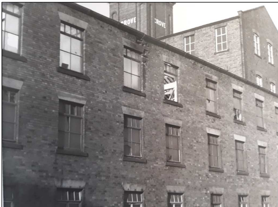
Plate 6: Grove Mill from canal, 1975 (RLSC RB 443 193 DIG)
