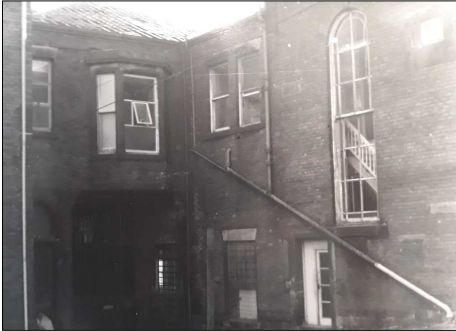
Plate 9: Grove Mill, engine house, 1975 (RLSC RBB 443 192 DIG)
