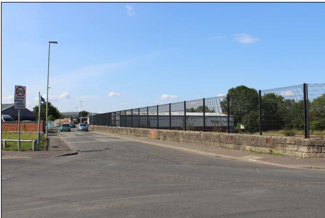
Plate 26: Western boundary wall of site, facing north
