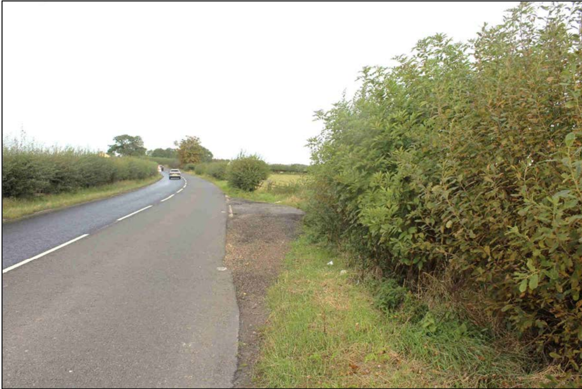
Plate 17: Present layby in vicinity of former garth (Asset 40), facing north-west
