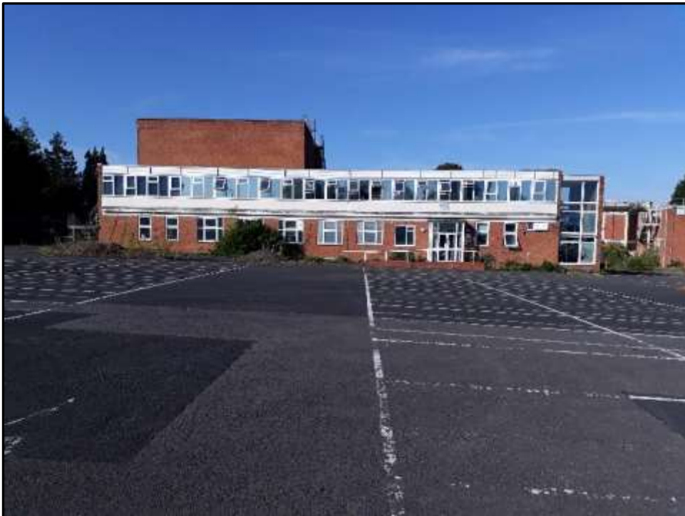
Plate H1 – H Building, South Elevation
