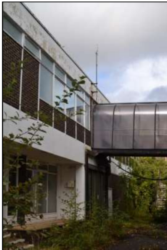
Plate 9b – Building 9, part east elevation
