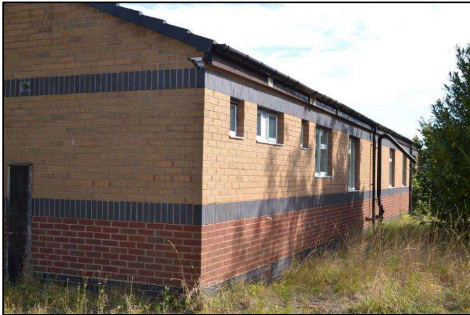
Plate 27d – Building 27, part south west elevation
