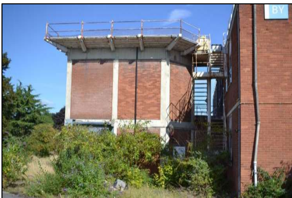
Plate 24j – Building 24, south elevation of former radar satellite platform
