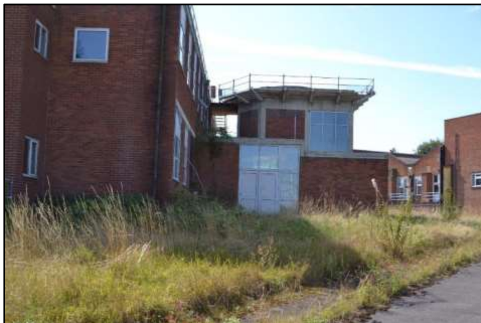
Plate 24a – Building 24, part north elevation showing former radar satellite platform
