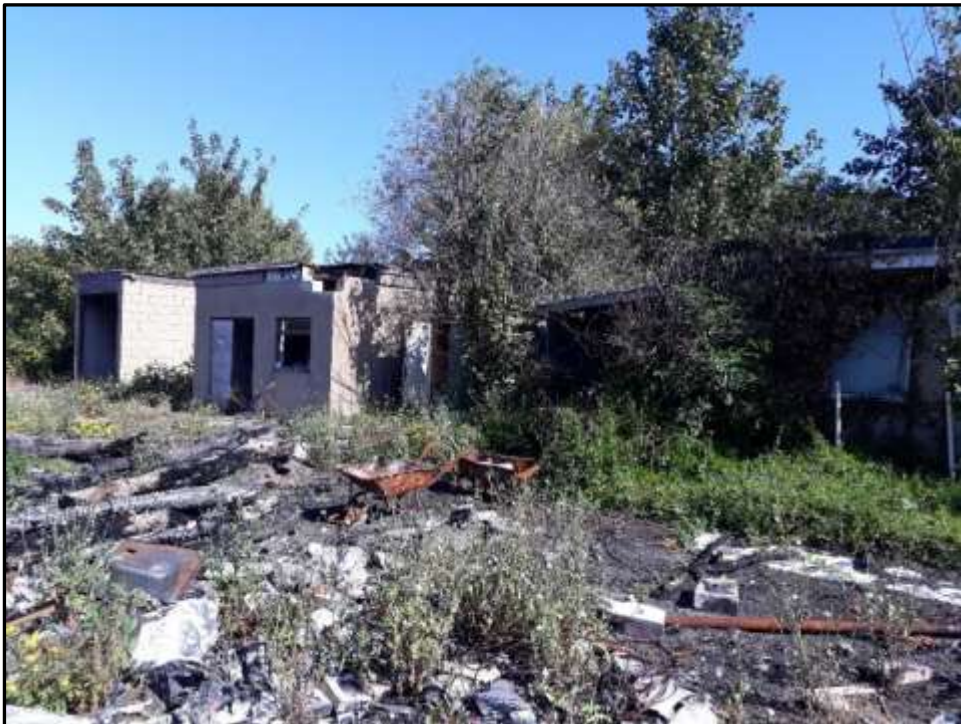
Plate 30b – Building 30, part north west elevation
