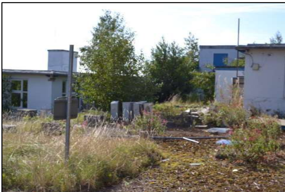
Plate D1 – D Block, part north elevation of spurs 6 and 8
