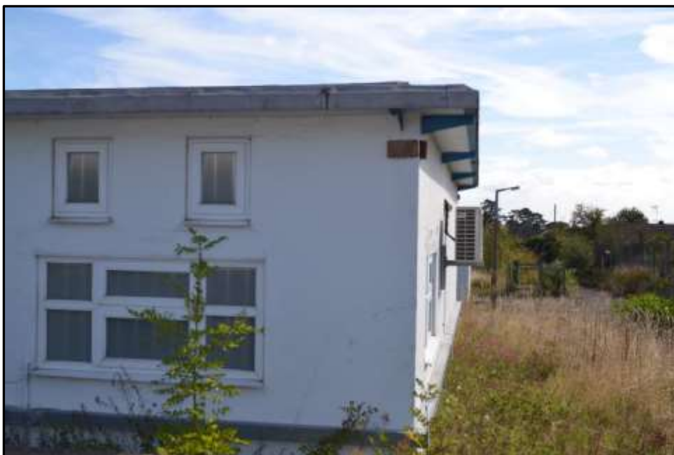
Plate D27 – D Block, part west elevation of spur 5 with altered window openings
