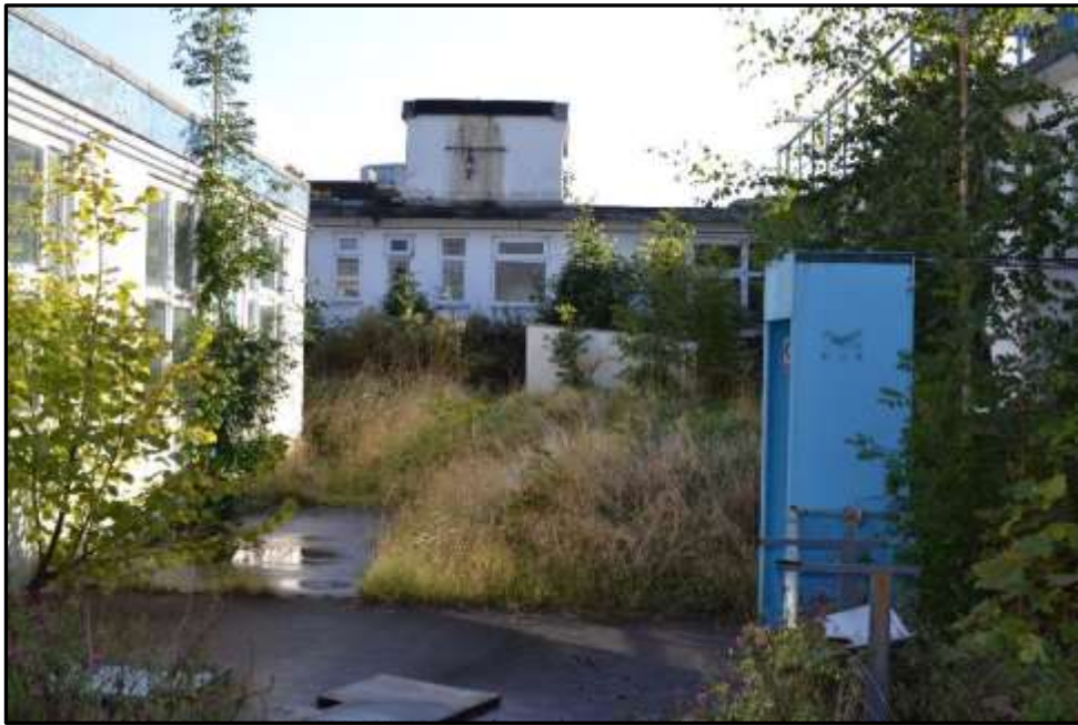
Plate E23 – E Block, north elevation of central corridor range between spurs 6 and 8
