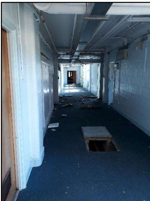
Plate A30 – A Block, interior of central corridor range from the south east
