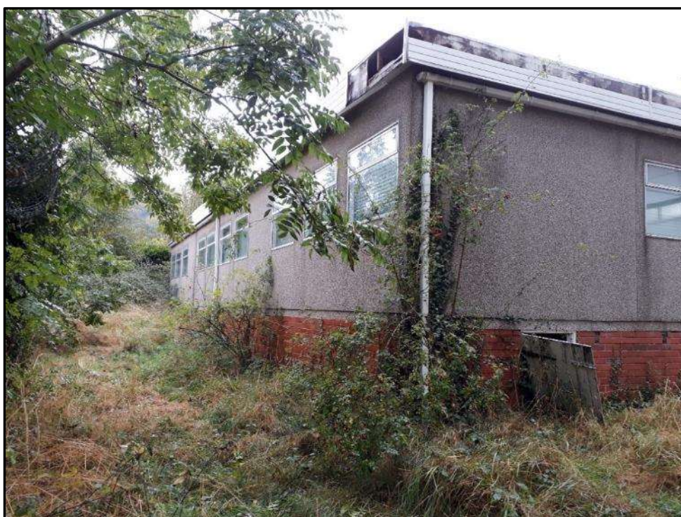
Plate 4a – Building 4, south elevation
