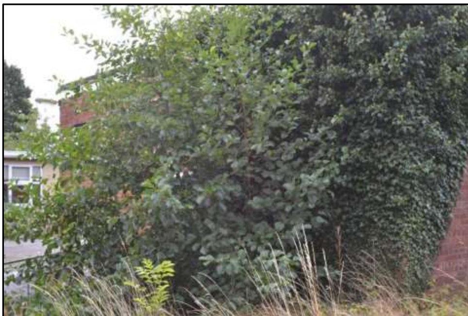
Plate 36h – Building 36, north east elevation of single storey range
