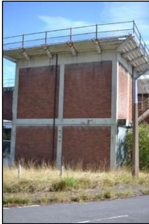
Plate 24k – Building 24, west elevation of former radar satellite platform
