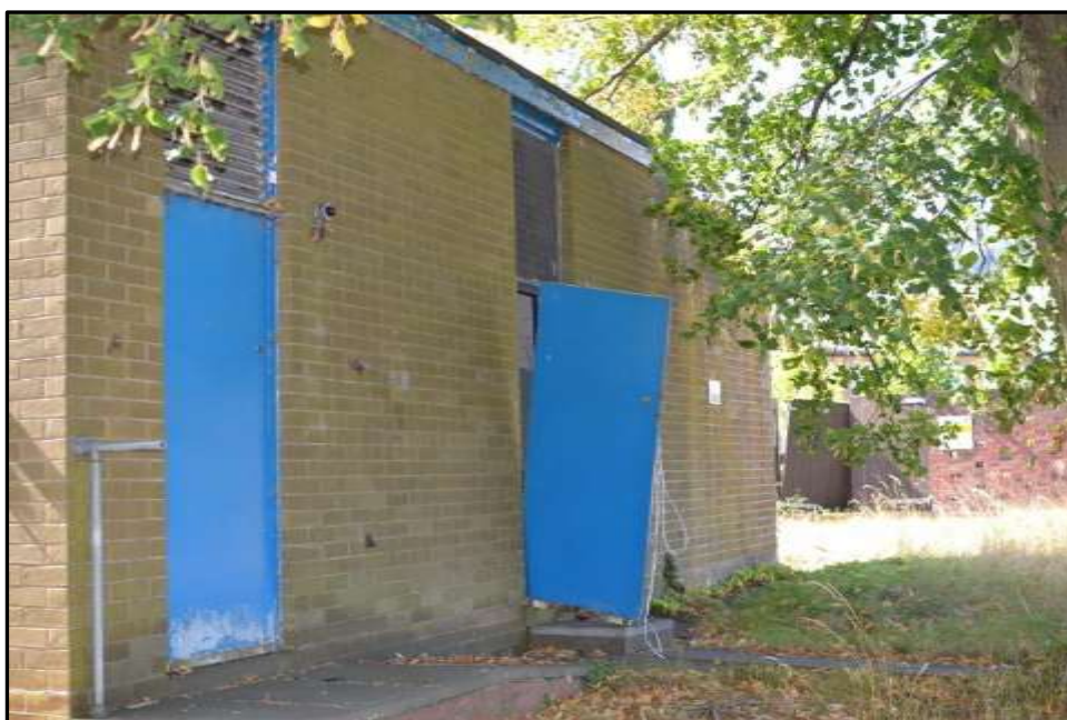
Plate 23c – Building 23, south elevation (viewed from the west)
