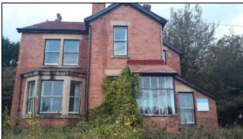
Plate T4 – T Block, east elevation of main range with canted bay window to the left at ground floor and later glazed porch addition to the right
