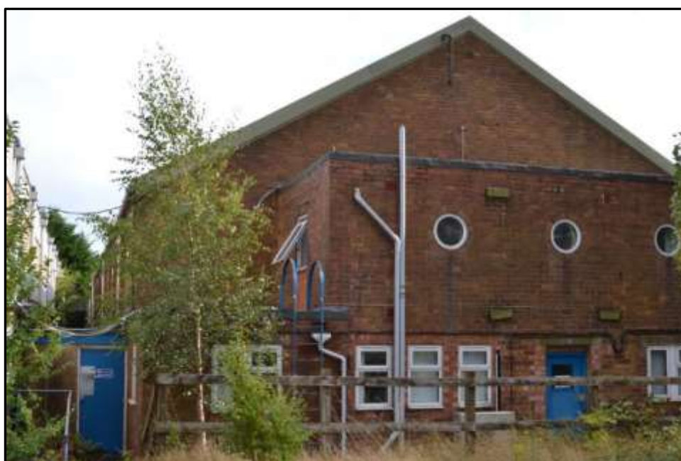
Plate 8k – Building 8, west elevation of the south range
