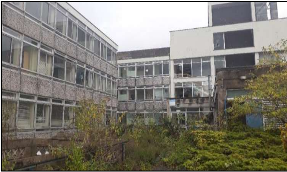
Plate 37f – Building 37, part south and east elevations
