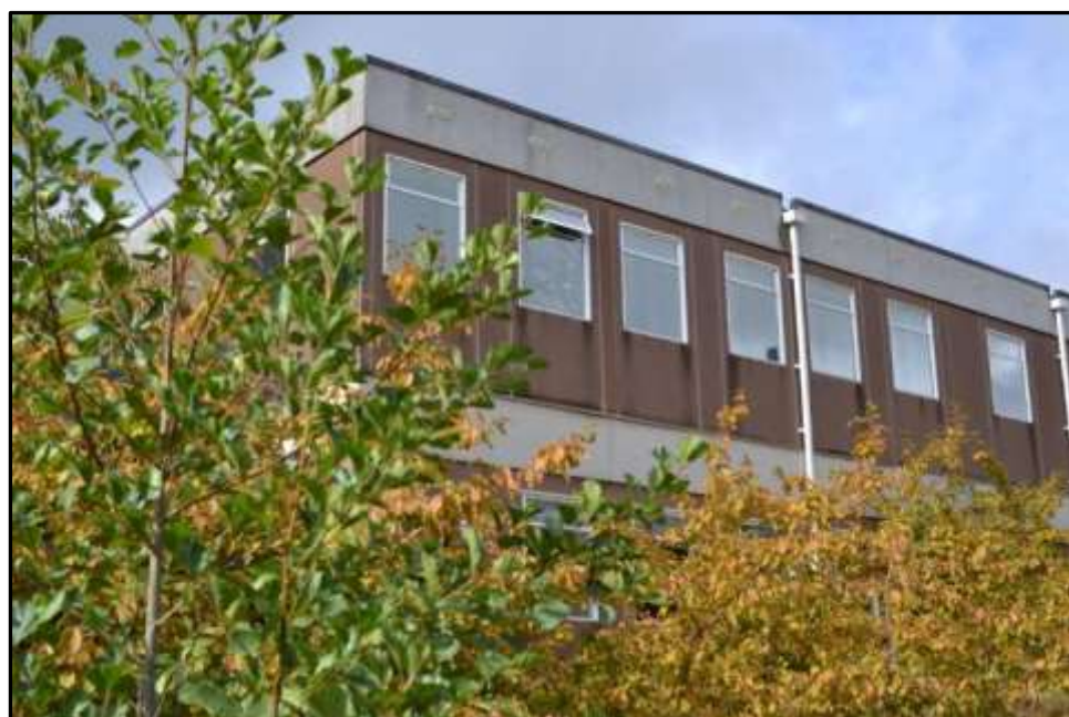
Plate 10b – Building 10, part south and east elevations
