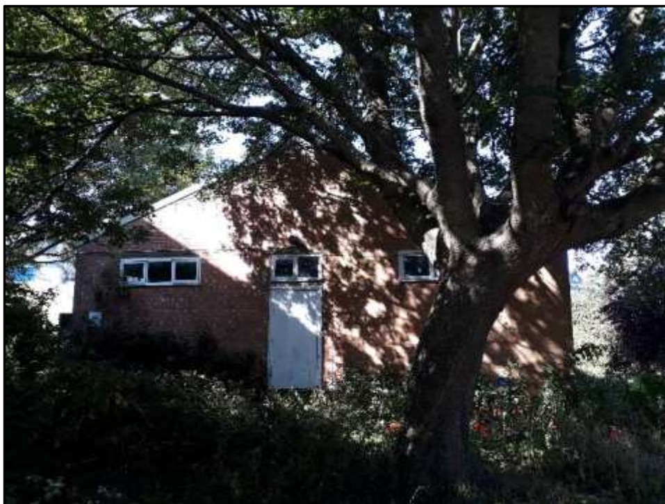
Plate L11 – Library building, south east end elevation of the later south west range
