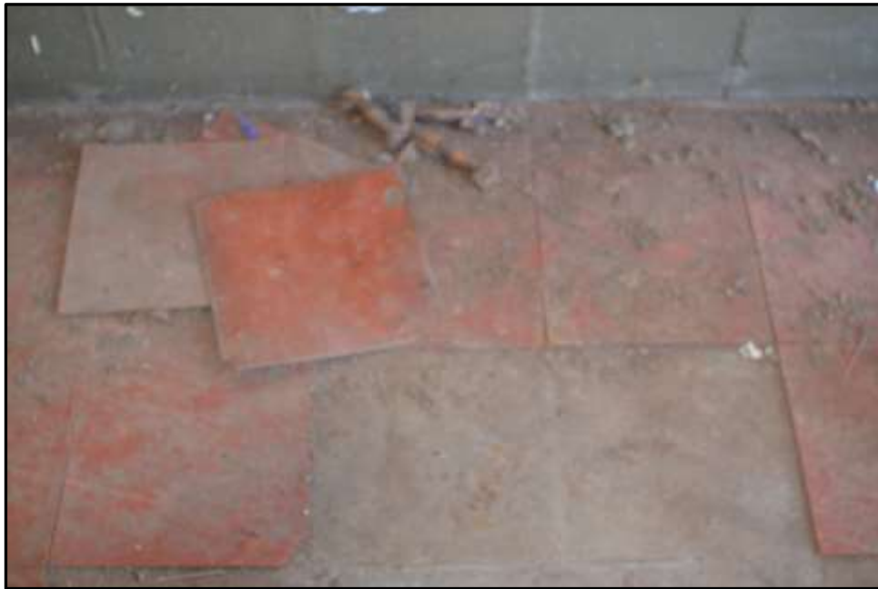
Plate KF13 – Possible original lino tile floor covering observed within the most northern tip of the central corridor
