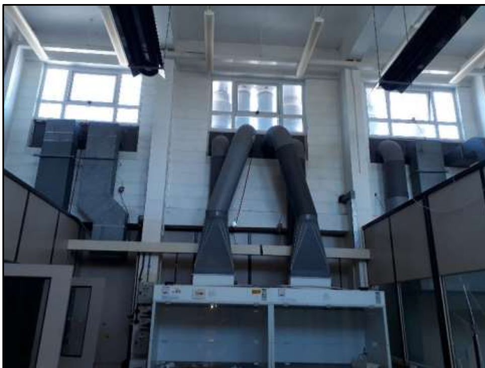
Plate A44 – A Block, infill extension between spurs 2 and 4 originally used for climatic testing of complete systems. Remaining features indicate research use continued within the extension
