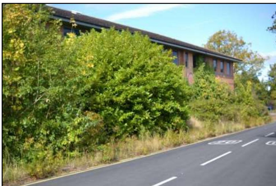
Plate 26c – Building 26, part east elevation
