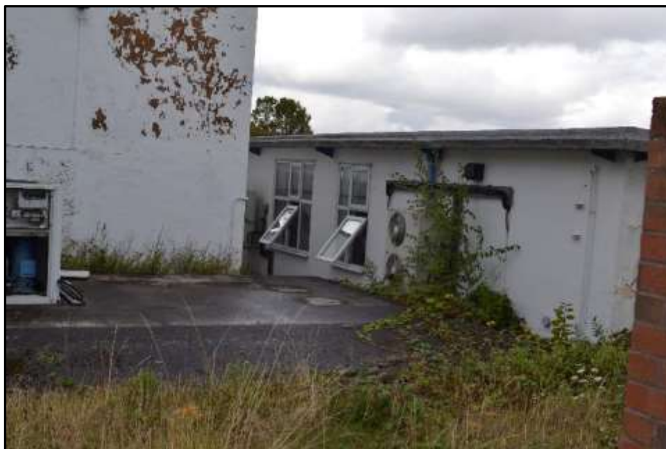
Plate E3– E Block, west elevation of spur 3
