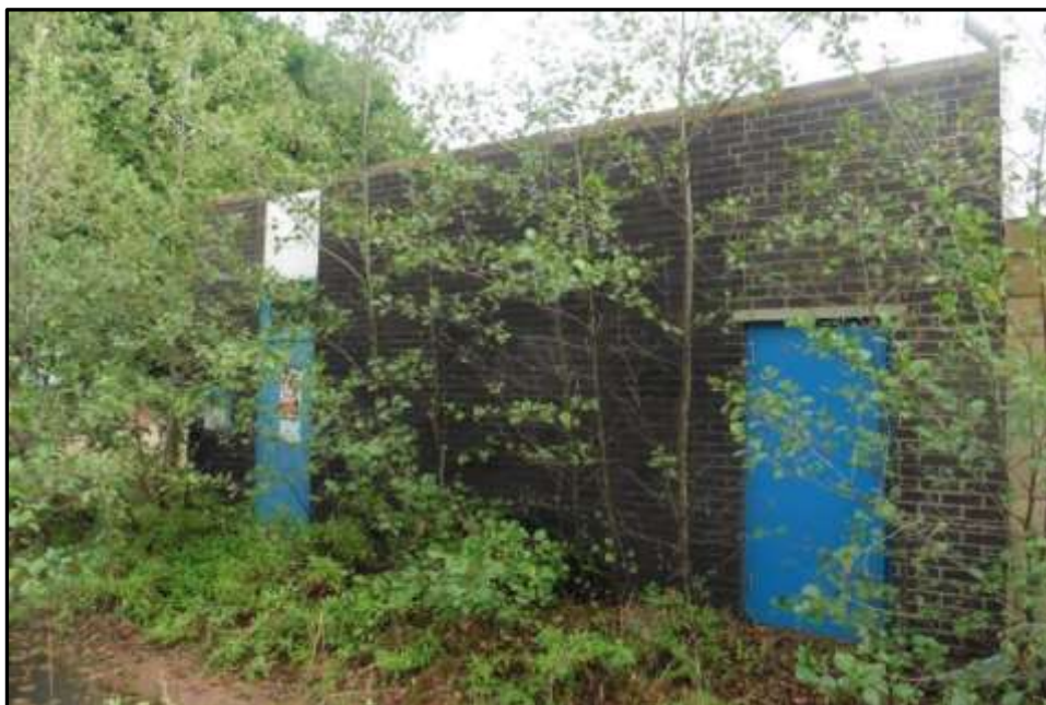
Plate 18c – Building 18, west elevation
