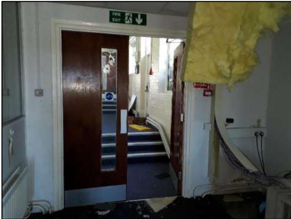
Plate L21 – Library building, doors leading into the link corridor connecting original range to the later south west range
