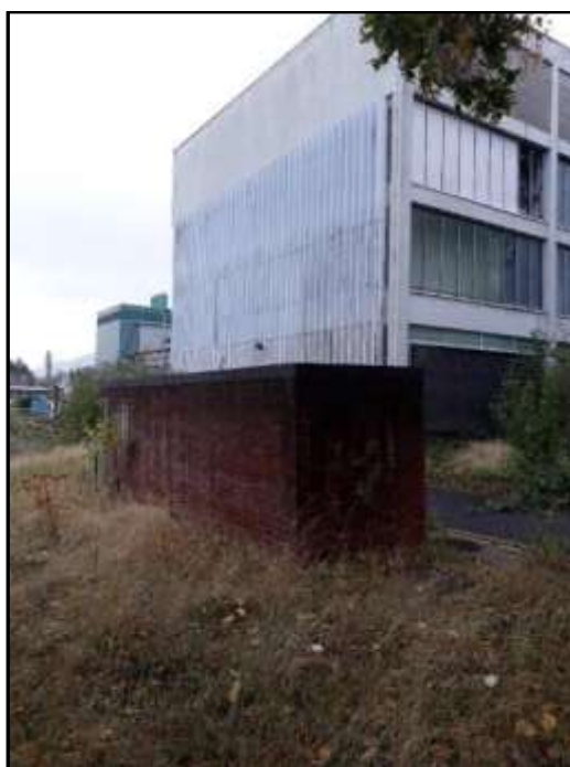
Plate 37e– Building 37, Part east elevation concrete fins
