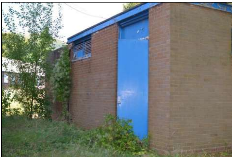
Plate 23b – Building 23, south elevation
