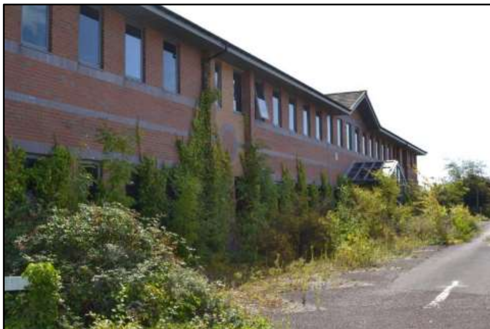
Plate 26a – Building 26, West elevation
