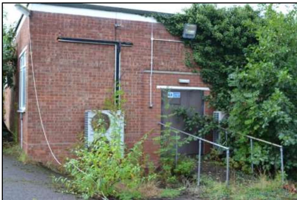
Plate 36i – Building 36, part north east elevation of single storey wing
