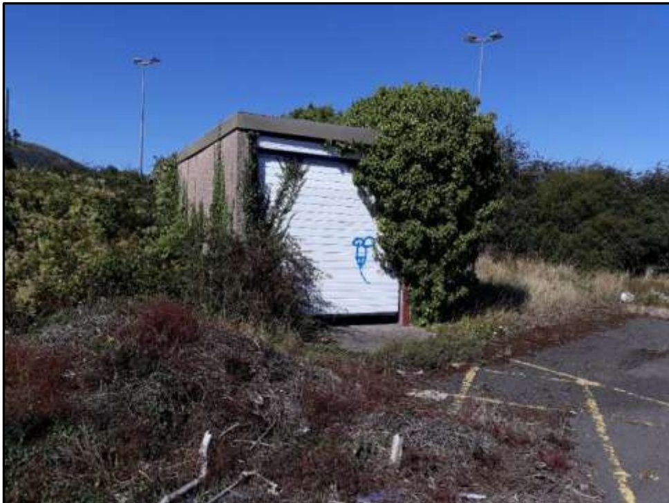
Plate 33a – Building 33, part south east and south west elevation
