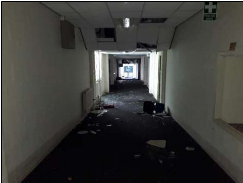
Plate D32 – D Block, central corridor looking east (from between spurs 7 and 8). Note inserted ceiling to conceal ducts and services and rounded edges of brick columns and brick tile internal walls to the right
