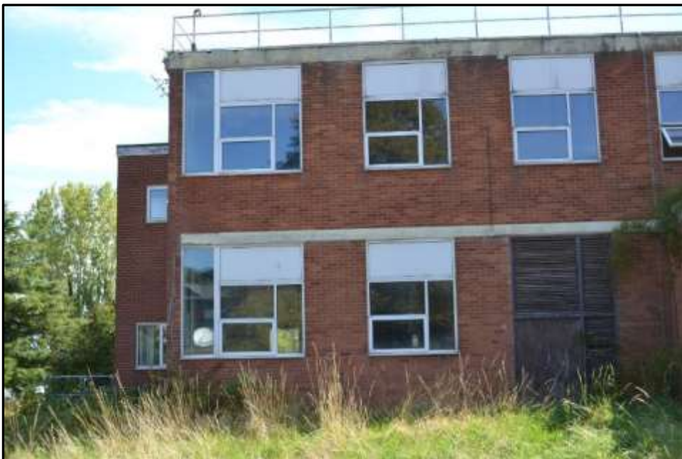
Plate 24n – Building 24, part west elevation of main two storey range
