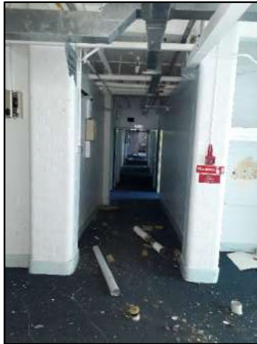
Plate A35 – A Block, secondary corridor to spur 8
