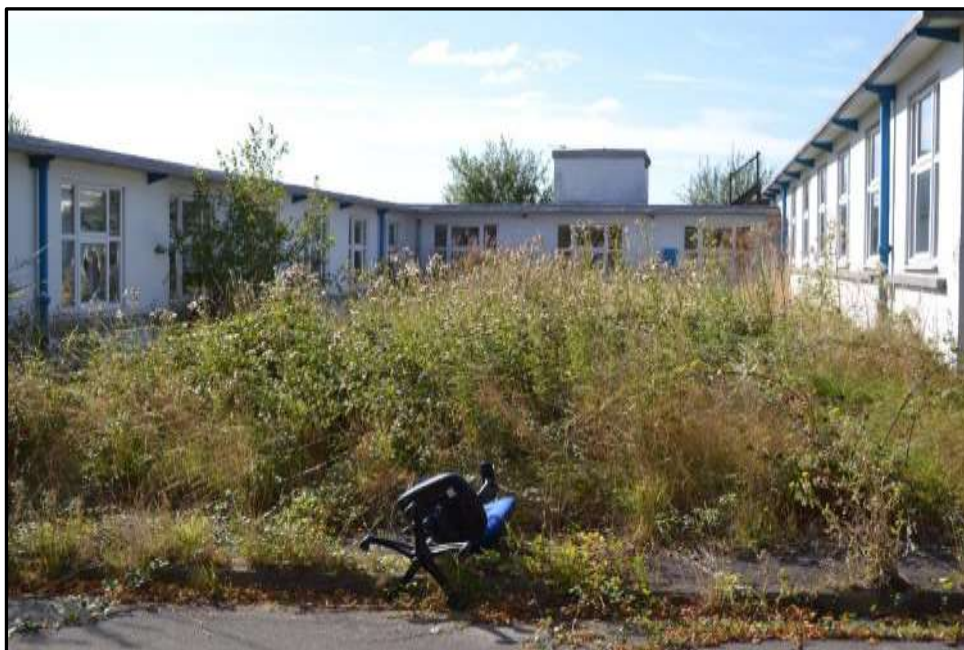
Plate D11 – D Block, typical arrangement of the spurs and central corridor range (spur 4, right, and spur 2, left)
