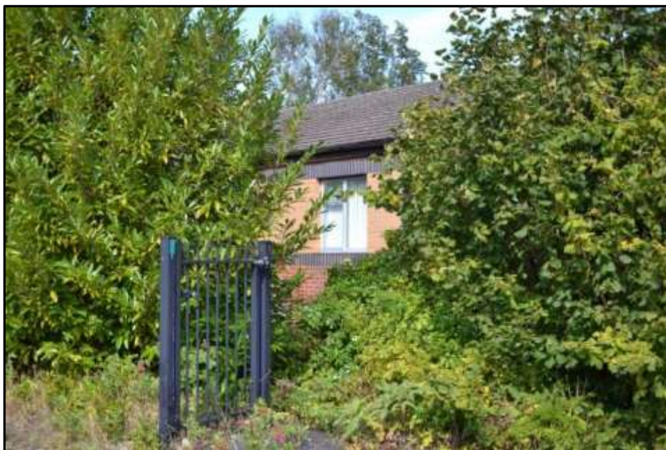
Plate 27b – Building 27, part north east elevation
