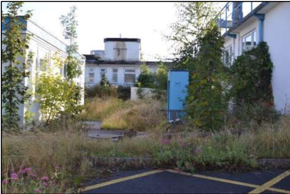
Plate E19 – E Block, view south towards the central corridor range between spurs 6 and 8 with east elevation of spur 6 to right and extension to spur 8 to left
