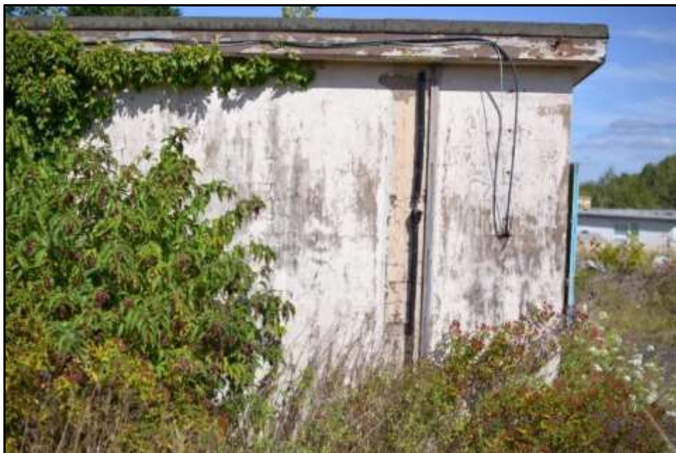
Plate 25d – Building 25, south elevation
