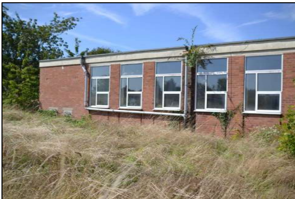
Plate 24e – Building 24, part east elevation (single storey section)
