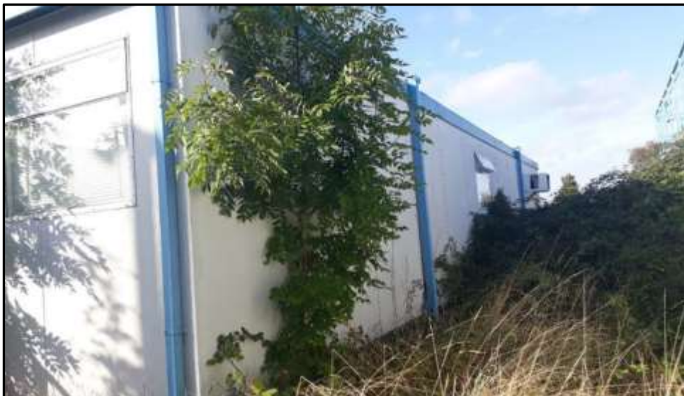
Plate 14b – Building 14, part north and east elevations
