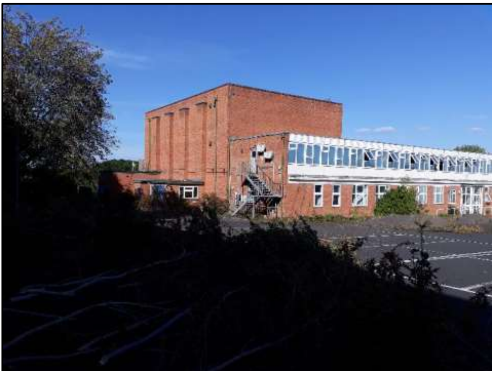
Plate H2 – H Building, part west and south elevations
