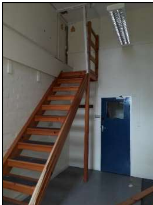
Plate H30 – H Building, ground floor office with north range; stairs previously accessed a storage space within the roof, altered when the first floor was created
