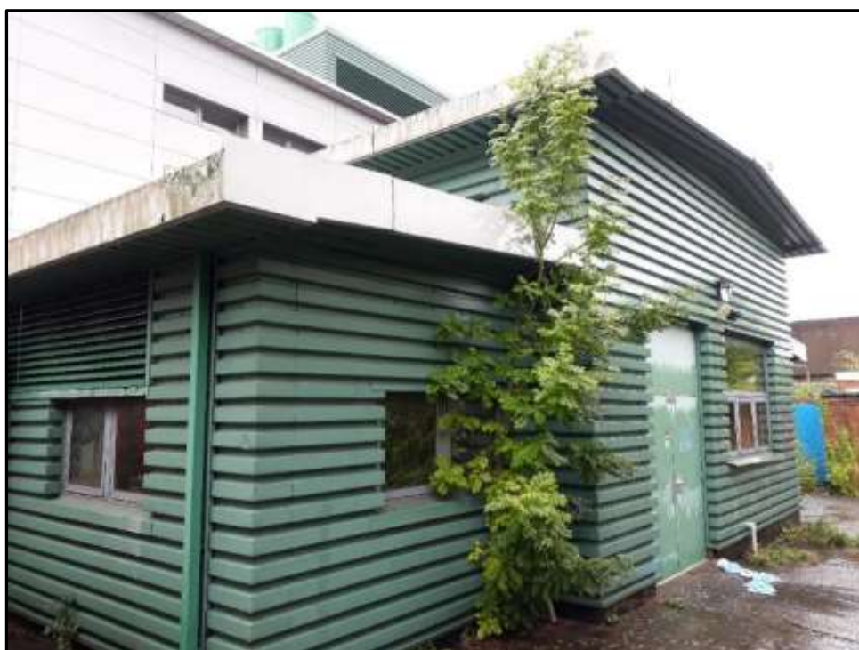
Plate 3d – Building 3, south elevation of south addition
