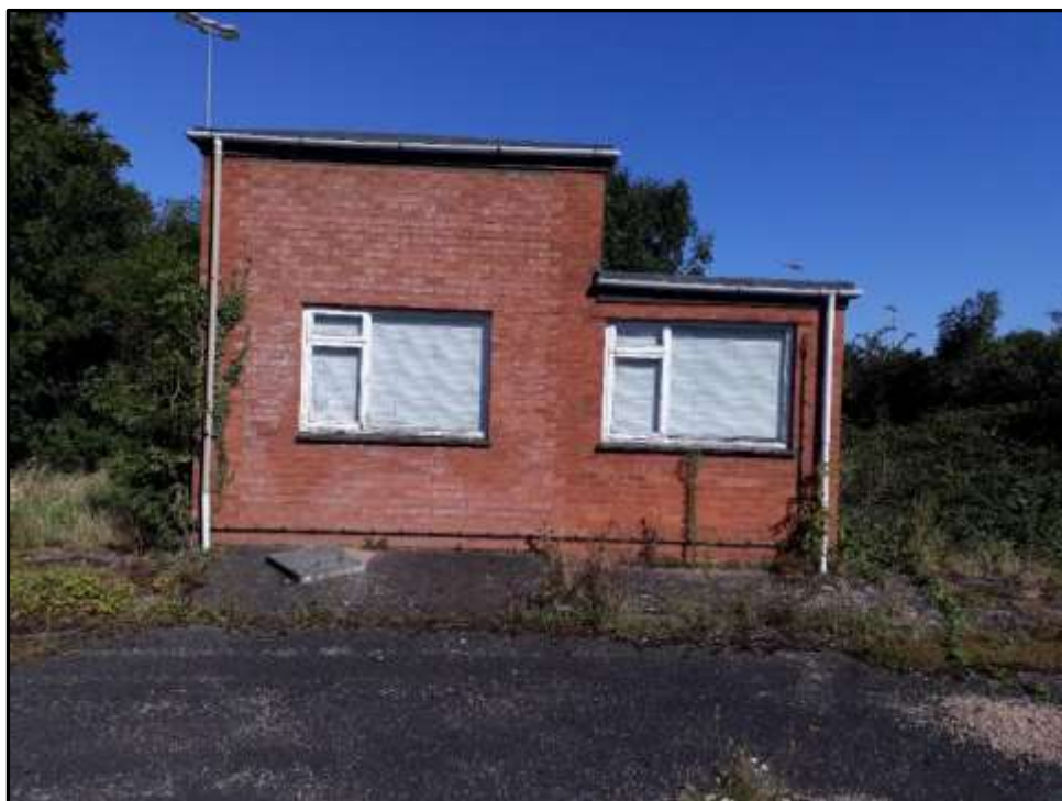
Plate 35b– Building 35, south east elevation
