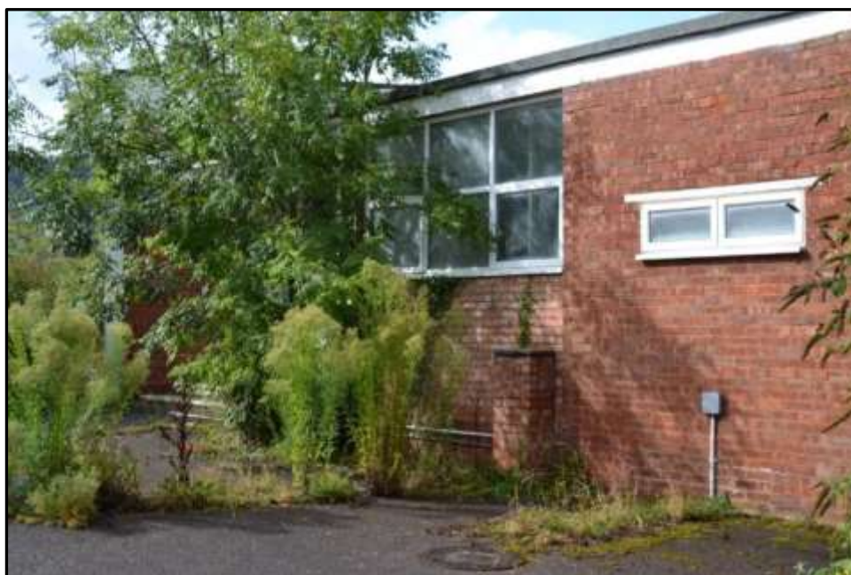
Plate 36k – Building 36, part south east elevation of single storey wing which formerly housed the centrifuge machine
