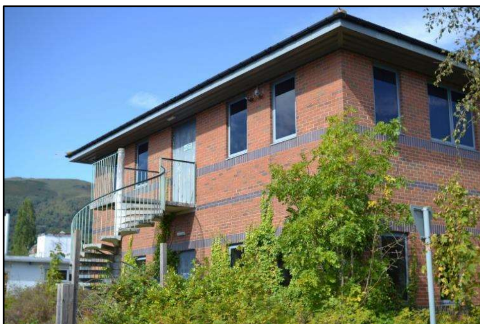
Plate 26d – Building 26, south elevation
