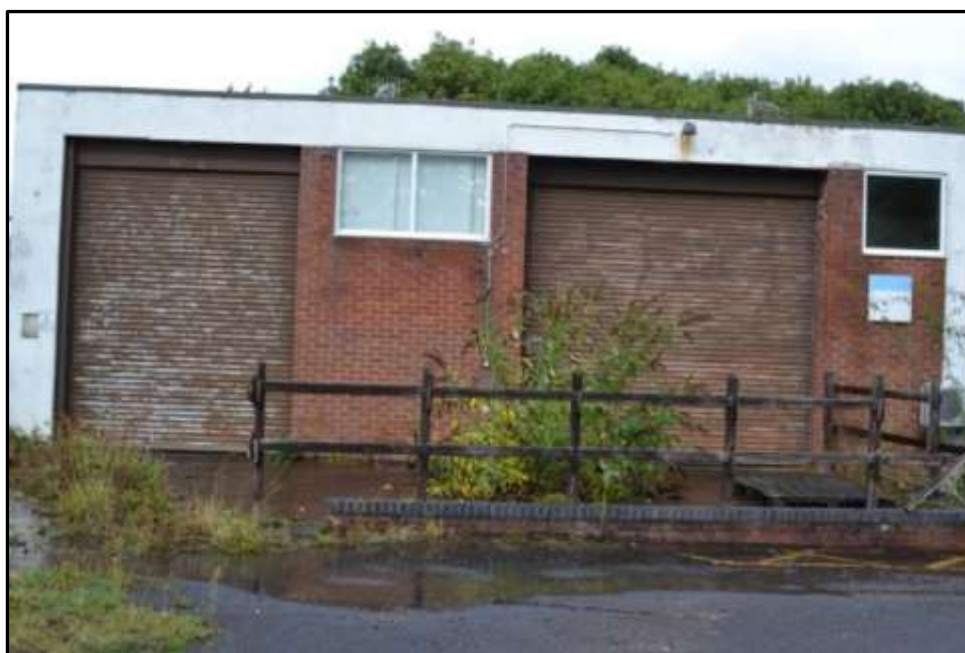
Plate 36a – Building 36, south elevation
