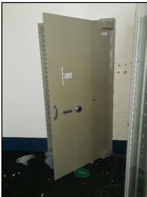
Plate D49 – D Block, safe door to secure document storeroom
