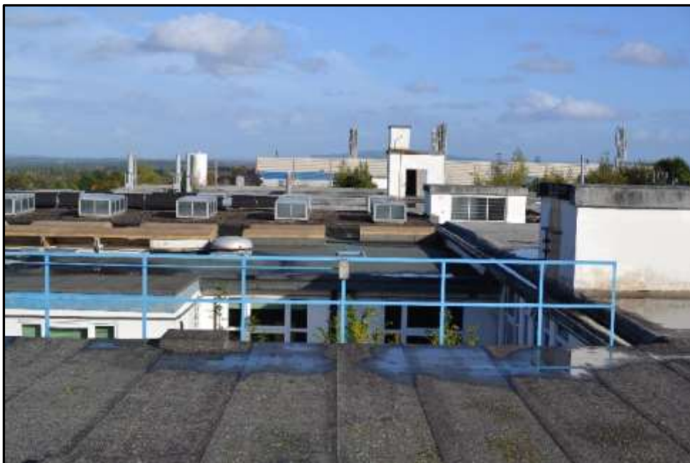
Plate E26 – E Block, view east across roofscape from spur 4
