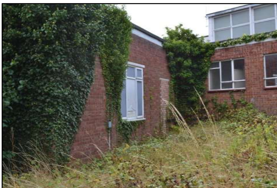
Plate 36g – Building 36, part north elevation of single storey wing
