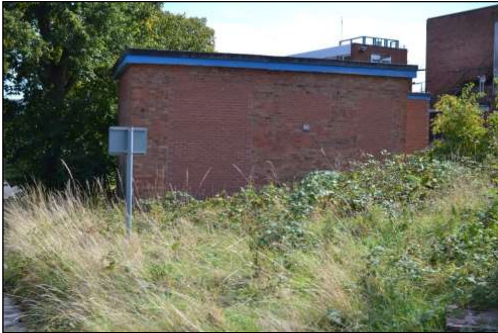
Plate 22b– Building 22, west elevation; note blocked former openings
