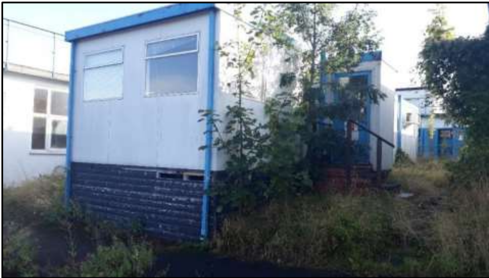
Plate 14a – Building 14, north and part west elevations
