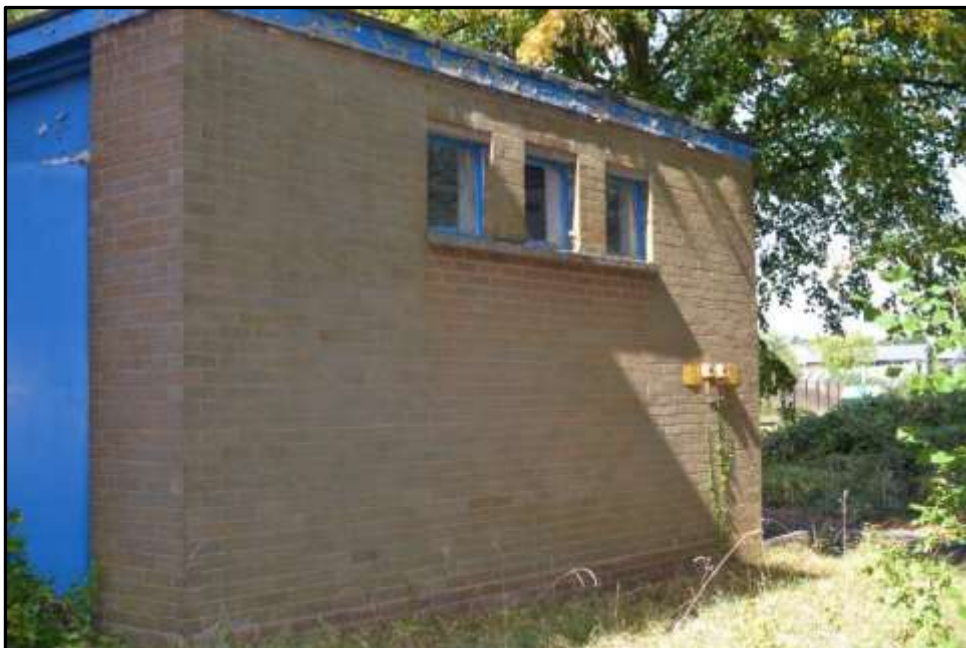
Plate 23a – Building 23, east elevation
