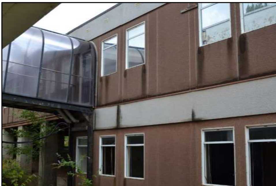
Plate 10c – Building 10, part west elevation with first floor link corridor to building 9
