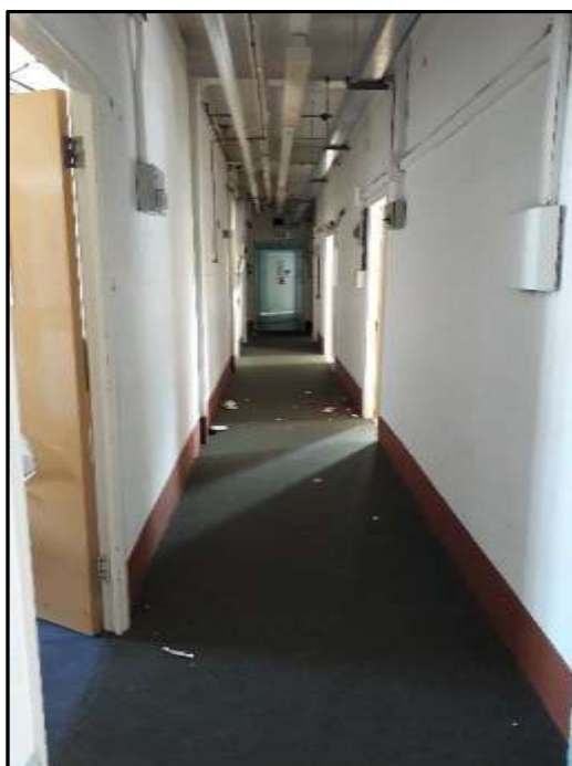
Plate E33 – E Block, view south along secondary corridor into 10
