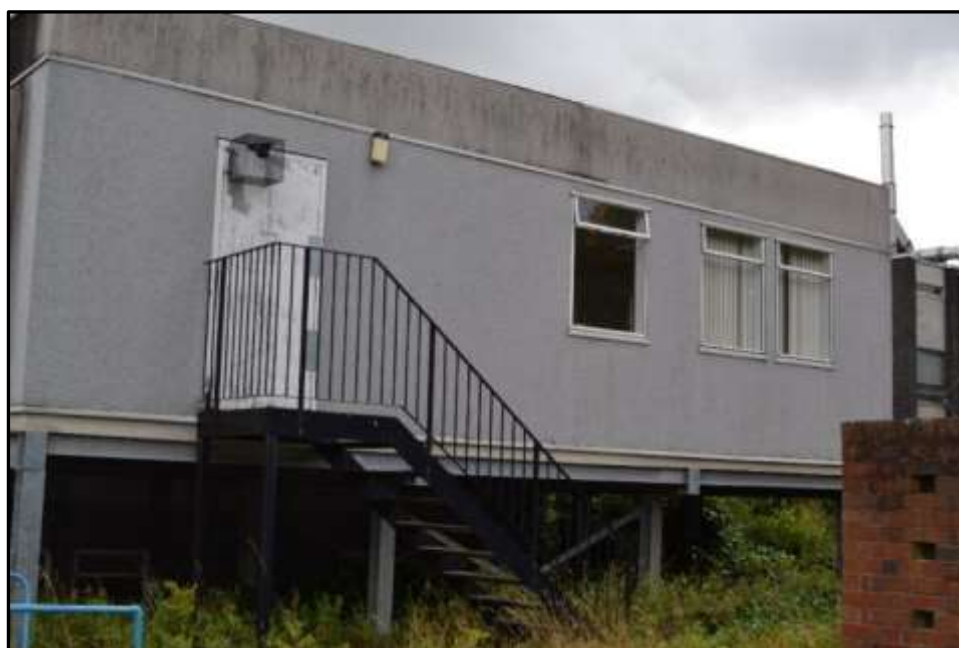
Plate 15c – Building 15, west elevation showing change in external ground level
