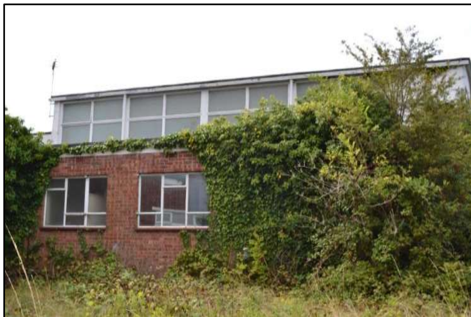
Plate 36f – Building 36, east elevation of stratosphere chamber
