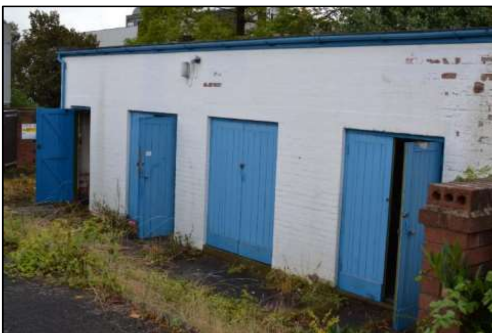
Plate 11a – Building 11, north elevation
