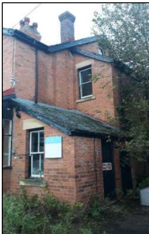
Plate T3 – T Block, part north elevation with later lean-to addition
