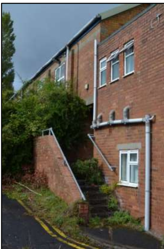
Plate 8f – Building 8, part south elevation of the south range
