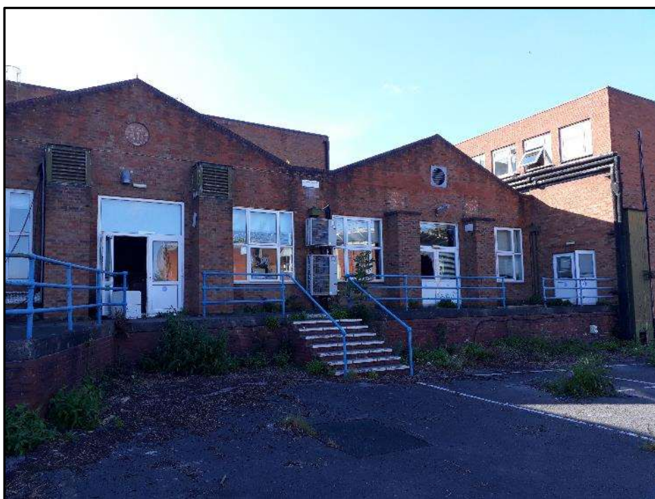
Plate H14 – H Building, part east elevation showing the gabled roof form of the original radar room and track telling room
