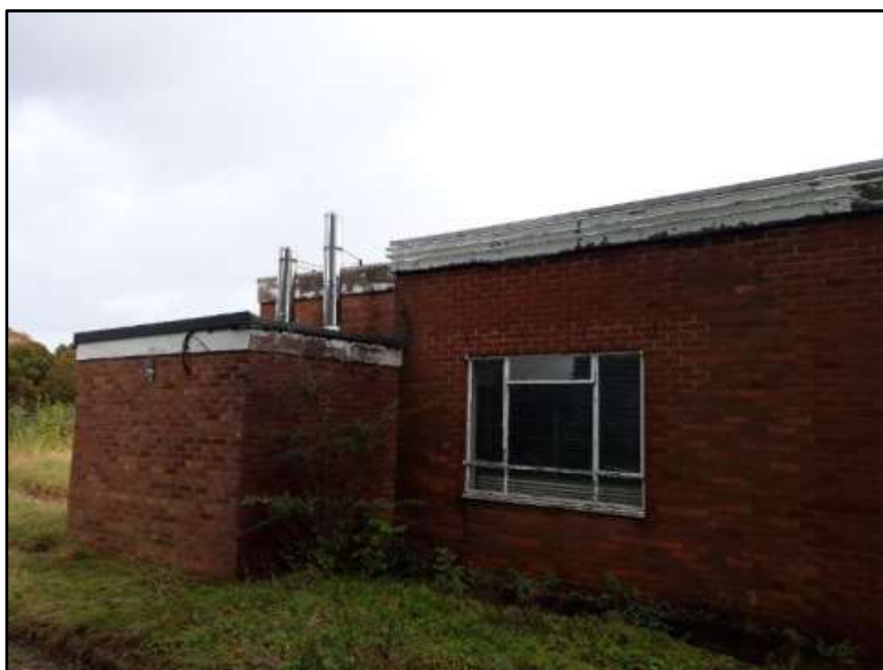
Plate 7d– Building 7, south elevation
