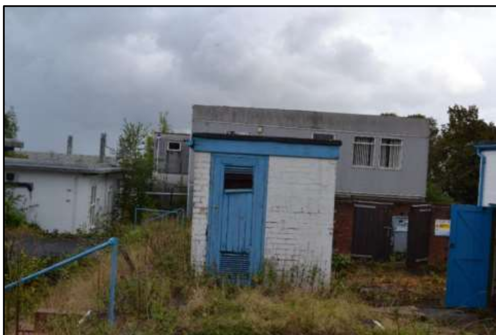
Plate 12b – Building 12, west elevation
