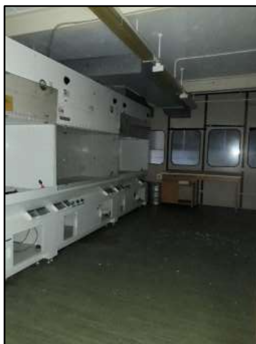
Plate A42 – A Block, modern fixtures associated with laboratory use observed in spur 2
