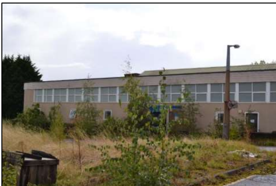
Plate 8o – Building 8, north elevation of the north range
