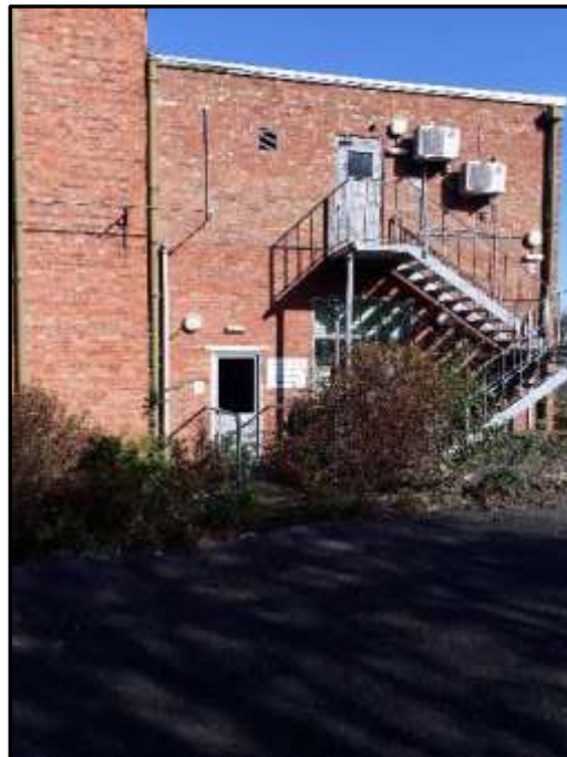
Plate H4 – H Building, altered west elevation of south range
