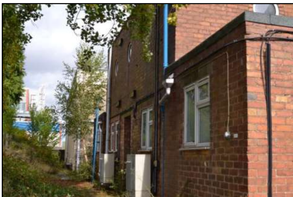
Plate 8j – Building 8, west elevation of the south range
