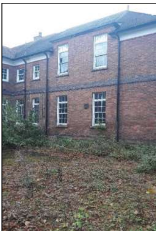
Plate S9 – Block S, north elevation of the south range
