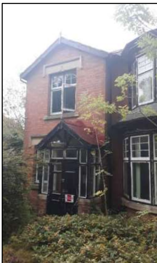
Plate T7 – T Block, west elevation with main entrance positioned off centre within advanced gable; note ogee shaped inscription to the stone lintels
