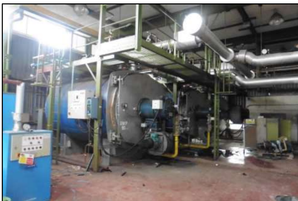
Plate 19d – Building 19, former boilers to the interior
