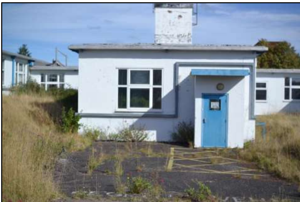
Plate D23 – D Block, south elevation of original boiler house range between spurs 3 and 5
