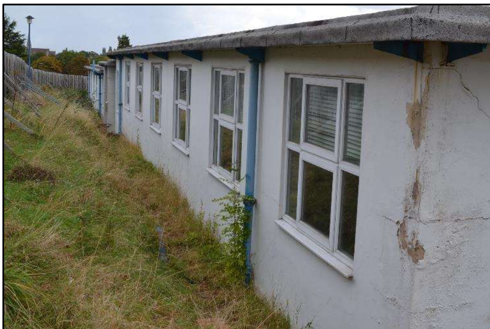
Plate E1 – E Block, west elevation of spurs 1 and 2
