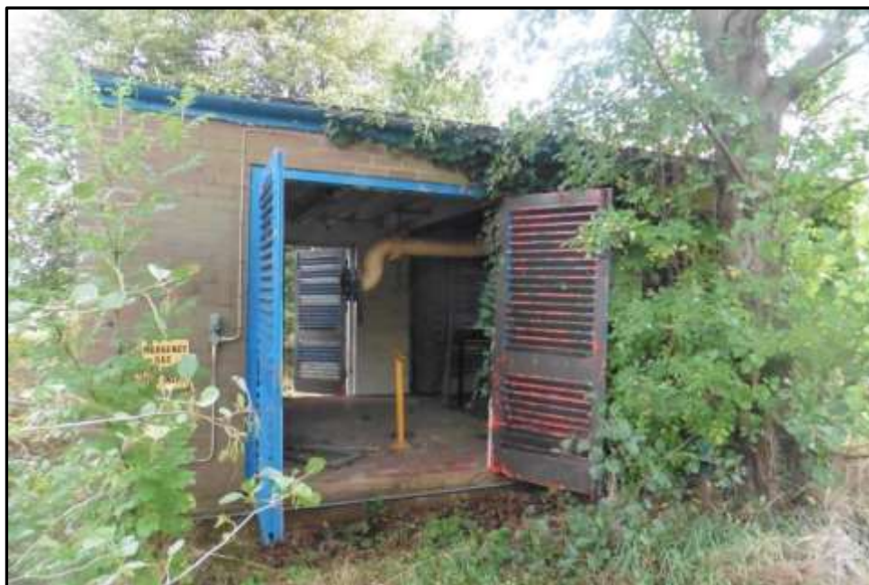
Plate 20c – Building 20, part west elevation
