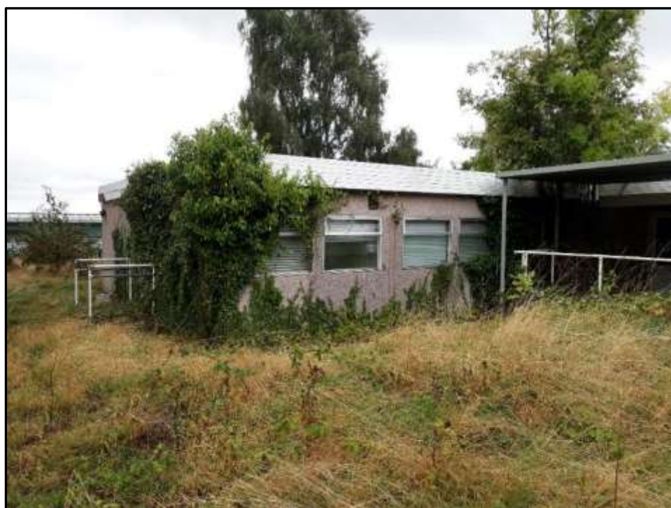
Plate 4c – Building 4, part north and west elevations
