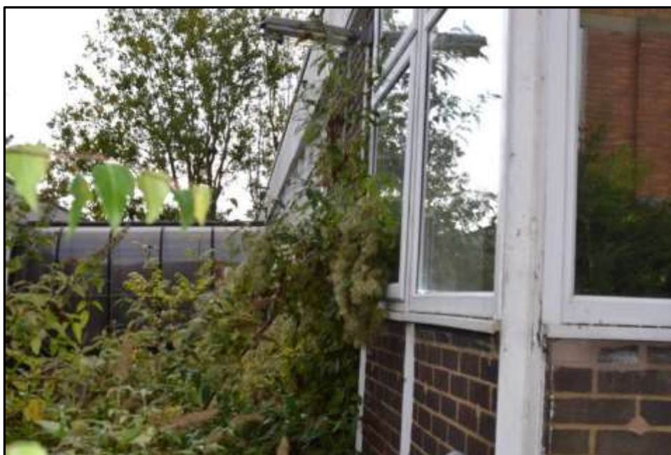
Plate 9j – Building 9, first floor link extension viewed from the north
