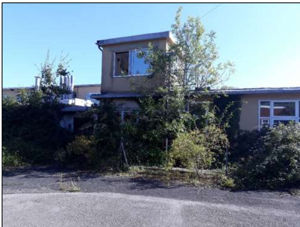
Plate A19 – A Block, north west elevation of spur 1 with secondary west entrance and small first floor addition
