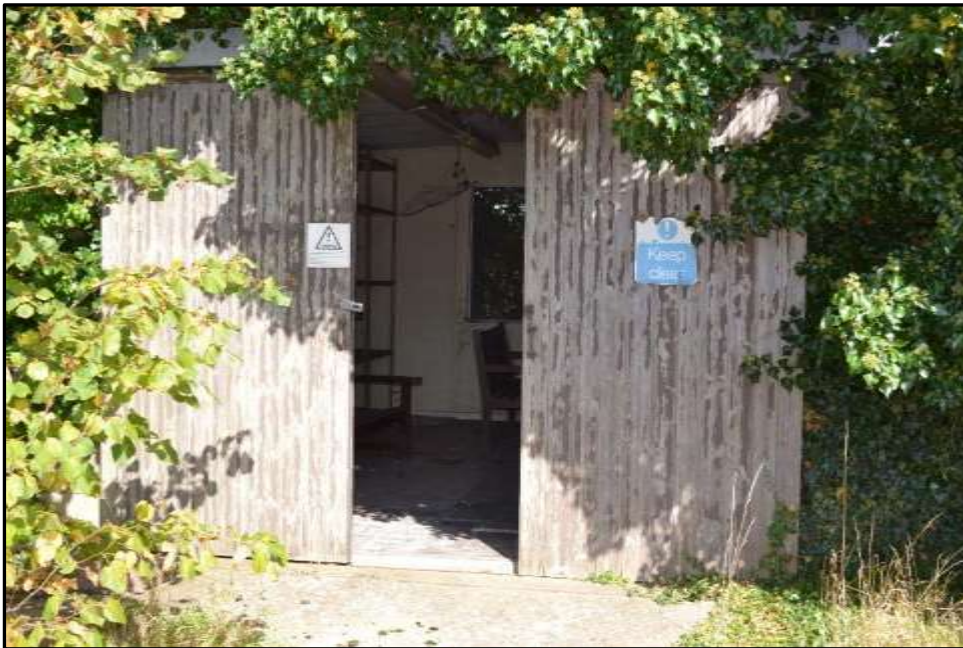
Plate 29a – Building 29, entrance doors to the south west elevation
