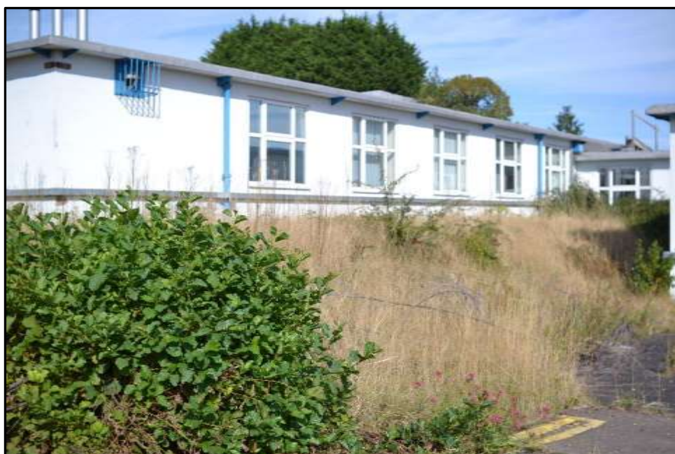
Plate D24 – D Block, east elevation of spur 5
