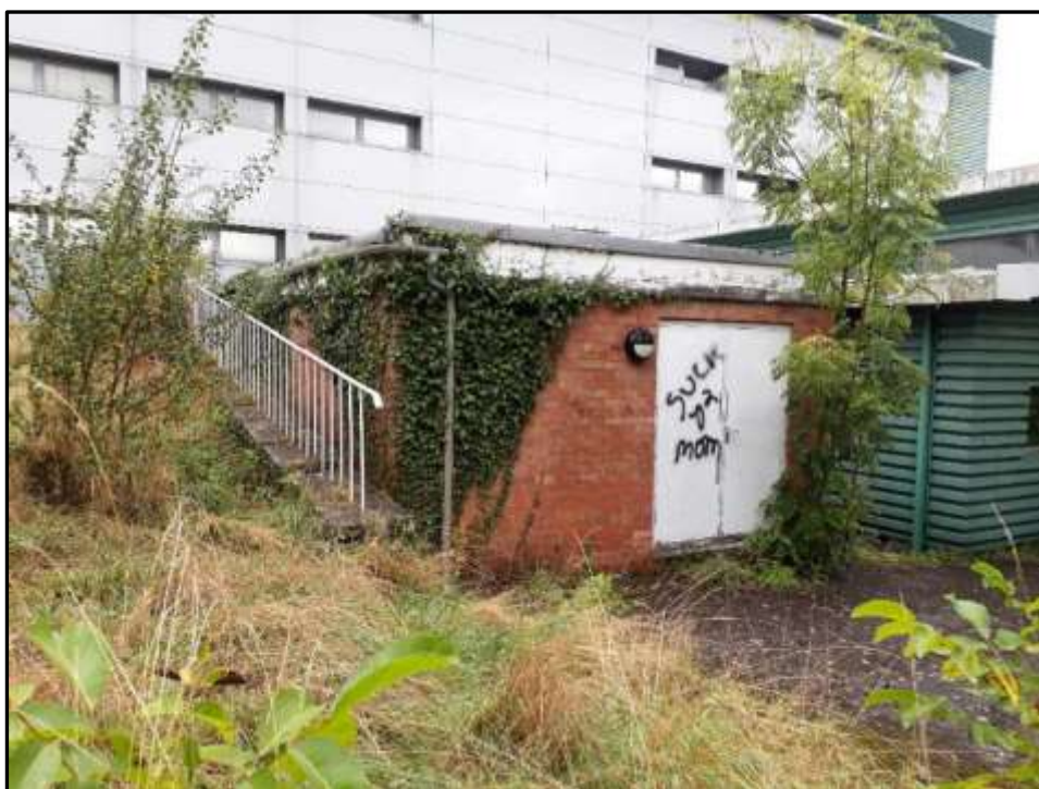
Plate 5a – Building 5, part west and south elevations
