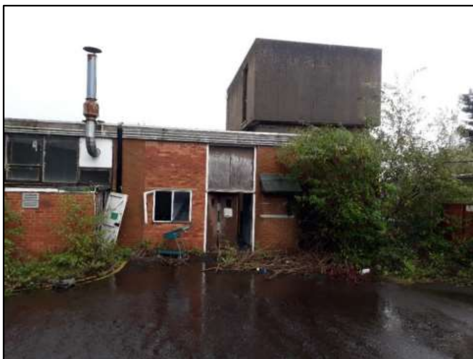
Plate 7e – Building 7, part west elevation
