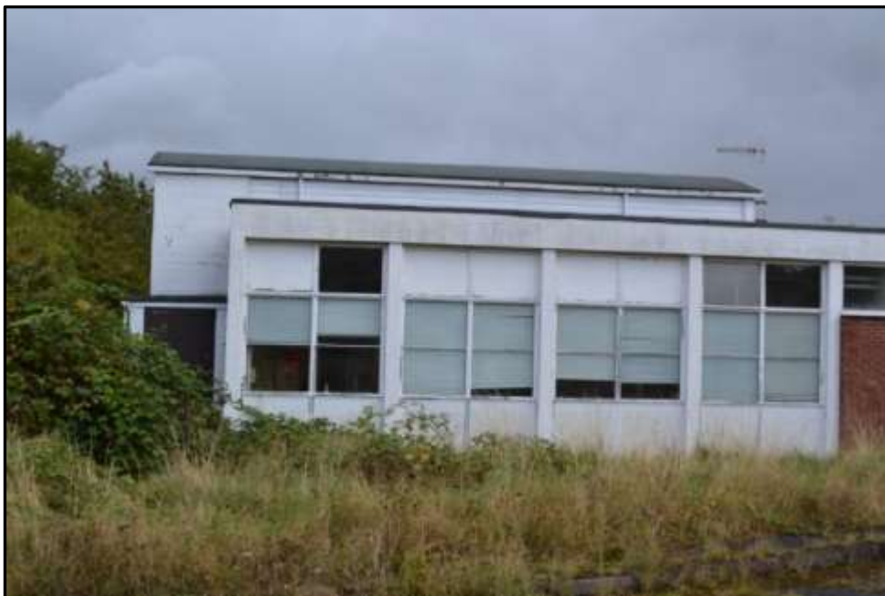
Plate 36c – Building 36, east elevation, note taller element which housed the stratosphere chamber
