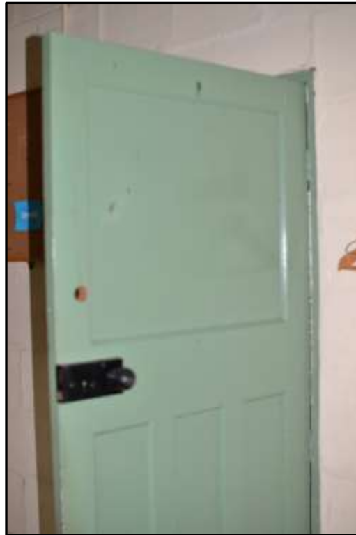
Plate KF17 – Early/original door within southern half of block
