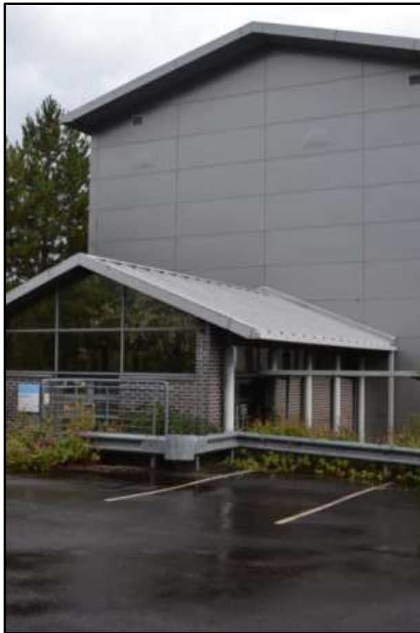
Plate 3f – Building 3, later porch addition to west elevation of main range
