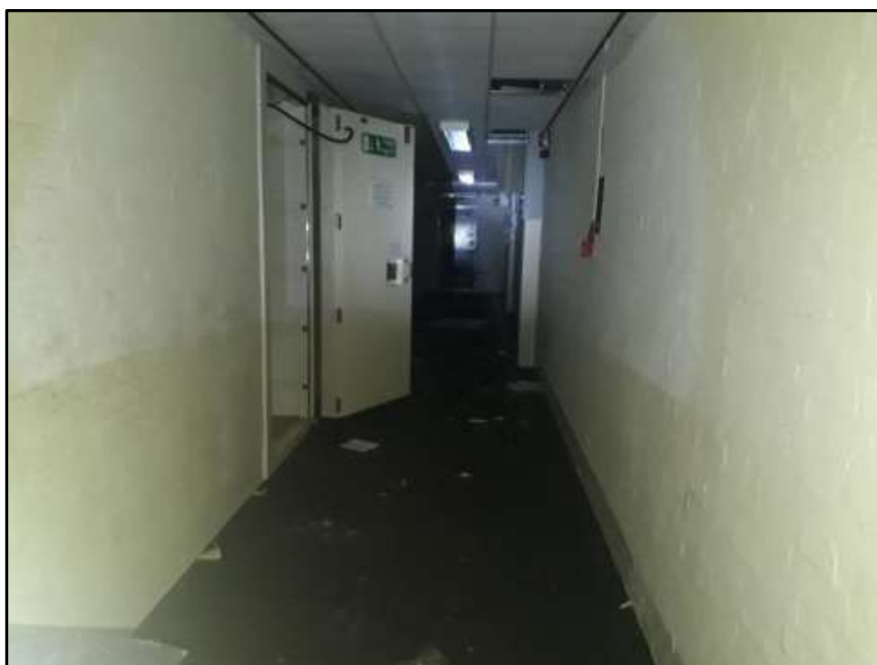
Plate H40 – H Building, ground floor corridor linking north and south ranges; former bunker and main entrance to right. Internal walls display painted brickwork finish
