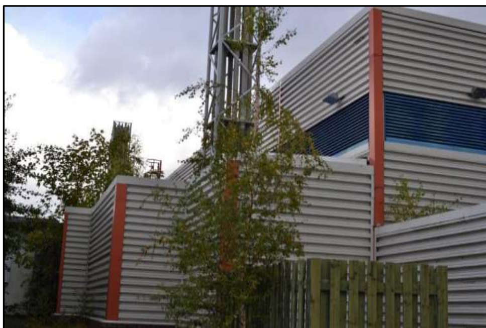
Plate 17g – Building 17, part west elevation of main range and stepped south elevation of additions
