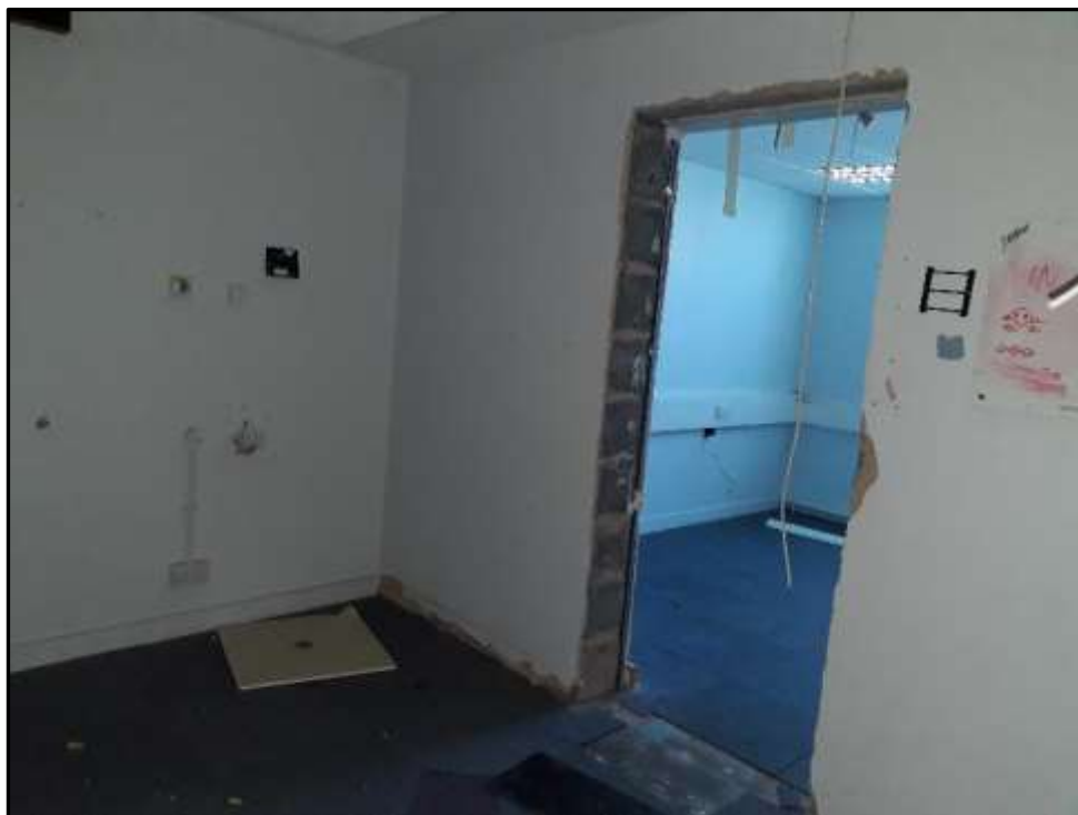
Plate A36 – A Block, evidence of new work and new opening observed in spur 5
