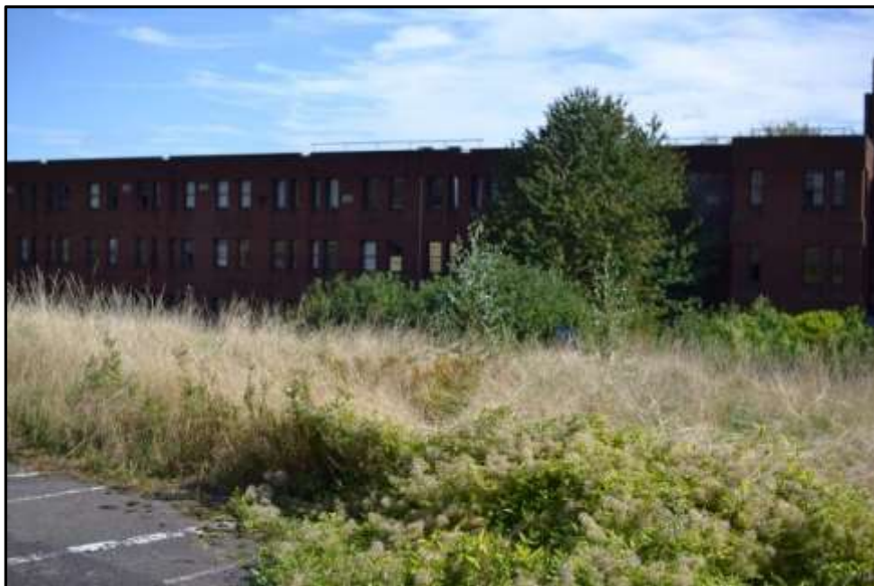
Plate 21f – Building 21, part west elevation (central portion)
