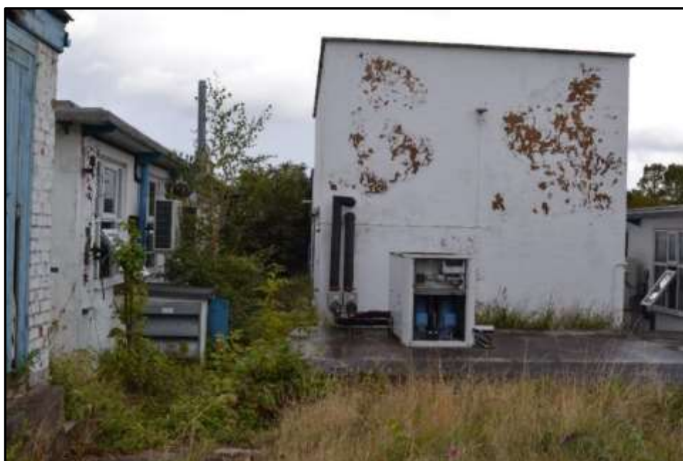
Plate 13b – Building 13, south elevation
