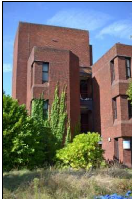
Plate 21d – Building 21, east elevation of entrance range
