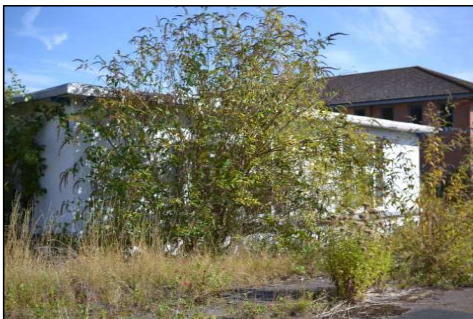
Plate D18 – D Block, south end elevation of spur 1
