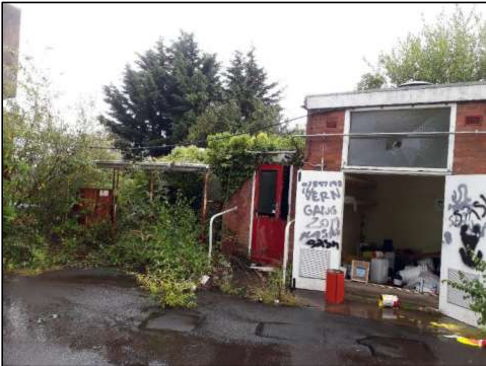
Plate 6a – Building 6, north elevation of lower section
