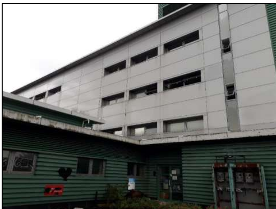
Plate 3b – Building 3, part south elevation of main range and part east elevation of south addition
