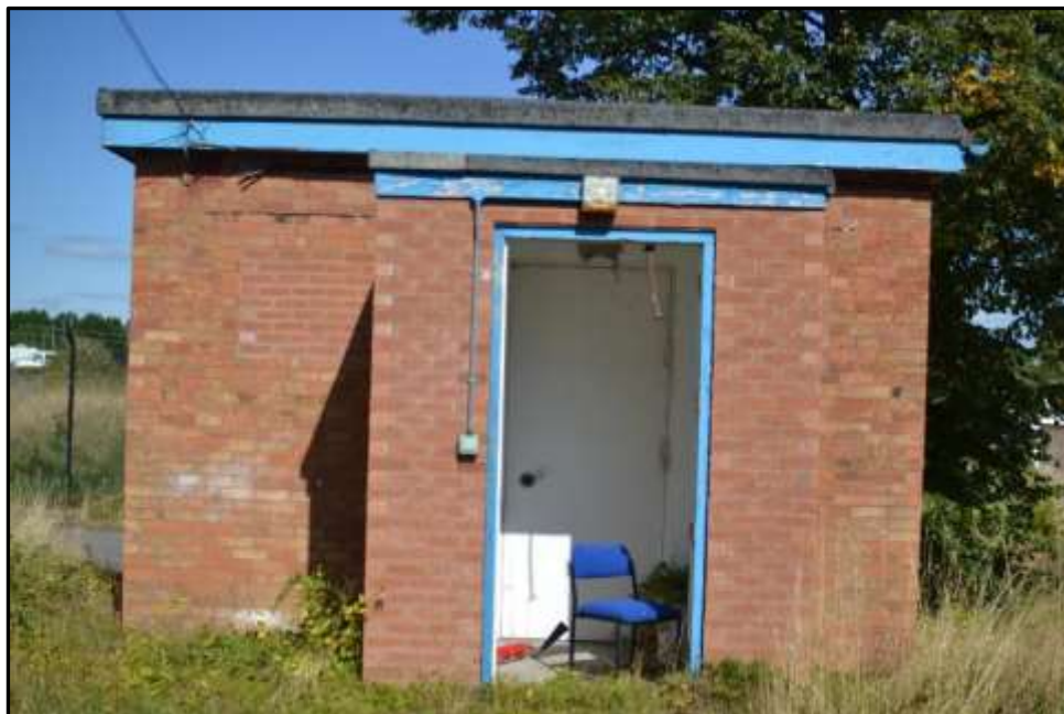
Plate 22a – Building 22, south elevation; porch addition is later
