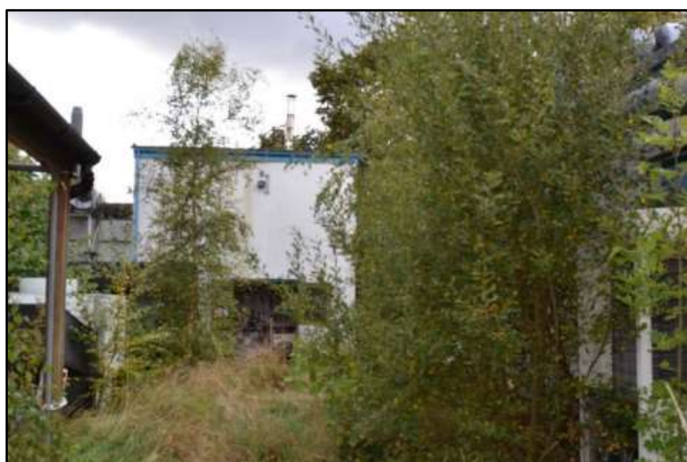
Plate 16b – Building 16, north elevation
