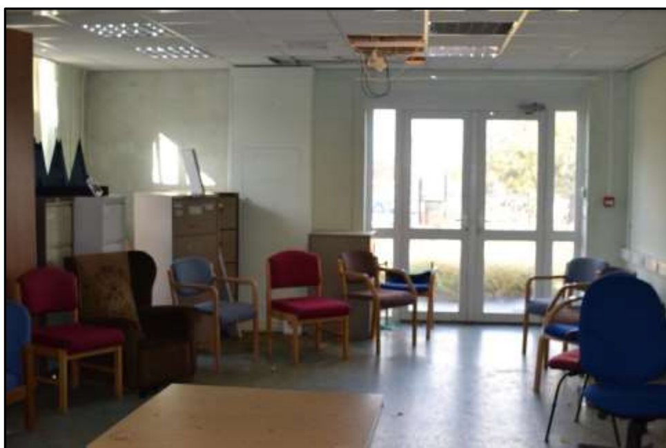
Plate E44 – E Block, interior of infill block between spurs 6 and 8
