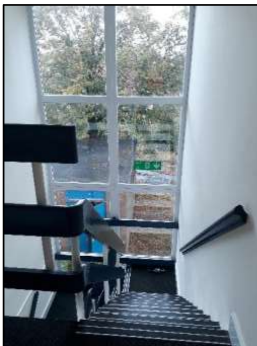
Plate H32 – H Building, stairs within the two storey extension to the north
