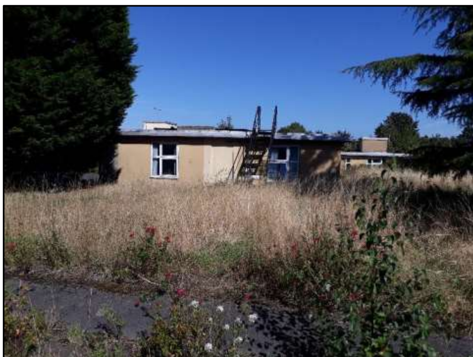
Plate A7 – A Block, south west end elevation of spur 5
