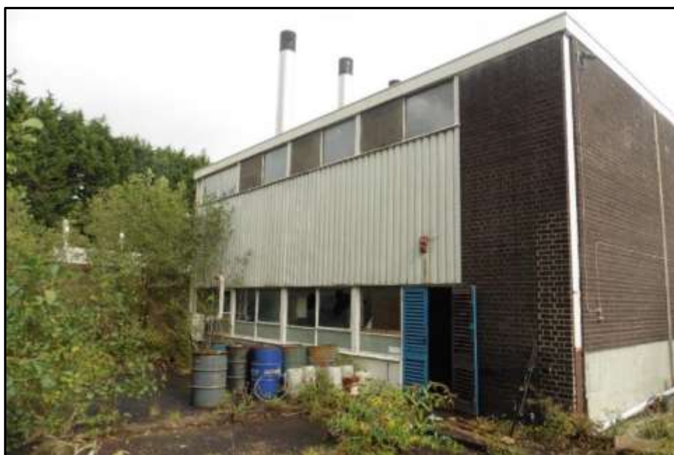
Plate 19b – Building 19, north elevation
