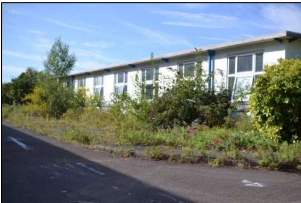
Plate D13 – D Block, east elevation of spur 2
