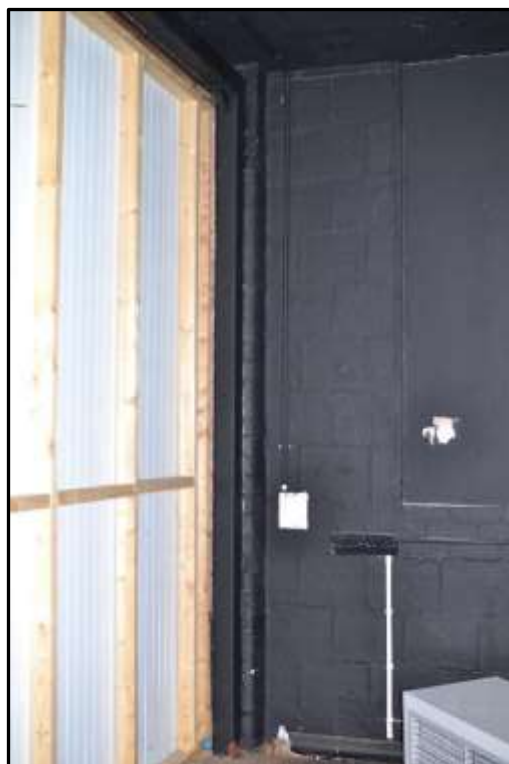
Plate E50 – E Block, spur 6, rounded edge of structural brick column exposed within later alterations to the interior
