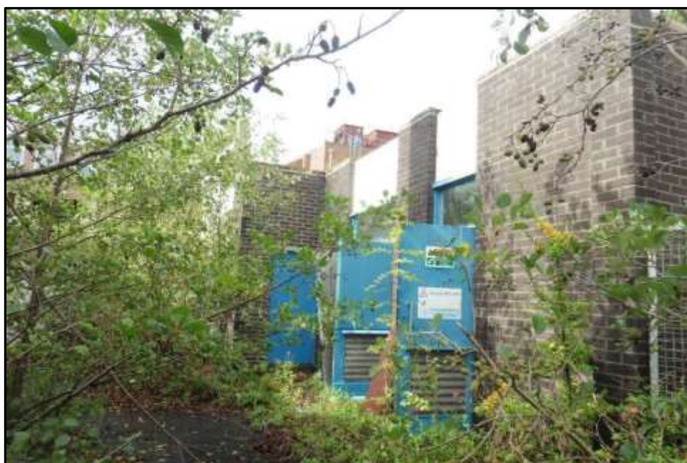
Plate 18b – Building 18, south elevation
