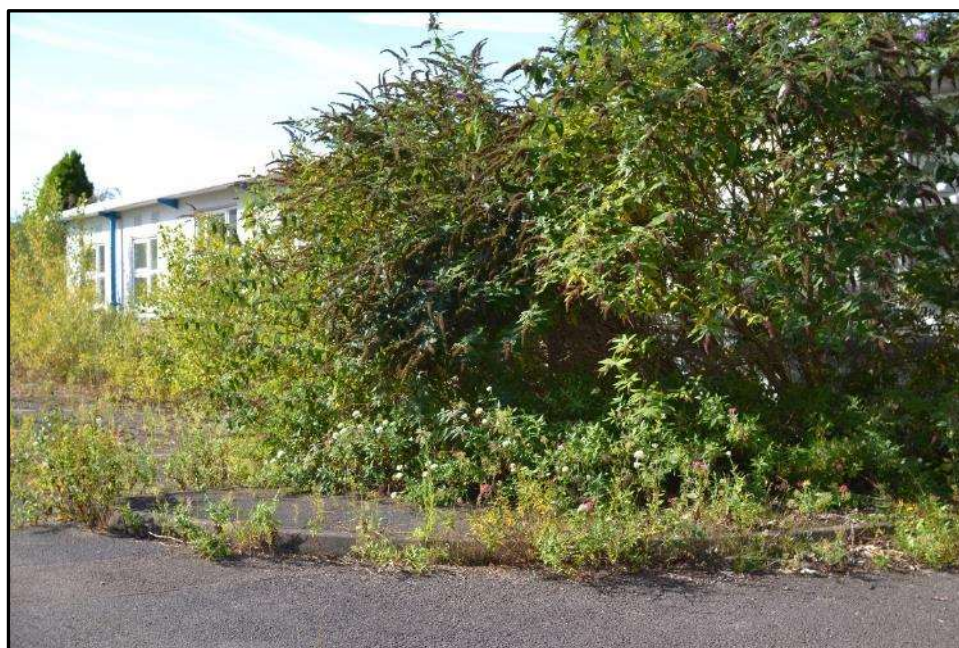
Plate D16 – D Block, east elevation of spur 1
