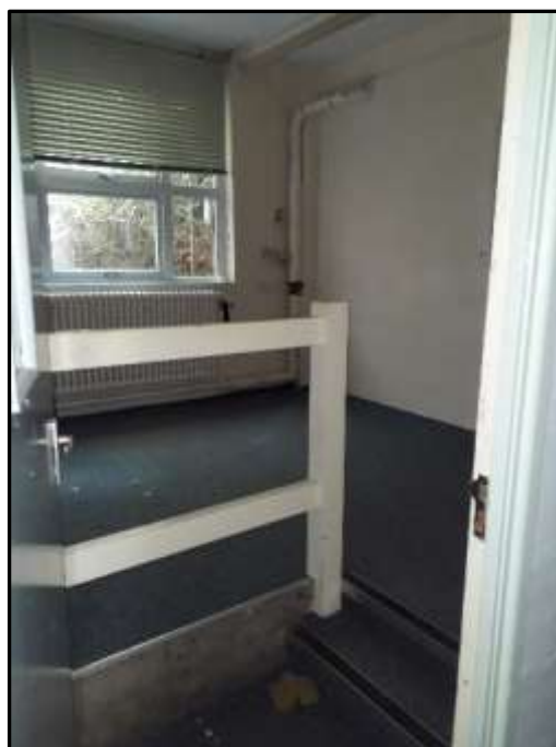
Plate A38 – A Block, evidence of internal alteration to spur 6 with floor level raised
