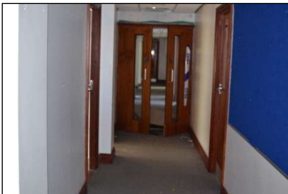
Plate E48 – E Block, altered secondary corridor to spur 5
