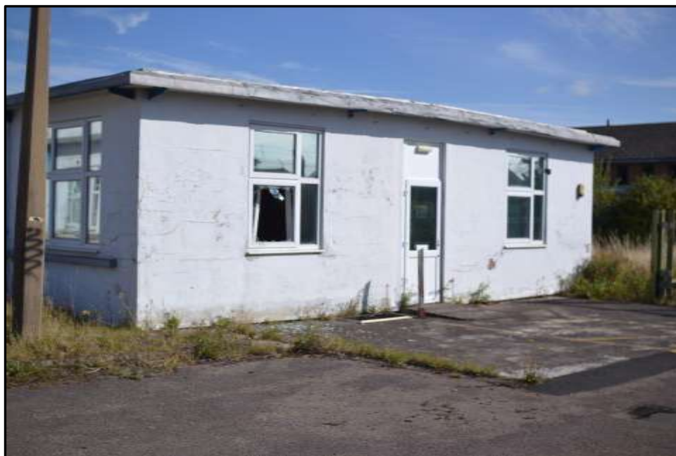
Plate D21 – D Block, south end elevation of spur 3
