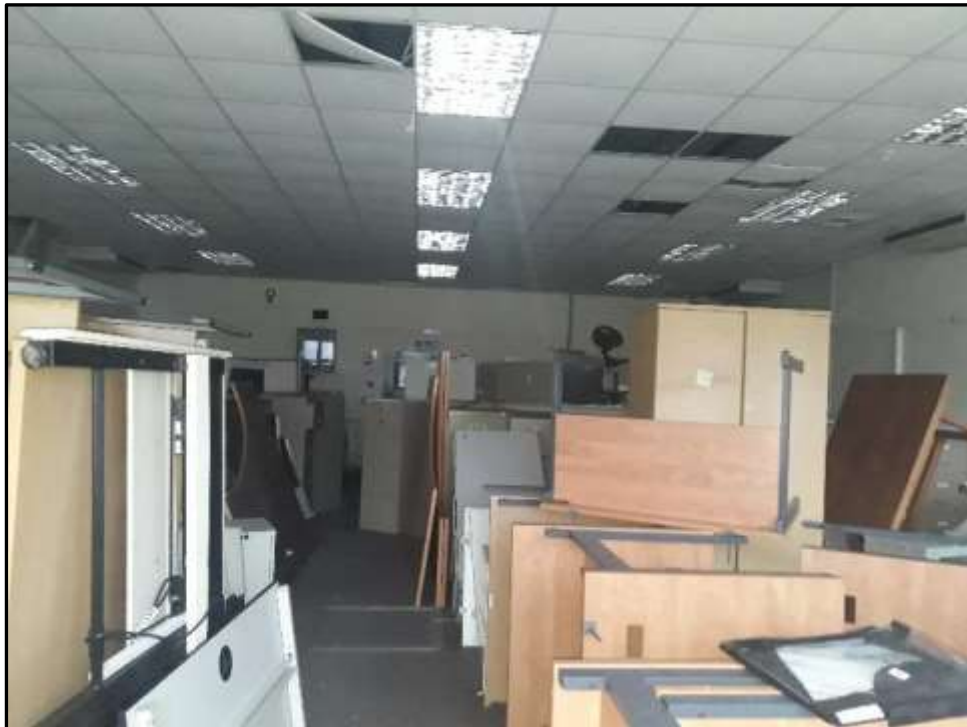
Plate H27 – H Building, ground floor office (former radar room)
