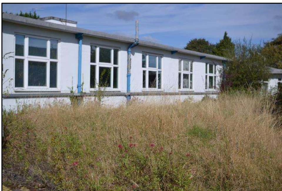
Plate D20 – D Block, east elevation of spur 3
