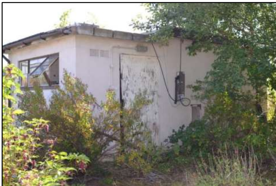
Plate 25a – Building 25, west elevation
