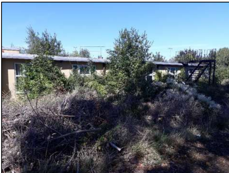
Plate A13 – A Block, south east elevation of spur 8
