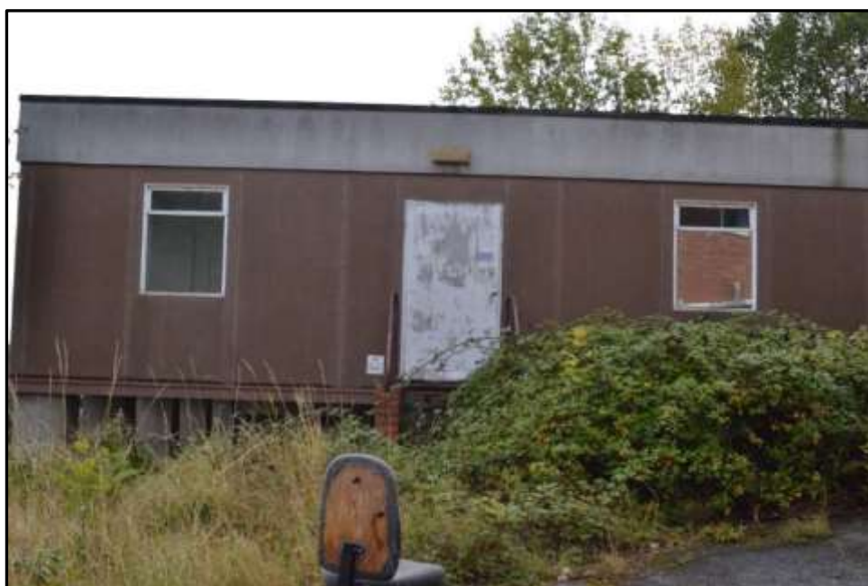
Plate 10e – Building 10, north elevation
