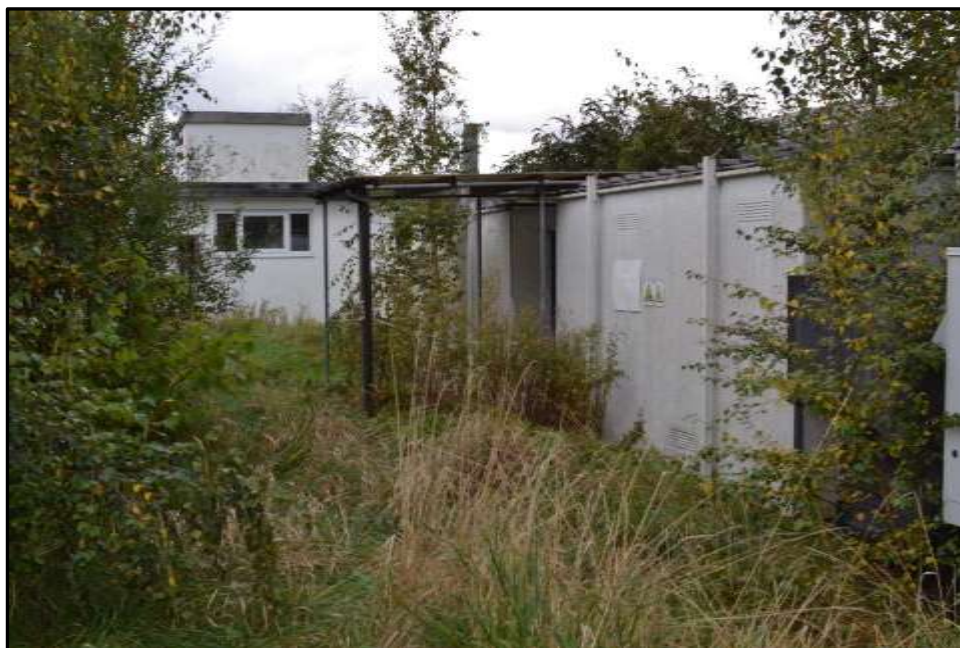
Plate E9 – E Block, west elevation of spur 11
