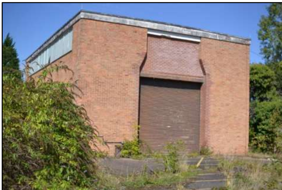
Plate 28d – Building 28, south east elevation
