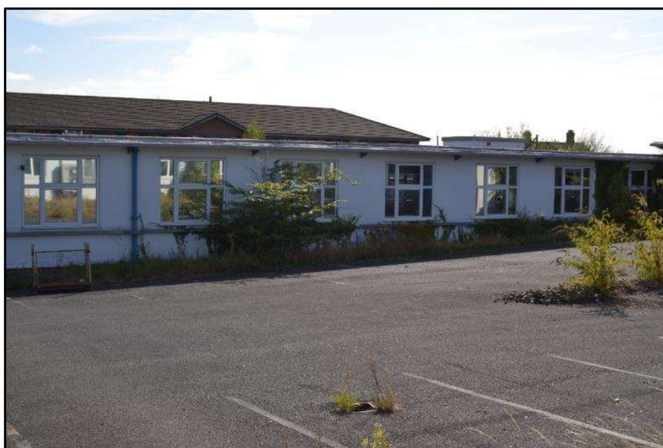
Plate D8 – D Block, west elevation of spur 4
