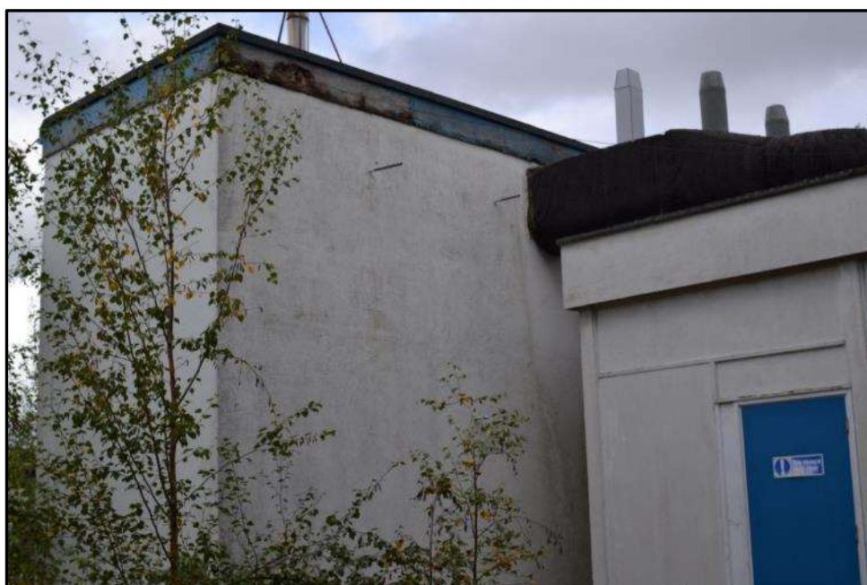
Plate 16a – Building 16, part south and west elevations
