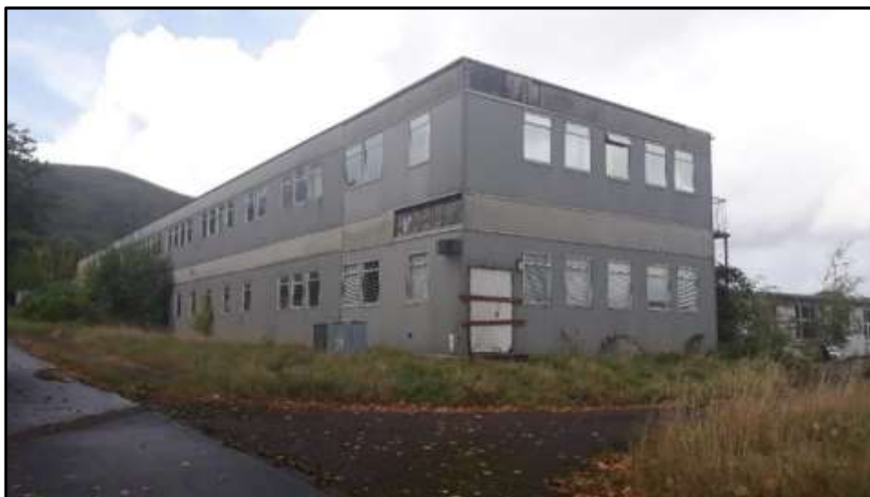
Plate 15a – Building 15, East and part south elevations
