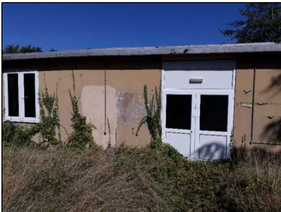
Plate A25 – A Block, south west end elevation of spur 1
