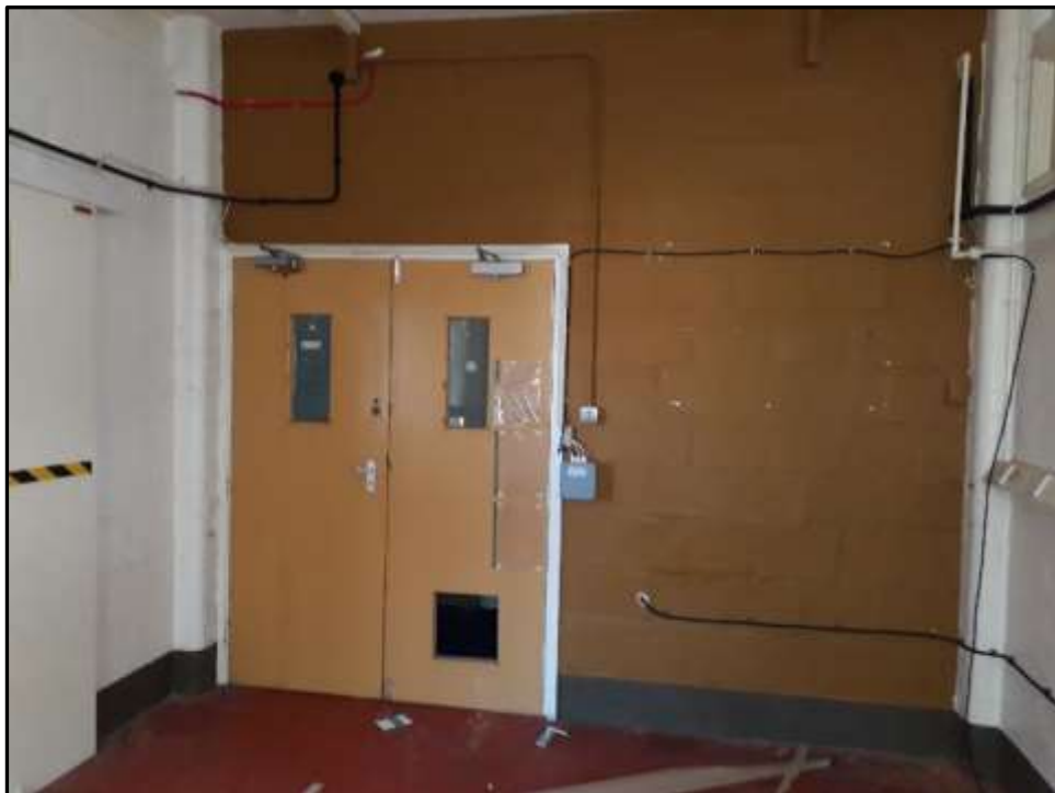
Plate A40 – A Block, evidence of most recent research and laboratory use of the internal spaces (spur 6), note the original rounded edge of the brick columns and the brick tile internal walls retained
