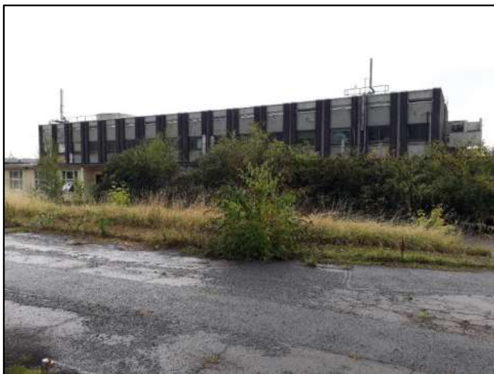
Plate 37i – Building 37, west elevation with KF block to the foreground (partially concealed by vegetation)
