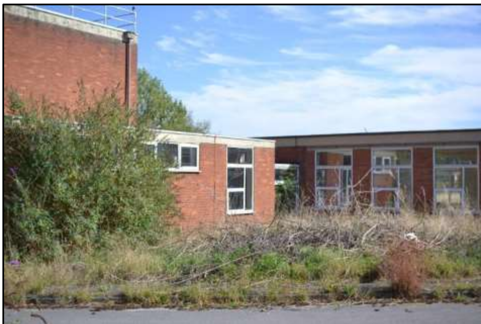
Plate 24g – Building 24, part west and south elevations
