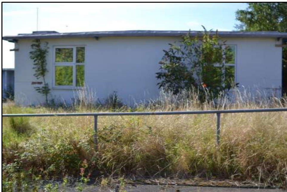
Plate D4 – D Block, north elevation of spur
