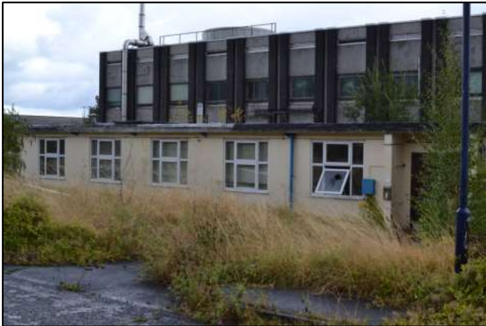
Plate KF5 – Part west elevation with M Block (Building 37) to the rear
