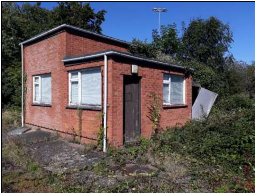
Plate 35a – Building 35, south west and south east elevations
