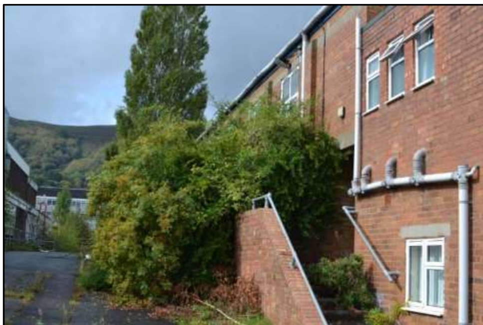
Plate 8g – Building 8, part south elevation of the south range
