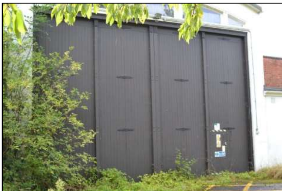
Plate 36e – Building 36, entrance doors to the stratosphere chamber
