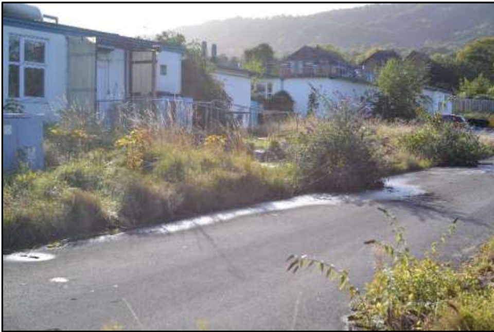
Plate E21 – E Block, north end elevations of spurs 6, 4 and 2
