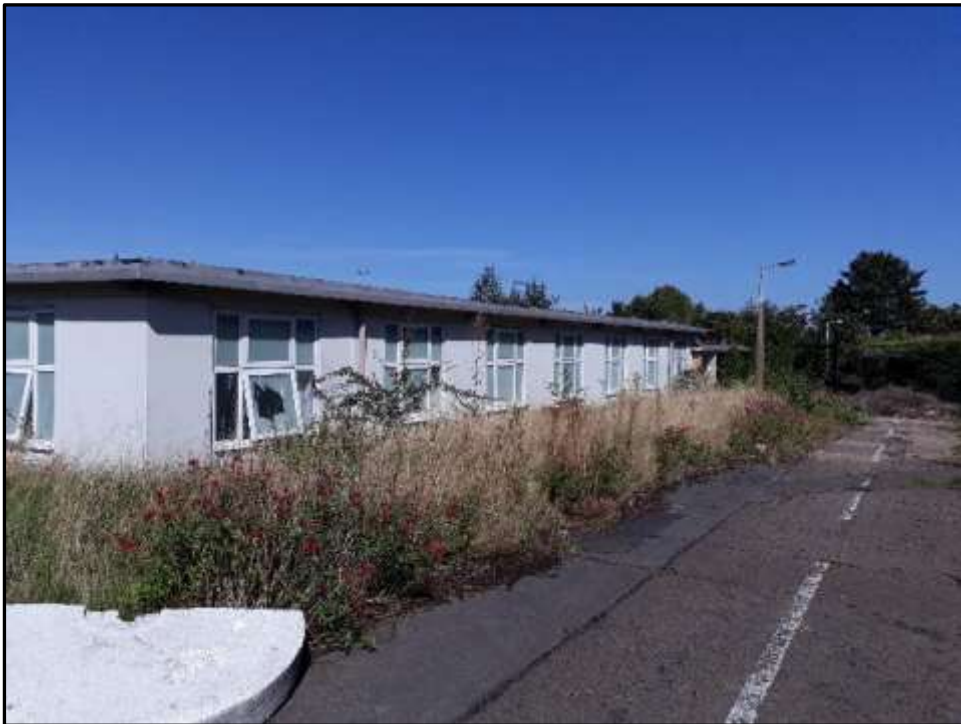
Plate A11 – A Block, south east elevation of spur 7
