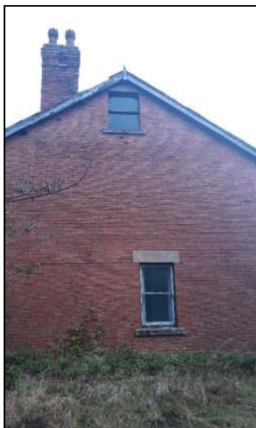
Plate T5 – T Block, south elevation
