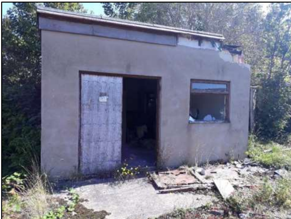
Plate 31a – Building 31, north west elevation
