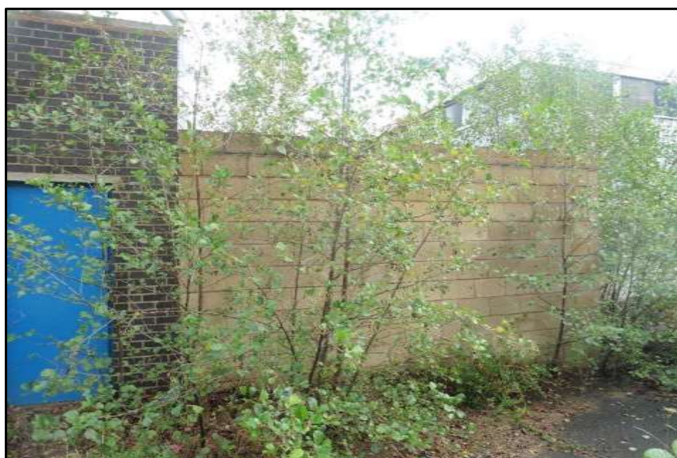
Plate 18d– Building 18, west elevation of blockwork enclosure
