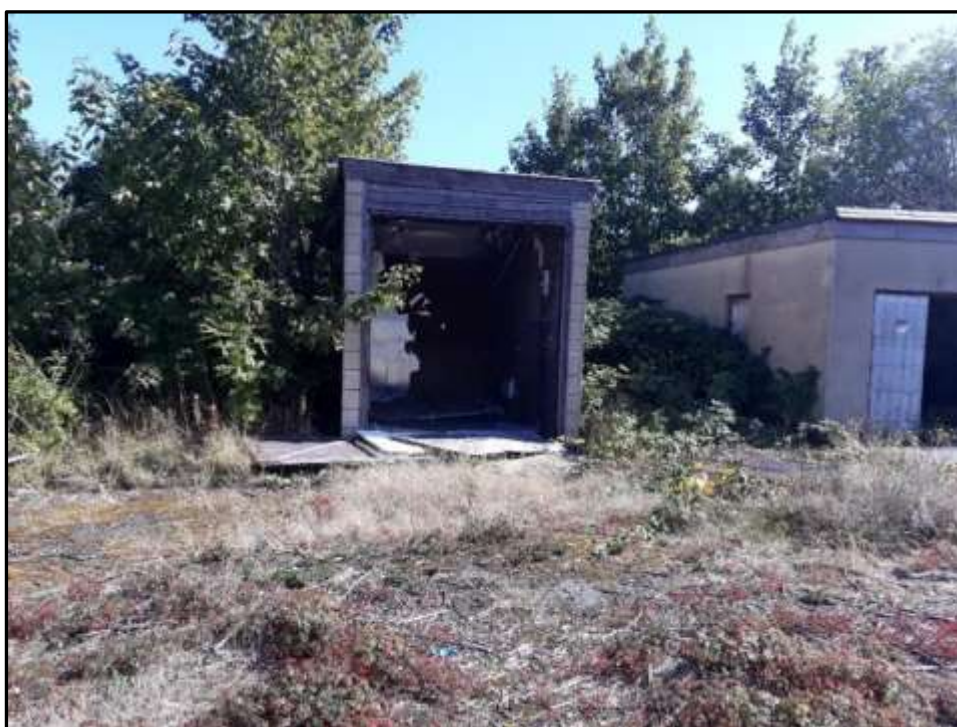
Plate 32a – Building 32, north west elevation and north east elevation of building 32
