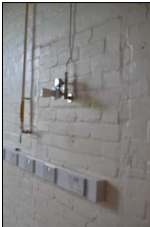
Plate E52 – E Block, evidence of blocked opening observed in spur 12
