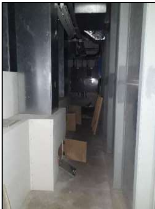
Plate H43 – H Building, perimeter corridor within former bunker area
