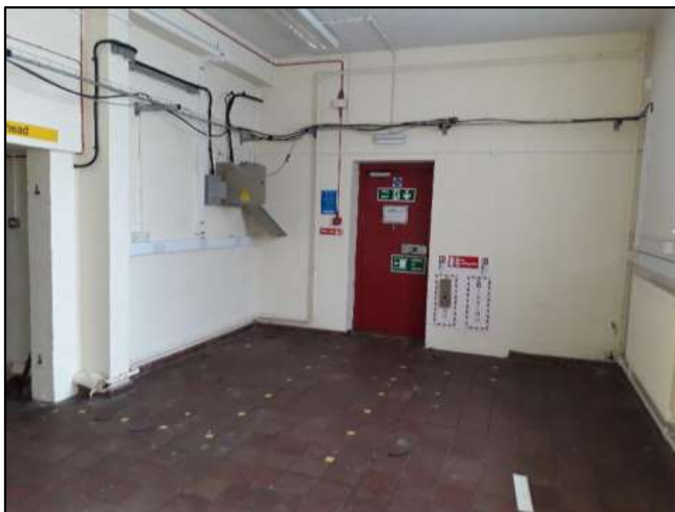
Plate H36 – H Building, former battery room within the north extension
