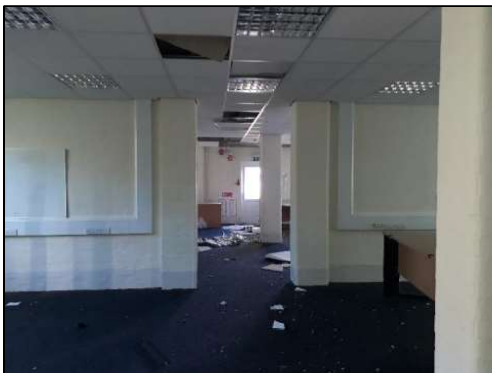
Plate D51 – D Block, interior of part of spur 8
