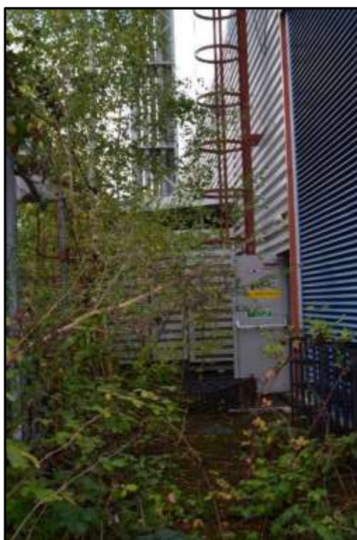
Plate 17h – Building 17, part west elevation of main range and south elevation of single storey link to E Block
