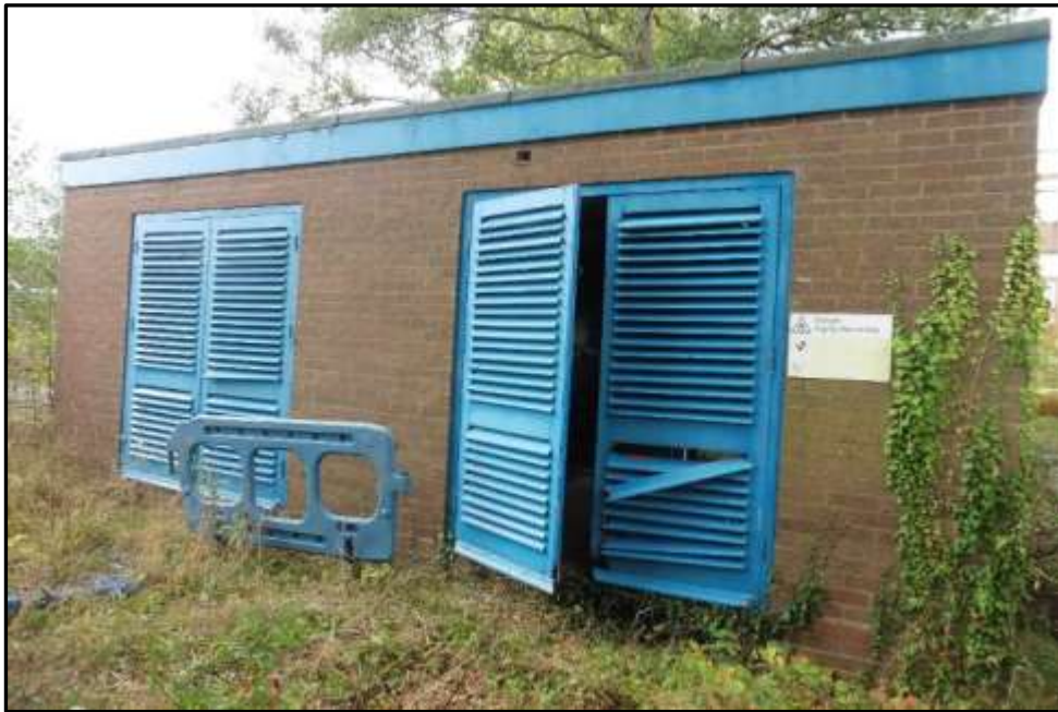
Plate 20a – Building 20, east elevation
