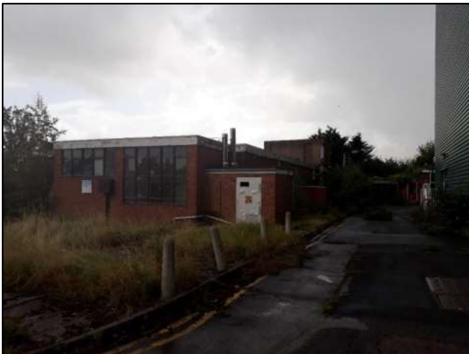
Plate 7a – Building 7, north elevation and part west elevation
