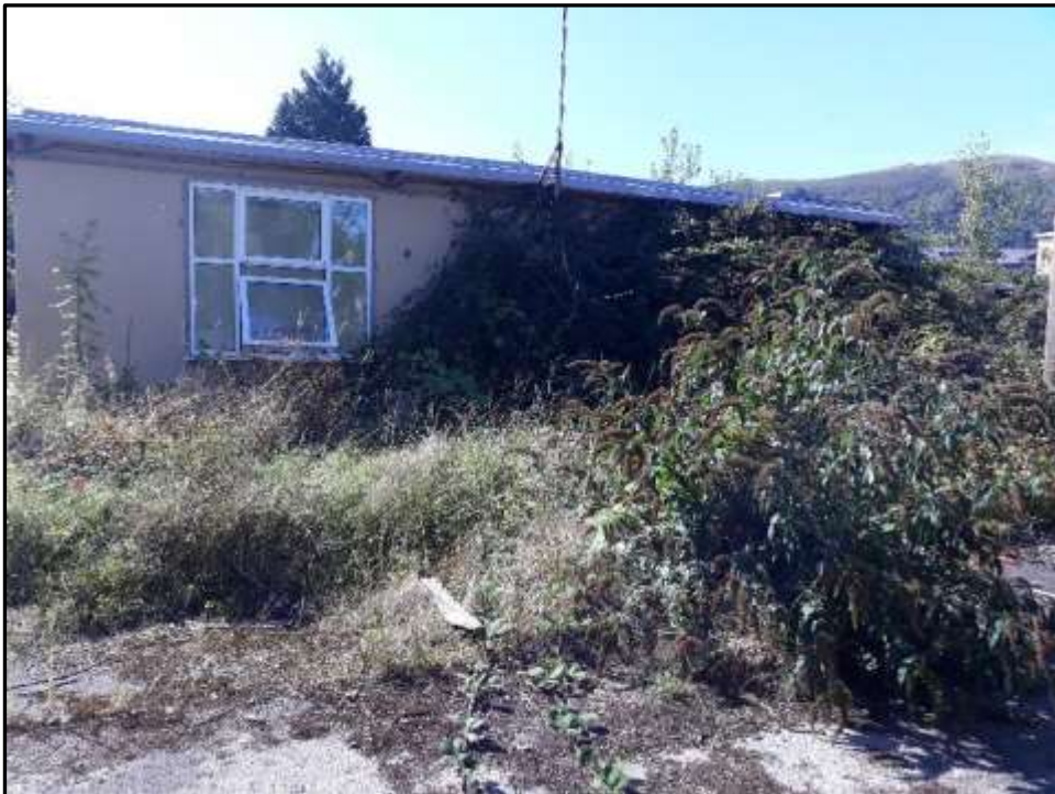
Plate A17 – A Block, north east elevation
