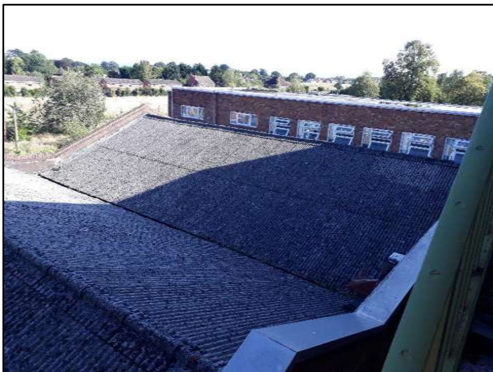
Plate H22 – H Building, corrugated cementitious type sheet roof to the gable east rooms and the north elevation of the first-floor addition to the south range
