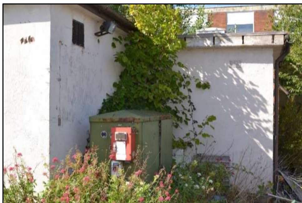
Plate 25b – Building 25, part east and north elevations
