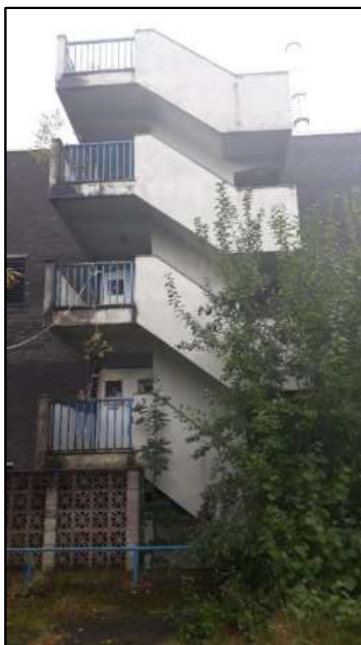
Plate 37b – Building 37, external concrete staircase to the north elevation
