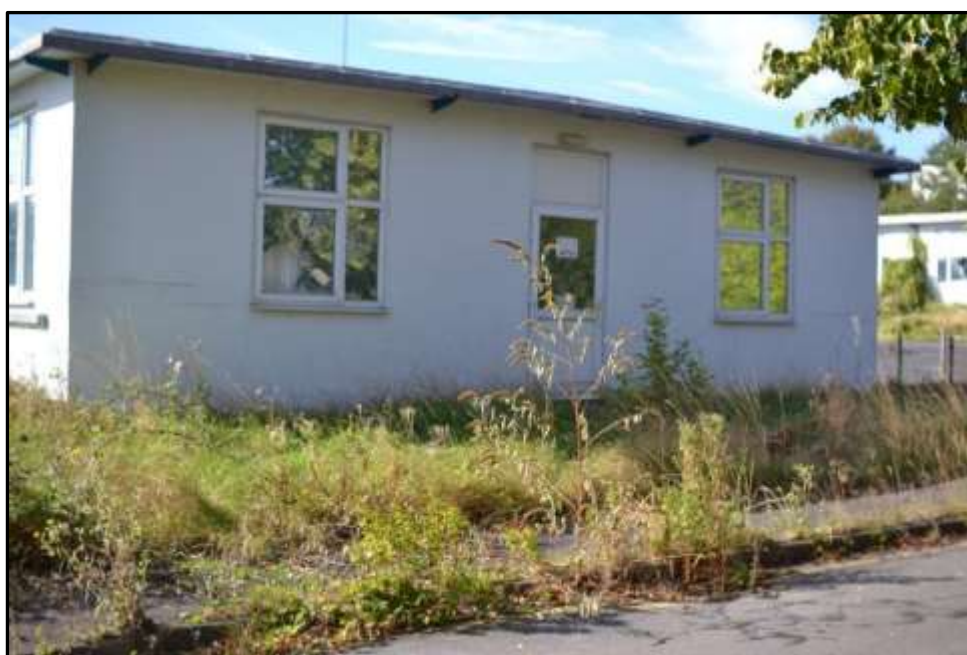
Plate D10 – D Block, north elevation of spur 4
