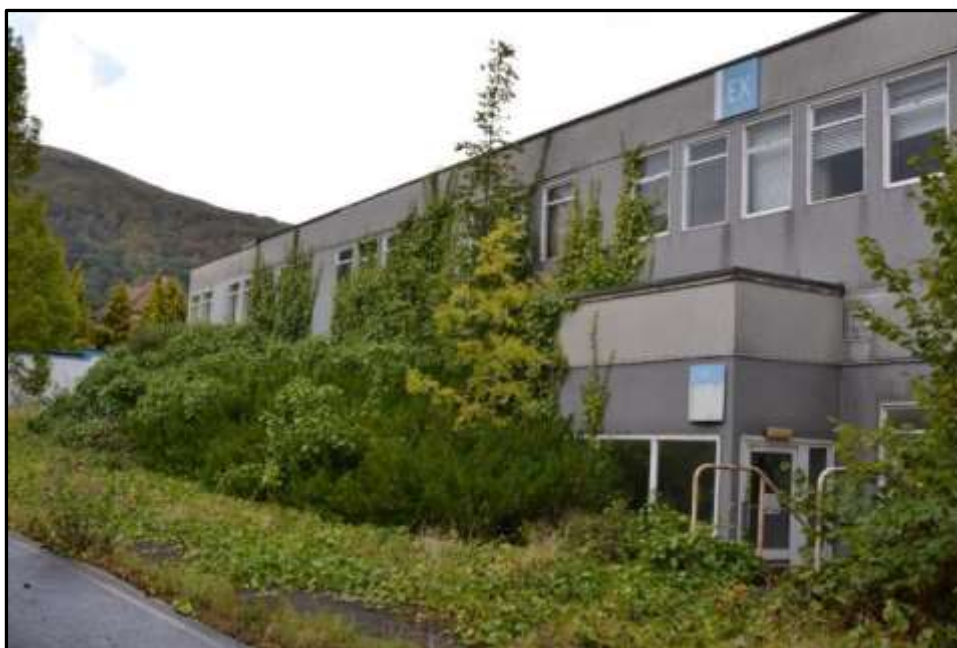
Plate 15b – Building 15, part south elevation with main entrance
