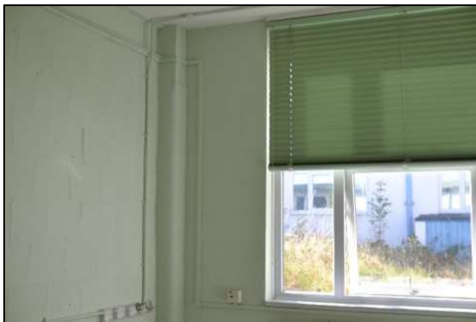
Plate E54 – E Block, remains of structural brick column with chamfered stops to top end. Common feature throughout the block where the early configuration remains (observed in small room to spur 4)
