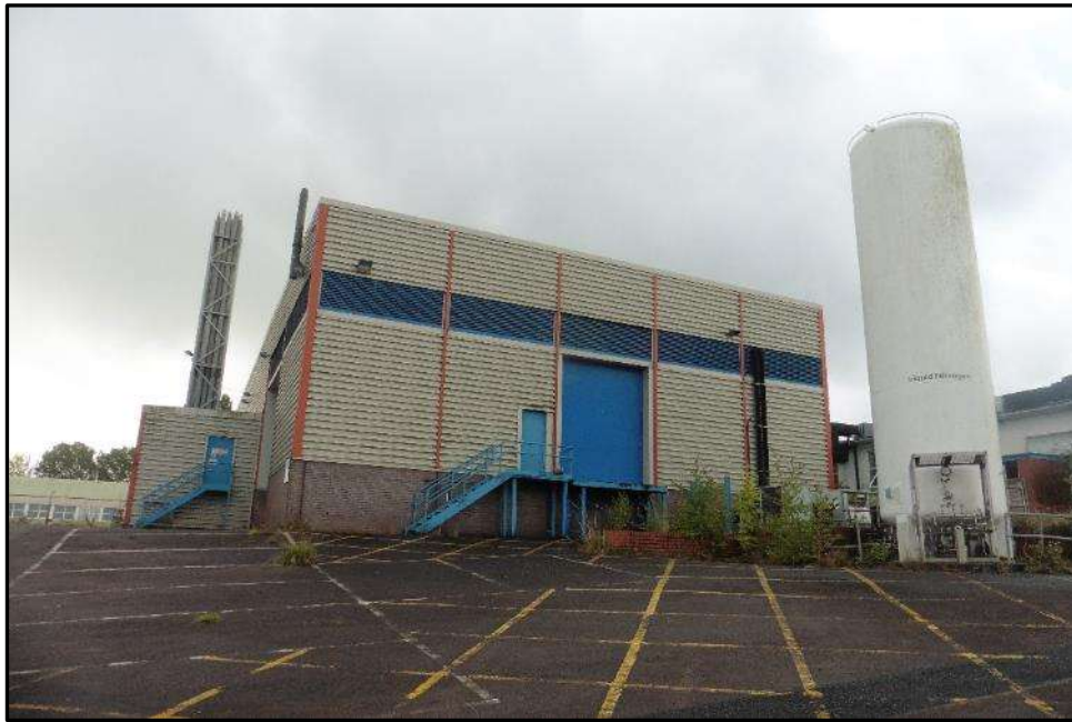
Plate 17a – Building 17, north elevation
