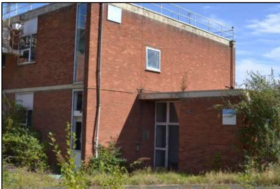
Plate 24i – Building 24, part south and west elevations of main two storey range
