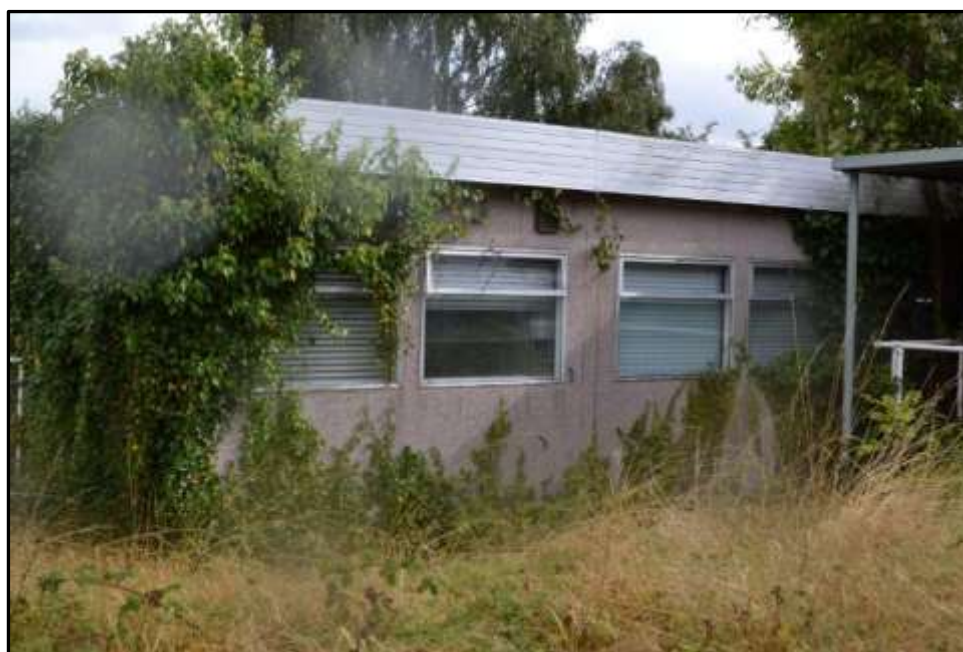
Plate 4d – Building 4, west elevation
