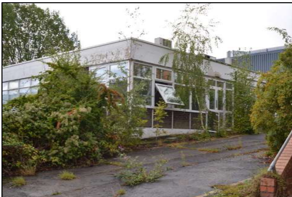
Plate 9i – Building 9, part north and east elevations
