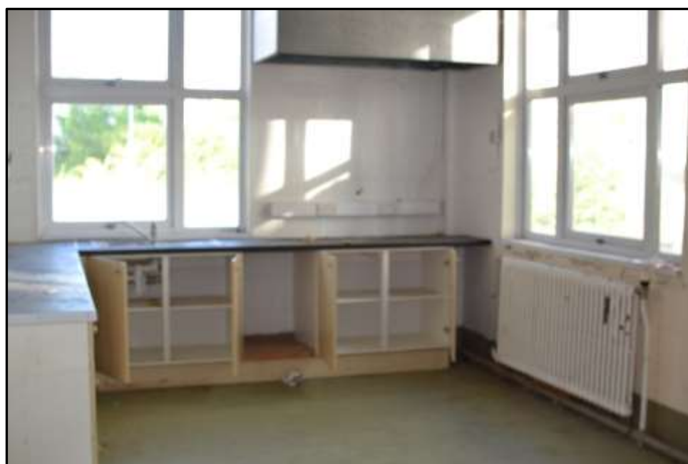
Plate KF12 – North west room showing more recent intervention with modern fixtures and fittings
