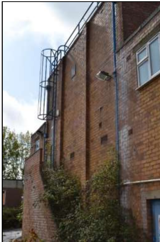
Plate 8c – Building 8, east elevation of south range
