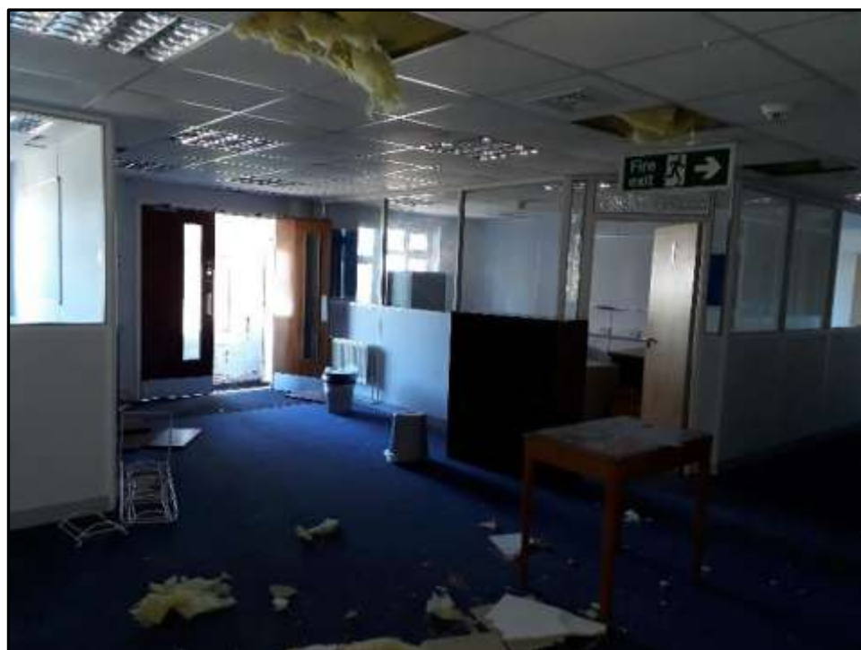
Plate L20 – Library building, lobby entrance area from the north east porch
