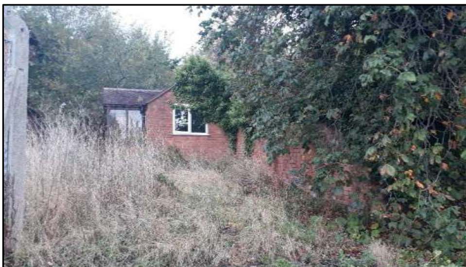
Plate T1 – T Block, part south and east elevations of the detached former garage range
