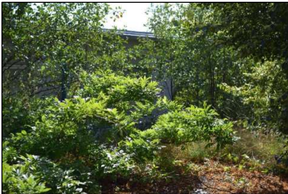
Plate D30 – D Block, obscured west elevation of spur 7
