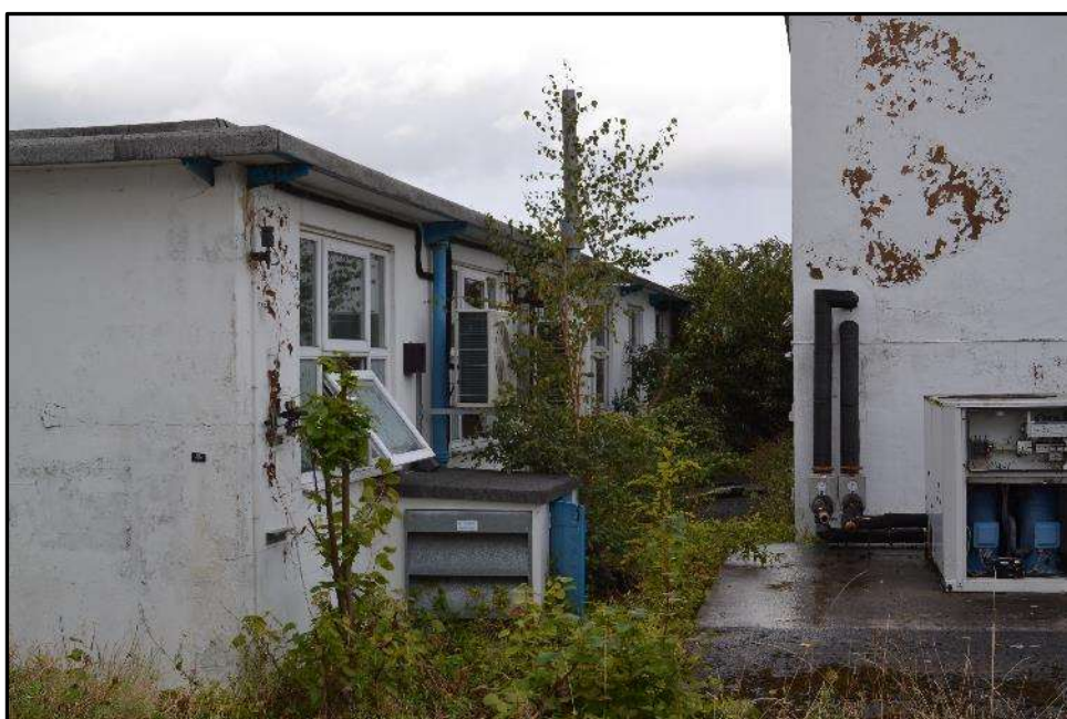
Plate E2 – E Block, east elevation of spur 1
