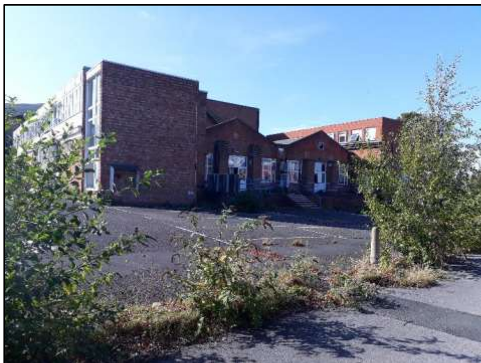
Plate H16 – H Building, east elevation
