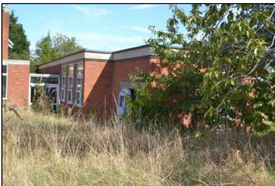
Plate 24f – Building 24, part west elevation of single storey range to east
