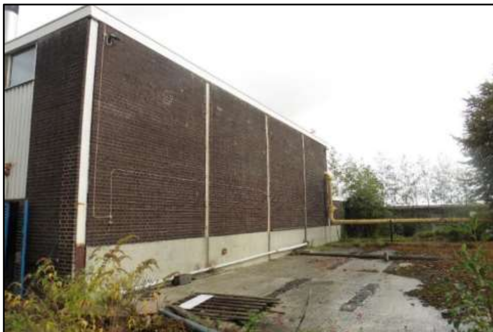
Plate 19a – Building 19, south elevation, note gas pipe extending towards building 20
