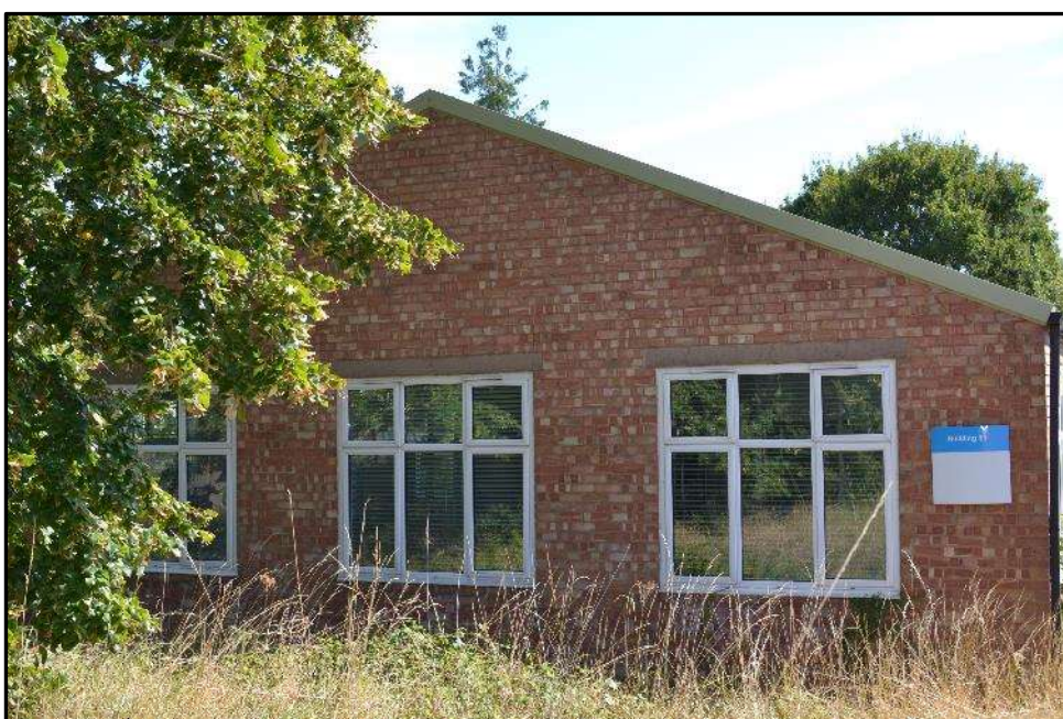
Plate L8 – Library building, north west end elevation of the later south west range
