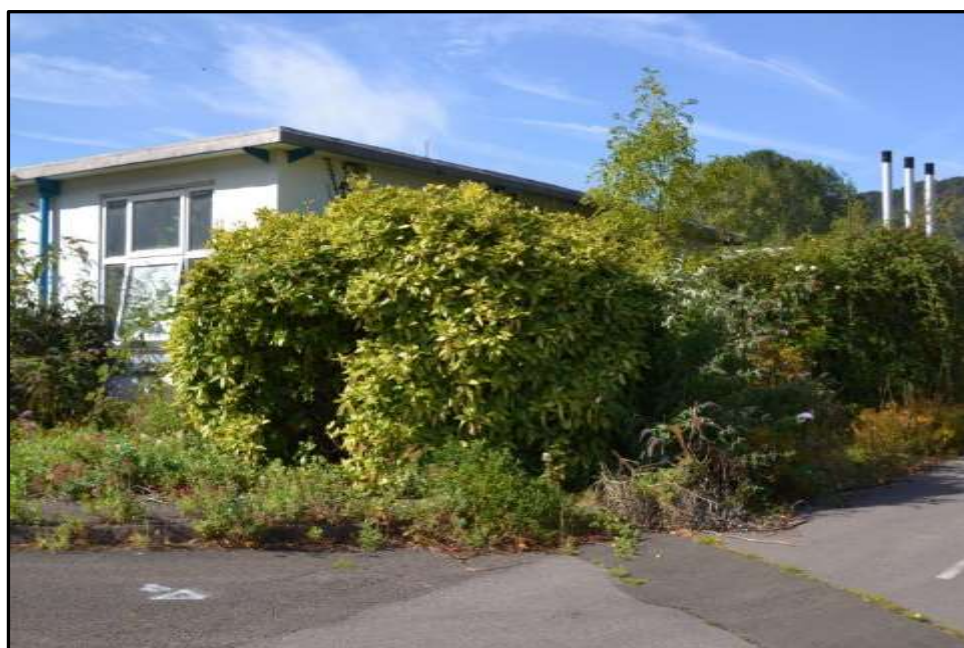
Plate D12 – D Block, obscured north elevation of spur 2
