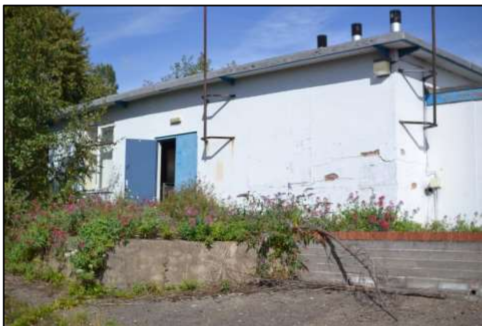
Plate D28– D Block, south end elevation of spur 7
