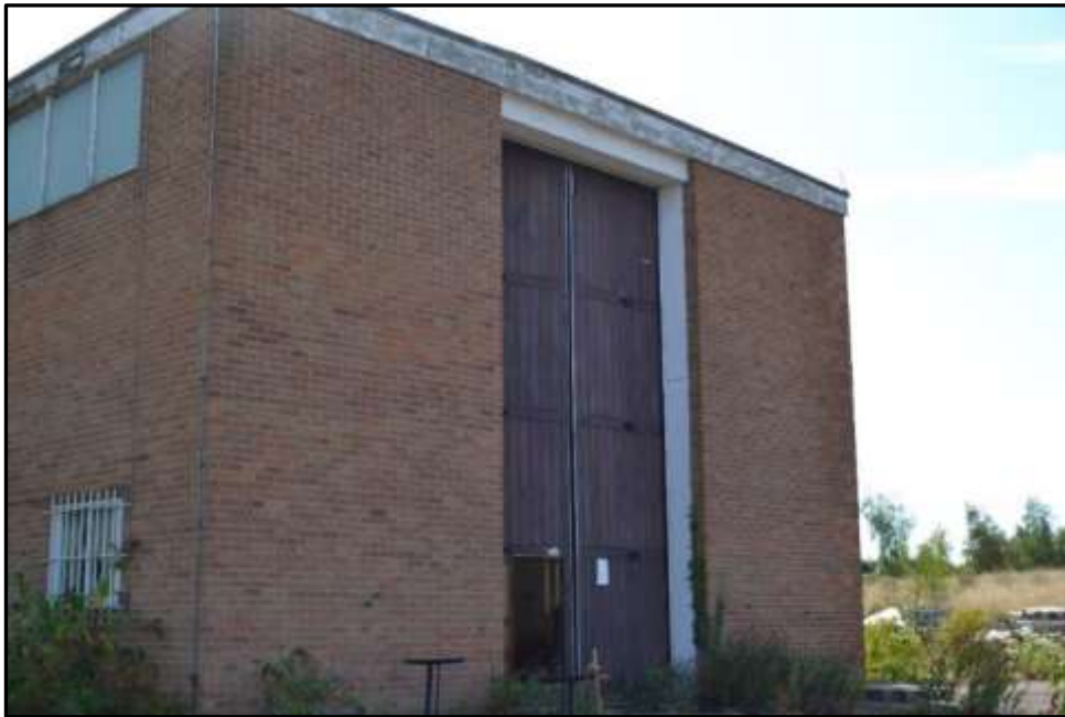
Plate 28b – Building 28, north west elevation
