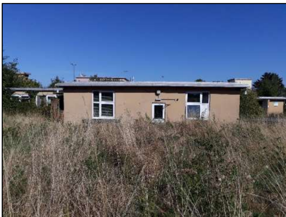
Plate A27 – A Block, south west end elevation of spur 3
