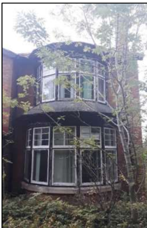
Plate T6 – T Block, two storey bow window to the west frontage
