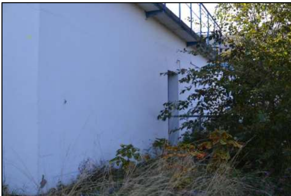
Plate E17 – E Block, part west elevation of spur 4
