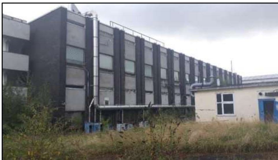
Plate 37a – Building 37, west elevation
