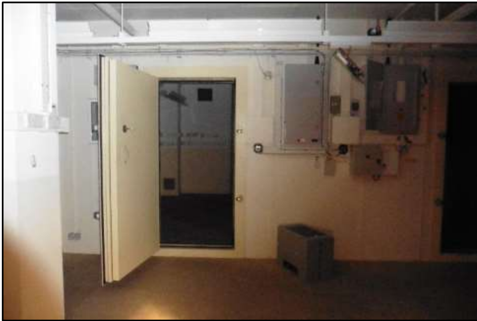
Plate H47 – H Building, ground floor of former bunker. Two small ‘pods’ built into the northern wall of the faraday cage with thick, metal security doors. Room to the right is the former computer server room and room to the left served as a secure research area
