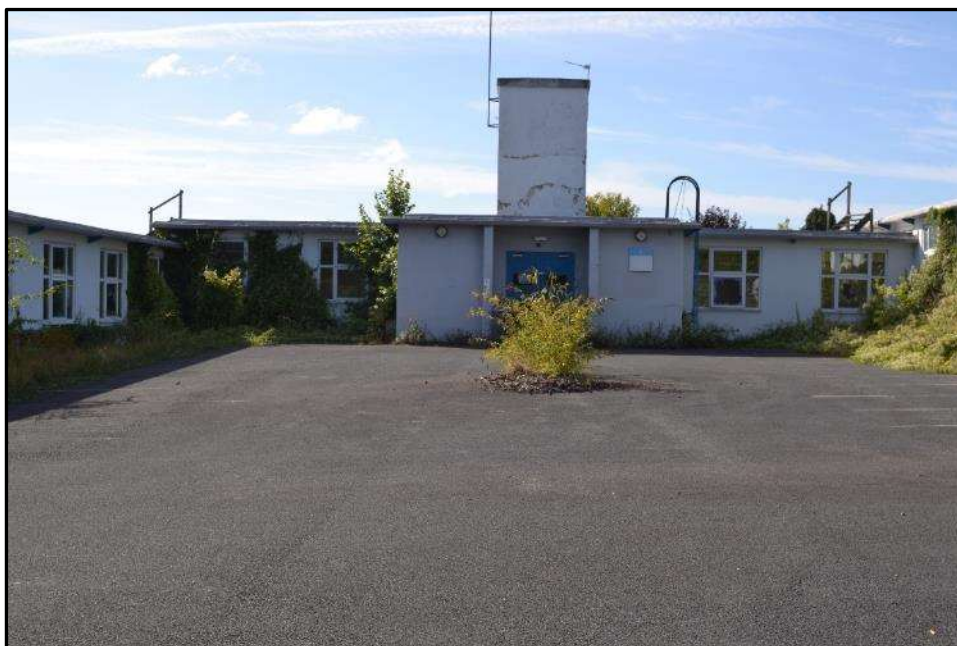
Plate D6 – D Block, north elevation with main centrally positioned entrance (flanked by spur 6, right, and spur 4, left)
