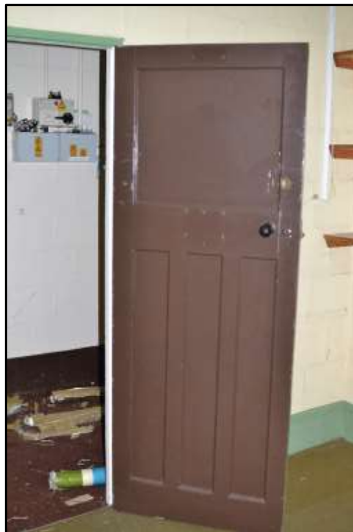
Plate KF16 – Early/original door within southern half of block
