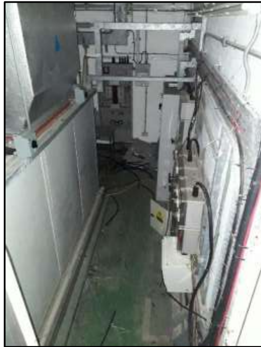
Plate H37 – H Building, plant room within the north west corner
