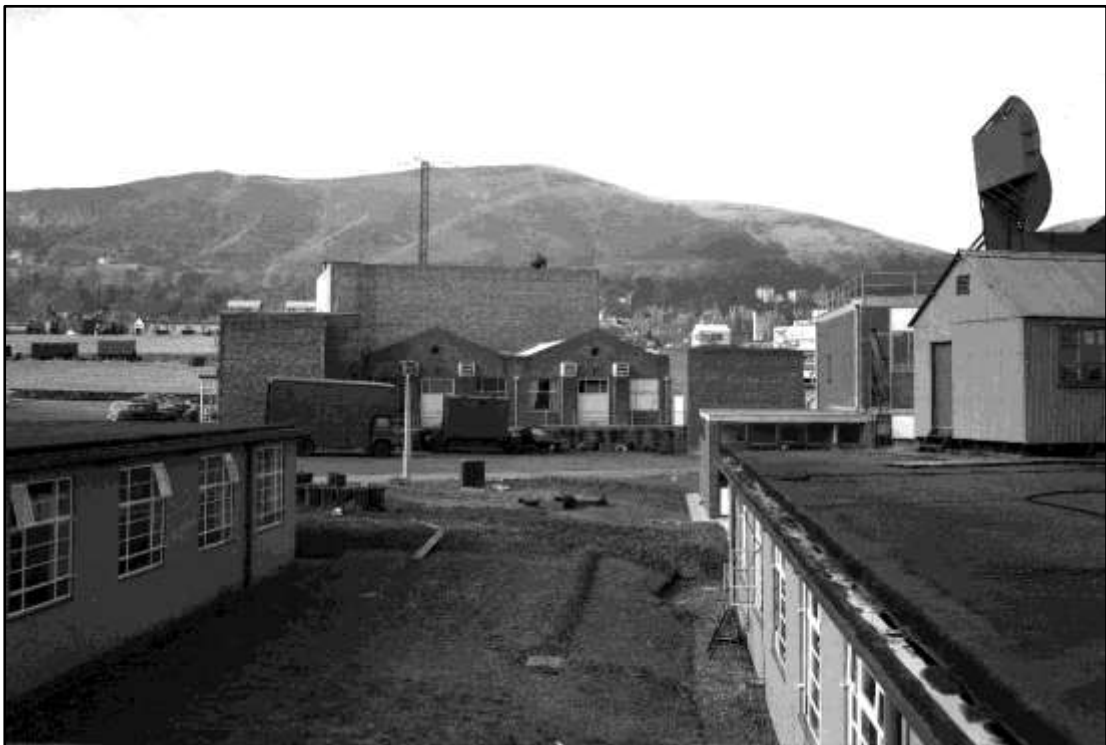
Image 7 - View towards the west elevation of H Building from the roof of B Block (now demolished). Image is undated however BY Block is visible to the right of the image so its likely early 1960s; note the large external radar satellite projecting from BY Block (Image reproduced with permission of MRATHS)
