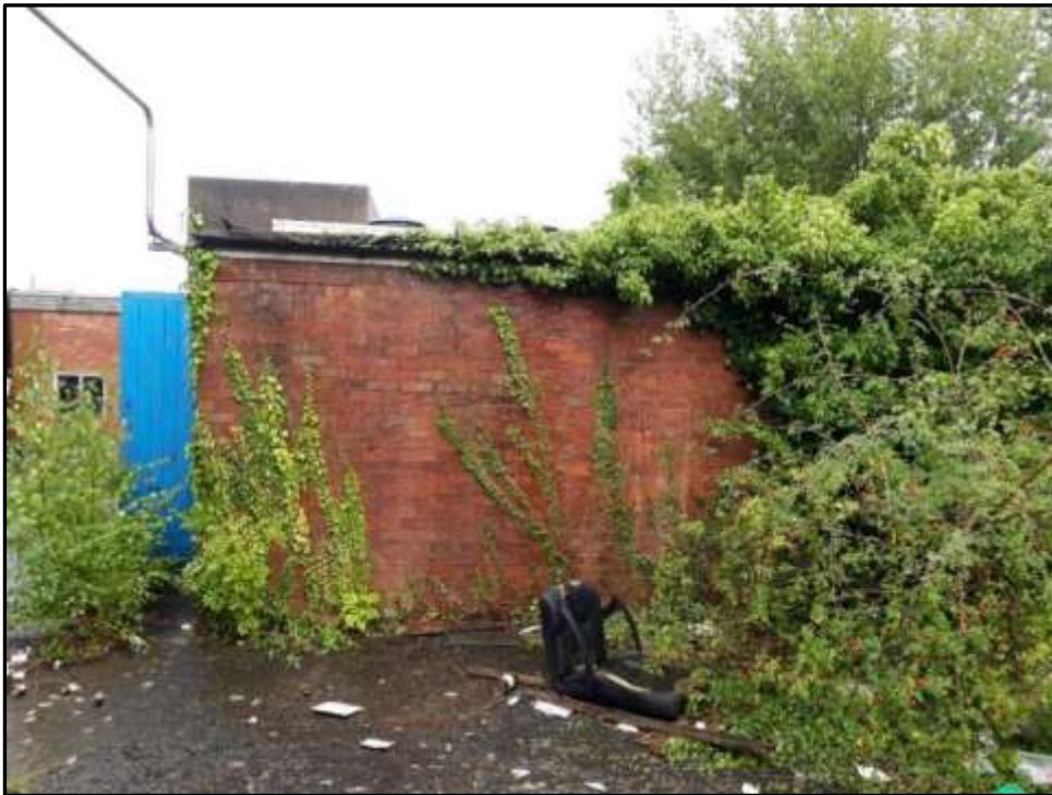
Plate 6c – Building 6, west elevation
