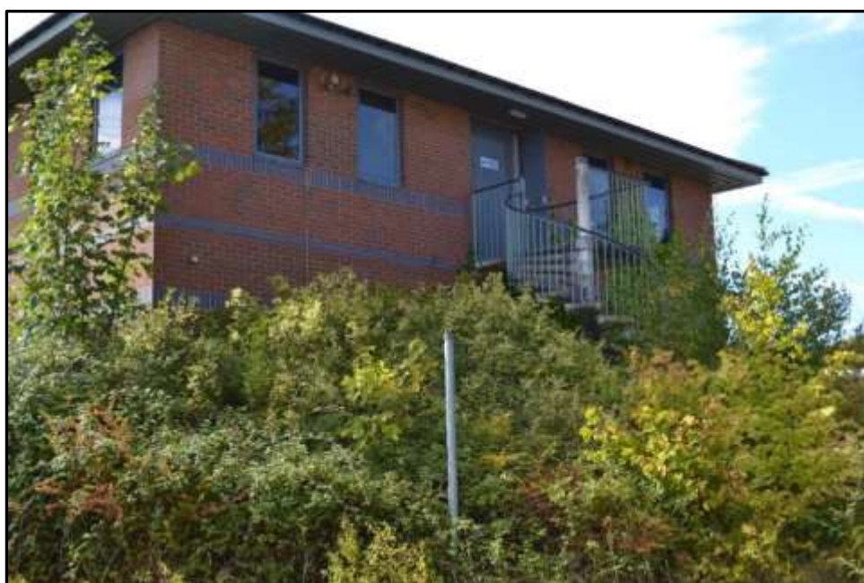
Plate 26b – Building 26, north elevation
