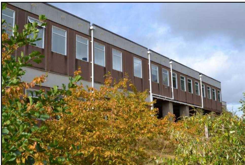
Plate 10a – Building 10, east elevation
