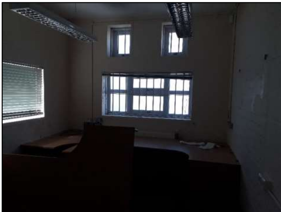
Plate D43 – D Block, spur 5. Most southern bay with original brickwork internal dividing wall to the right
