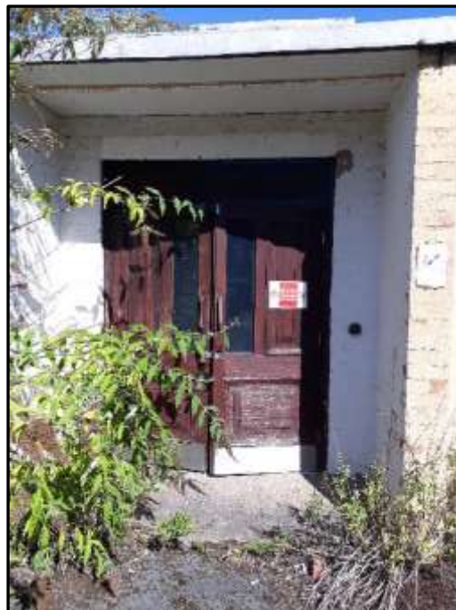
Plate A6 – A Block, timber doors to main south west entrance
