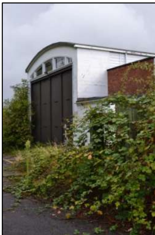
Plate 36d – Building 36, part north elevation with entrance to the stratosphere chamber
