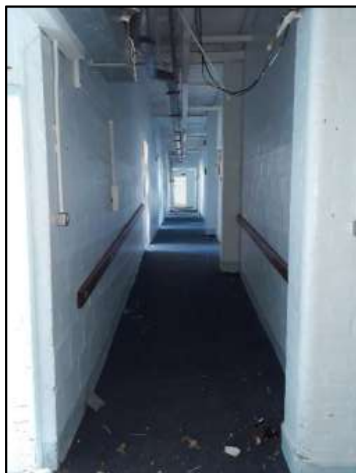
Plate A32 – A Block, secondary corridor to spur 7
