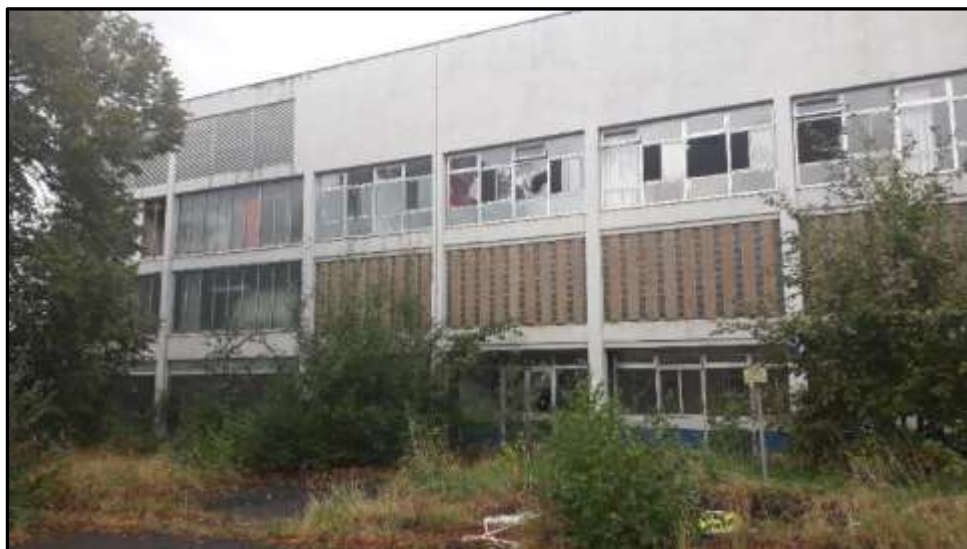
Plate 37d – Building 37, part north elevation with decorative concrete work panels
