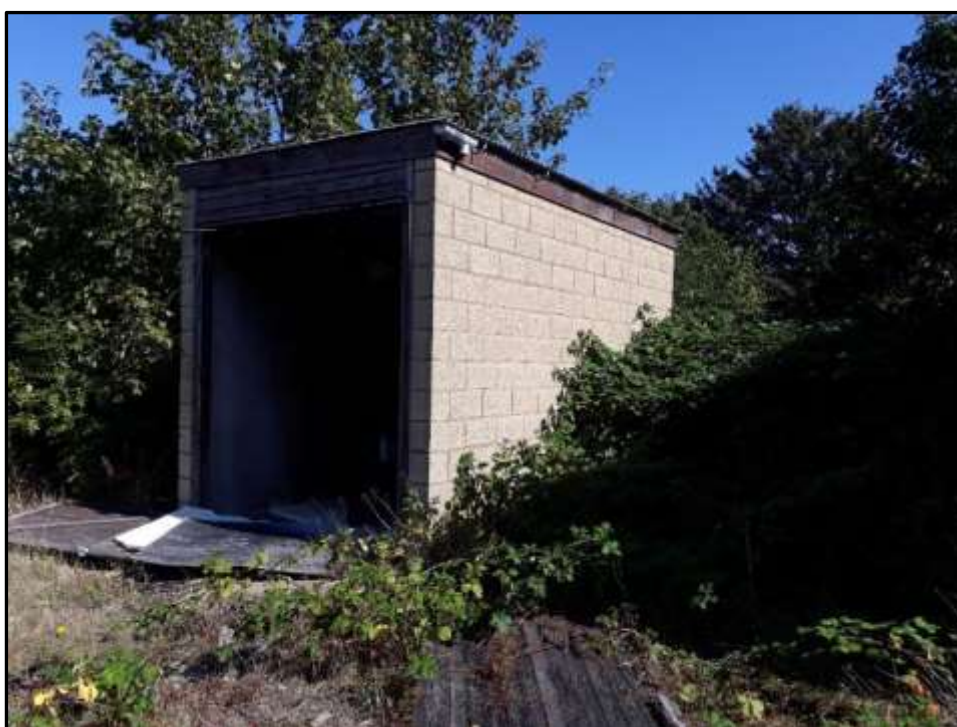
Plate 32b – Building 32, south east elevation
