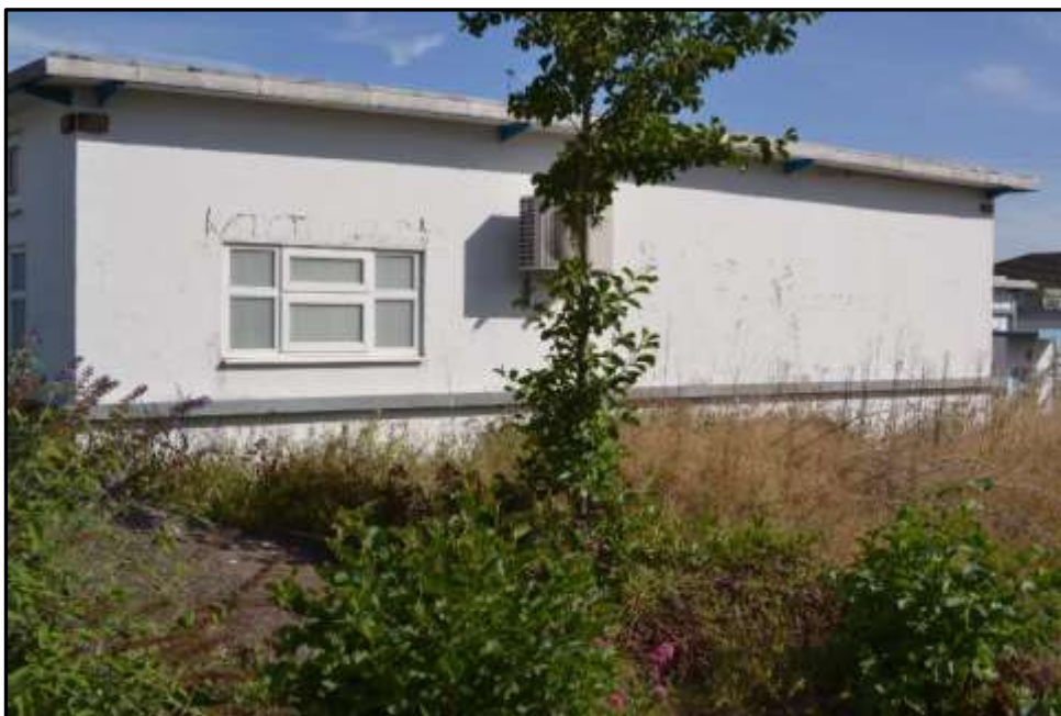
Plate D25 – D Block, south end elevation of spur 5
