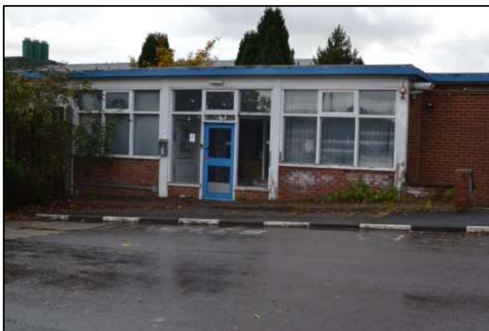
Plate 1a – Building 1 north elevation
