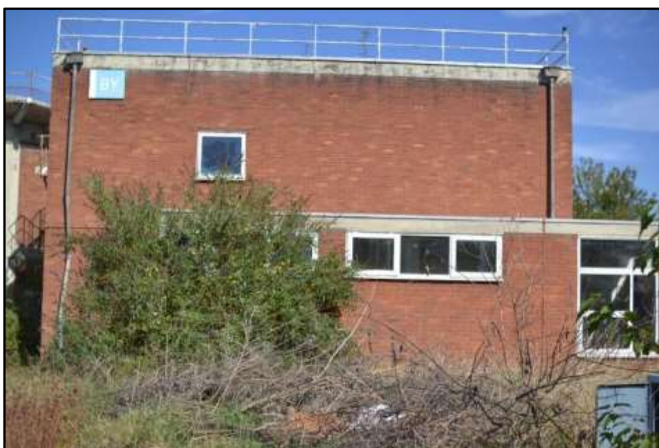
Plate 24h – Building 24, south elevation of main two storey range
