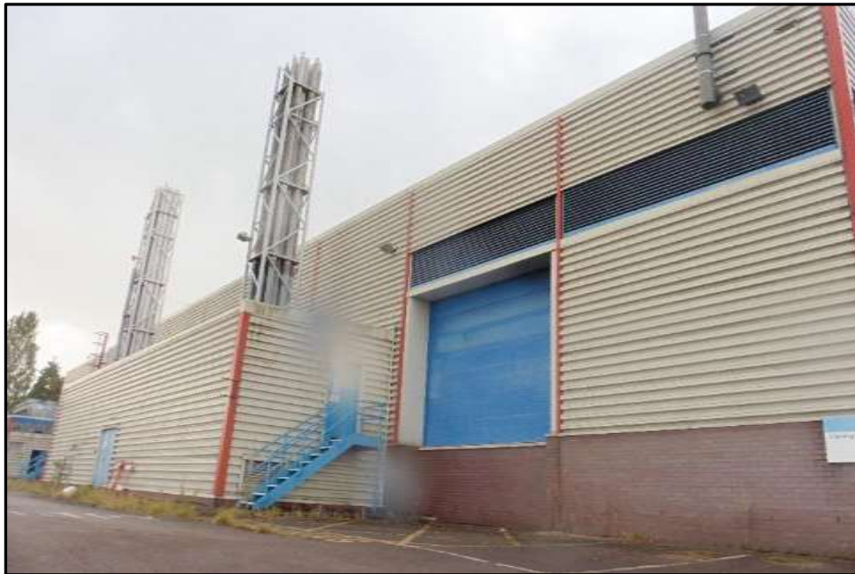
Plate 17c – Building 17, part east elevation
