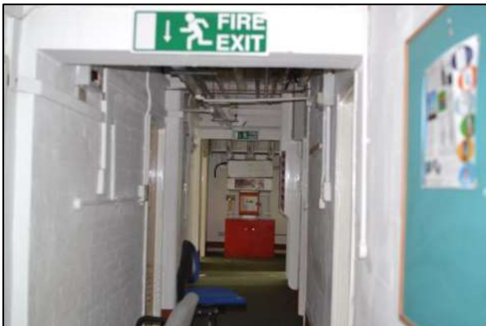
Plate E42 – E Block, secondary corridor of spur 7
