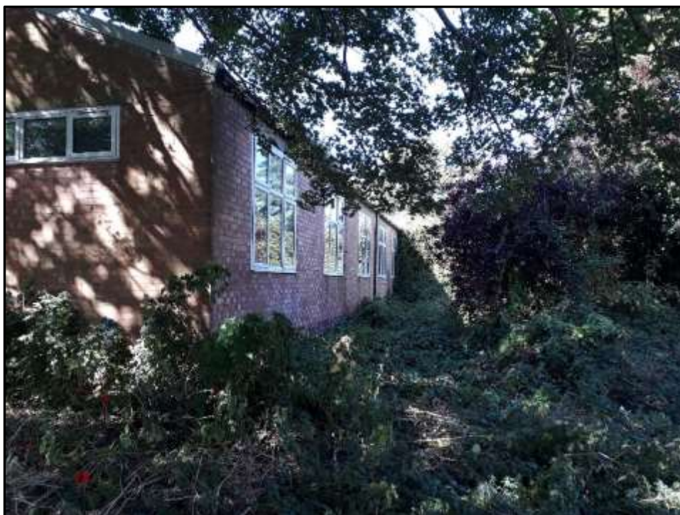
Plate L12 – Library building, north east elevation of the later south west range
