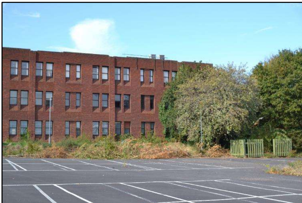
Plate 21b – Building 21, part east elevation (northern portion)
