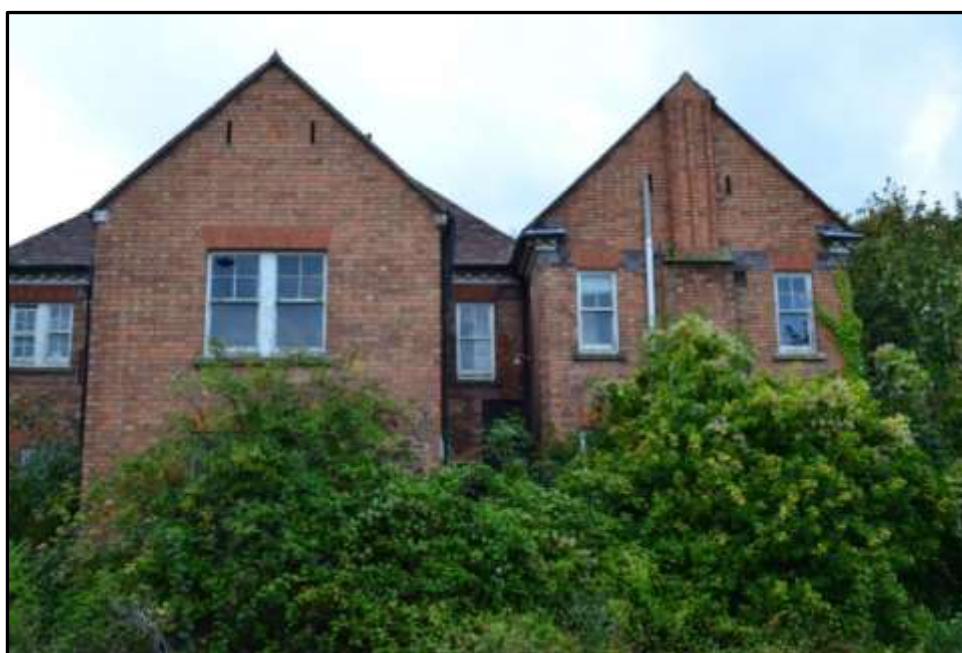
Plate S2 – Block S, advanced gable upper storeys to east elevation
