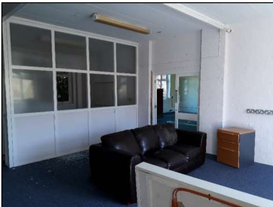
Plate L26 – Library building, south west range. Lobby area looking into the south east half of the range
