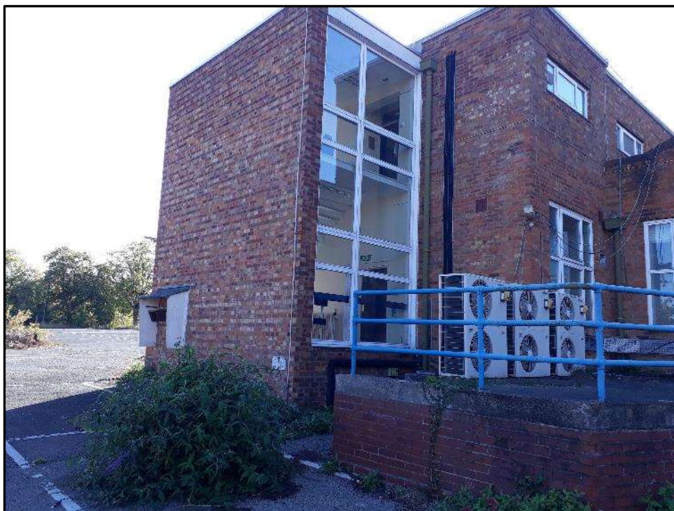
Plate H15 – H Building, part inner north elevation of south range and east elevation; change in brickwork to the first floor and the stair block relates to early phase of external alteration
