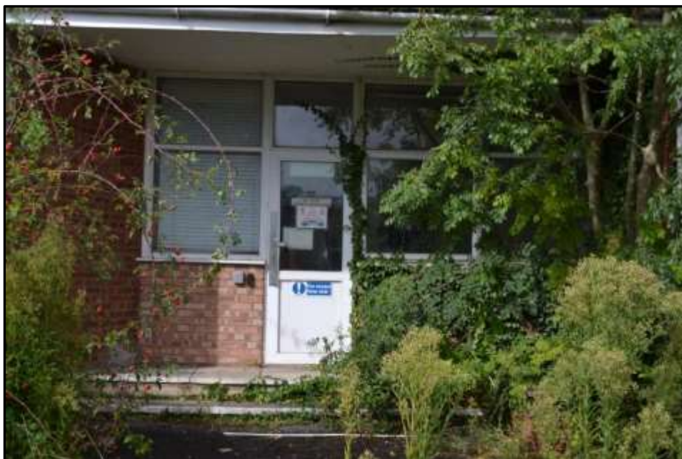
Plate 36l – Building 36, main entrance to the south east elevation
