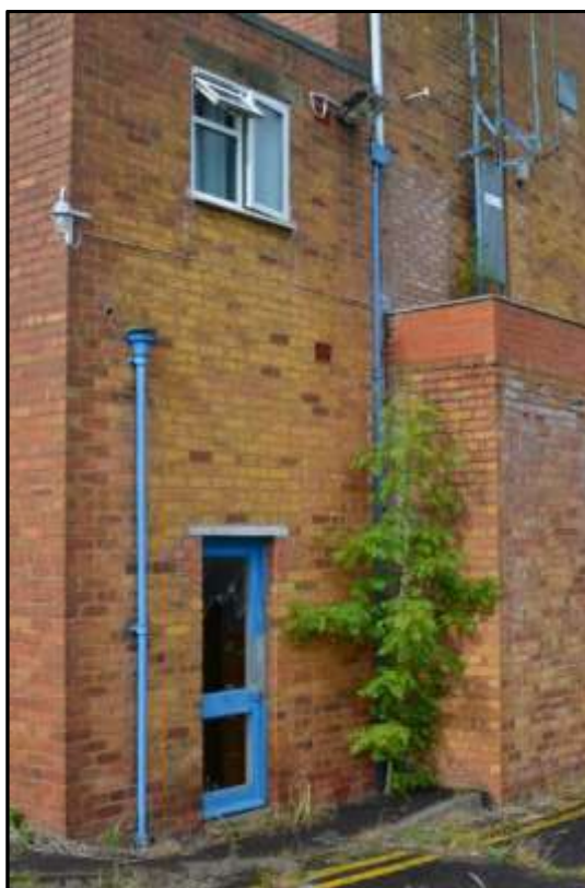
Plate 8d – Building 8, part east elevation of south range
