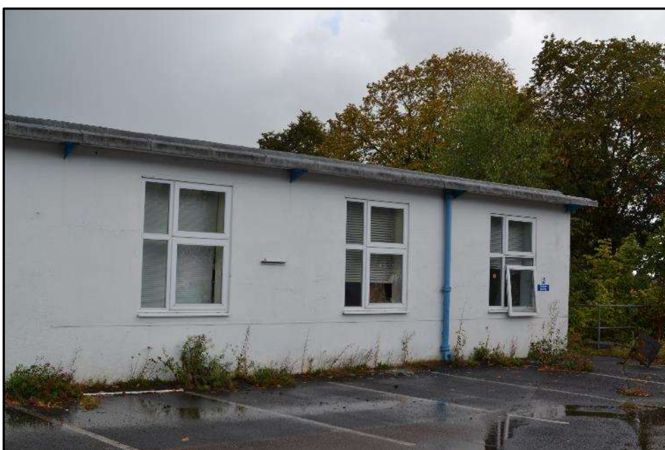
Plate E8 – E Block, southern three bays of west elevation of spur 9
