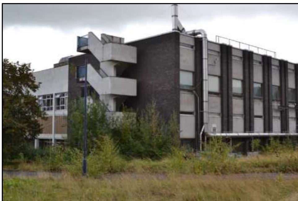
Plate 37c – Building 37, part west and north elevation
