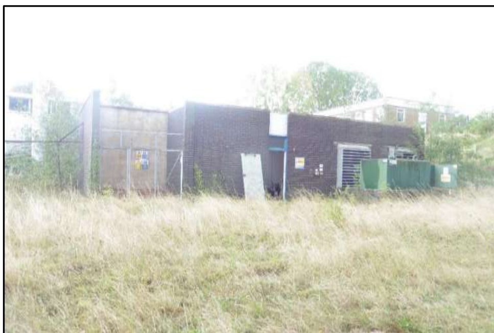
Plate 18a – Building 18, north elevation
