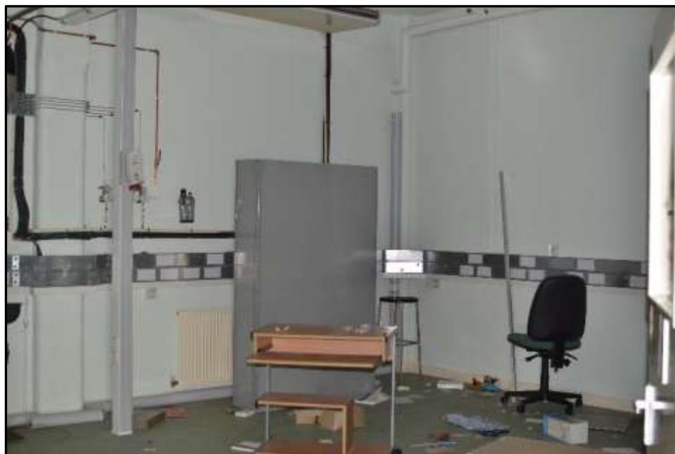
Plate E49 – E Block, spur 6, fixtures and fitting relating to most recent laboratory and research use
