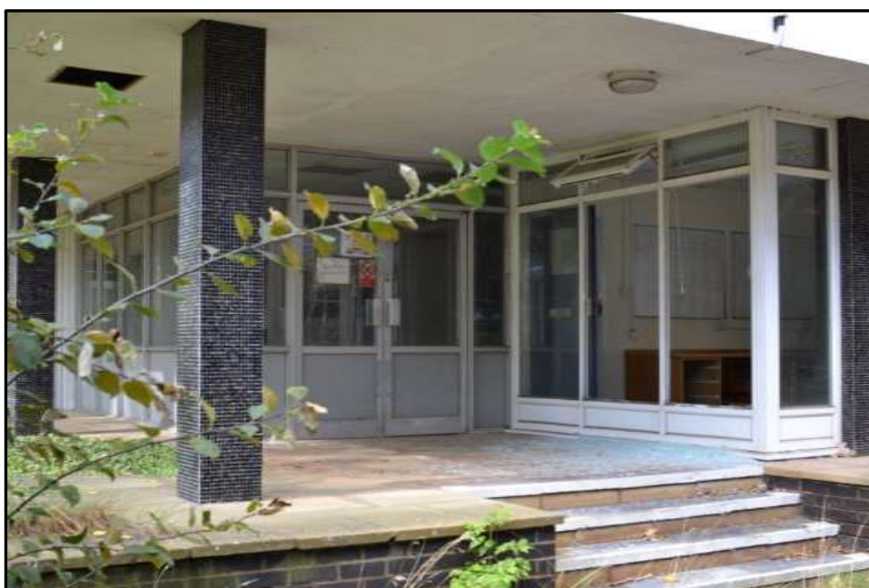
Plate 9c – Building 9, recessed entrance at the south east corner
