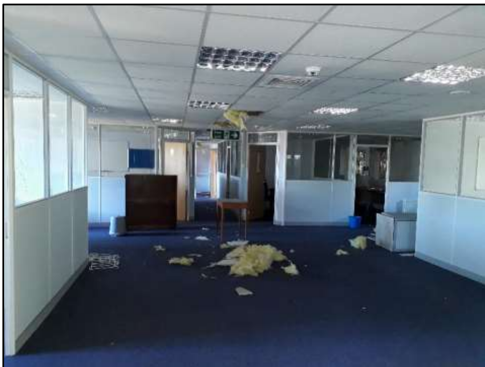
Plate L17 – Library building, internal arrangement of the south east half of the original range. All partitions and fixtures are modern
