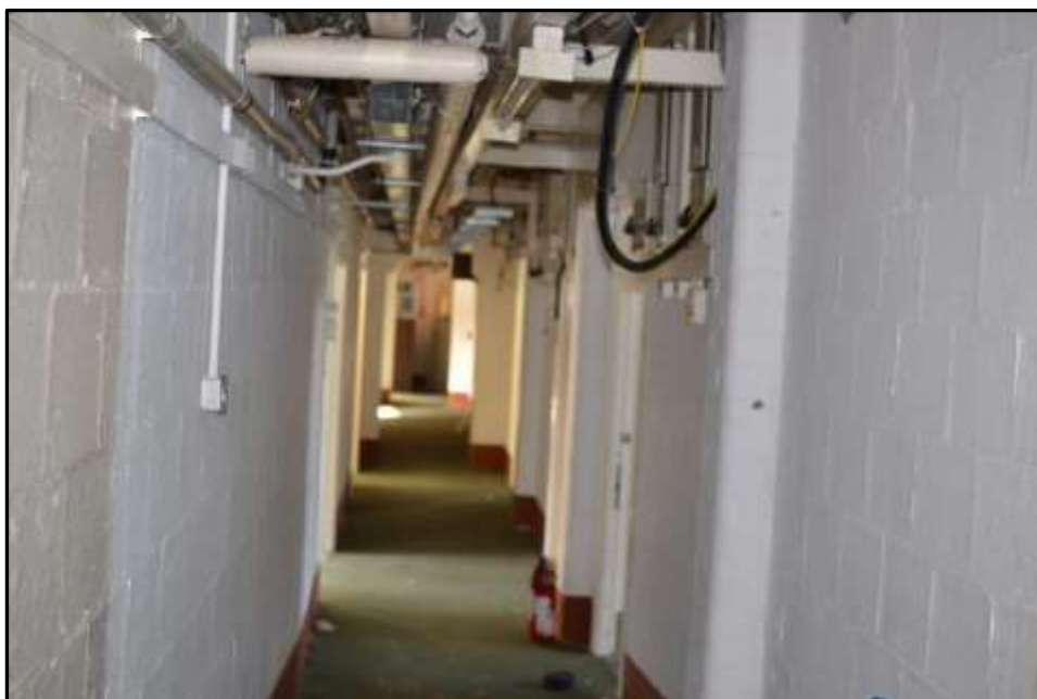
Plate E34 – E Block, secondary corridor to 9 with rounded edge of brick columns and brick tile internal dividing walls typical of each original block
