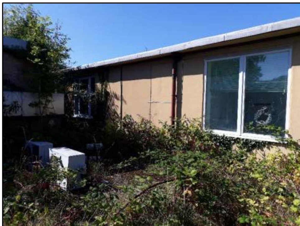
Plate A16 – A Block, part south east elevation of spur 6
