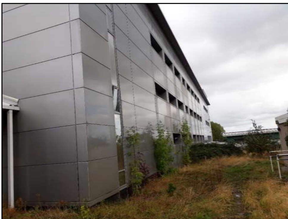
Plate 3e – Building 3, south elevation of main range
