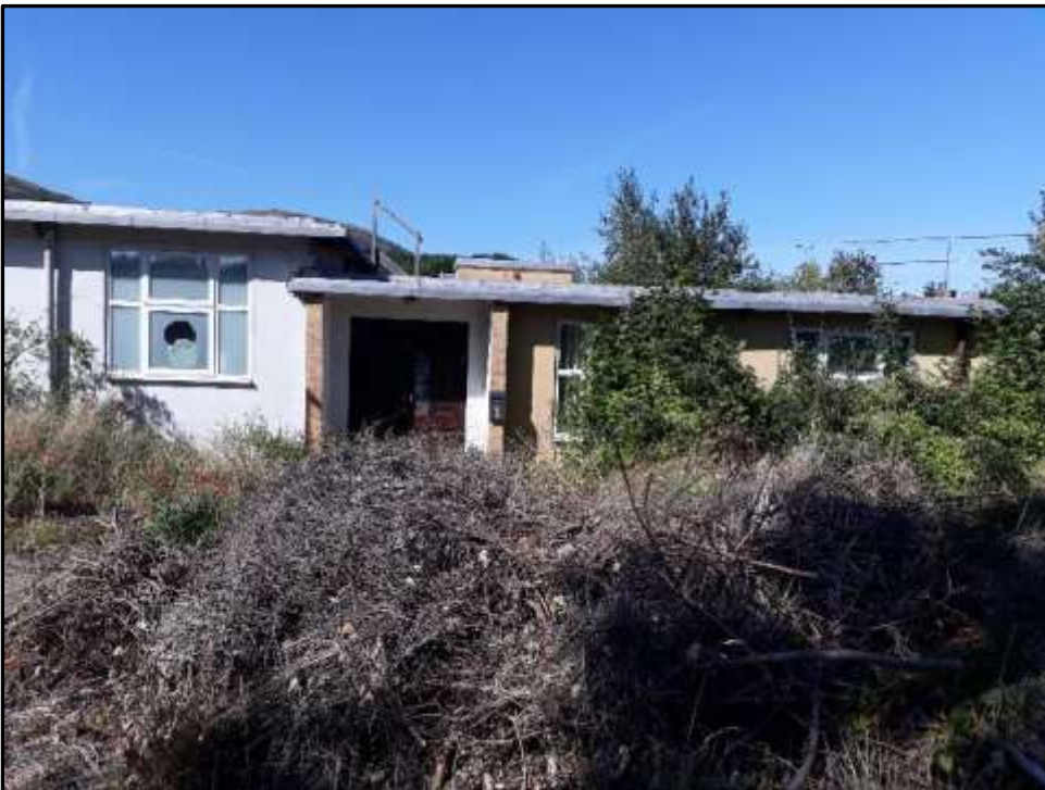
Plate A12 – A Block, secondary entrance at central junction between spurs 7 (left) and 8 (right)
