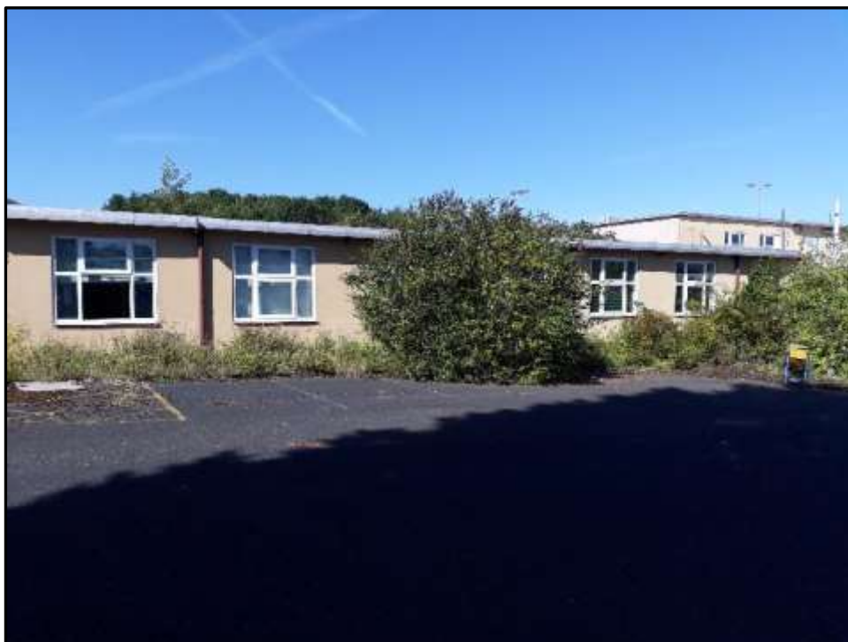
Plate A1 – A Block, part south east elevation of spur 3
