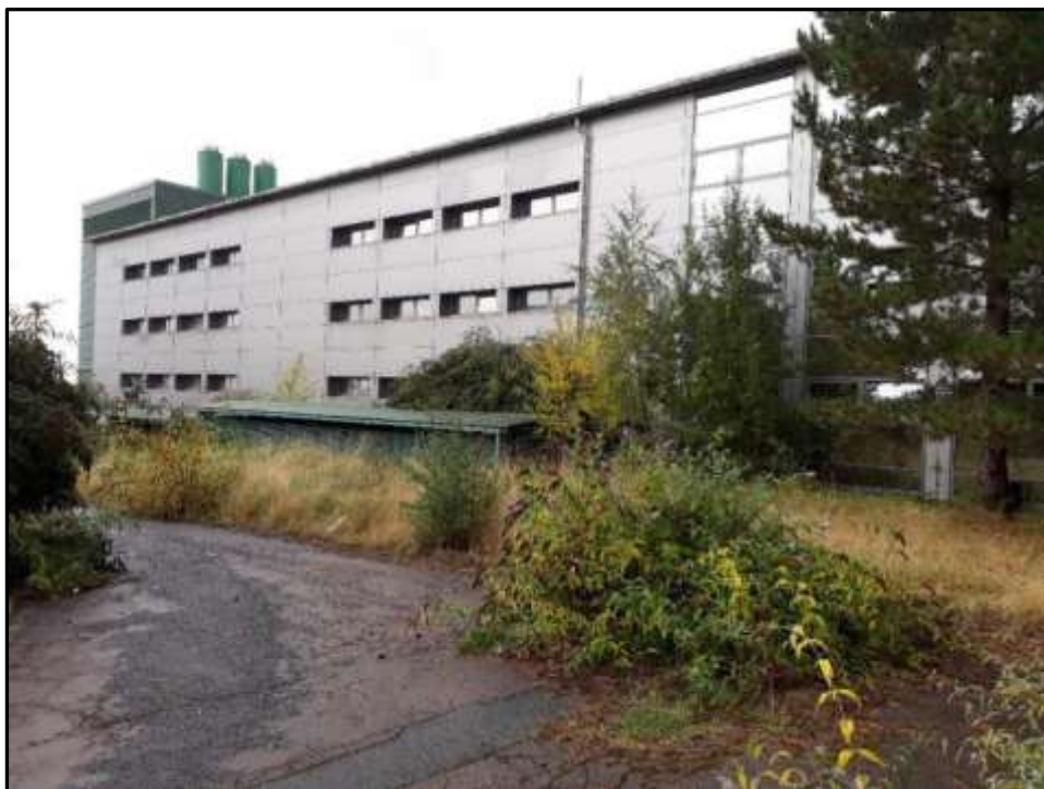
Plate 3g – Building 3, north elevation
