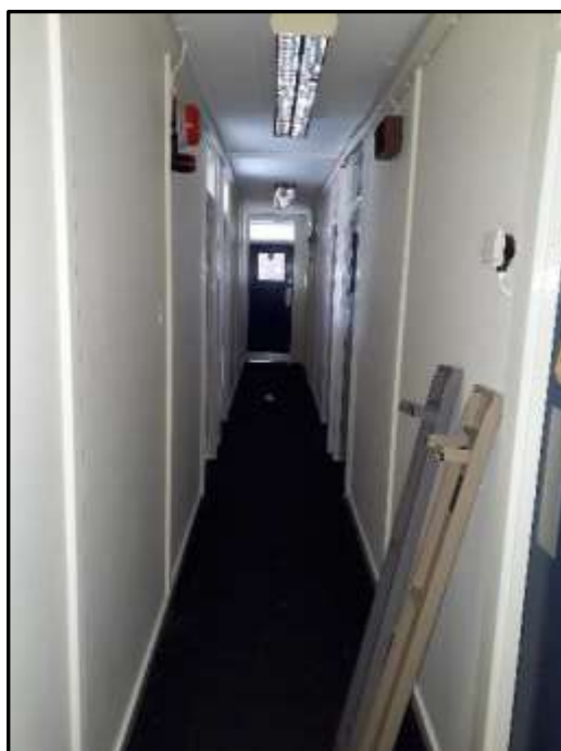
Plate H33 – H Building, ground floor corridor aligned east to west through the north range (former radar room to right)
