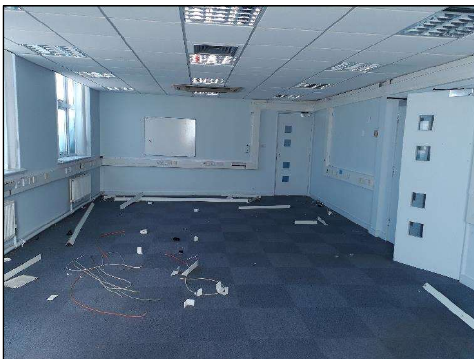
Plate A53 – A Block, modern interventions observed within spur 3
