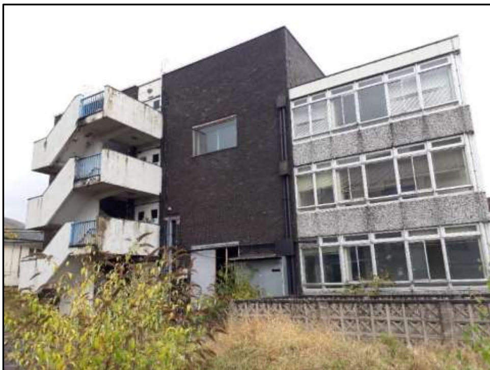
Plate 37h – Building 37, south elevation with external concrete stair that matches north elevation
