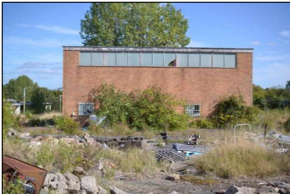
Plate 28c – Building 28, south west elevation
