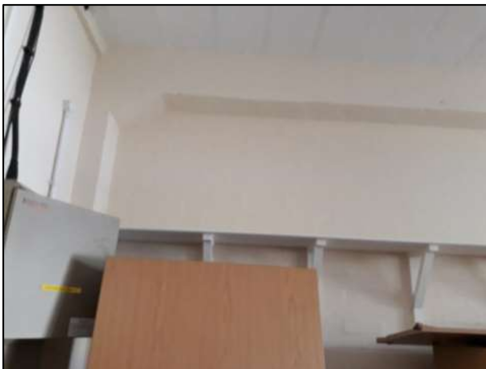
Plate E38 – E Block, remains of original construction to the interior
