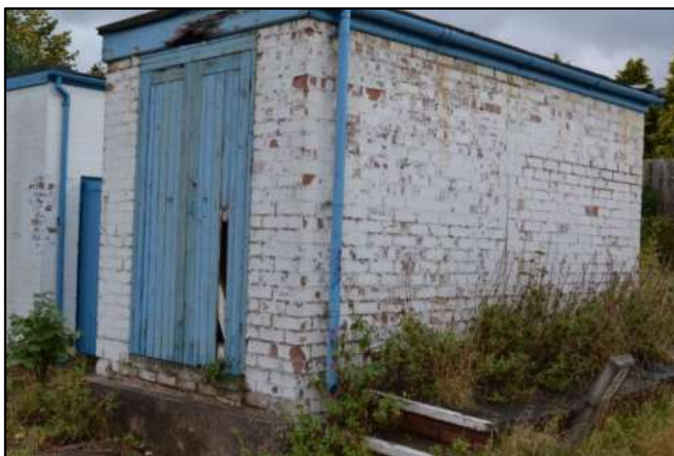
Plate 12a – Building 12, east and north elevations
