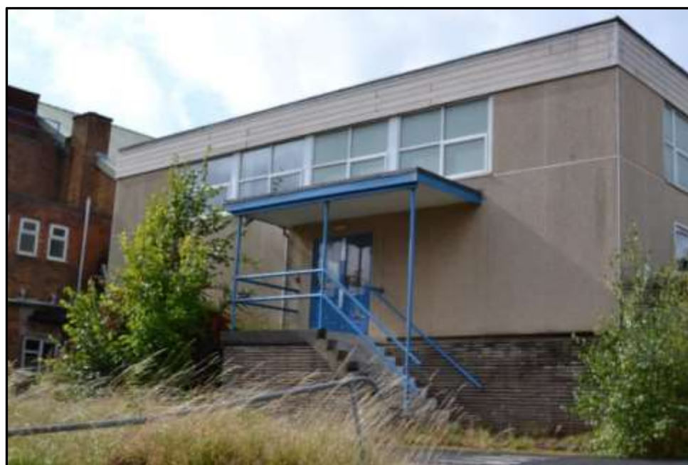
Plate 8a – Building 8, east elevation of north range
