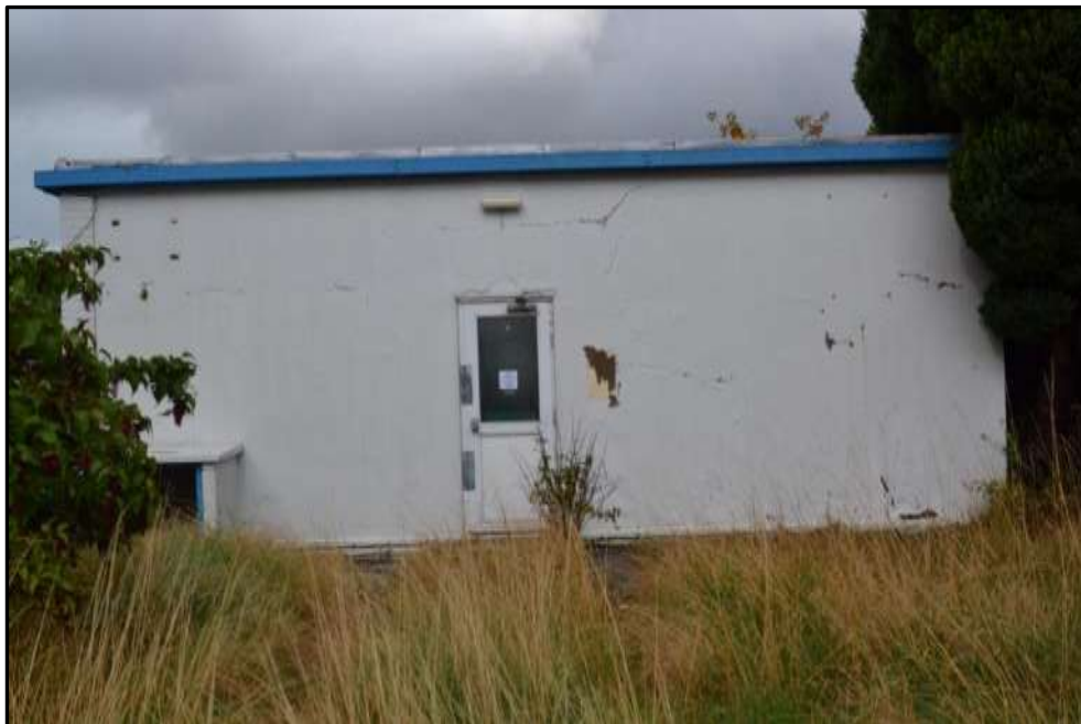
Plate 1d – Building 1, part south elevation
