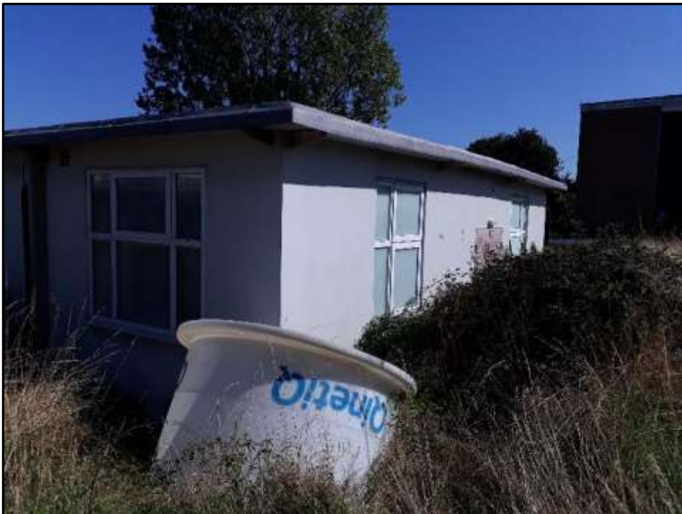
Plate A10 – A Block, south west end elevation of spur 7
