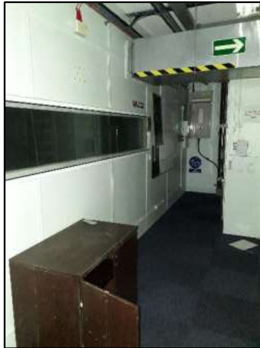
Plate H53 – H Building, first-floor. Sound proof conference pod to the east wall of the former bunker
