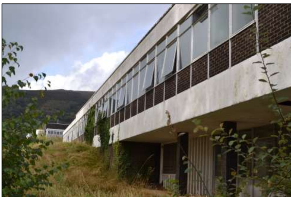
Plate 9d – Building 9, part south elevation
