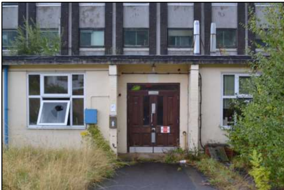
Plate KF6 – West elevation, main entrance
