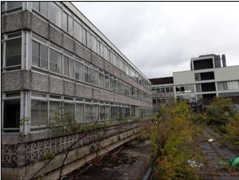
Plate 37g – Building 37, part east and south elevations
