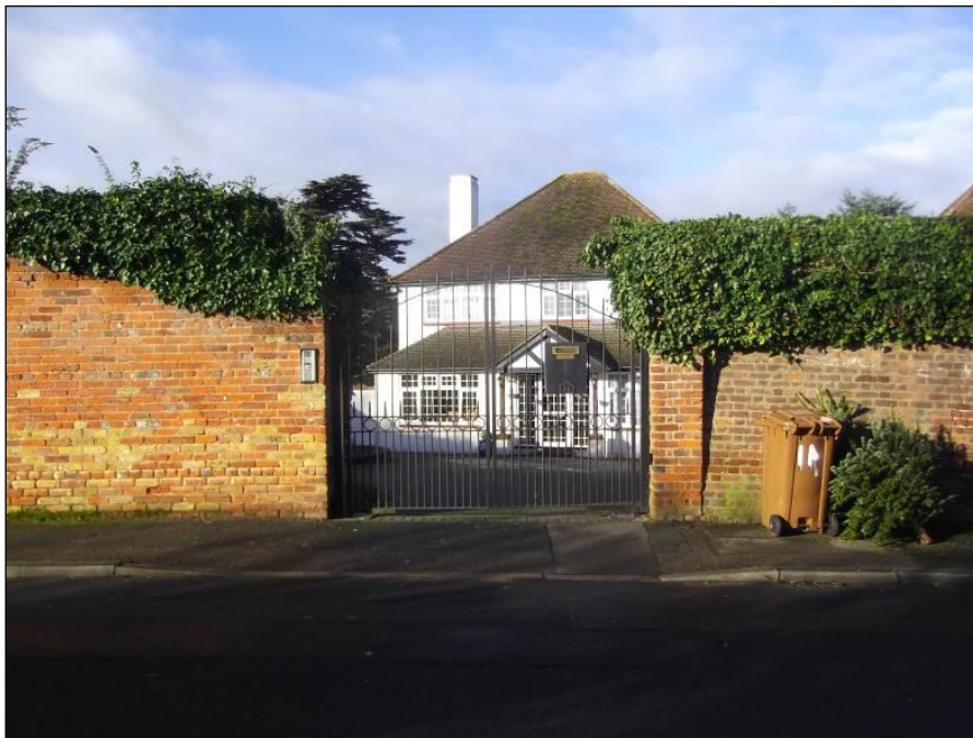
Plate 6: Change of construction in wall between Nos. 14 and 16 (2016 photograph)
