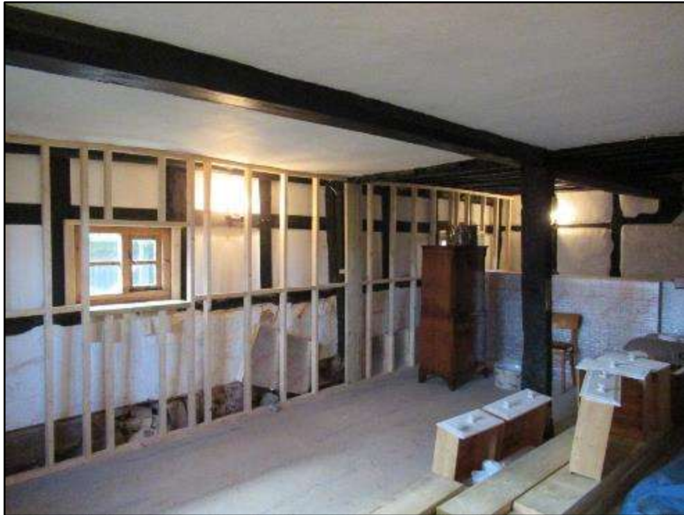
Plate N – Ground floor three-storey south range
