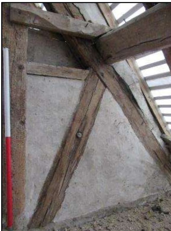
Plate MF149– Wattle and daub infill panels and angled strut to the central roof truss
