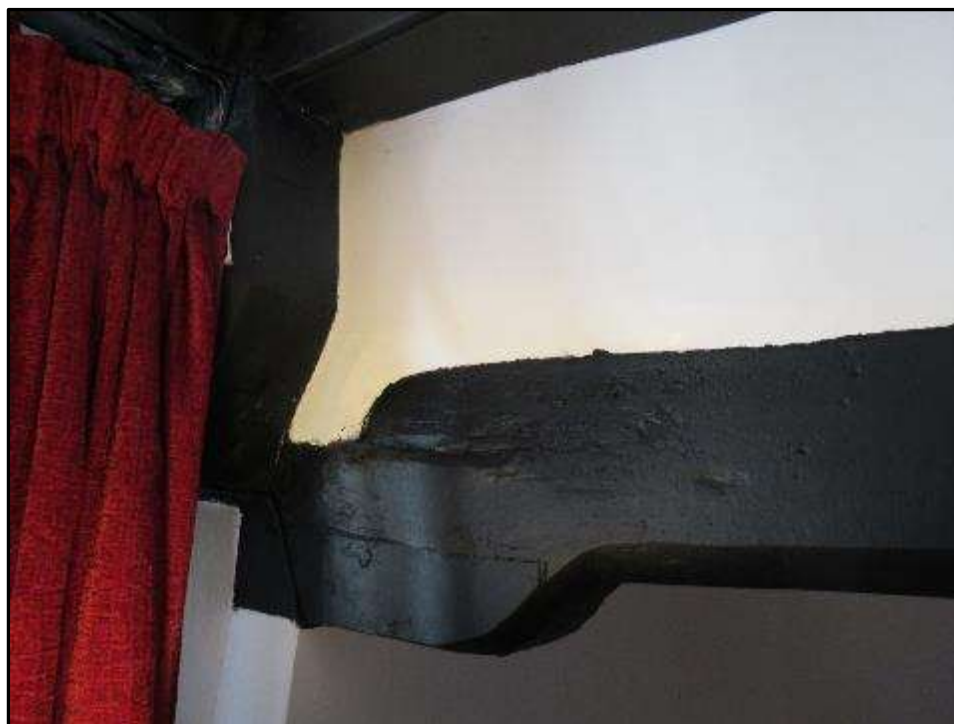
Plate MF42 – Moulded timbers bressumer to inglenook fireplace in entrance hall
