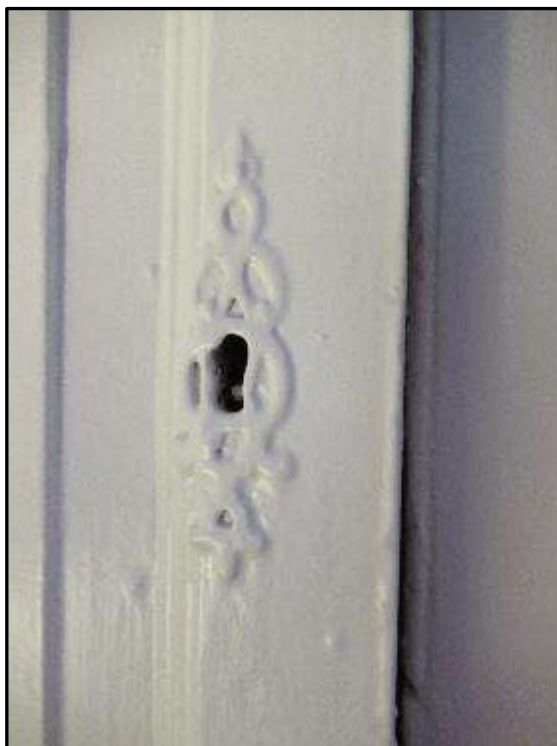
Plate MF59 – Key plate to built-in cupboard
