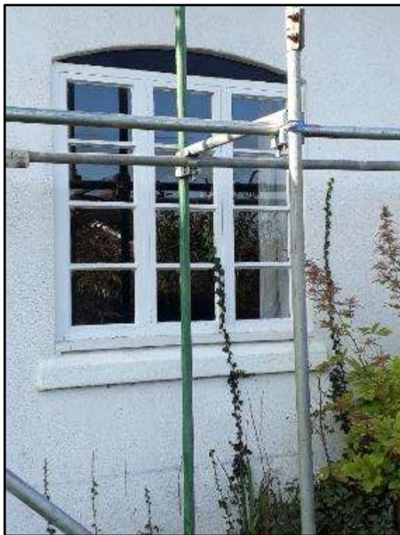
Plate MF10 – East elevation, ground floor window
