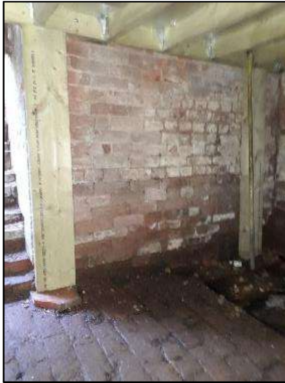
Plate MF107 – Brick setts to the cellar wall
