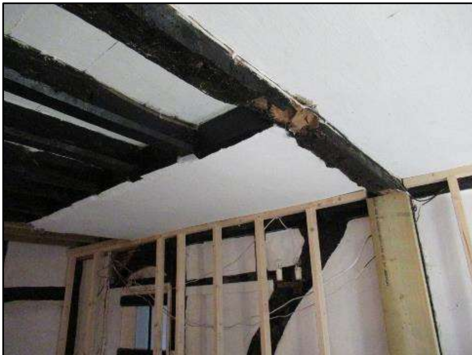
Plate MF100 – Arrangement of ceiling timbers to the north west corner of the g/f room of the south range indicative of possible former subdivision
