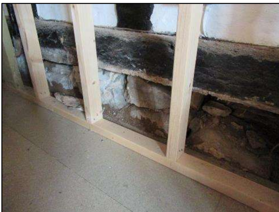
Plate MF101 – Sole plate and stone plinth to the north wall of the g/f room of the south range
