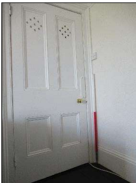
Plate MF52 – Four panel door to main sitting room (interior view)
