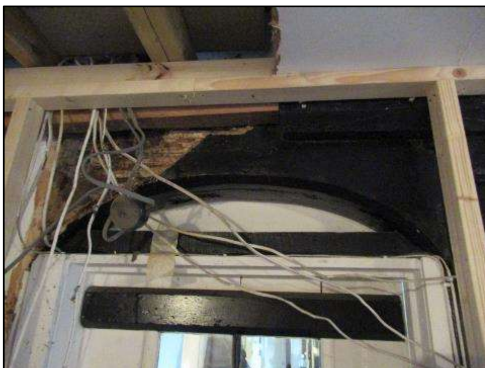
Plate MF88– round arch head to door opening between the main g/f passageway and the g/f of the three-storey south range
