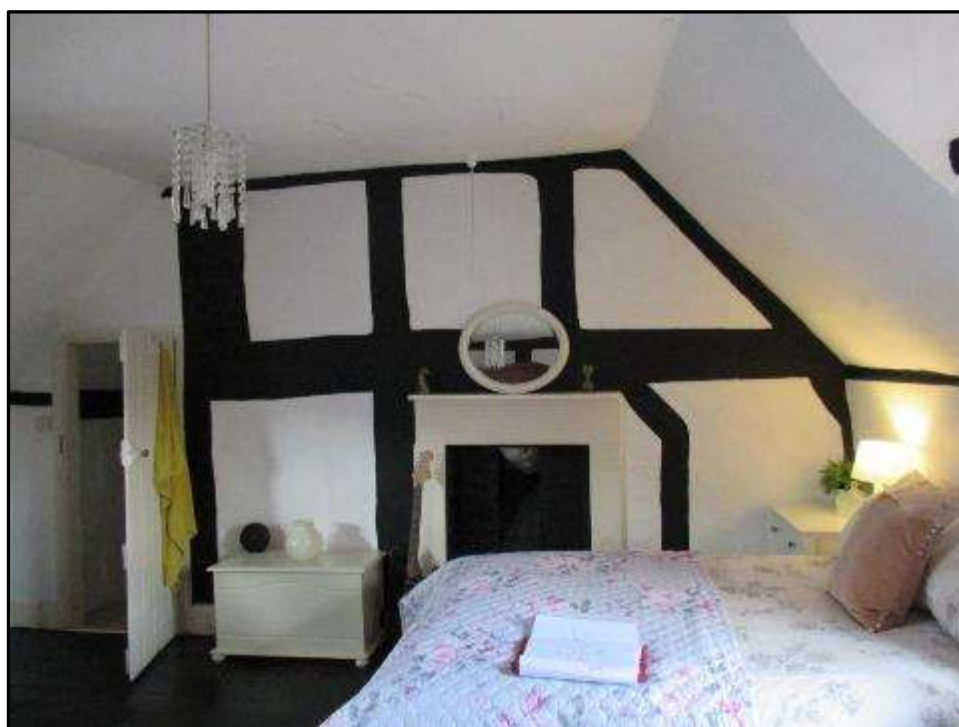
Plate MF127 – Timber frame construction to the north internal wall of the bedroom to the south bay of the central range
