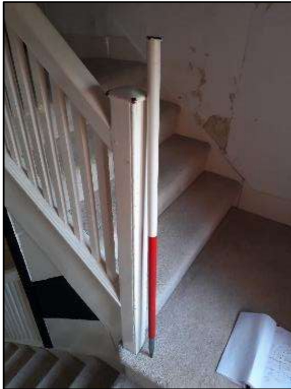
Plate MF109 – Half landing area of the main staircase
