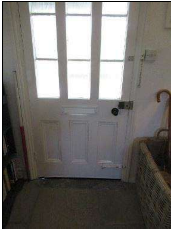
Plate MF45– Main entrance door (internal view)
