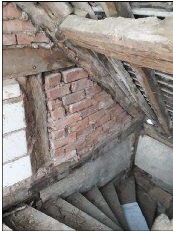
Plate MF143 – Brick infill panel to the west gable end elevation of the south range
