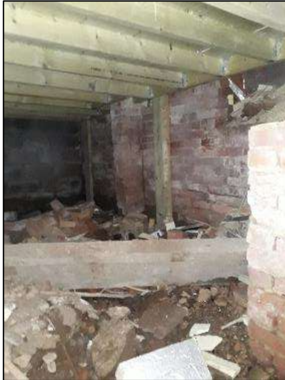
Plate MF105– South wall of cellar area below the south range
