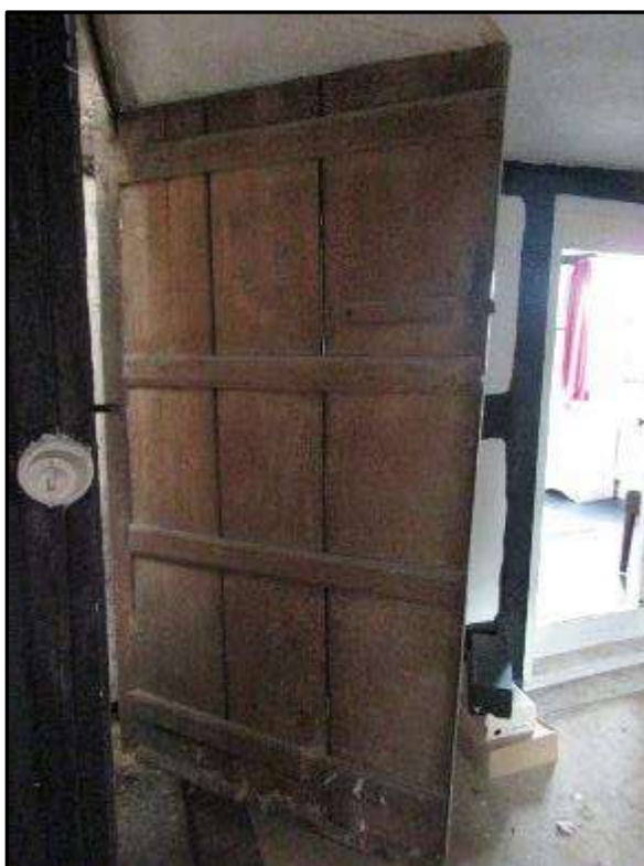
Plate MF133– 17 th Century oak boarded door to the staircase to the second floor of the south range
