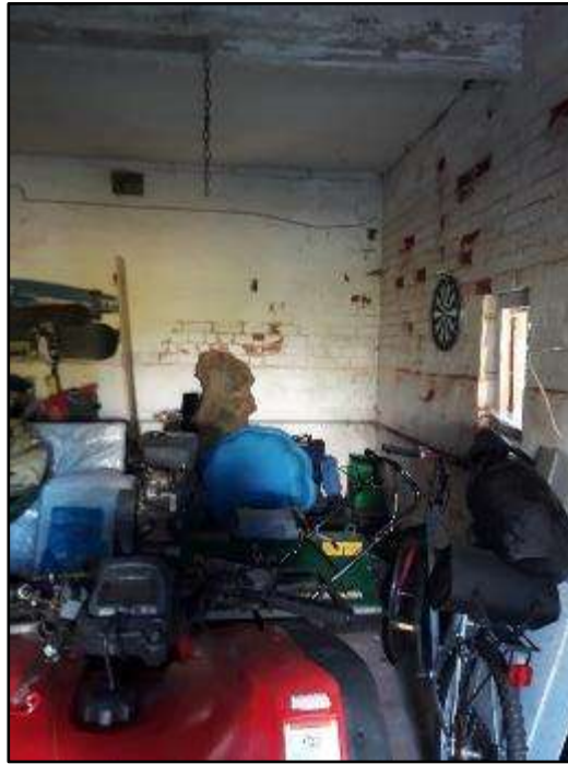
Plate M – Former dairy with west addition of south range
