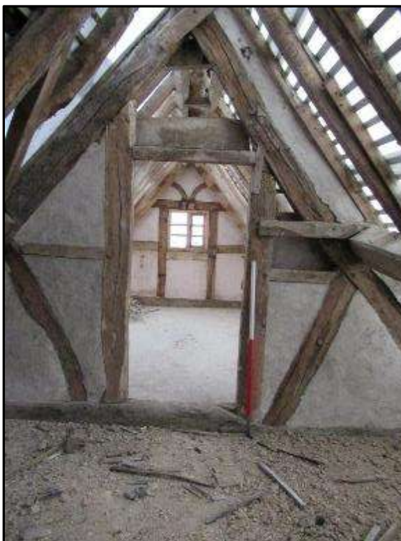
Plate MF147 – Internal partition wall and opening within the central roof truss
