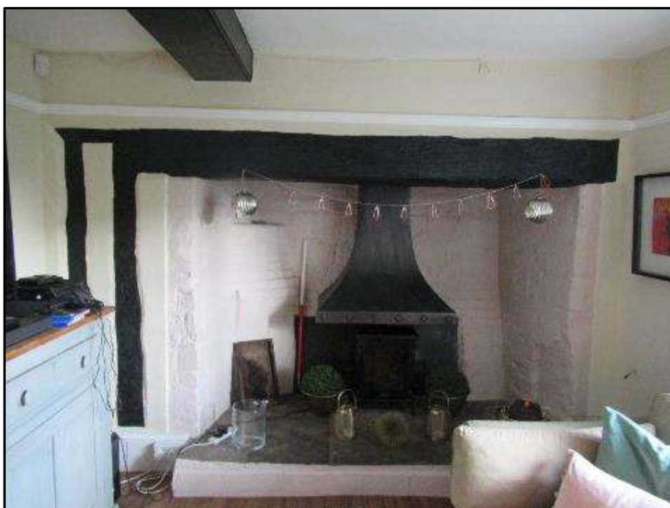
Plate MF68 – Inglenook fireplace with bressumer beam and stud posts within small sitting to south bay of the central range
