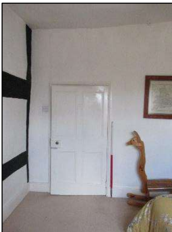
Plate MF125 – Diminutive four panel door to first floor bedroom within central range
