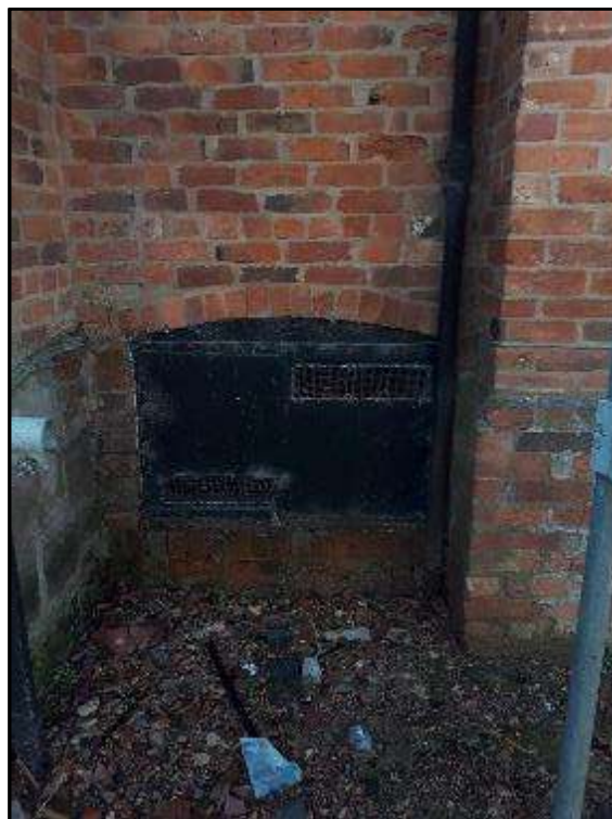
Plate MF40 – Cellar window to the north elevation (west addition)
