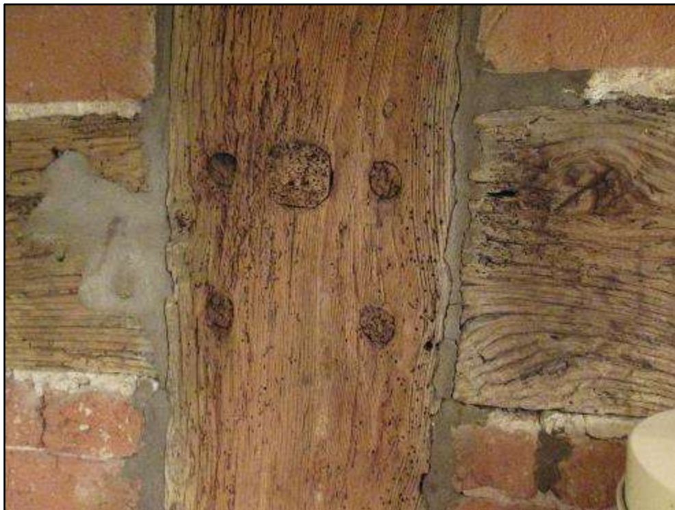
Plate L – Section of timber frame to west elevation of south exposed to extant kitchen
