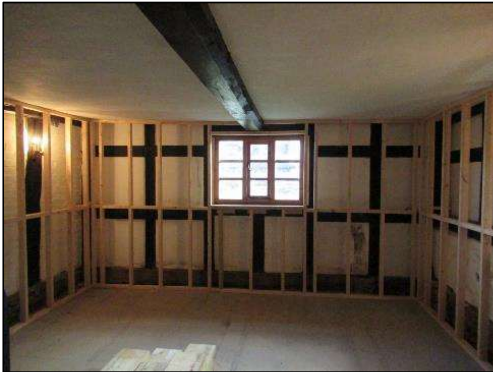
Plate MF91 – Renewed timber frame construction to the east wall of the g/f room of the south range
