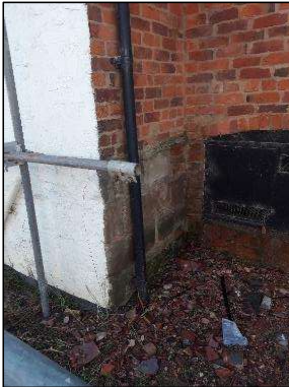
Plate MF39 – Stone plinth to the north elevation
