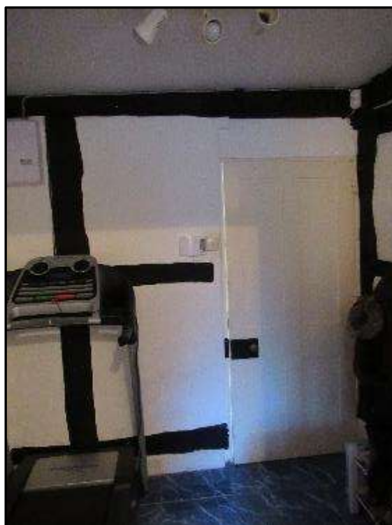
Plate MF56 – Timber frame to south wall of g/f bathroom
