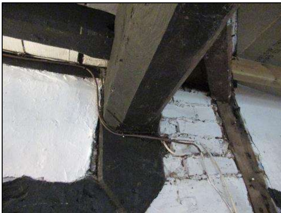
Plate MF98 – Chamfered bridging beam with stops aligned east to west through the g/f room of the south range (west end)
