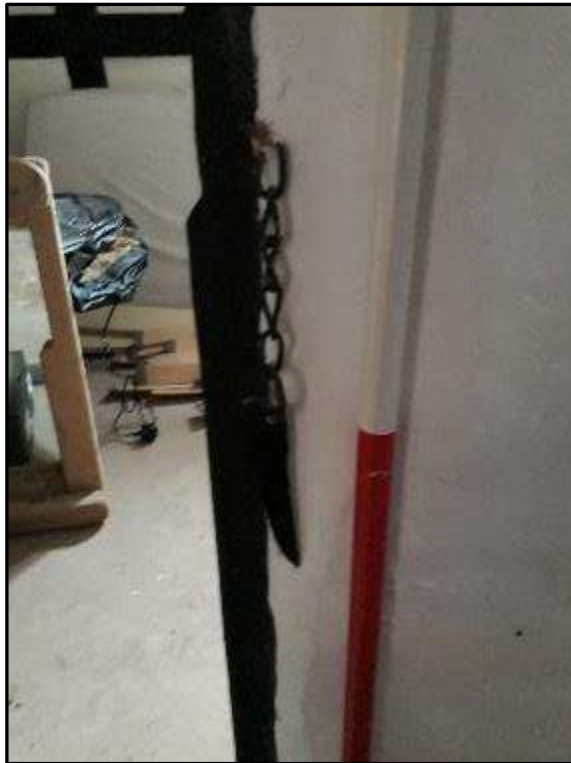
Plate MF137 – Remains of metal door catch/lock to opening frame
