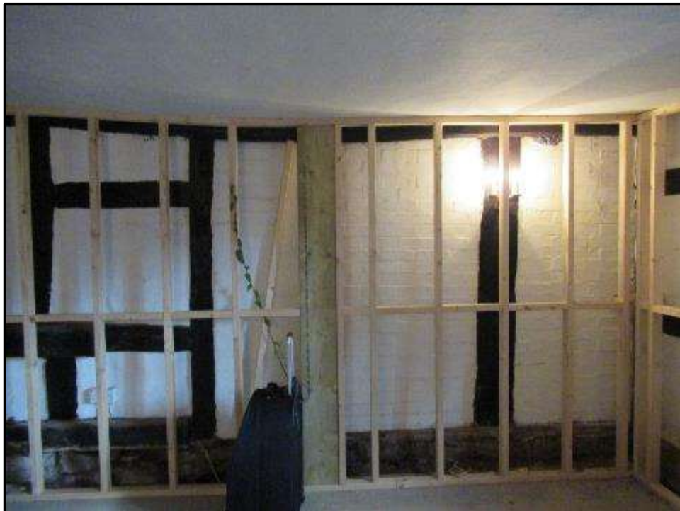
Plate MF90 – Change in timber frame to the north wall of the south range; the change in framing indicative of where the south range projects forward (right) of the central range (left)
