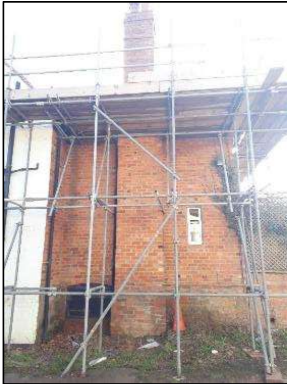
Plate MF37 – North elevation of the north range (west addition)
