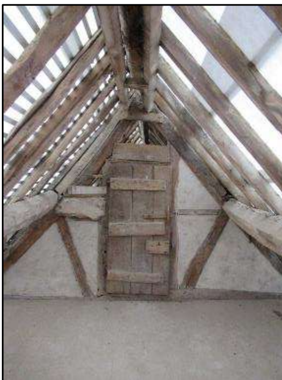
Plate MF151 – Interior view of the 17 th Century oak boarded door to the second floor of the south range looking west
