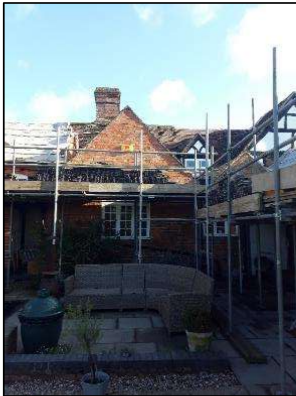
Plate MF25 – West elevation, single storey addition
