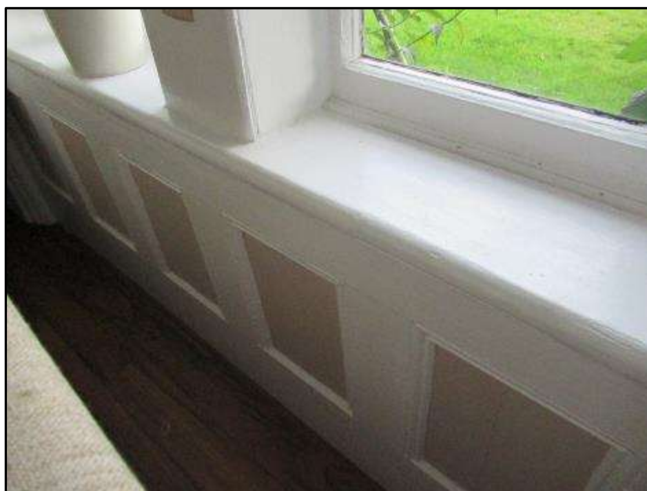
Plate MF71 – Fielded panels to base of east window in small sitting room
