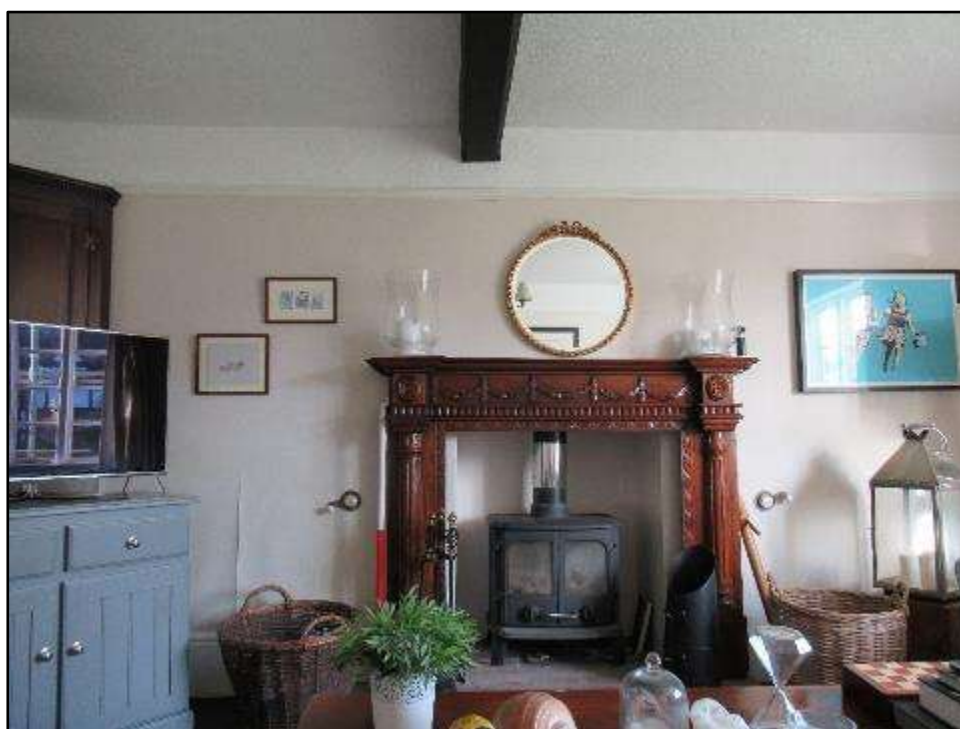
Plate MF48 – Renewed fireplace to main sitting room, note beam and picture rail
