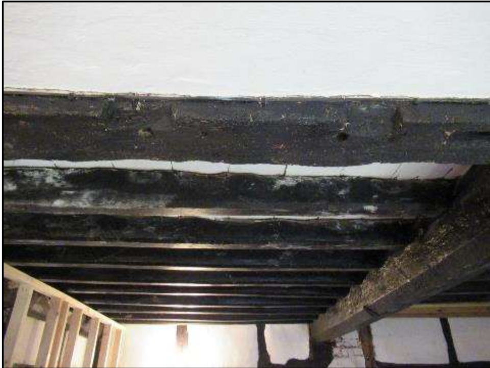
Plate MF99 – Chamfered joists to g/f room of south range; mortice to the joist to the top of the image indicates possible former partition
