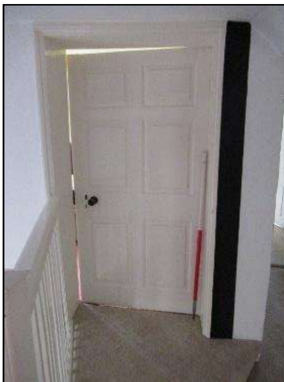
Plate MF114 – Six panel to the bedroom in the west addition of the north range
