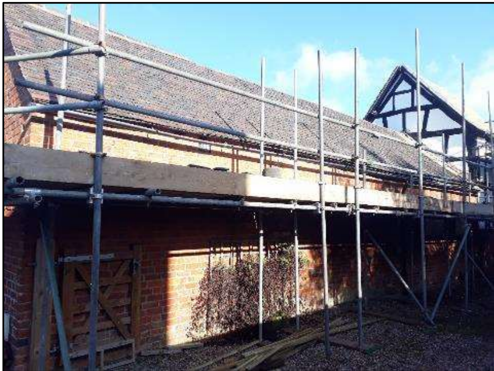
Plate MF14 – Single storey addition to west of the south range
