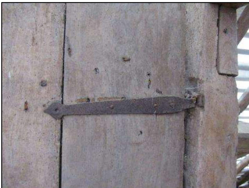
Plate MF152 – Spear head strap hinge to second floor door
