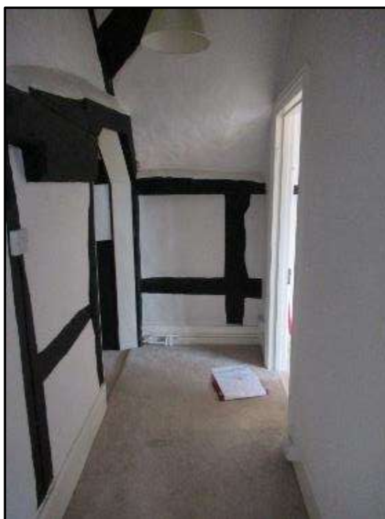
Plate MF119 – Passageway through the north range; timber frame of the north wall of the central range to right and remains of timber frame to the west wall in centre of the image
