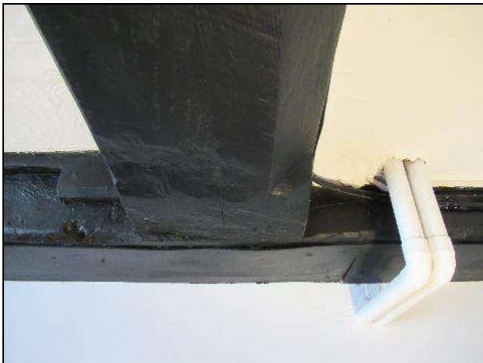
Plate MF46 – Chamfered bridging beam with stops to entrance hall
