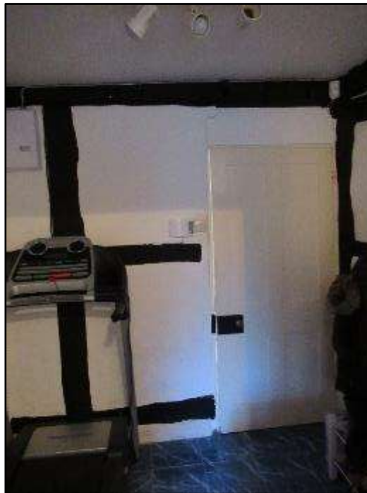
Plate H – Timber frame to downstairs bathroom
