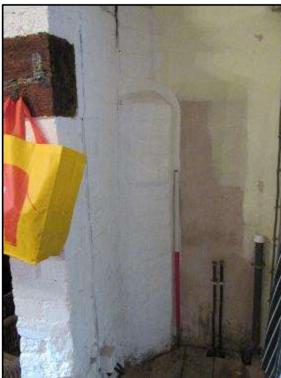
Plate MF81 – Shaped brickwork edge to inserted fireplace in kitchen
