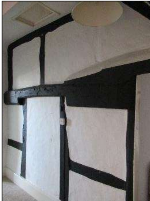
Plate P – Timber frame to first floor cross wall of central range
