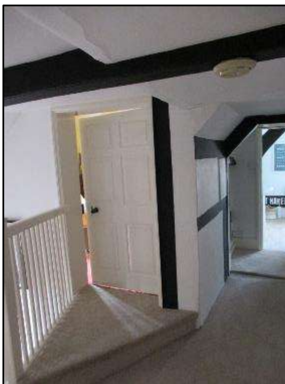
Plate MF111 – Landing area looking north towards the north range, change in floor level often indicative of different phases of development
