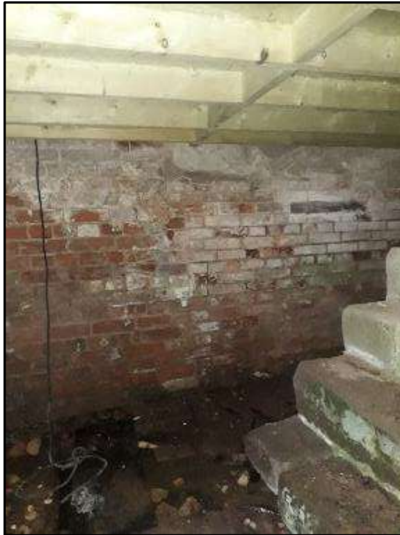
Plate MF103 – West wall of the cellar area below the south range; renewed joists indicative of the renewed and lowered floor level of the g/f room of the south range
