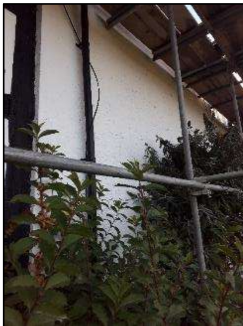
Plate MF5 – East elevation of central range, step in render suggests timber frame may be retained beneath
