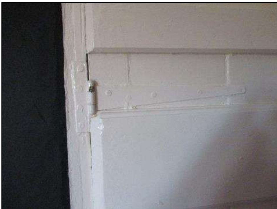
Plate MF131 – Metal strap hinge to the plank and braced door to the south wall of the central range giving access to the first floor of the south range
