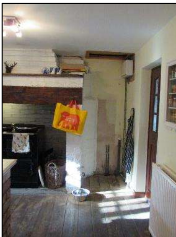
Plate MF79 – View west through kitchen towards brick partition wall to externally accessed storerooms
