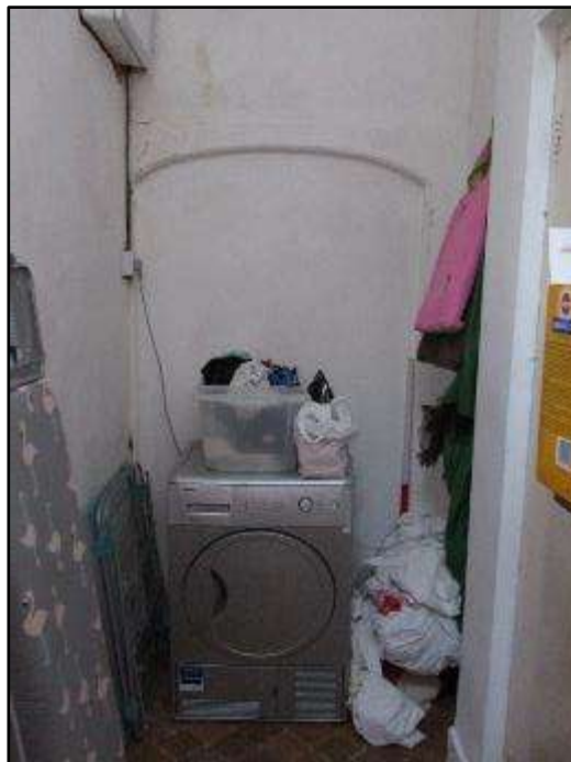
Plate K – Infilled round arch opening visible to west elevation
