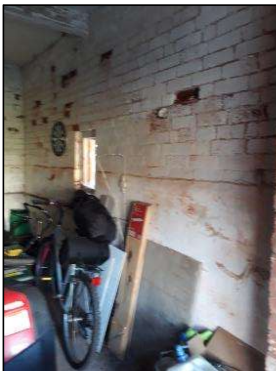
Plate MF87 – Tanking and painted brickwork interior to former dairy
