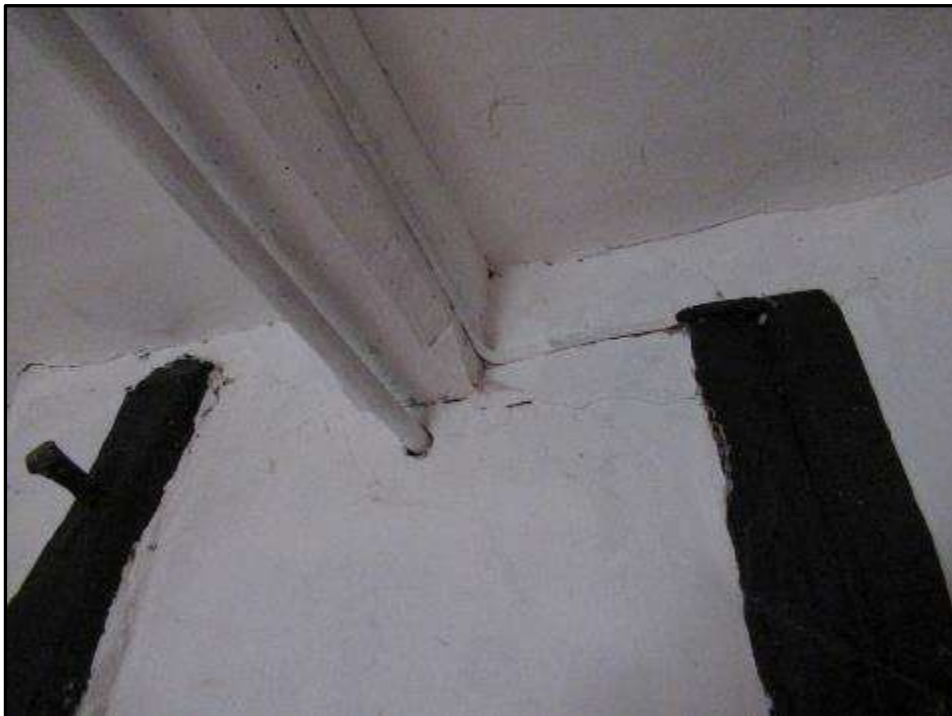
Plate MF140 – Chamfered joists with stops to small first floor room to the south range
