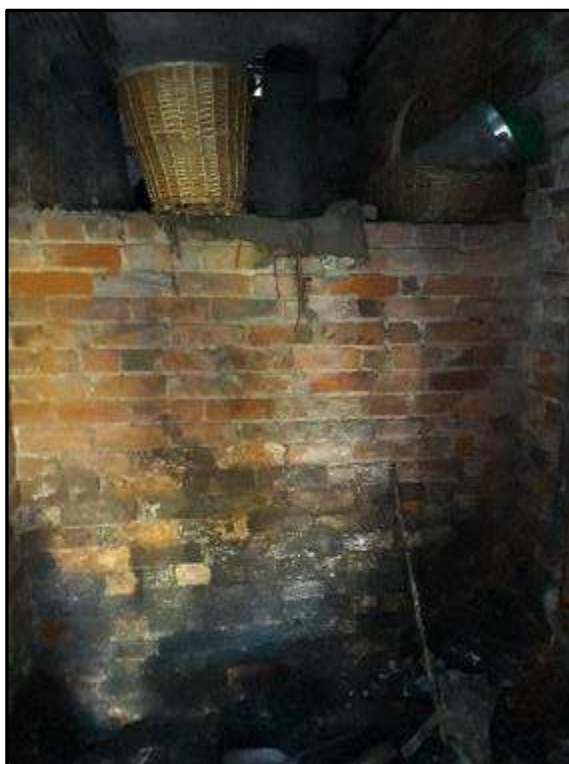
Plate MF83 – Brickwork of the small coal store within the single storey west wing of the south range
