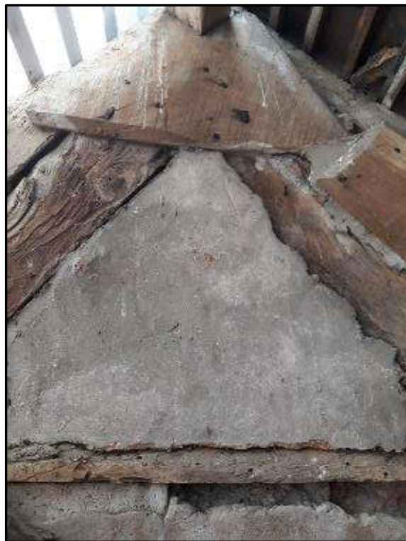
Plate MF156 – Wattle and daub infill panel to the apex of the west elevation of the south range
