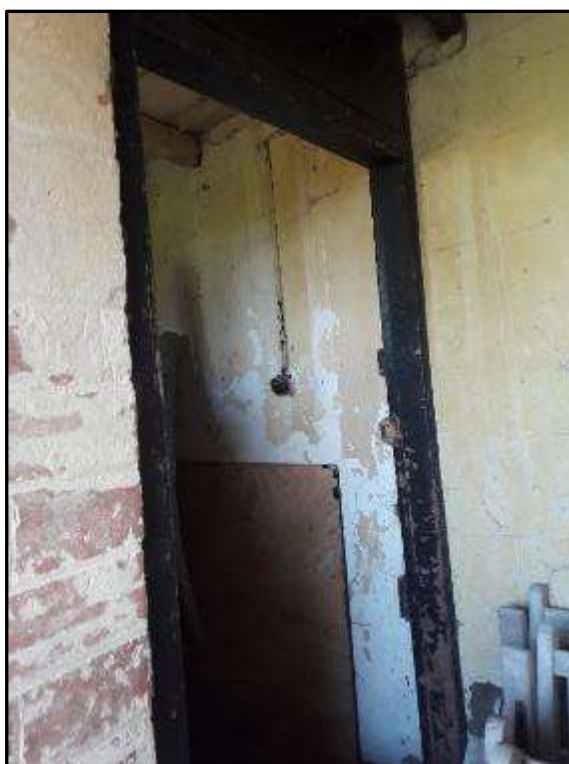
Plate MF30 – Store/outhouse to single storey rear porch (west elevation)
