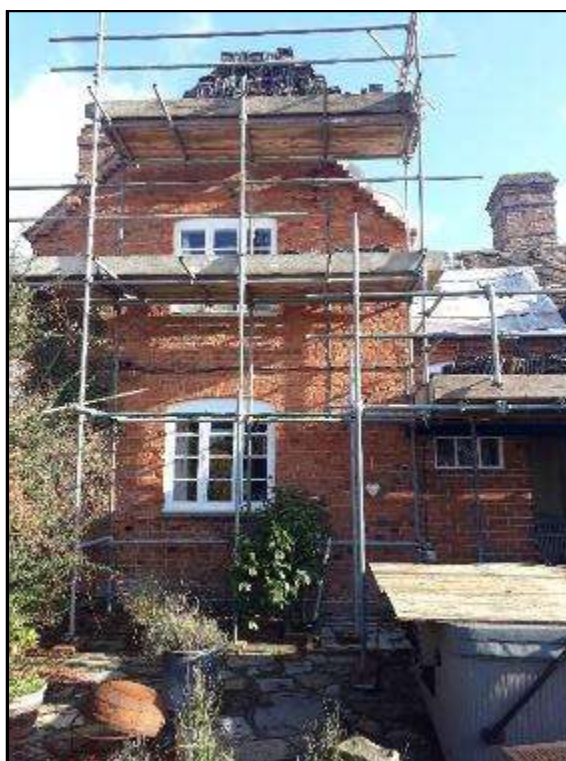
Plate MF32 – West gable end of west addition of north range
