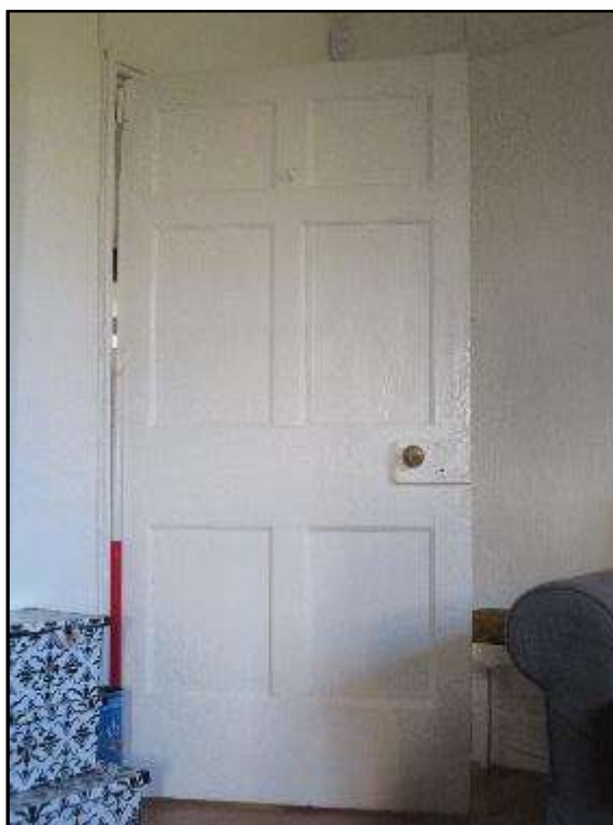
Plate MF60 – Six panel door to sitting room in west addition (north rage)
