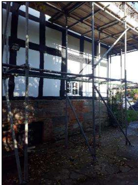
Plate MF12 – South elevation of south range show stone and brickwork plinth and renewed timber frame to ground floor
