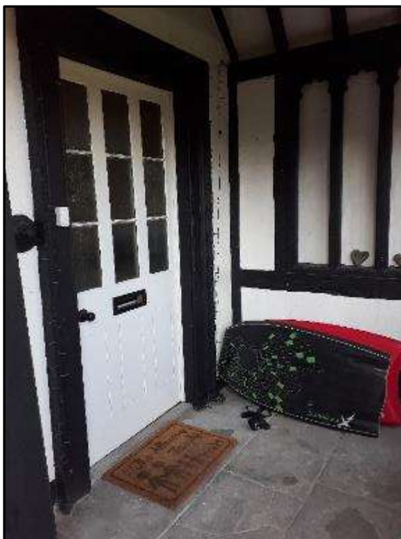
Plate MF7 – East elevation, main entrance door within gabled porch
