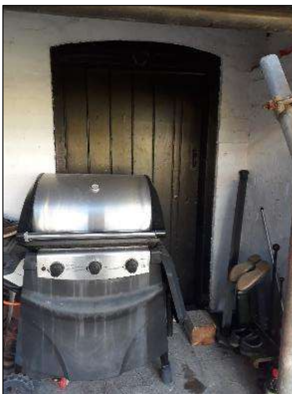
Plate MF21 – North elevation of single storey addition (overlooking rear garden) with timber boarded door with segmental arch opening to an external store/former outhouse
