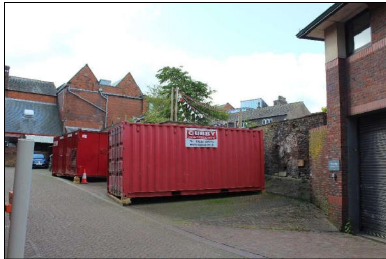
Plate 7: Location view of boundary wall, facing south
