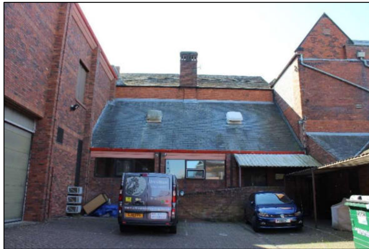
Plate 5: Kitchen area from west service yard/goods yard, facing south-east
