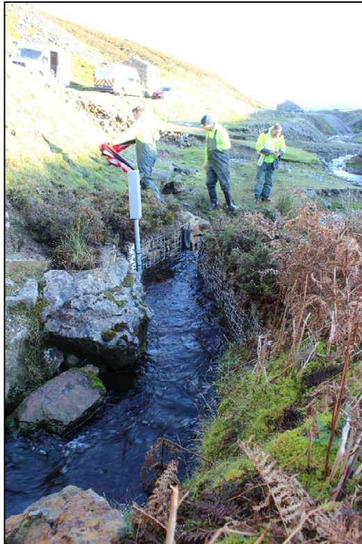
Plate 1: Completed structures, channel and monitoring structure facing south
