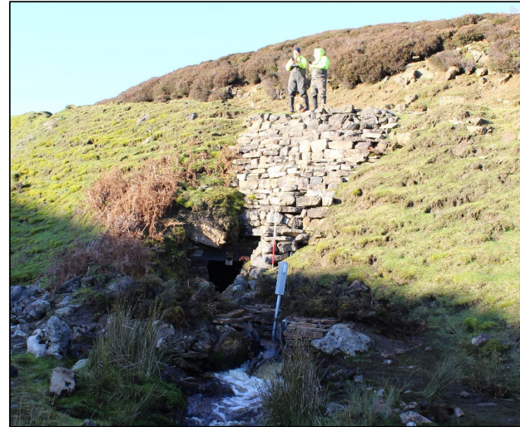
Plate 6: View of Hard Level Adit from south-south-east
