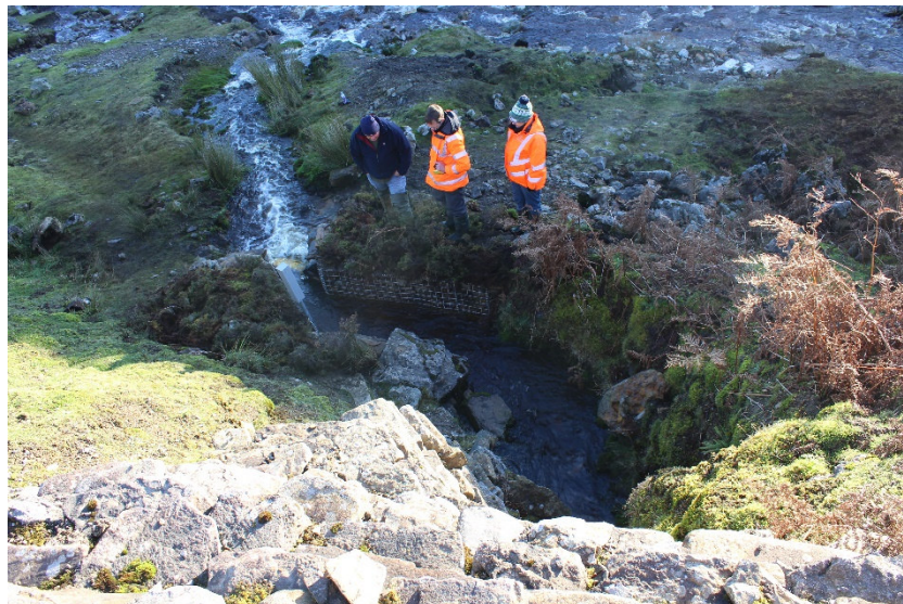
Plate 2: Completed structures, channel and monitoring structure facing north
