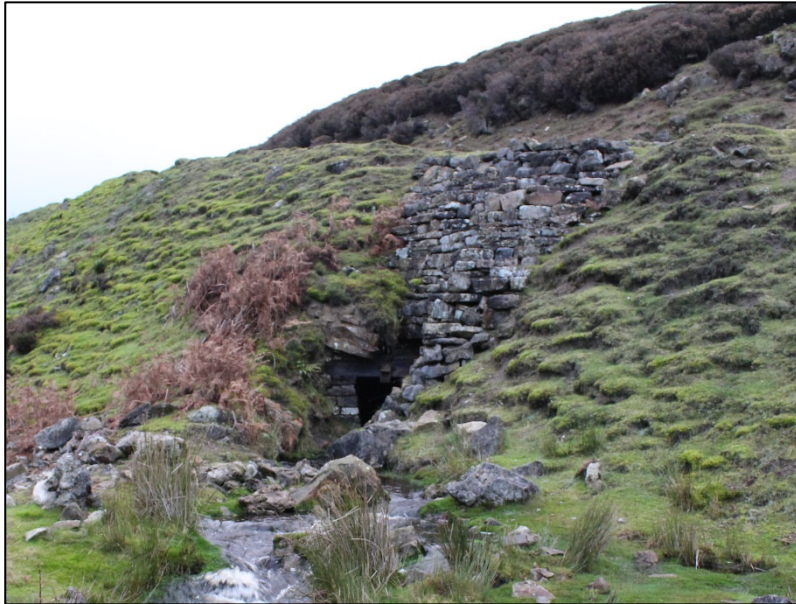
Plate 5: View of Hard Level Adit from south-south-east
