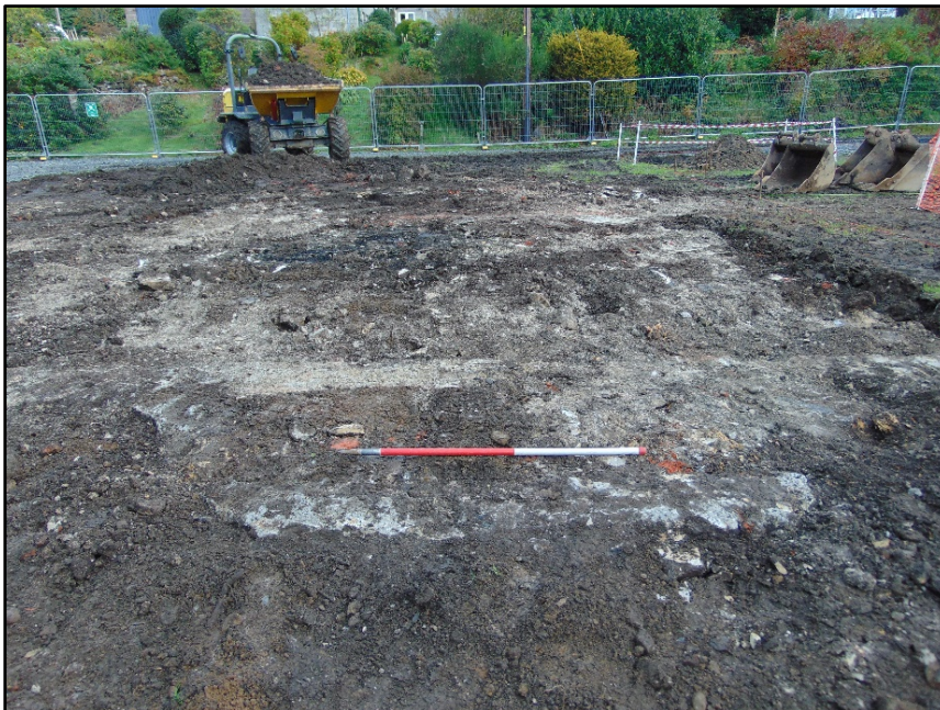
Plate 2; Wall foundations of earlier building seen in topsoil strip. Looking north East. 1m scale
