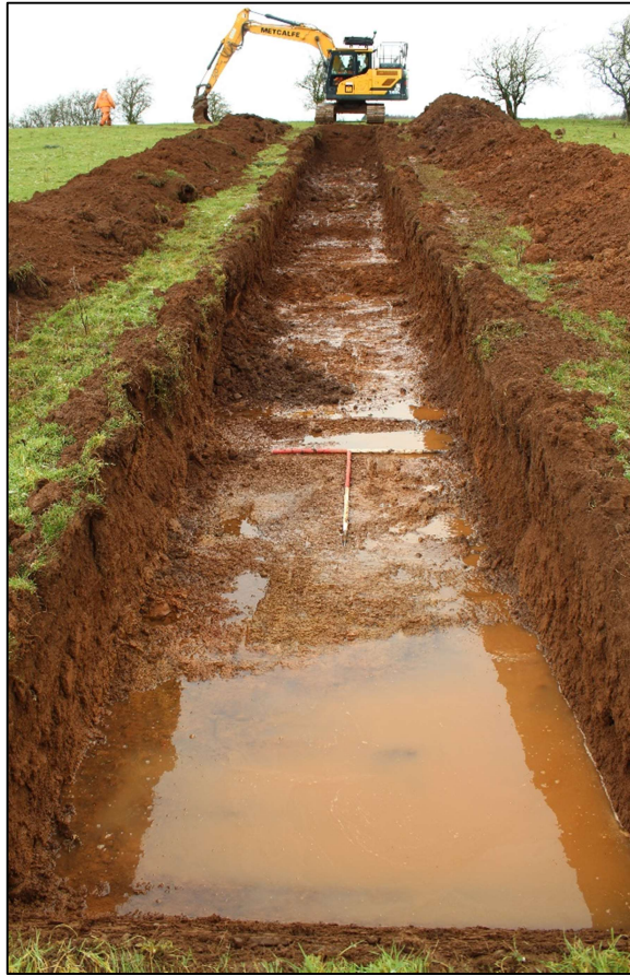
Plate 7; Trench 6, Looking north. 2 x 1m scale
