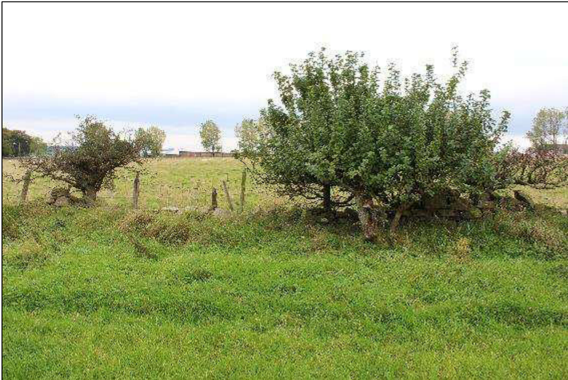
Plate 7: Asset 19: north-eastern side showing drystone wall, facing south-west
