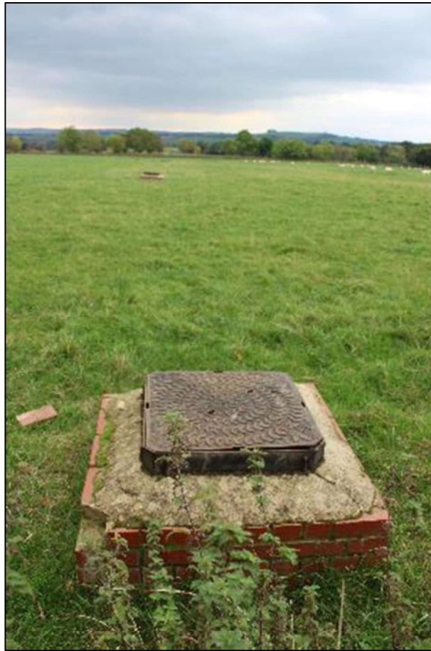
Plate 4: Westernmost access chamber, facing south-east
