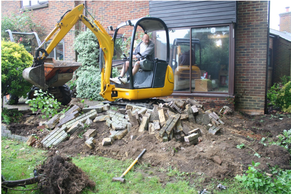
Plate 1: Workings shot of site
