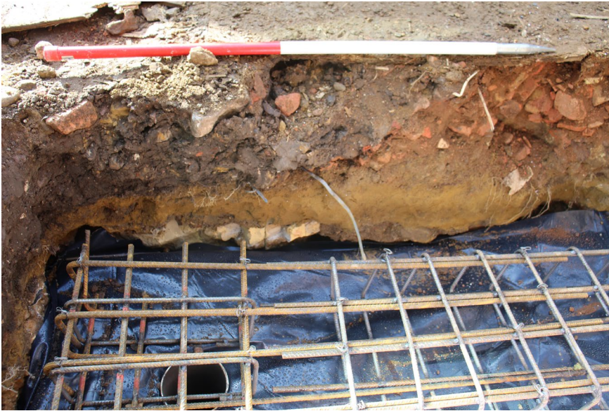
Plate 5: Sample Section 3 looking south-east
