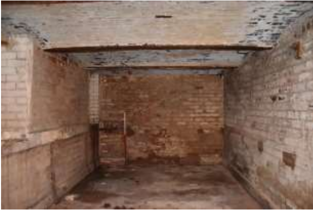
DP 49: Internal view of the vaulted cellar, taken from the north-east.
