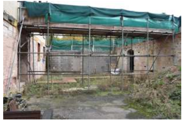
DP 8: General view of the former basement, taken from the west.
