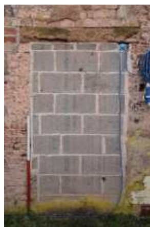
DP 28: Detail of the short fenestration with its stone lintel, taken from the south-east.
