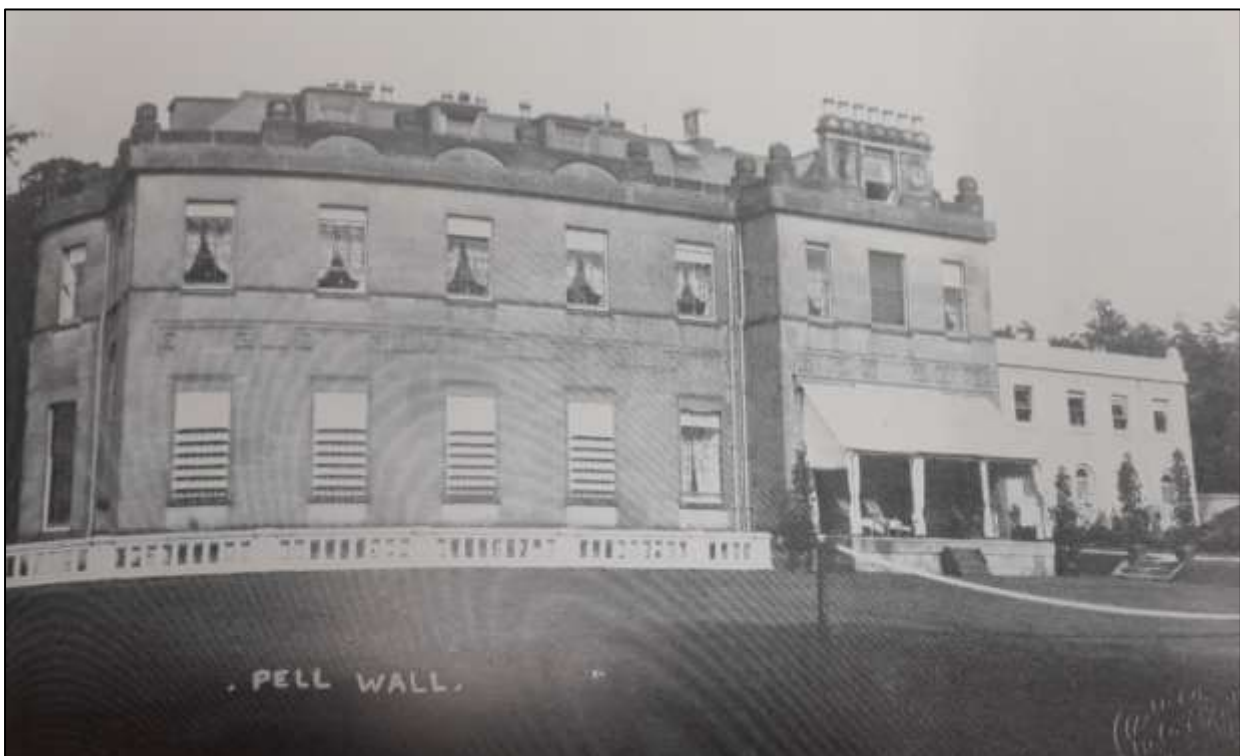
Fig.I: A c.1930 photograph of the western elevation following Edwardian alteration (Morris and Morris 1989)
