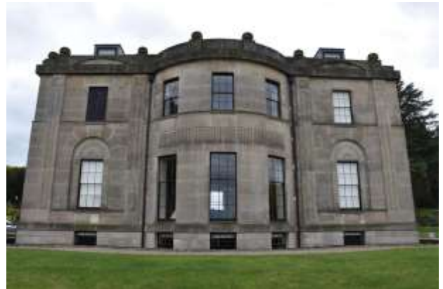
DP 2: The north-western elevation, taken from the north-west.
