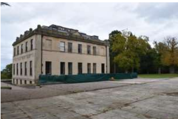
DP 5: The concrete-surfaced yard, taken from the south.
