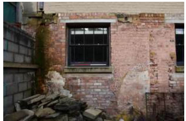
DP 12: The westernmost modern window in the position of original doorway, with infilled area below, taken from the south-east.
