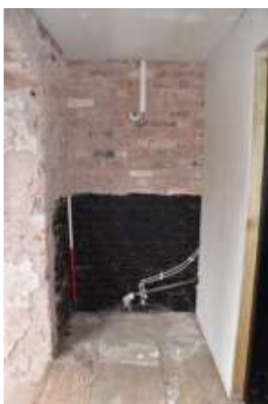
DP 23: Interior of the recessed entrance, taken from the north-east.
