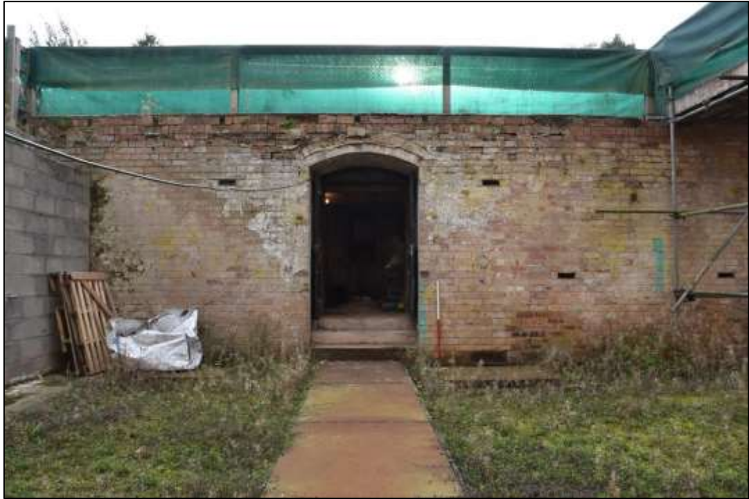
Plate 13: The Victorian wall of the vaulted cellar (DP 36)
