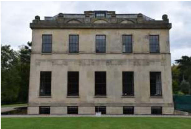
DP 3: The south-western elevation, taken from the south-west.
