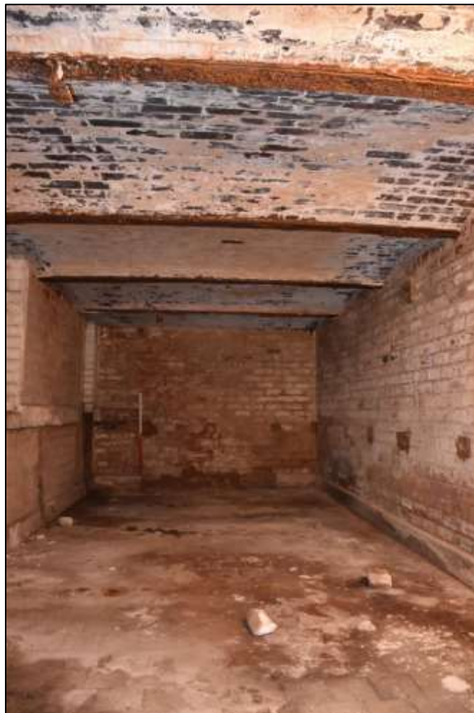
Plate 16: The barrel-vaulted cellar (DP 50)
