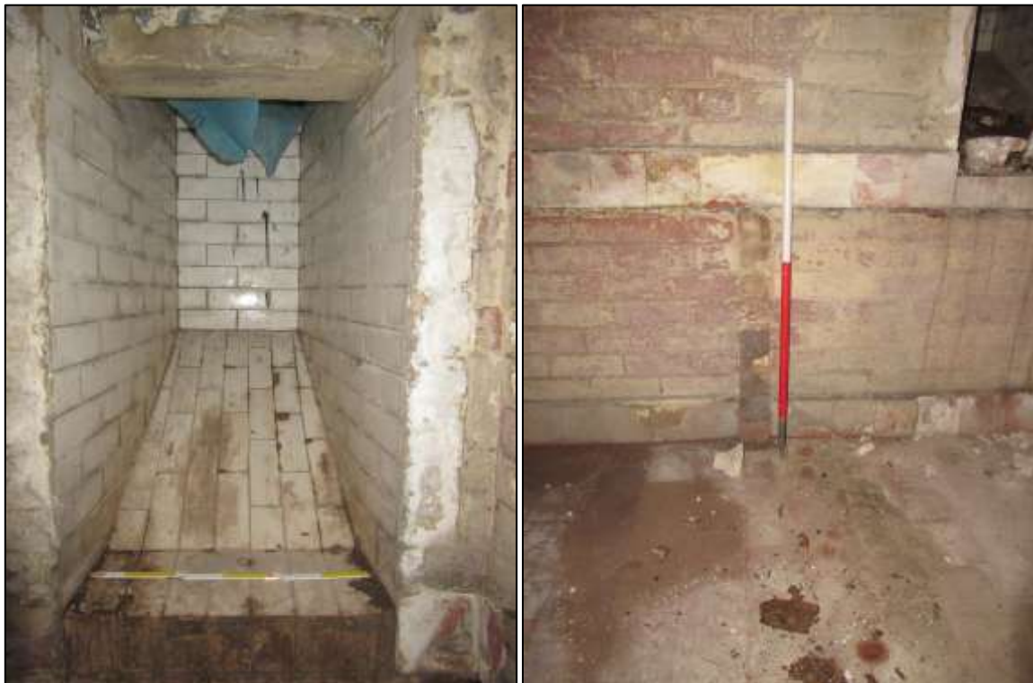
Plate 17: The cellar chutes or light wells – left (DP 52)
