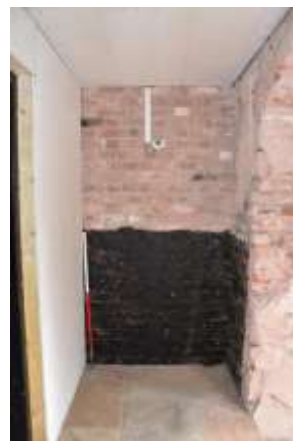
DP 22: Interior of the recessed entrance, taken from the south-west.
