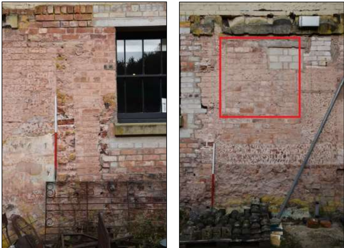
Plate 5: Remnants of an original demolished wall – left (DP 16).
