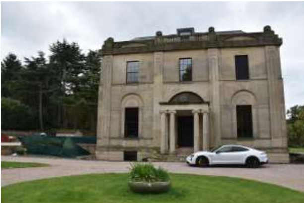
DP 1: The north-eastern elevation, taken from the north-east.
