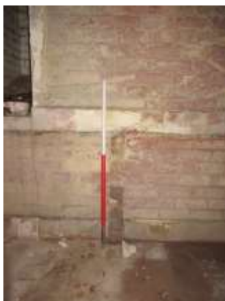
DP 53: Detail of the possible remnants of a shelf, with the tile 'splashback', taken from the north-west.
