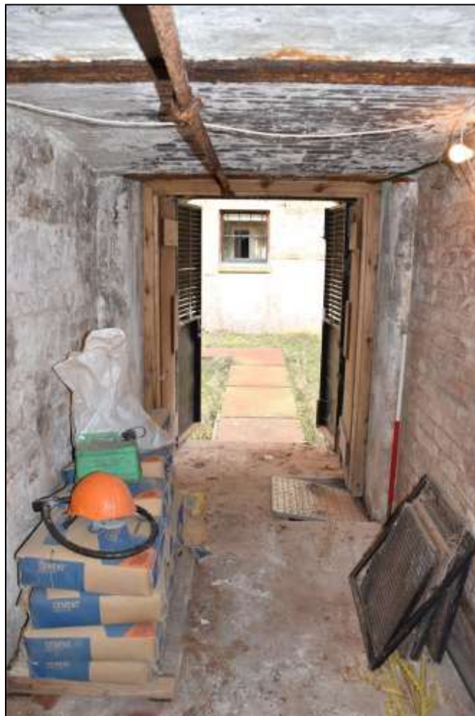
Plate 15: The corridor of the vaulted cellar (DP 45)
