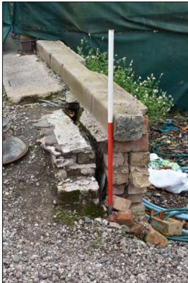
Plate 14: The Victorian wall and Soane's original (DP 41)
