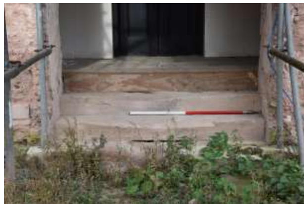
DP 20: The worn stone steps up to the recessed area, taken from the south-east.
