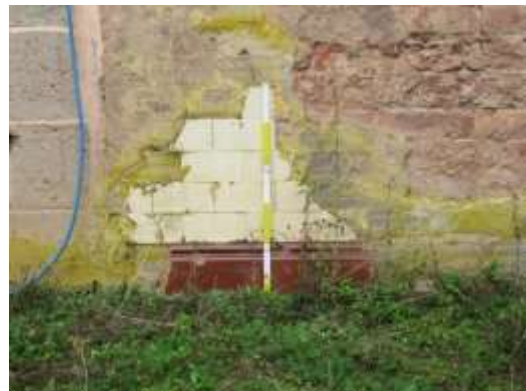
DP 34: Sample of the tiles that once lined the eastern section of the elevation, taken from the south-east.
