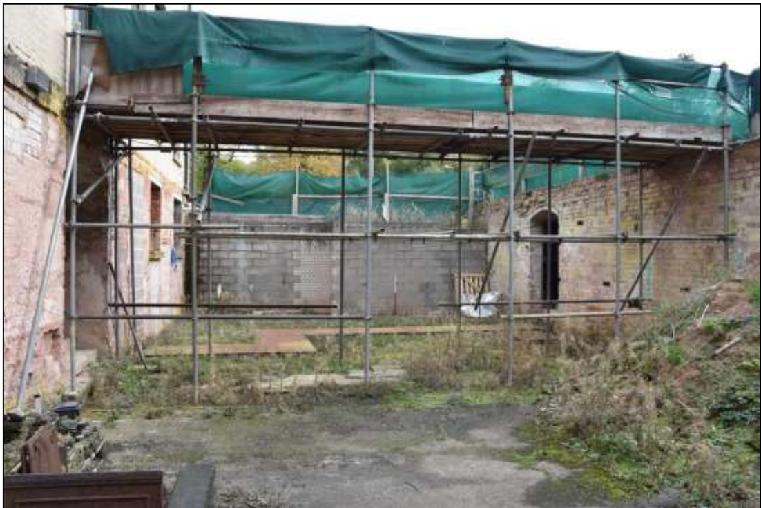
Plate 2: The former southern basement (DP 8).
