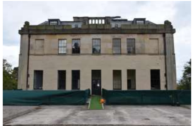
DP 4: The south-eastern elevation, taken from the south-east.
