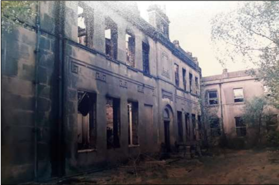
Fig.G: A 1992 photograph of the derelict Victorian extension (Shropshire SMR Slide Storage) - showing the south east elevation and later Edwardian wing adjoining perpendicular. Evidence of the covered passageway ( Confer para 3.5.2 )
