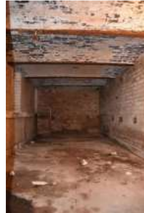
DP 50: Internal view of the vaulted cellar, taken from the north-east.
