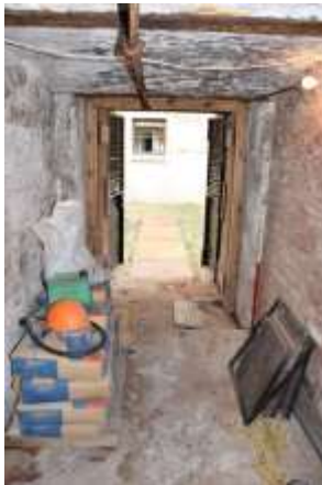
DP 45: Internal view of the cellar corridor, taken from the south-east.
