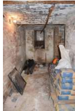
DP 44: Internal view of the cellar corridor, taken from the north-west.
