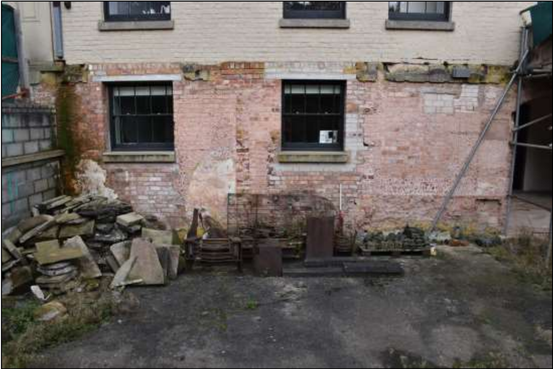
Plate 4: The western section of the south-eastern elevation (DP 11).
