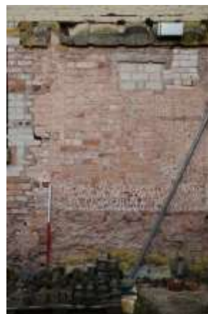
DP 14: Infilled area of original recess in brickwork, taken from the south-east.
