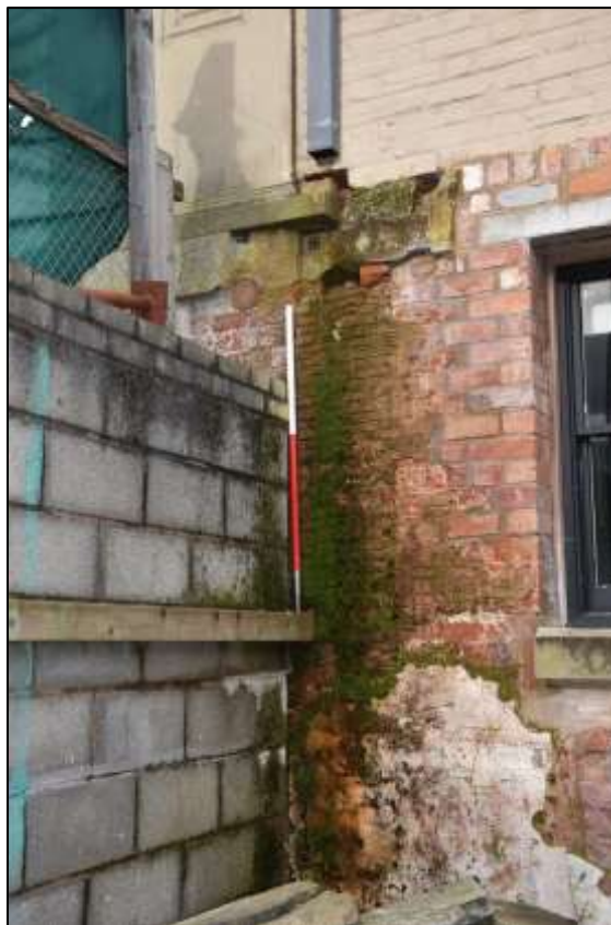
Plate 11: Potential remnants of the original retaining wall and later render (DP 15)
