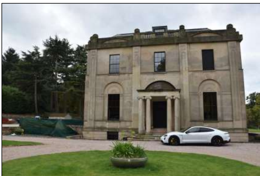
Plate 1: The north-eastern elevation of Pell Wall Hall (DP 1).
