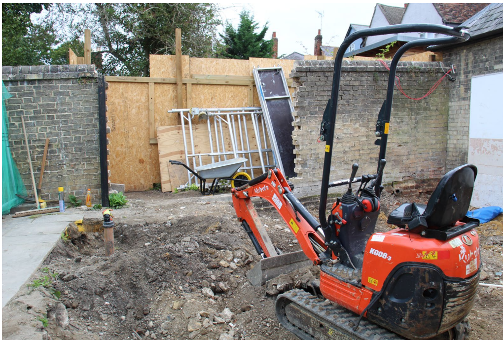
Plate 2: General working shot of northern area looking east
