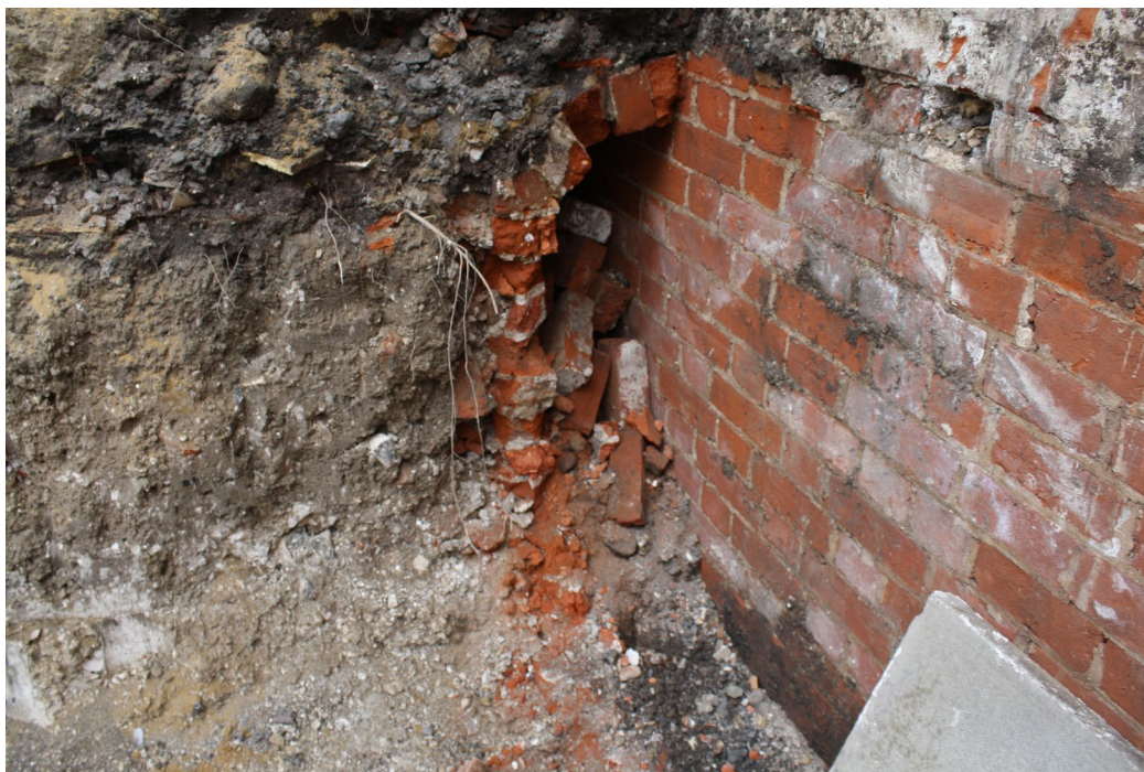
Plate 7: Detail of the post-medieval brick archway
