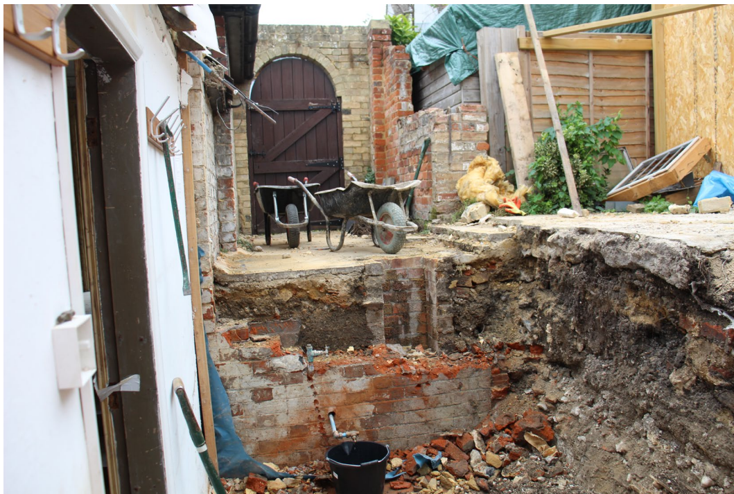
Plate 5: The kitchen area looking north-east
