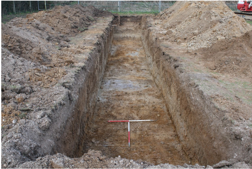
Plate 5: Pre-excitation shot of the trench looking north-west
