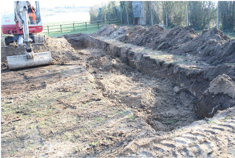
Plate 9: Site being backfilled
