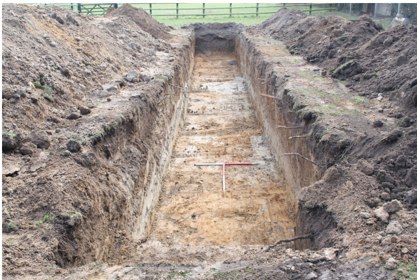
Plate 4: Pre-excavation shot of the trench looking south-east
