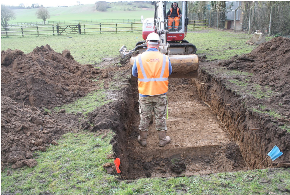
Plate 3: working shot of trench being opened
