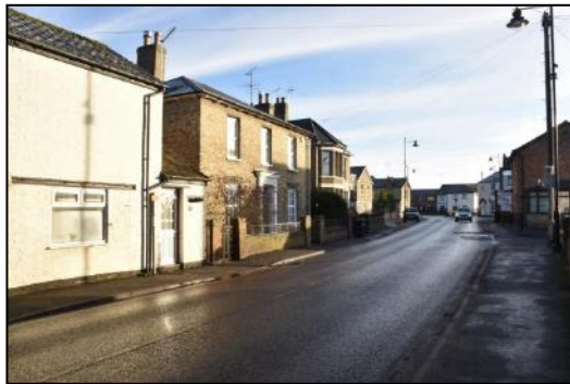
DP 1 View along Wellington Street from the assessment structure, taken from the west
