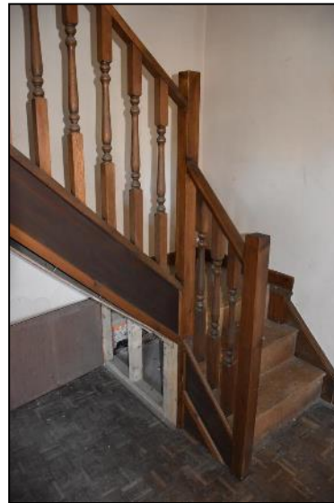
DP 80 Modern staircase in GF04 (Range 3), taken from the north-east
