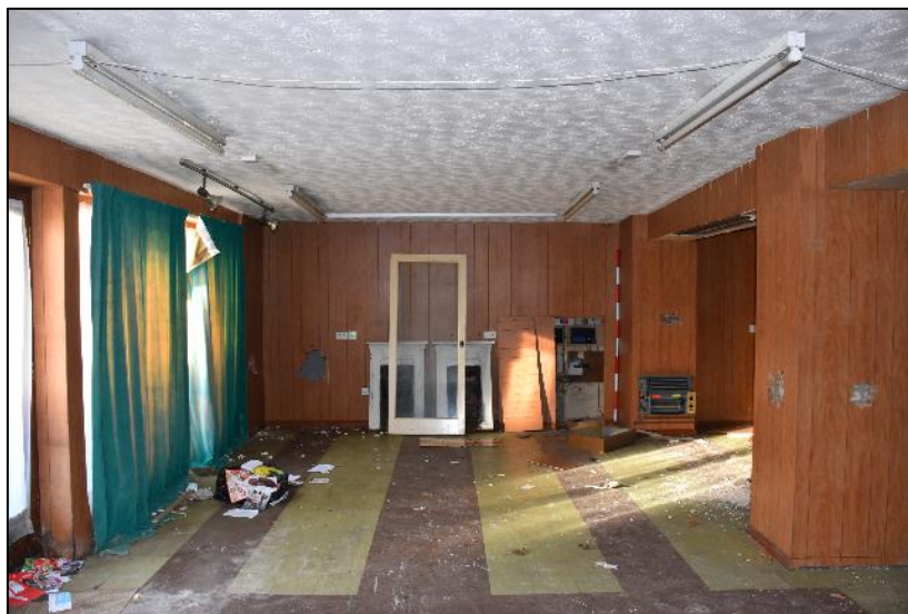
Plate 9 GF01 (Range 1) showing modern wall surfaces and openings created in the rear wall of the building (right), taken from the east (DP 61)
