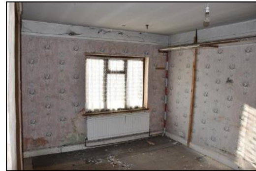
DP 112 South side of FF04 (Range 1), taken from the north-east
