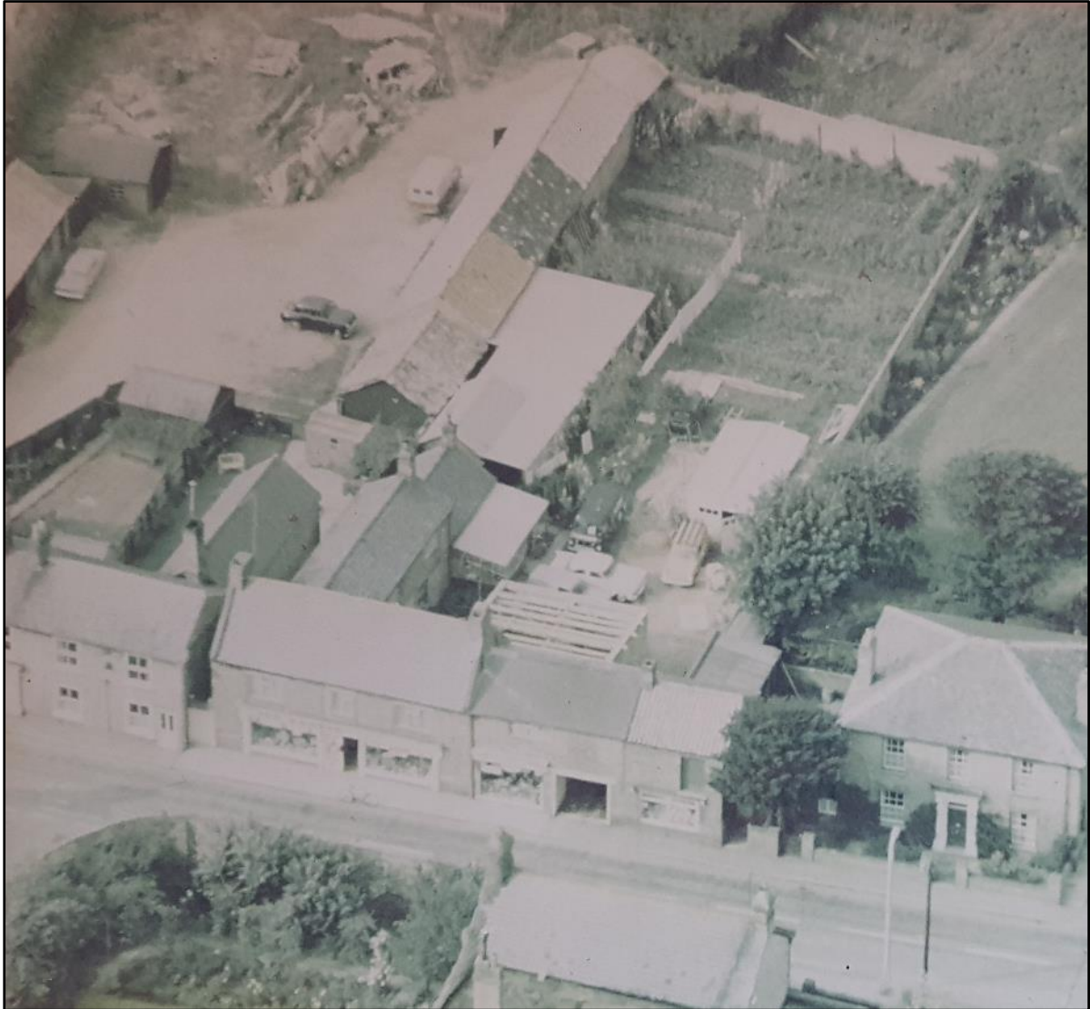
1.1 Aerial photograph of No. 20 Wellington Street, 1965 (Source: surviving within No. 20)
