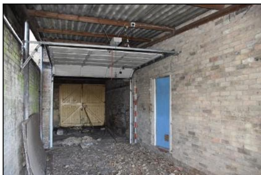
DP 47 The interior of the throughway (Range 1), taken from the north
