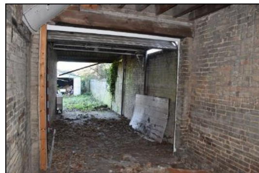
DP 48 The interior of the throughway (Range 1), taken from the south
