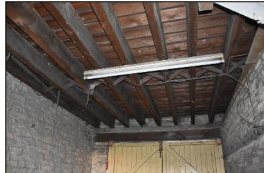
DP 50 Ceiling of the throughway (Range 1), taken from the north
