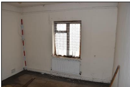
DP 125 South side of FF02 (Range 1), taken from the north
