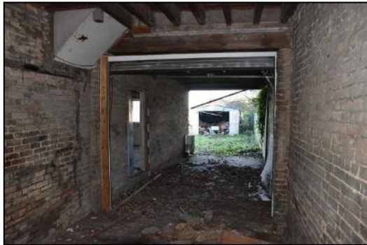
DP 49 The interior of the throughway (Range 1), taken from the south
