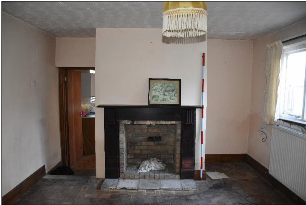
Plate 11 GF04 (Range 3), taken from the south (DP 77)
