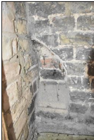
DP 75 West wall of GF02a (Range 6) showing junction between Ranges 3 and 5 and position of boot scraper, taken from the east
