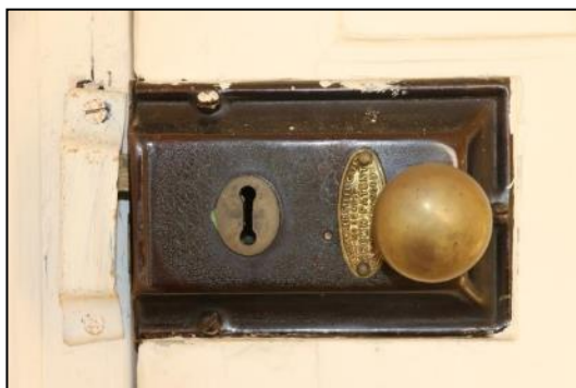
DP 131 Detail of the patent rim-lock on the door in FF02 (Range 1), taken from the south
