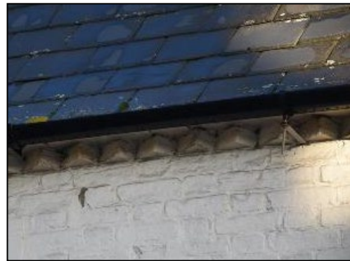
Plate 3 Dog-tooth dentilation at eaves level (Range 1), taken from the south (DP 9)
