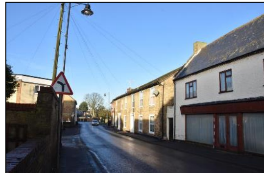
DP 2 View along Wellington Street from the assessment structure, taken from the east
