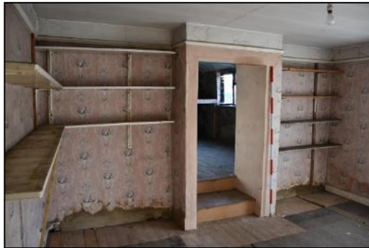
DP 111 East side of FF04 (Range 1) showing doorway punched through the chimney stack into the adjoining range, taken from the west
