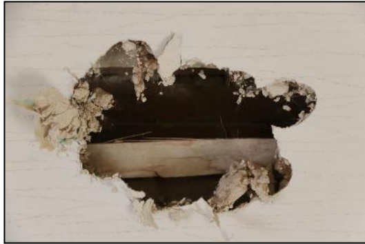
DP 127 West wall of FF02 (Range 1) showing hair rich lime plaster over studwork, taken from the south
