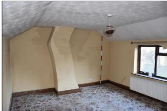
DP 157 FF10 (Range 3) showing integral chimney stack, taken from the south
