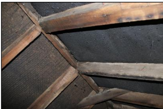
DP 155 The roof structure above FF09 (Range 3), taken from the north
