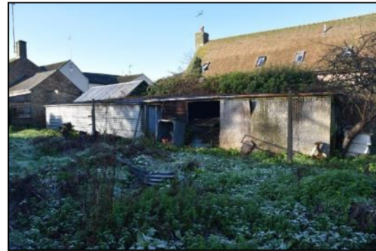
DP 44 Western outbuilding, taken from the east
