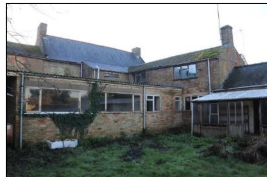
DP 42 Rear side of No. 20 with mid-20 th century Range 6 at low level, taken from the north-east
