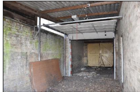
DP 46 The interior of the throughway (Range 1), taken from the north
