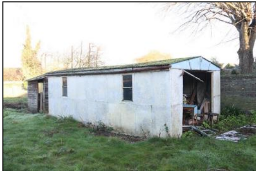
DP 45 Eastern outbuilding, taken from the south-west
