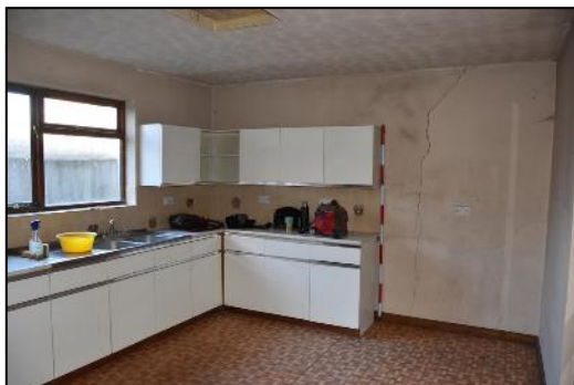
DP 89 GF05 (Range 4), taken from the south-east
