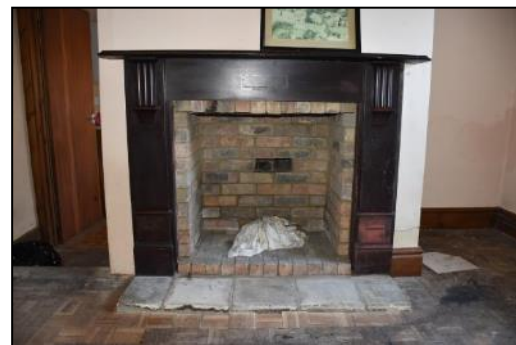
DP 82 Modern fireplace in GF04 (Range 3), taken from the south
