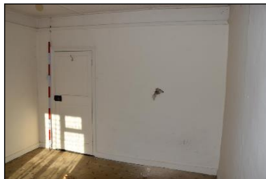
DP 126 North side of FF02 (Range 1), taken from the south
