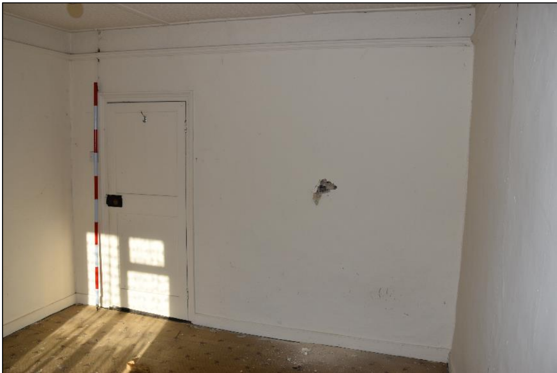
Plate 13 GF04 (Range 3), taken from the south (DP 77)
