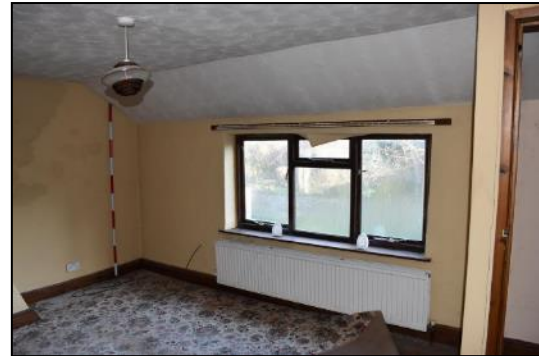
DP 158 FF10 (Range 3), taken from the south-west
