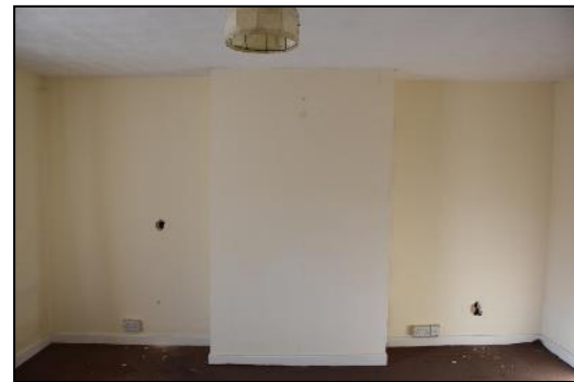
DP 136 West side of FF01 (Range 1), taken from the east
