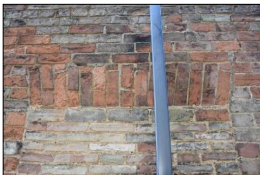
DP 35 West elevation (Range 3) showing brick arch over the blocked doorway, taken from the west
