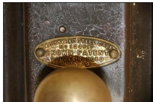
DP 132 Detail of the patent rim-lock on the door in FF02 (Range 1), taken from the south
