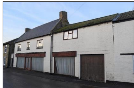
DP 4 South elevation, taken from the south-east
