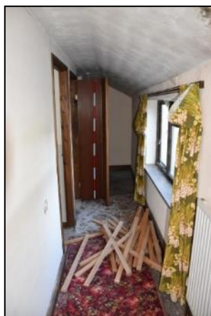
DP 149 Corridor FF07 (Range 3), taken from the south
