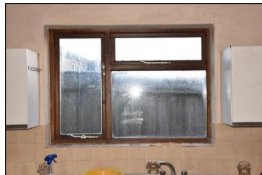
DP 90 West side of GF05 (Range 4) showing modern window, taken from the south-west
