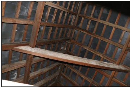
DP 133 Roof structure over FF02 (Range 1), taken from the east
