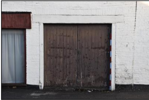
DP 19 Double doors enclosing the throughway (Range 2), taken from the south
