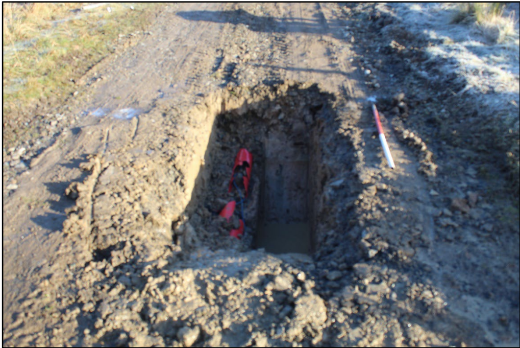
Plate 5; Cable Joint Pit 2, facing SSW, 1m scale.
