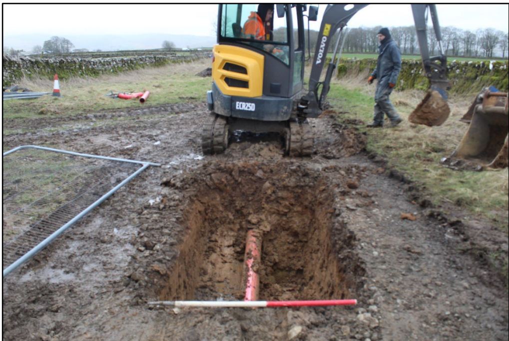
Plate 4; Cable Joint Pit 1, facing SSW, 1m scale.
