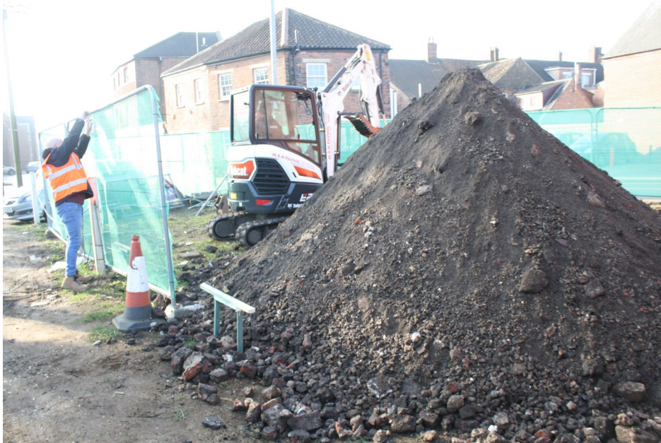
Plate 1: Working shot of Site
