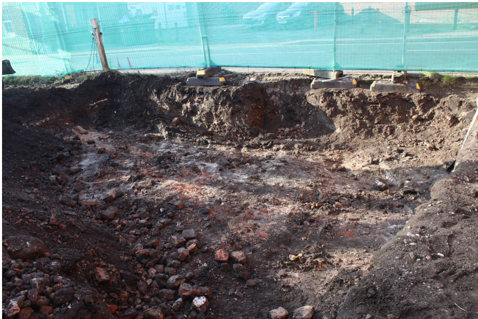
Plate 2: Working shot of site
