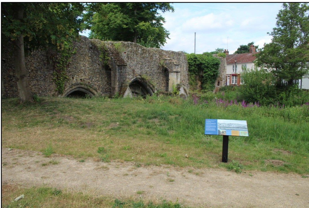
Plate 8: Post excavation shot of Test Pit 5, containing information panel. Northwest facing towards the Abbot's Bridge.
