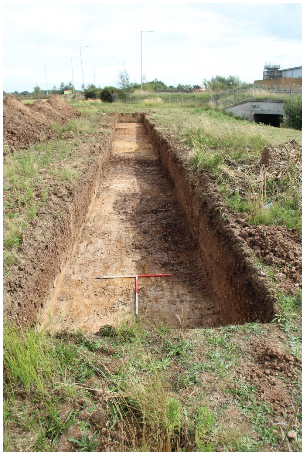
Plate 8: Trench 2 pre-excitation looking E
