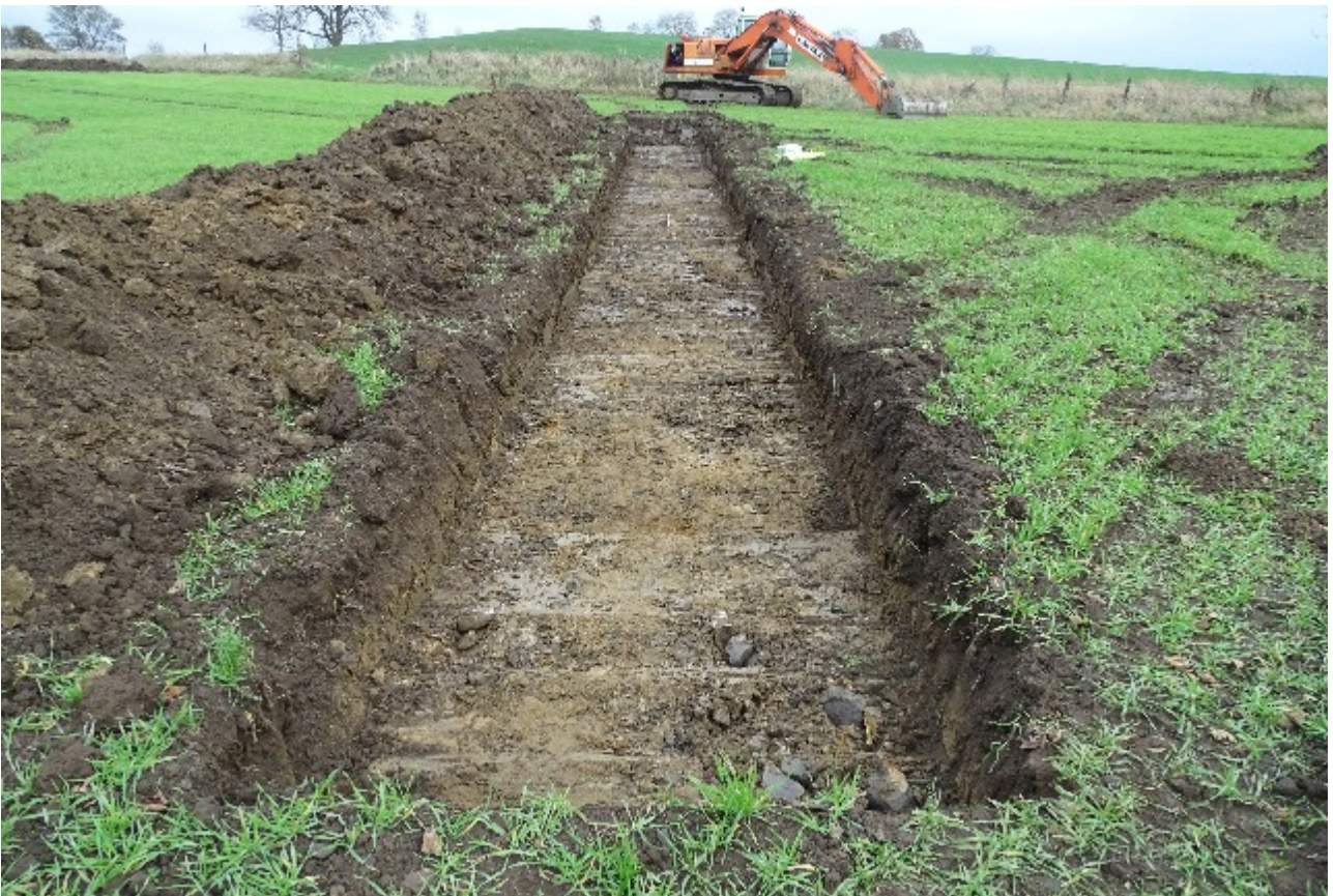
Plate 7. Trench D, looking northeast.
