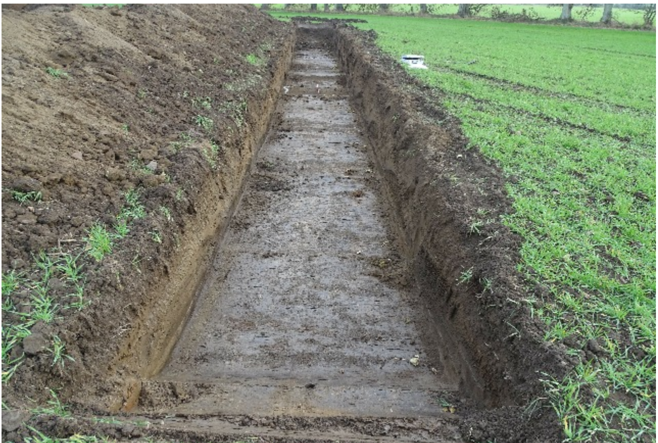
Plate 13. Trench J, looking southeast.
