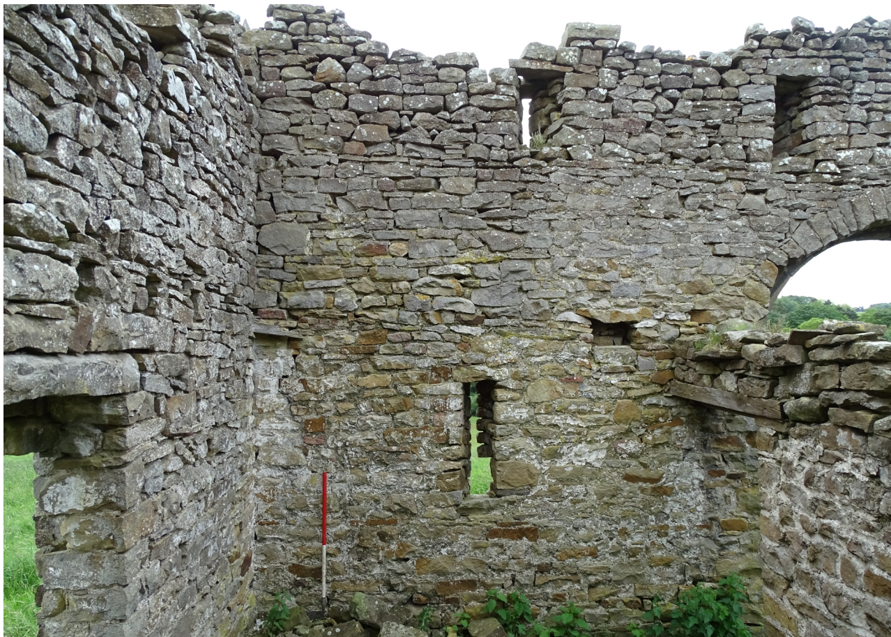
Plate 22. The south wall of Area B (frame GVB19039)
