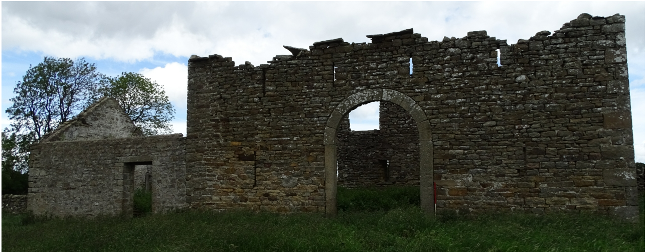
Plate 10. The southern elevation of the building (frame GVB19048)
