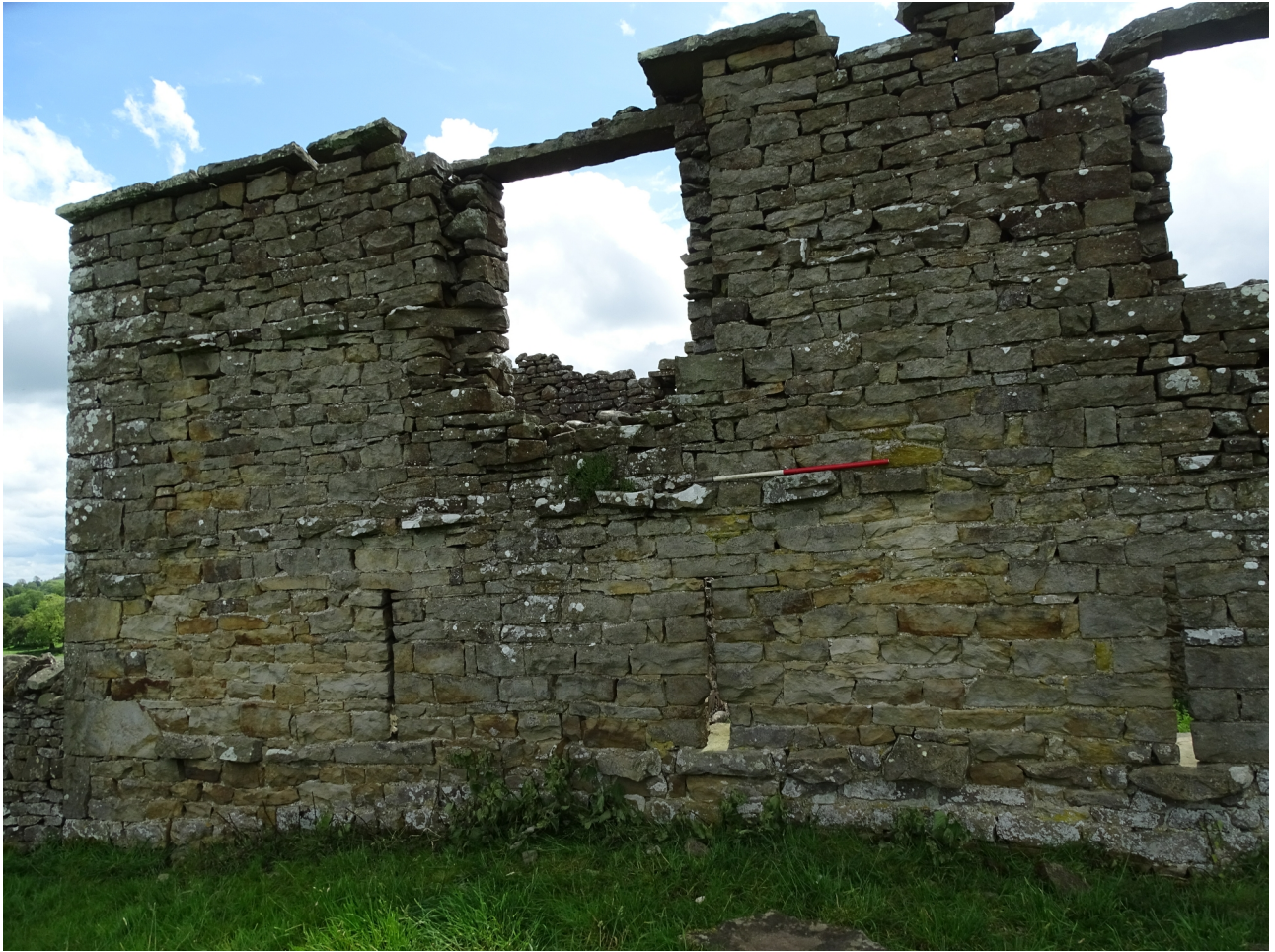
Plate 6. The northern elevation of the original barn (frame GVB19005)
