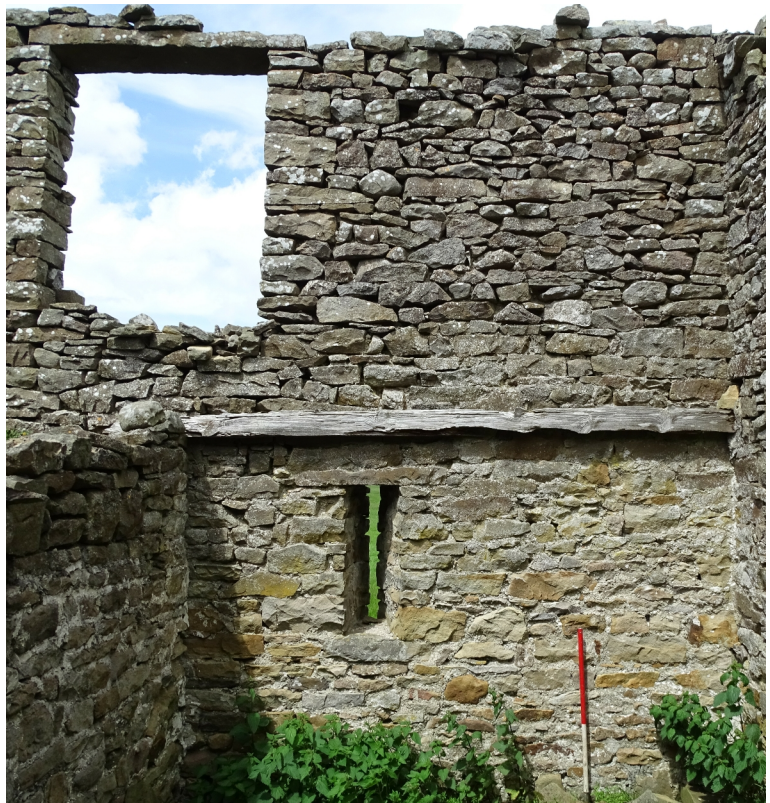
Plate 20. The north wall of Area B, showing detail of upper floor joists (frame GVB19040)
