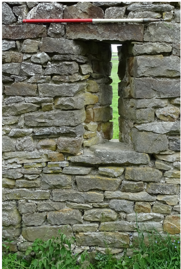
Plate 16. Area A, arrow loop window detail (frame GVB19032)
