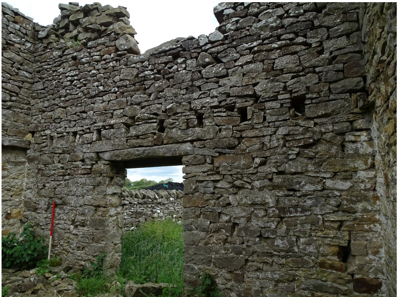
Plate 21. The east wall of Area B, showing detail of upper floor joist sockets (frame GVB19043)
