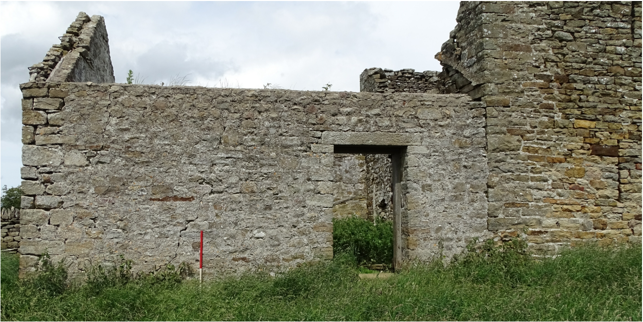
Plate 12. The southern elevation of the extension (frame GVB19011)
