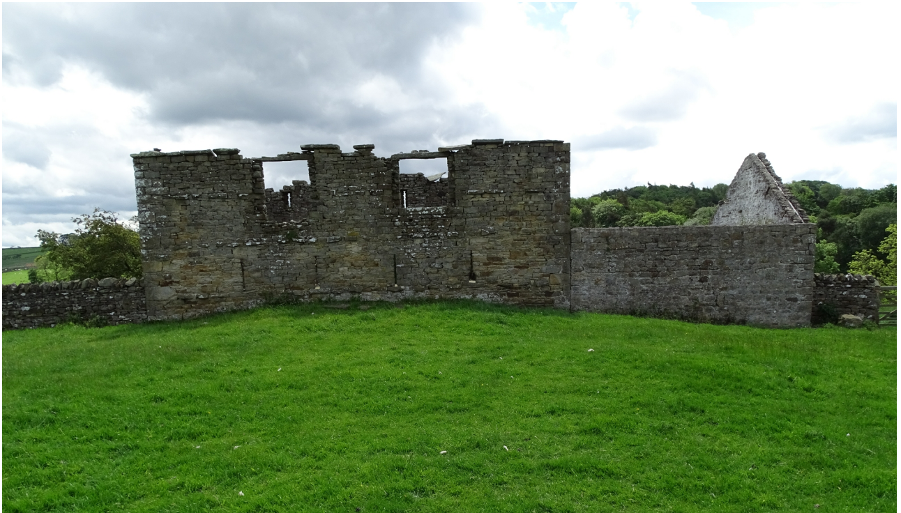
Plate 5. The northern elevation of the overall building (frame GVB19002)
