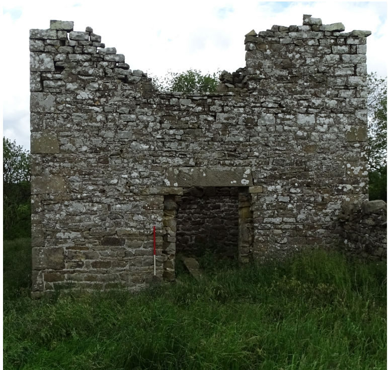
Plate 13. The eastern elevation (frame GVB19050)
