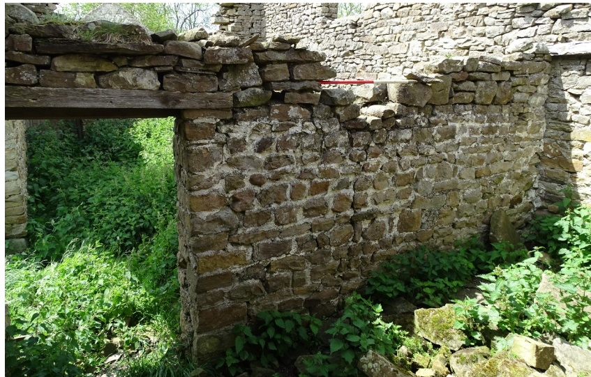
Plate 19. The west wall of Area B, (frame GVB19040)
