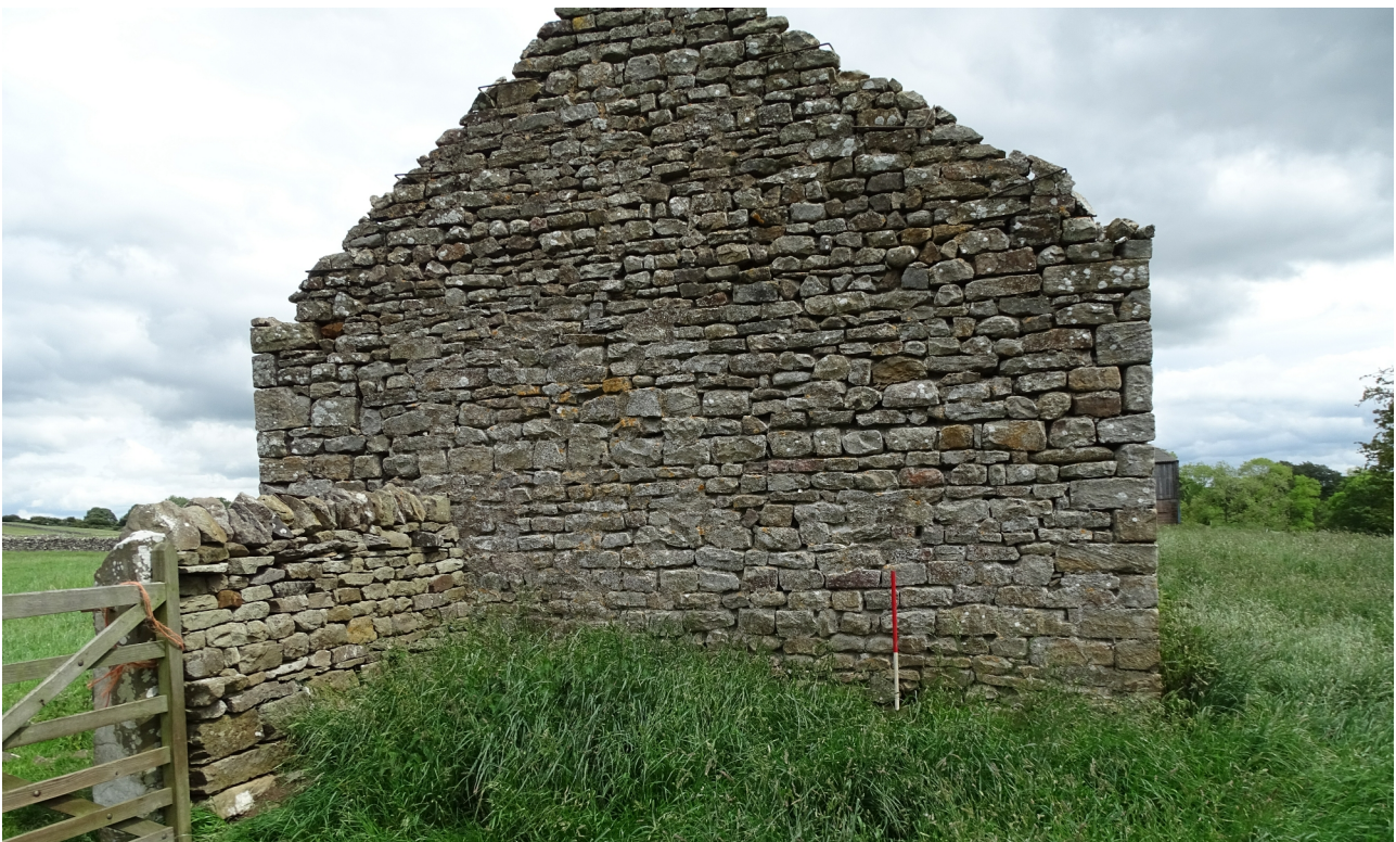
Plate 9. The western elevation of the extension (frame GVB19008)
