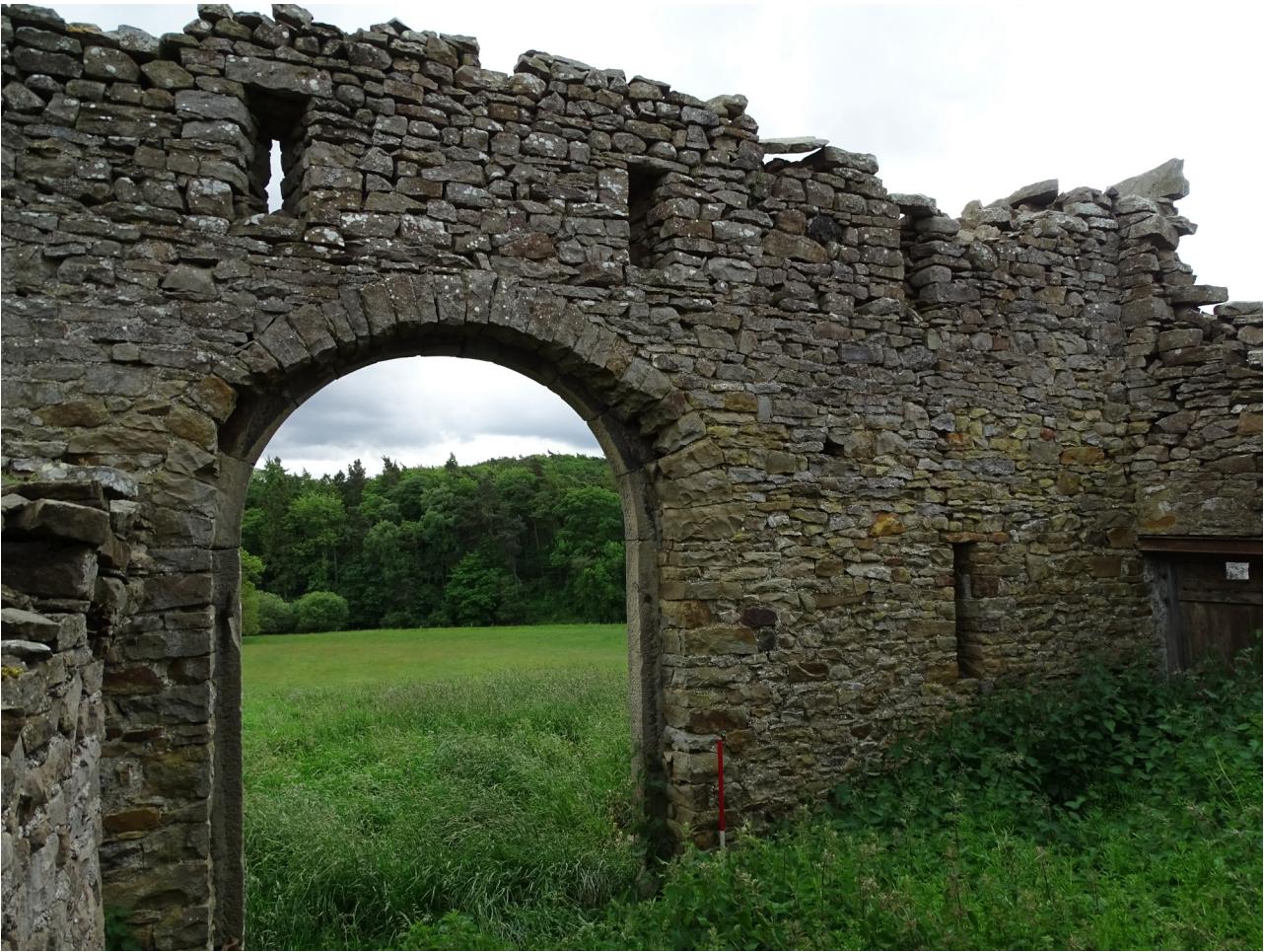
Plate 18. The south wall of Area A, showing detail of the arch and arrow loop windows (frame GVB19025)
