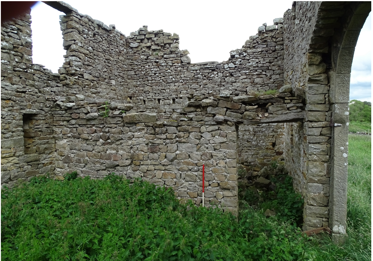
Plate 17. The eastern wall of Area A, with Area B beyond (frame GVB19028)
