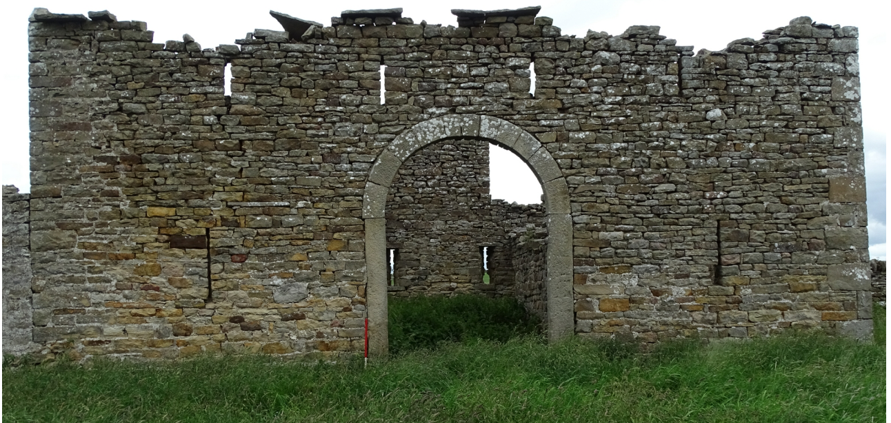
Plate 11. The southern elevation of the original barn building (frame GVB19020)
