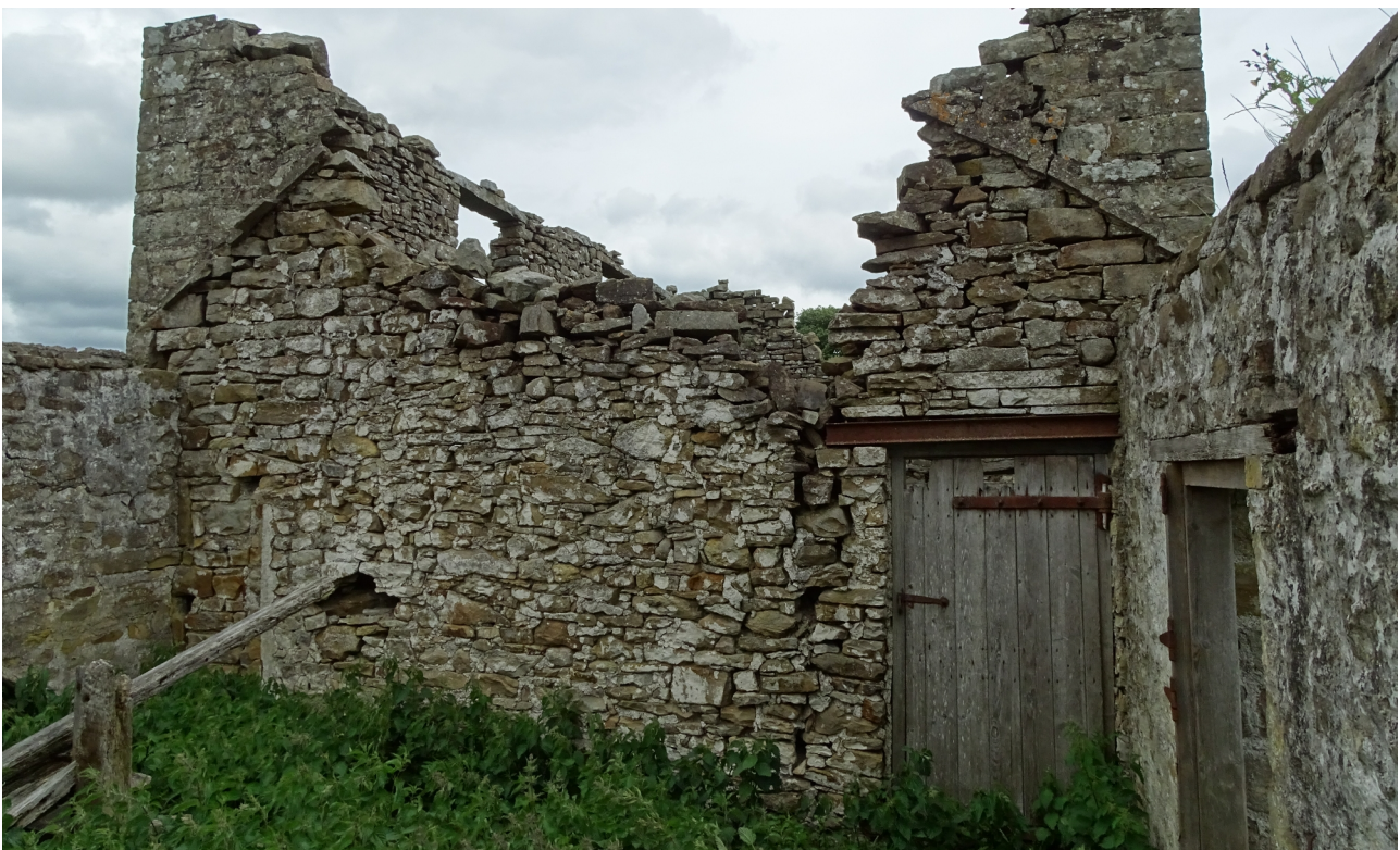
Plate 25. The eastern wall of Area C (frame GVB19017)
