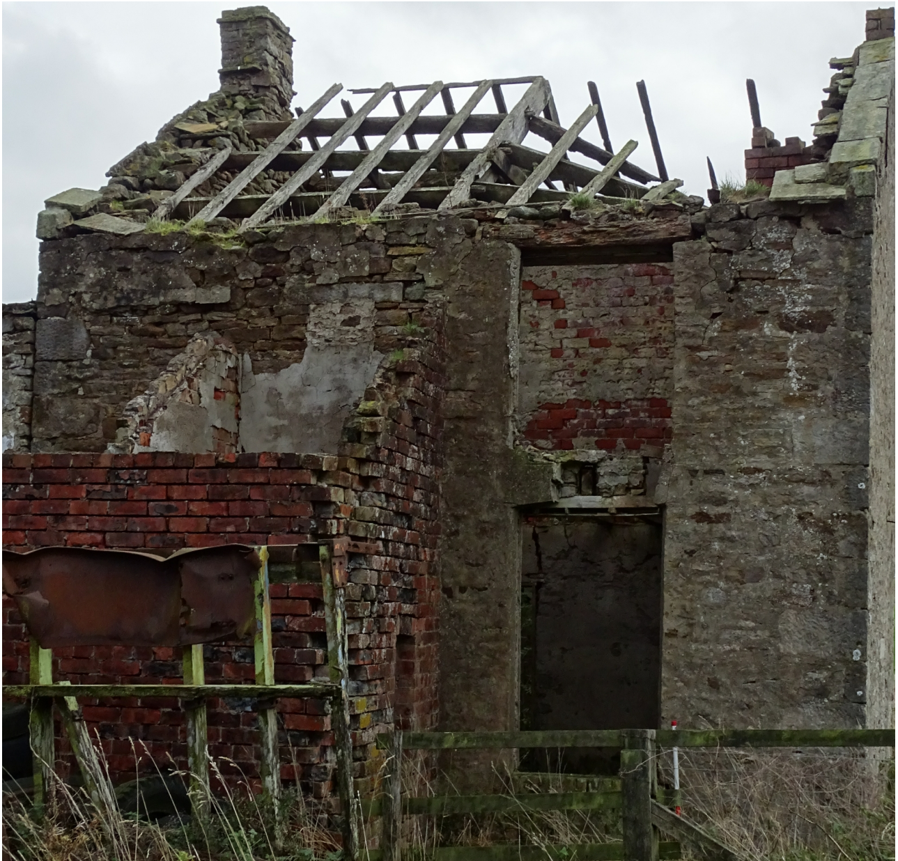
Plate 12. The north-west elevation of the main house (frame WCW010).
