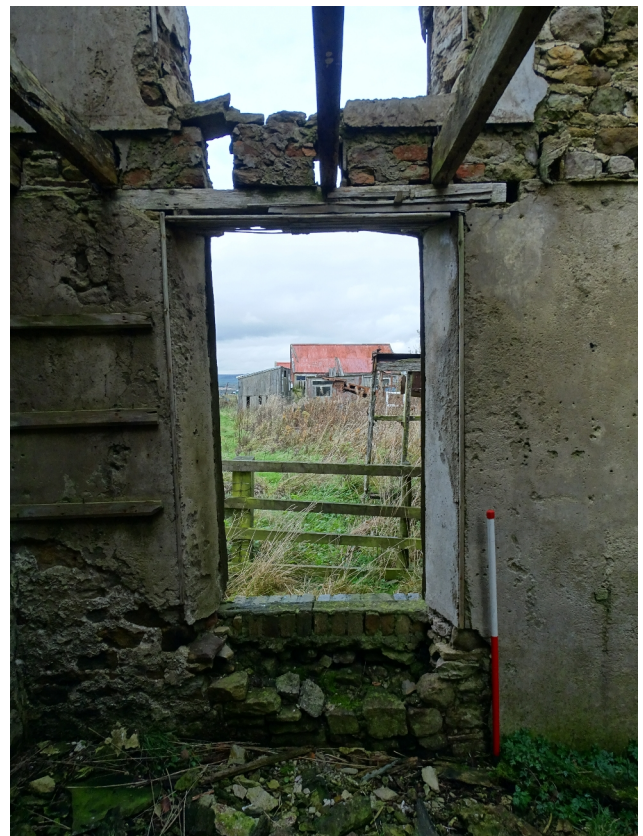
Plate 28. The ground floor window in Room B (frame WCW031).
