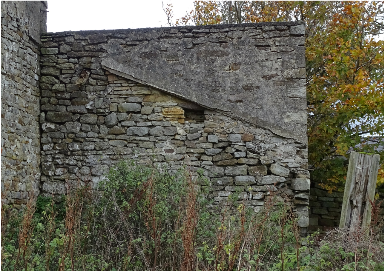
Plate 16. The internal south-facing wall of the lean-to (frame WCW017).
