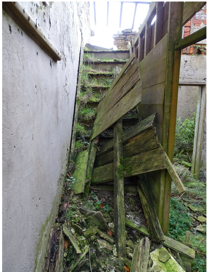
Plate 25 (right). The timber framed staircase in Room B (frame WCW035).
