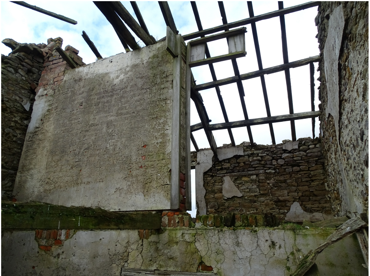
Plate 22. The northwestern wall of Room A, upper floor (frame WCW021).
