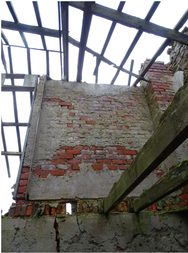
Plate 26. The first floor southeast wall of Room B (frame WCW030).
