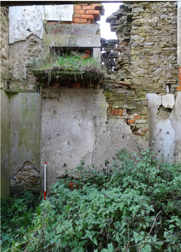
Plate 19. The chimney and suspended upper floor hearth (frame WCW018).
