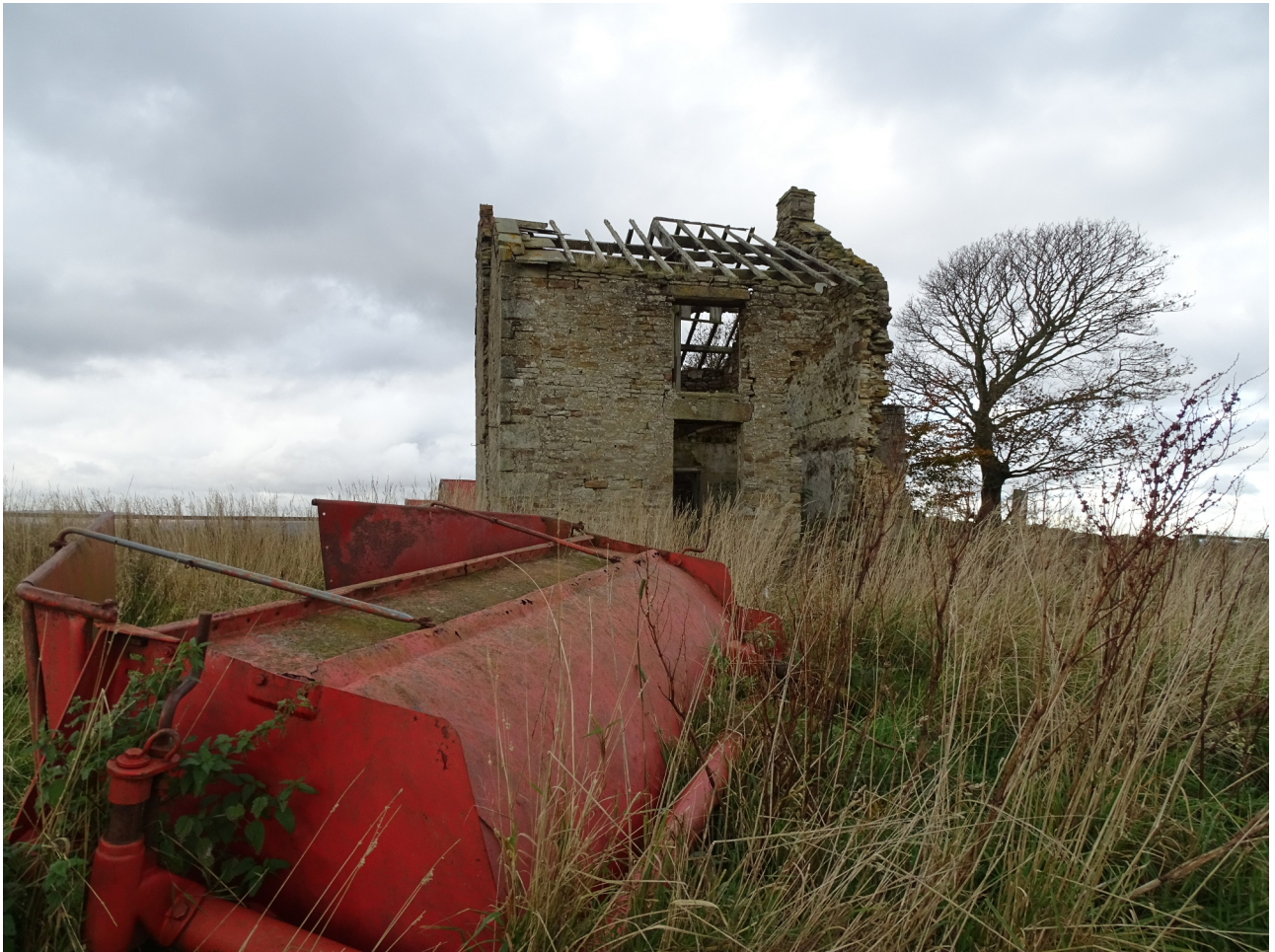
Plate 36. The house from the southeast (frame WCW001).
