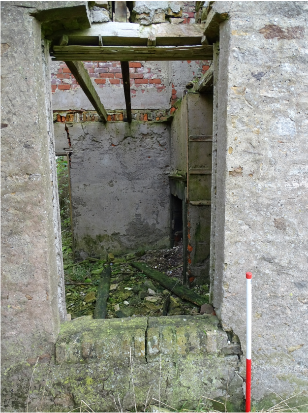
Plate 13. The north-west elevation ground floor window (frame WCW011).
