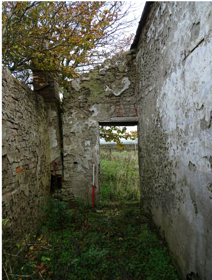
Plate 30. The late 19 th century extension looking northeast (frame WCW039).
