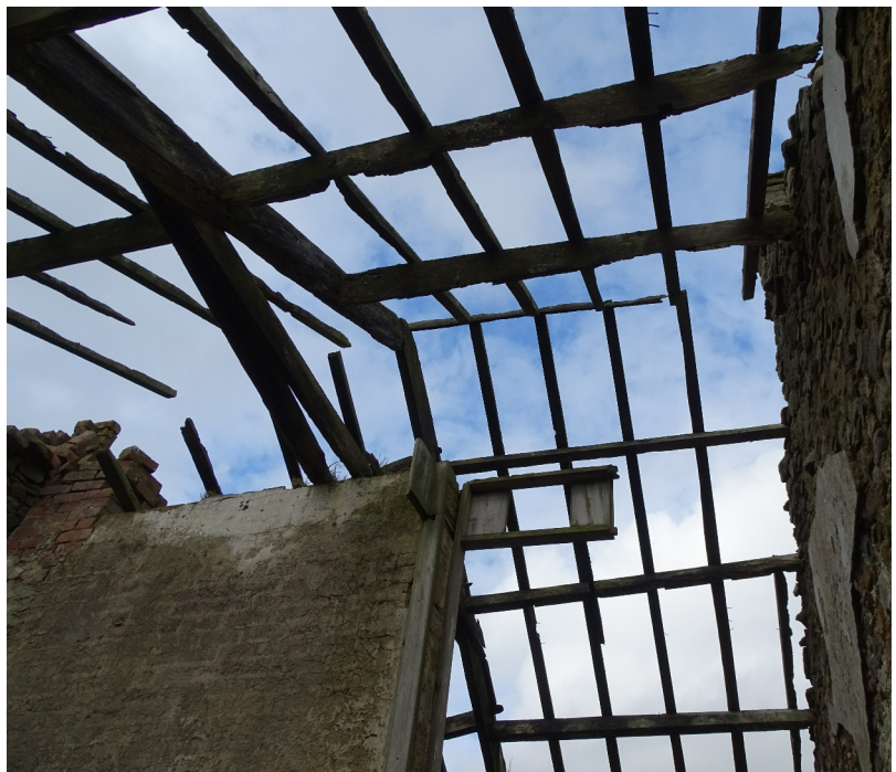
Plate 23. The roof structure from Room A (frame WCW022).
