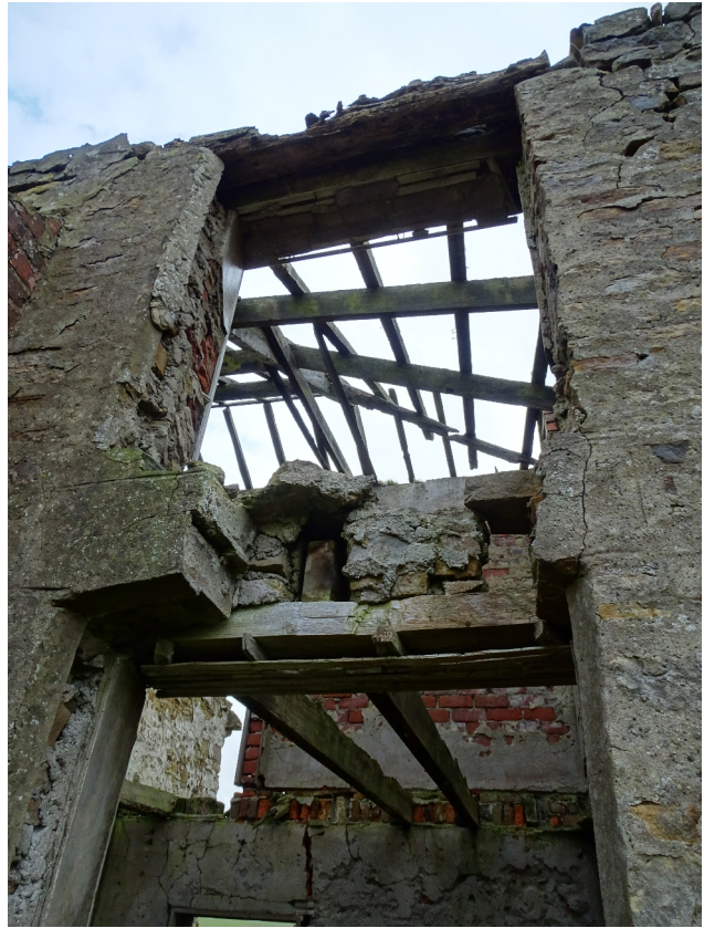
Plate 14. The north-west elevation first floor window (frame WCW011).
