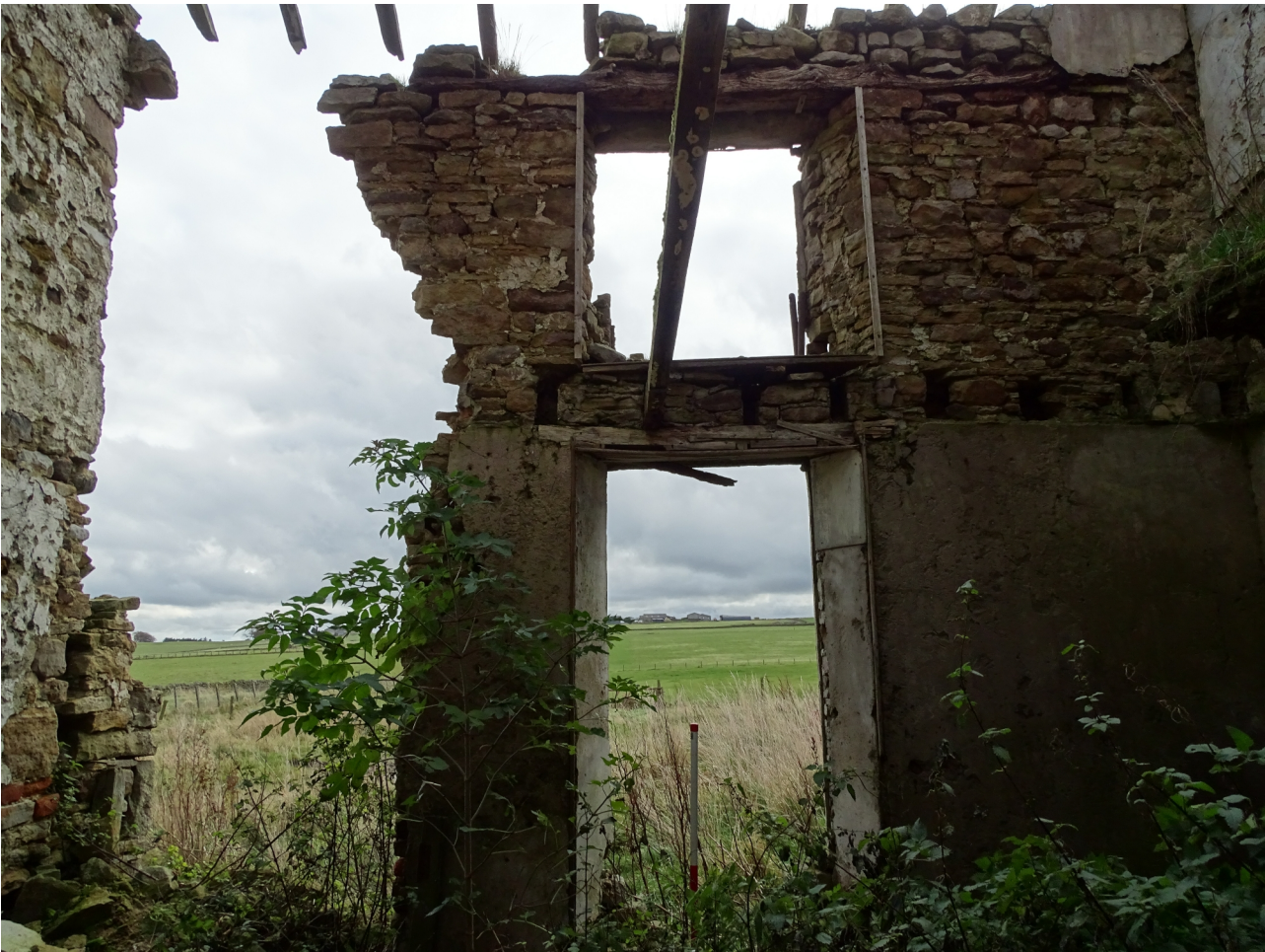
Plate 18. The internal north-west facing wall of Room A (frame WCW025).
