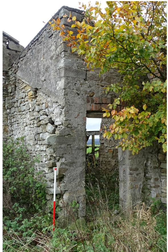
Plate 17. The north-east elevation of the extension (frame WCW014).
