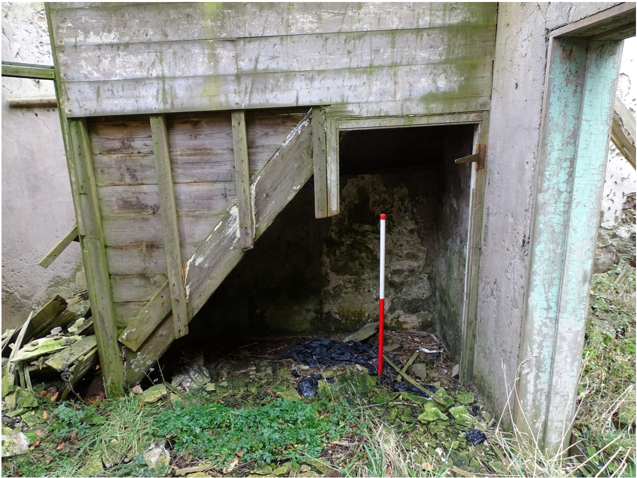
Plate 24 (above). The timber framed staircase in Room B (frame WCW033).
