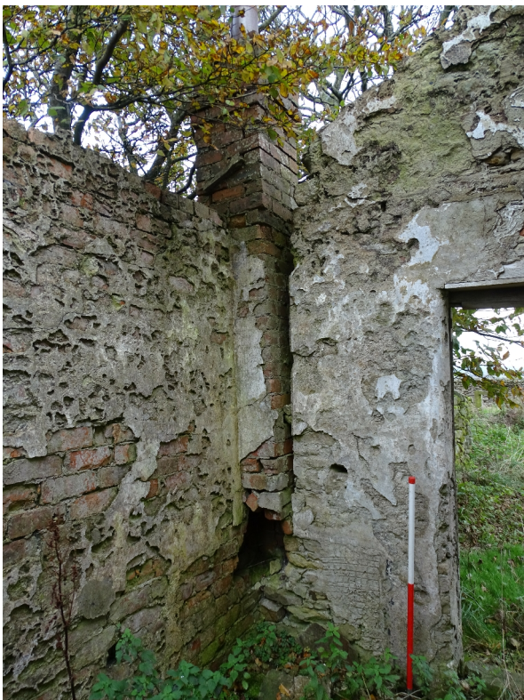
Plate 32. The chimney in the northeast corner of the extension (frame WCW040).
