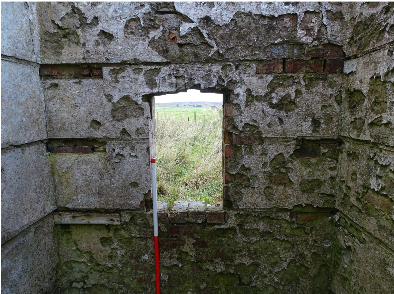
Plate 35. Room D looking southwest (frame WCW037).
