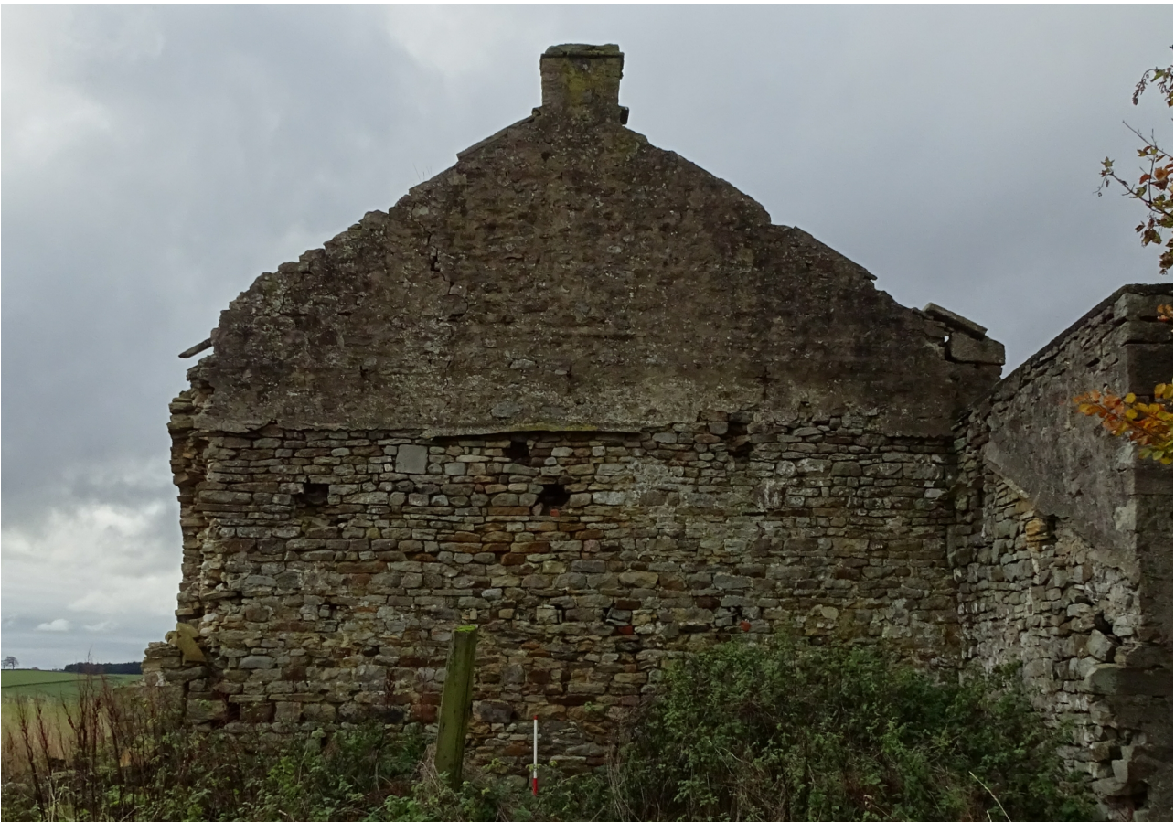
Plate 15. The north-east elevation (frame WCW015).
