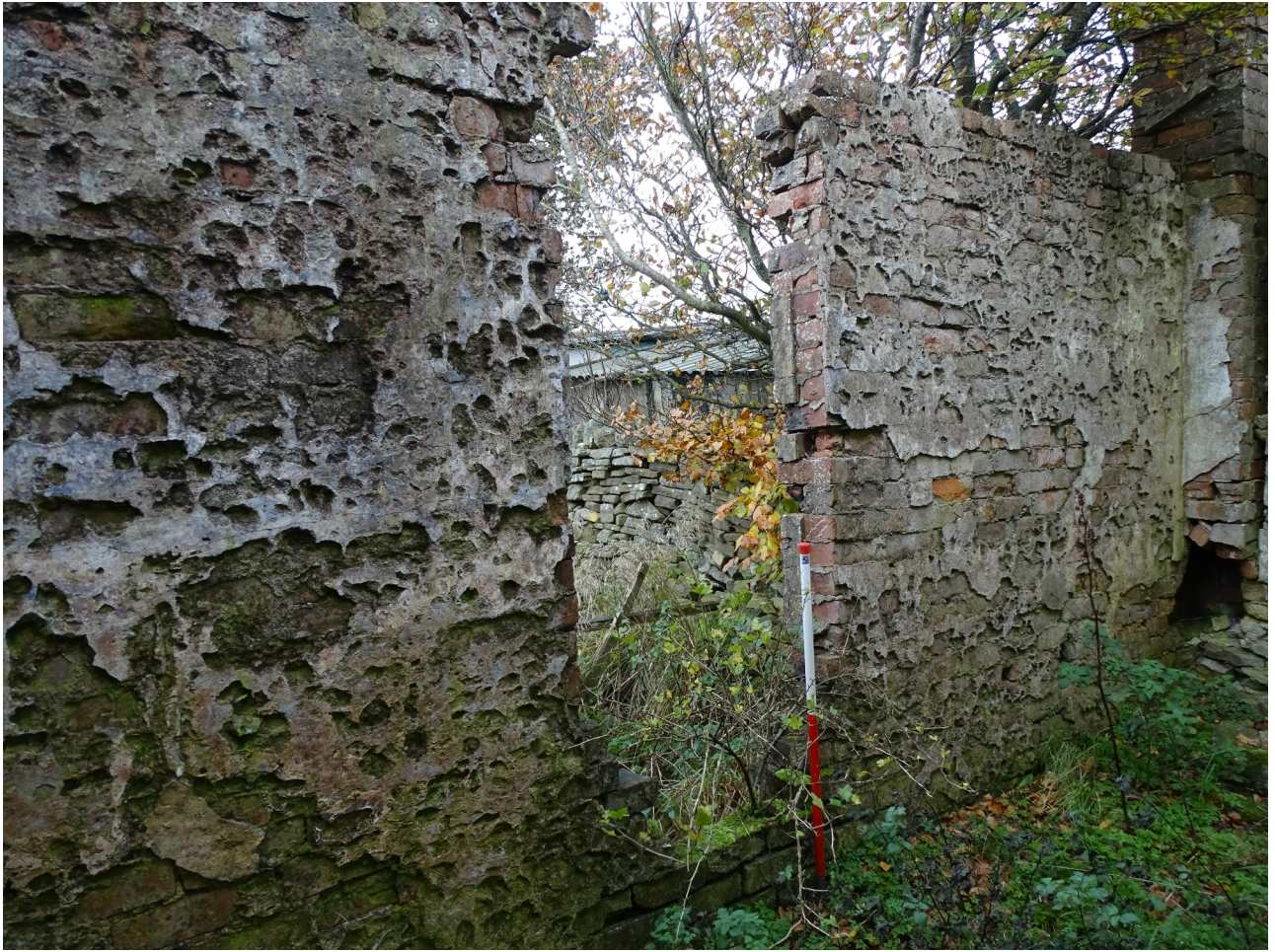
Plate 31. The window within the northwestern wall of the extension (frame WCW042).
