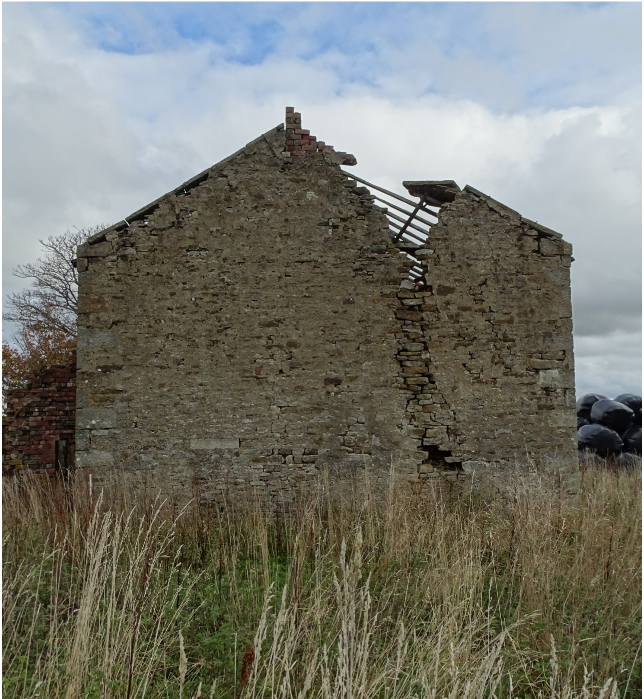
Plate 9. The south-west elevation (frame WCW007).
