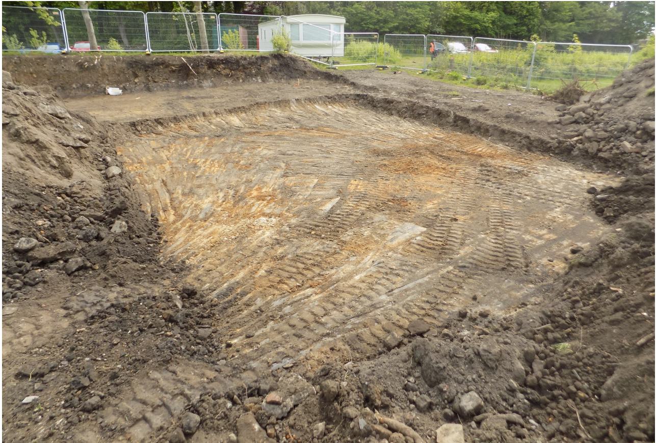
Plate 4 (above). The platform strip for the house foundations, looking southeast.
