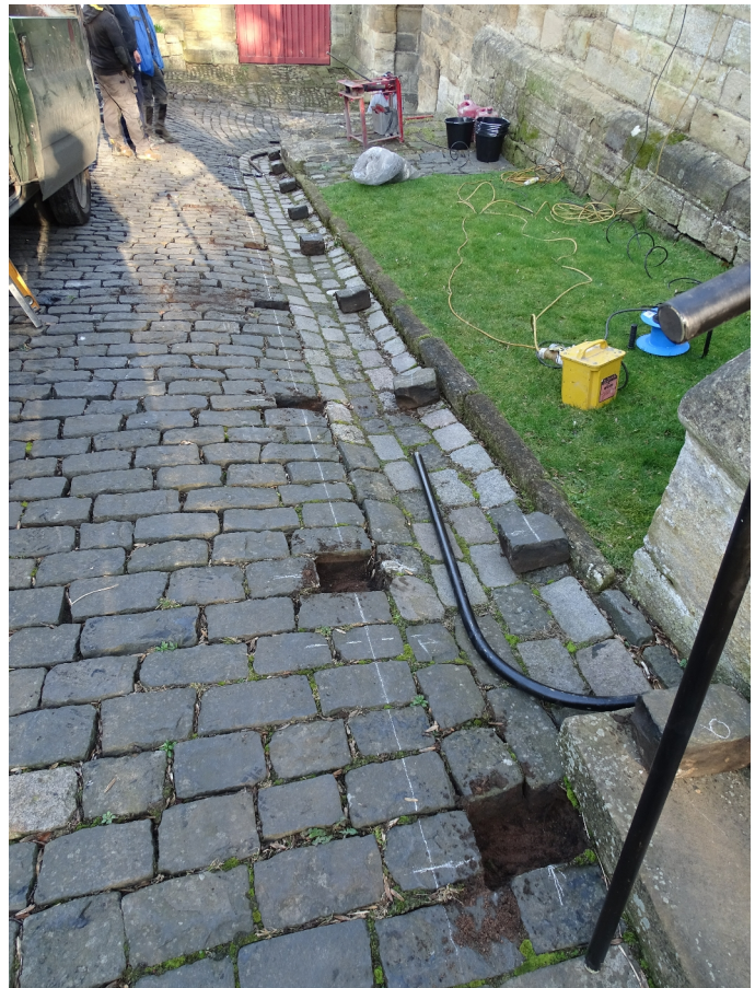
Plate 4 (above). The hand-dug post-holes along the verge, looking north.
