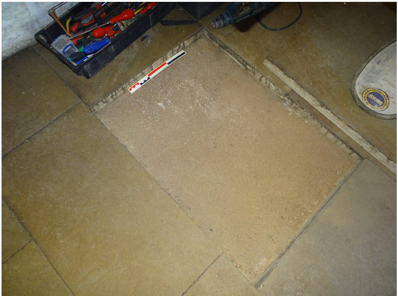
Plate 5 (below). One of the slab holes showing the packing sand).
