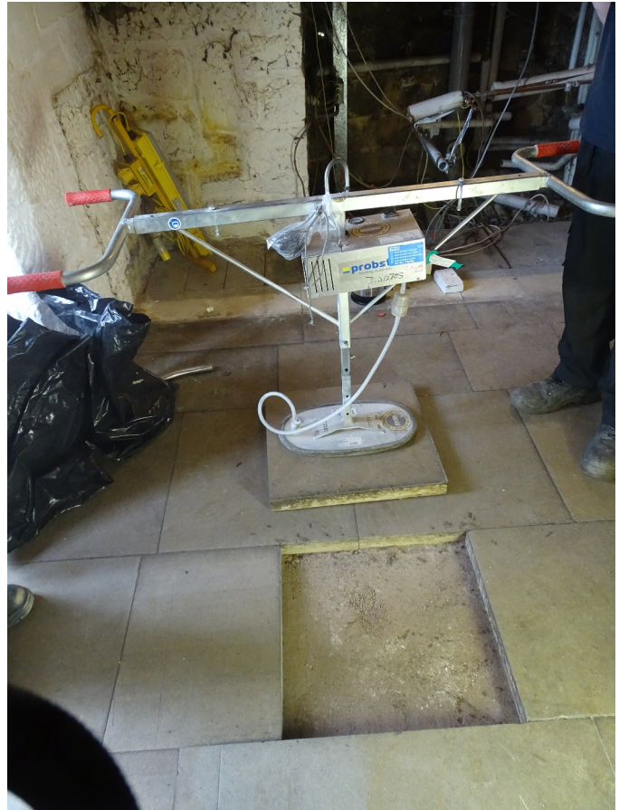
Plate 4 (right). Lifting a slab using suction to prevent the need to scrape and dig between slabs.
