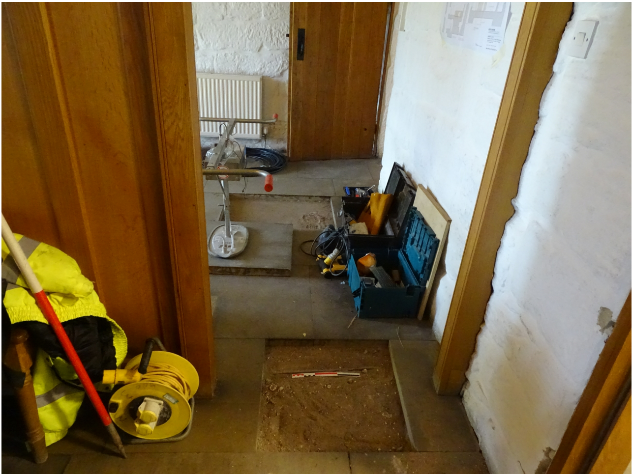
Plate 2. The new cable location in the foreground with a further lifted slab for levelling in the background, looking southeast.
