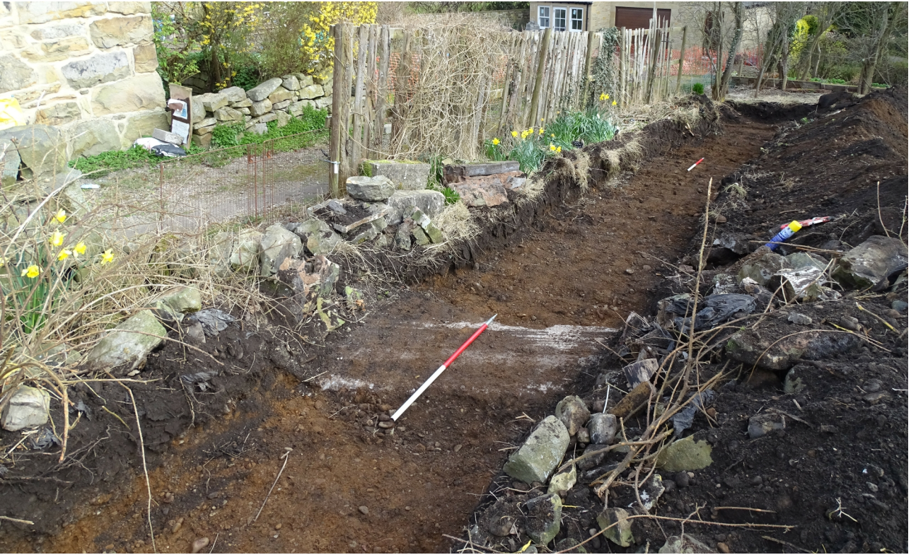
Plate 4 (above). The long arm of the trench looking north. The concrete foundation and remains of the drystone wall can be seen.
