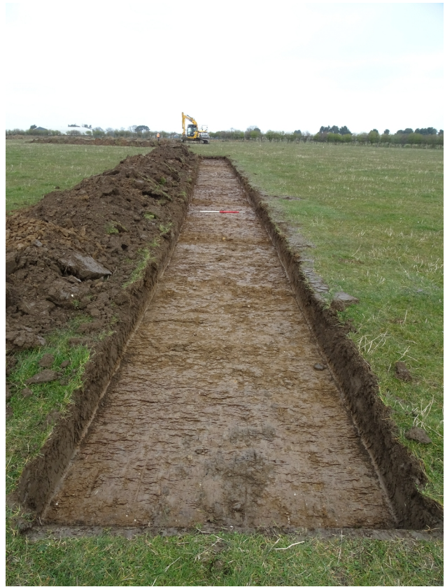
Plate 52. Trench 50 looking northeast
