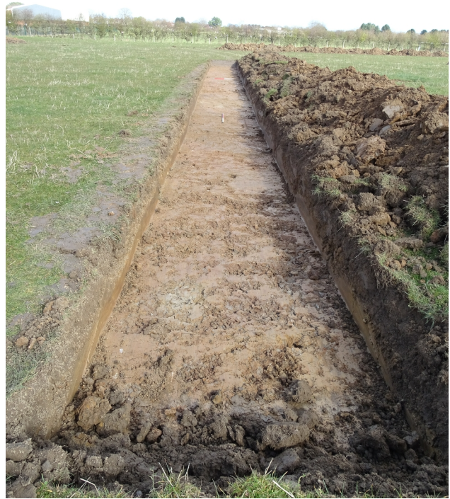
Plate 28. Trench 26 looking east
