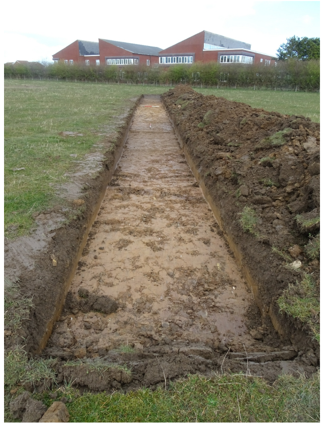
Plate 20. Trench 18 looking east
