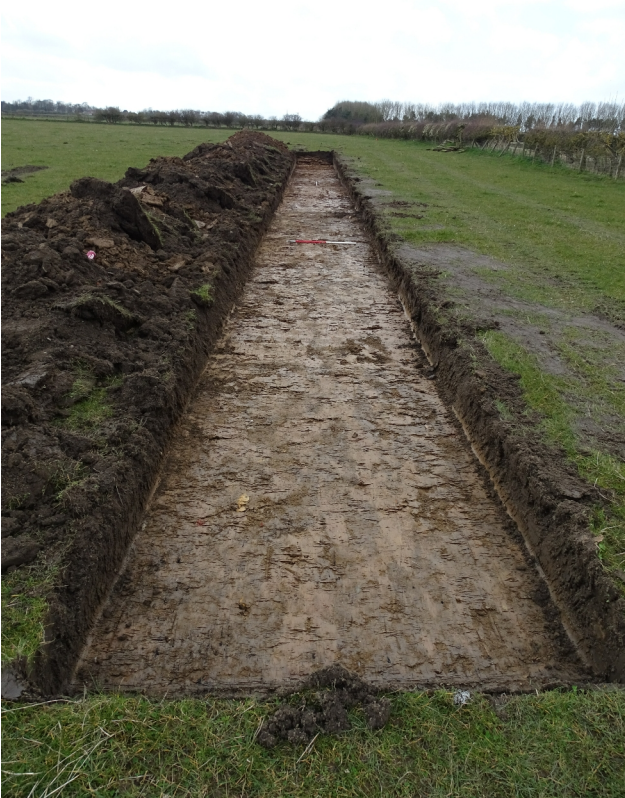
Plate 5. Trench 3 looking southwest
