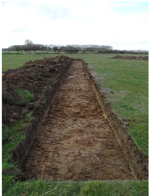
Plate 22. Trench 20 looking northwest
