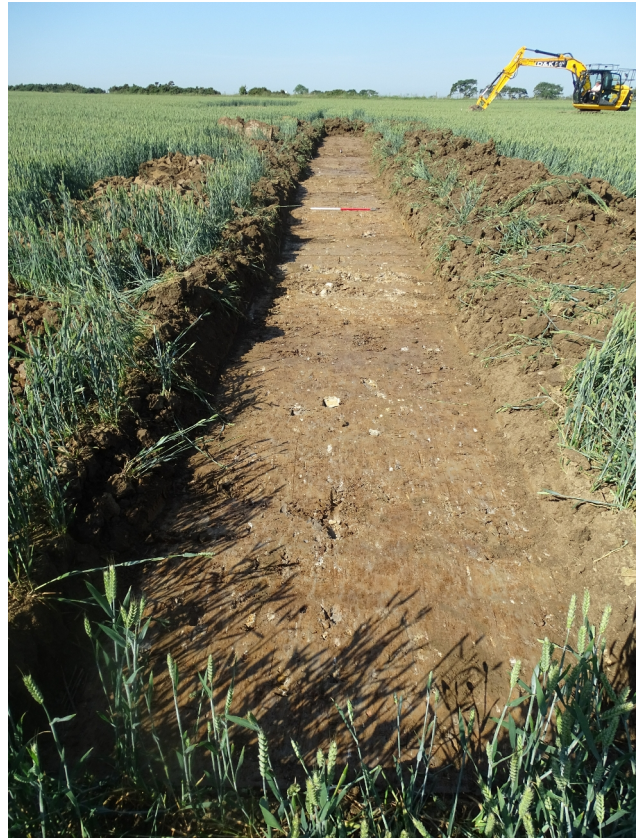
Plate 23. Trench 17 looking southwest.
