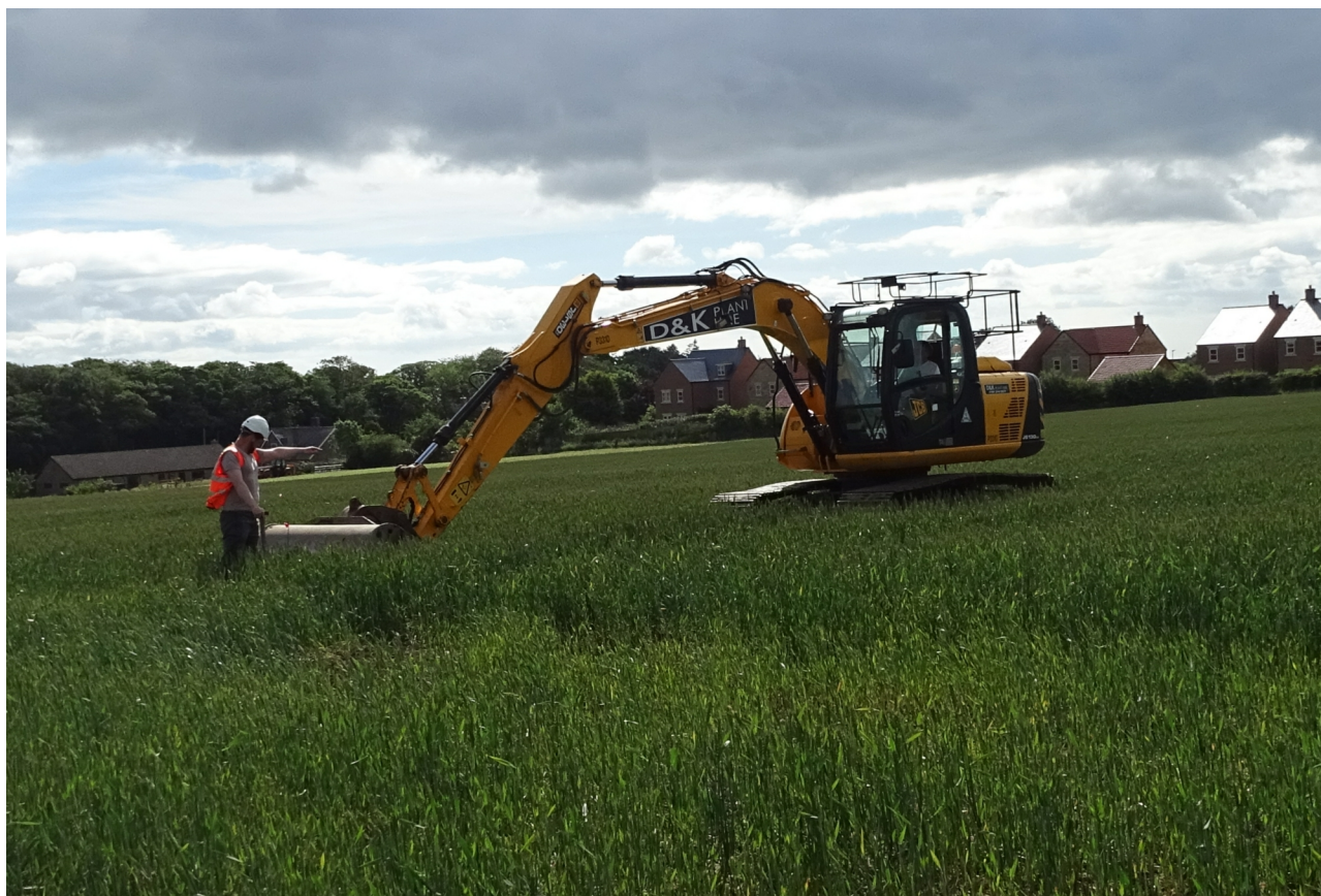
Plate 4. Trench excavations underway under constant archaeological supervision
