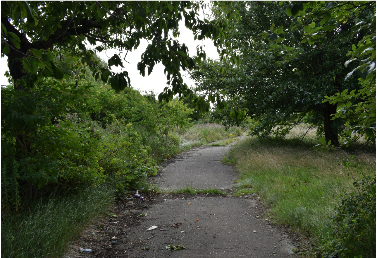
Plate 10. The main access road into the site, looking east.
