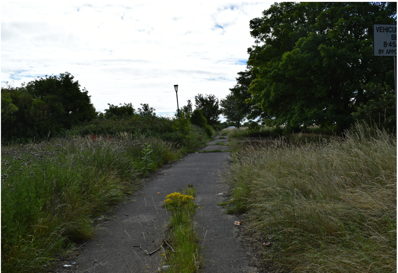
Plate 11. The main access road into the site, looking east.
