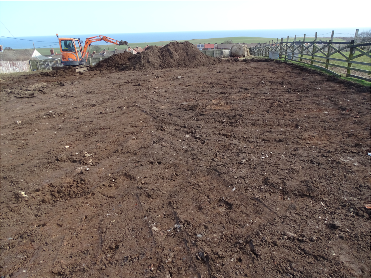
Plate 4. Observing the initial topsoil strip, looking east.
