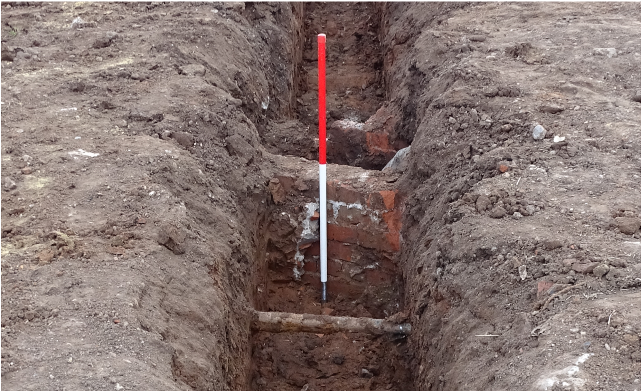
Plate 7. The conduit with Manhole A beyond, looking south.
